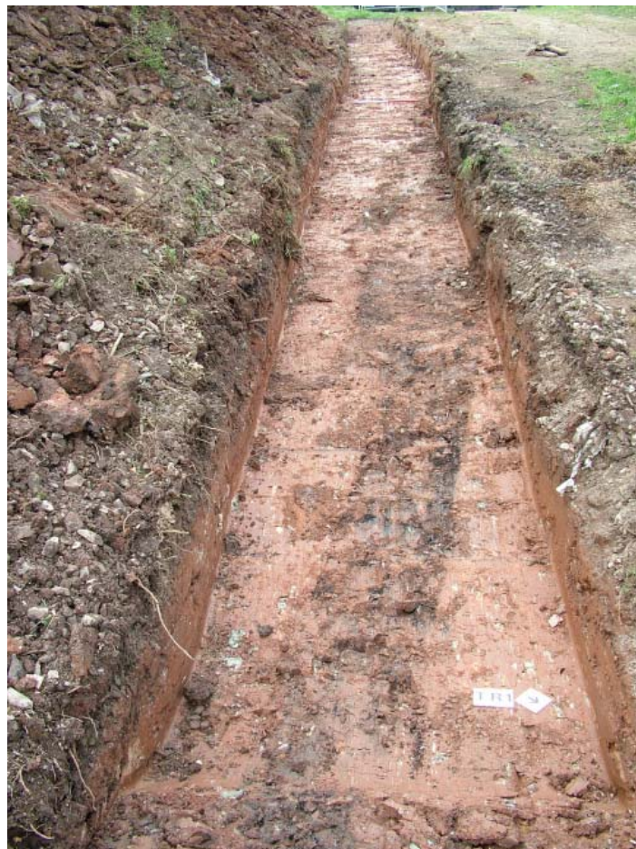
Plate 1: Trench 1 with sewer trench at north east end, looking south west
