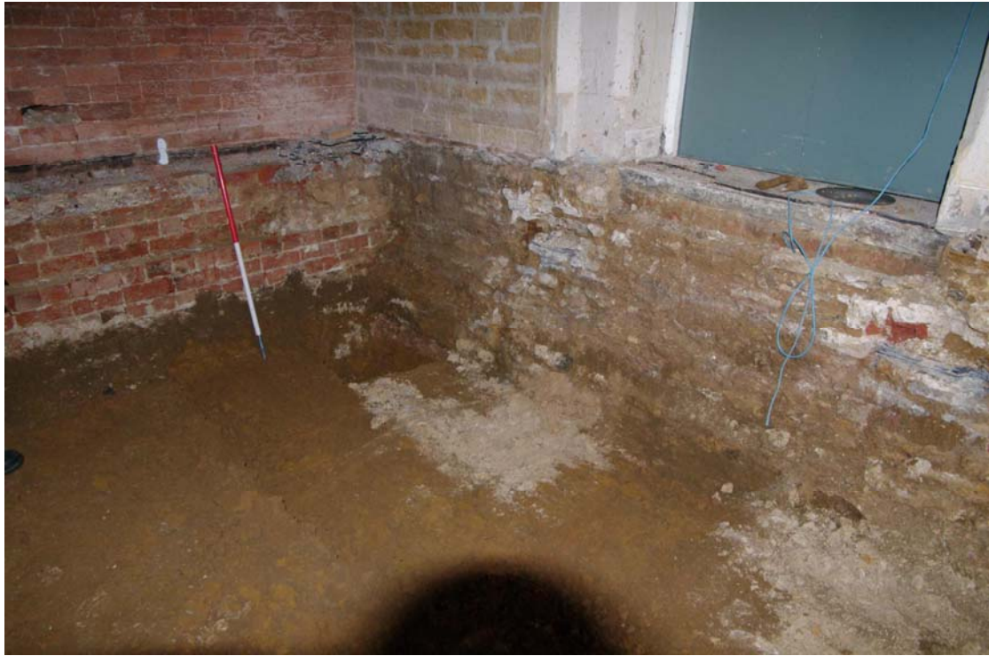
Figure 27: Reduced floor level in G.01. Looking north-east
