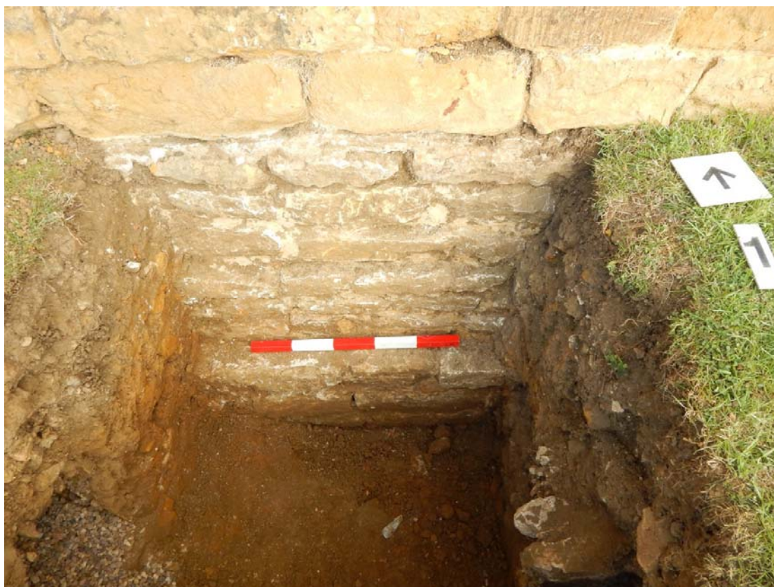
Figure 22: Test Pit 01, post excavation showing foundations (1)
