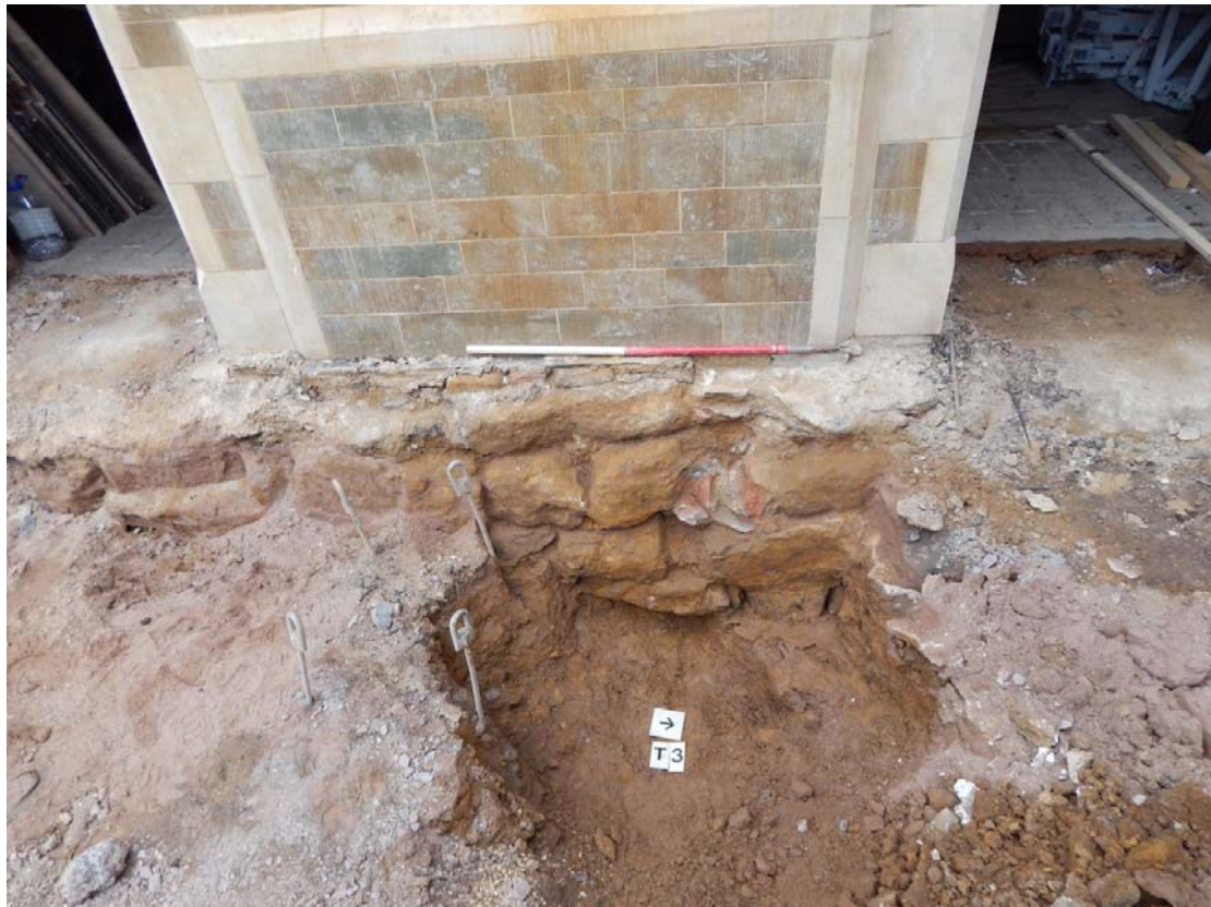
Figure 21: Test Pit 03, post excavation showing foundations (3)
