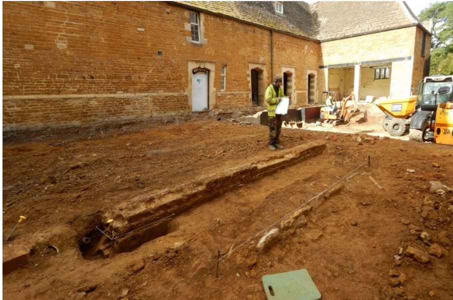
Figure 18: Work in progress on courtyard walls, looking north-west
