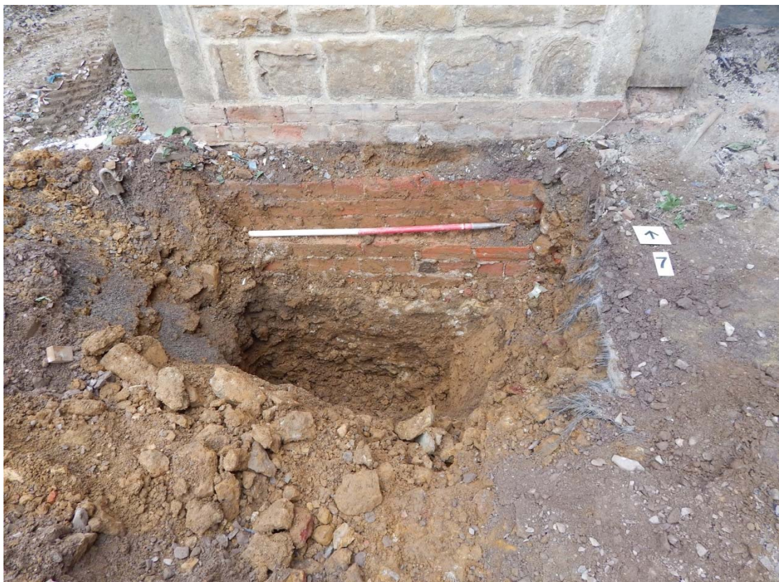
Figure 26: Test Pit 07, post excavation showing brick foundations
