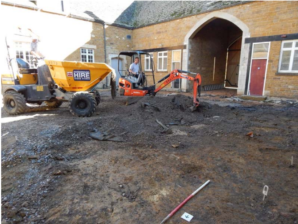
Figure 13: Work in progress, looking south-east, note anchor points in foreground
