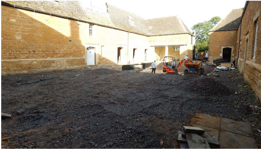
Figure 12: The courtyard area during removal of mill waste, looking north-west
