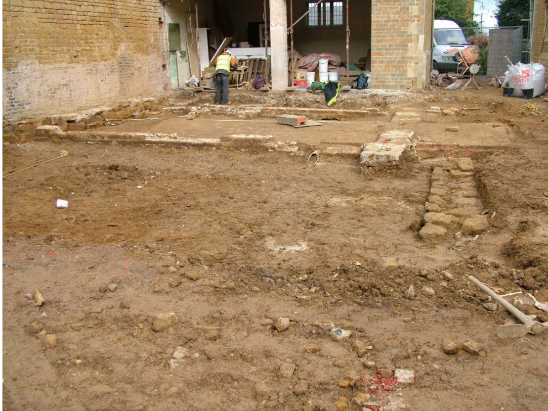
Figure 7: Work in progress on northern end of courtyard from 2005-6, looking north-west
