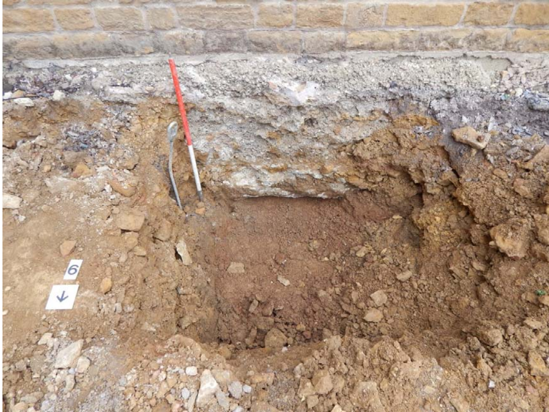
Figure 24: Test Pit 06, post excavation showing concrete underpinning
