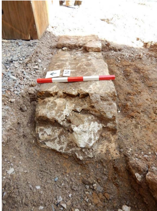
Figure 14: Western end of wall (2) revealed during courtyard strip. Previously recorded as (25), looking east
