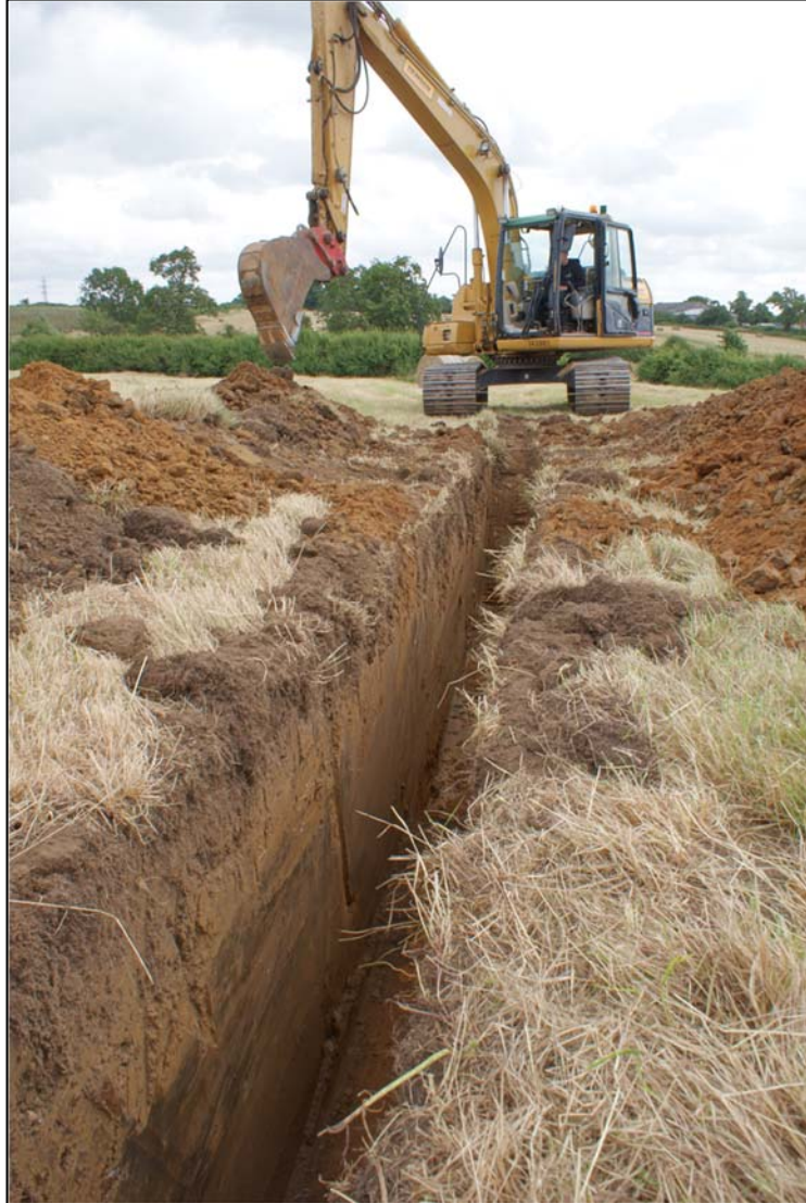
Figure 7. Cable trenching looking south east.
