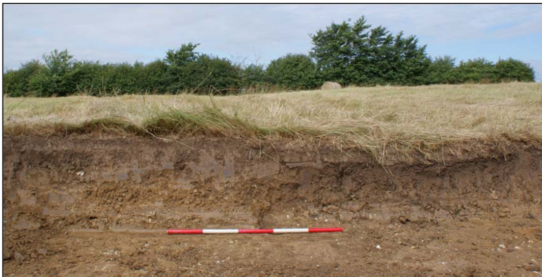
Figure 6. Photograph showing the eastern half of turbine base stripped and underlying geology (above) and trench section showing effect of ridge and furrow (below).
