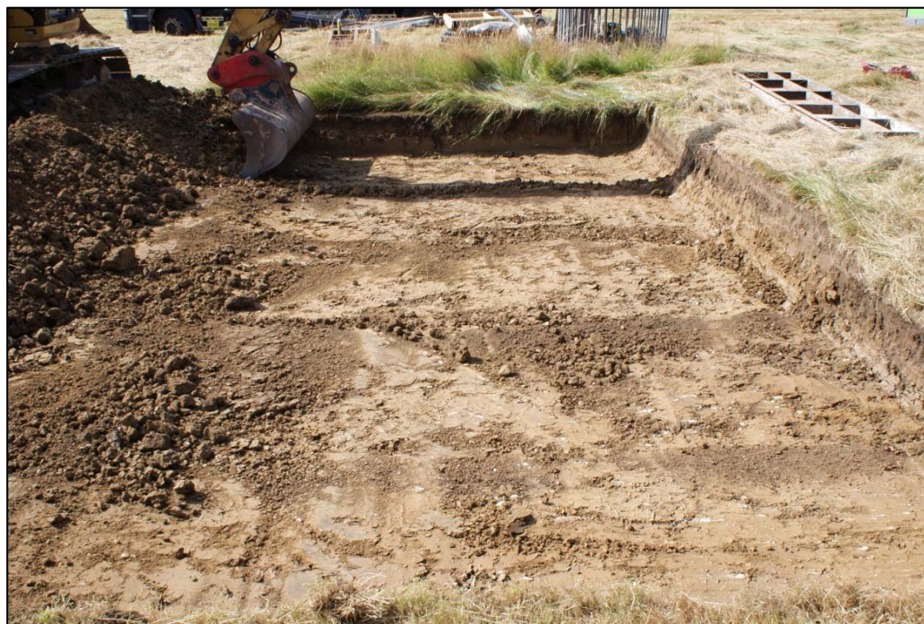
Figure 5. Stripping of western half of turbine base. Looking south.
