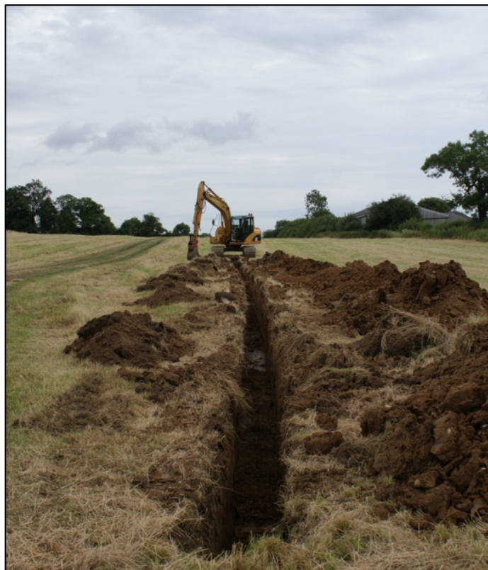
Figure 9. Trenching of Length C. Looking East.
