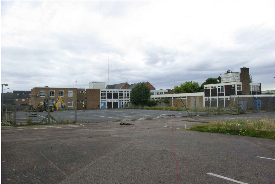
Figure 4 Rear of site Looking north-west
