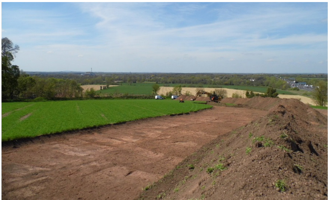
Figure 8 Stripping in progress. Looking North
