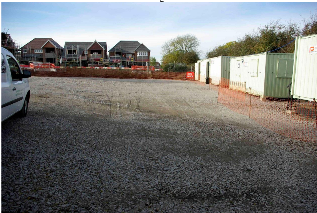
Figure 22 North-west corner of site and site car park Looking west
