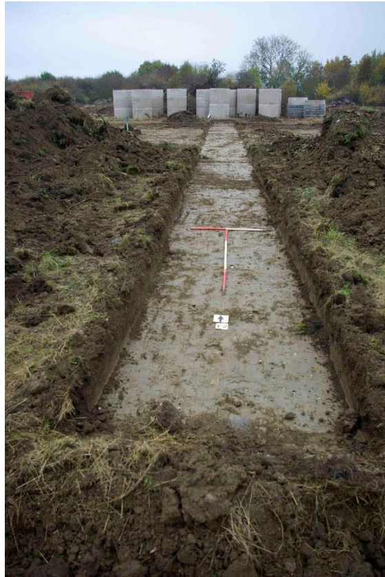
Figure 5 Trench 2 Looking north
