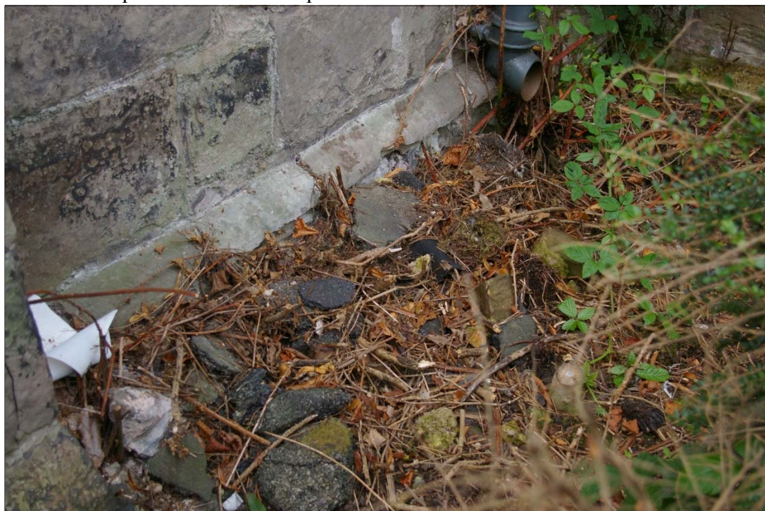
Figure 7: East wall of porch prior to excavation
