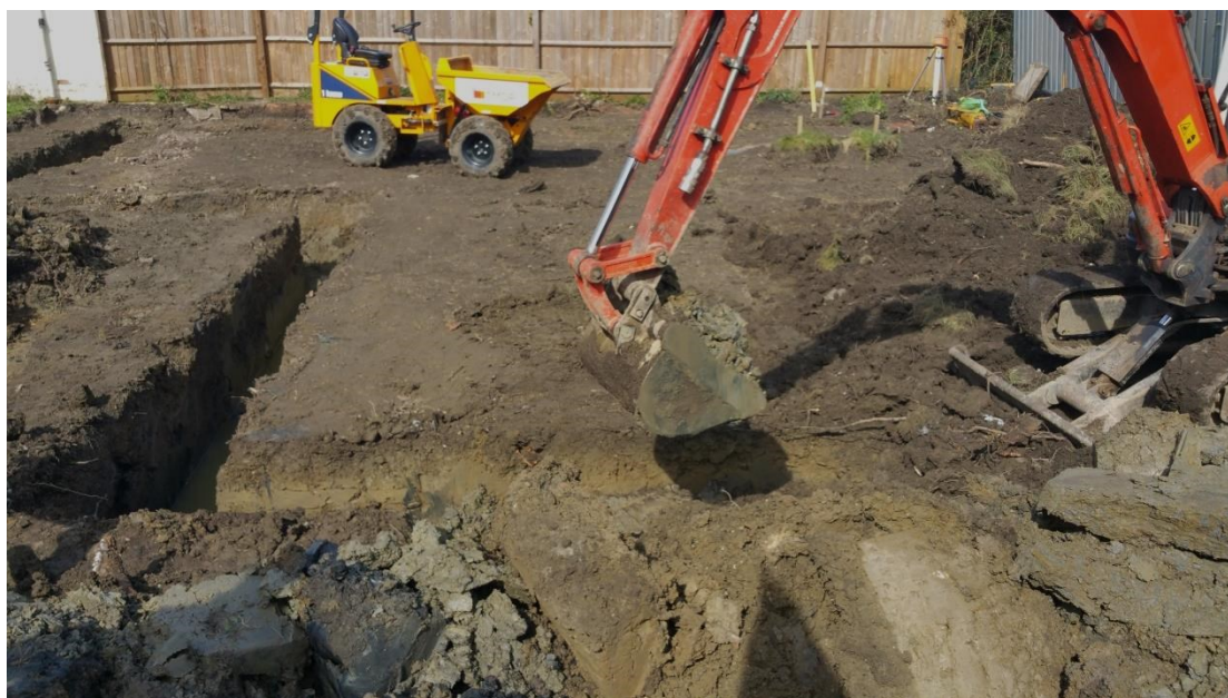
Figure 4: Groundworks in progress; general view south-west across site
