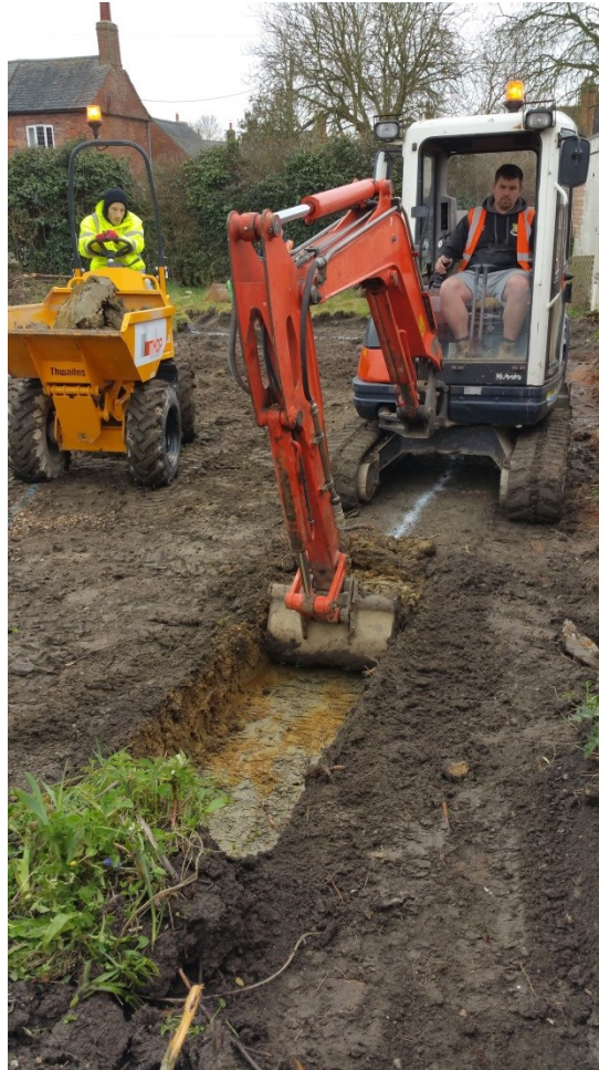
Figure 5: Excavation on the Middle Street frontage; view north
