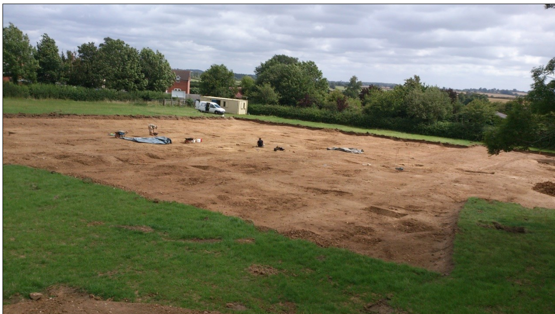
Figure 8: Area of excavation, looking north-east
