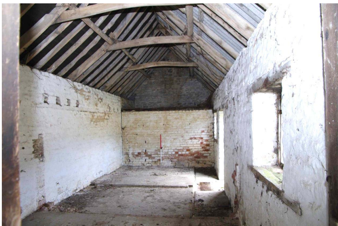
Figure 97: South range, west end inside Looking west, 1m scale
