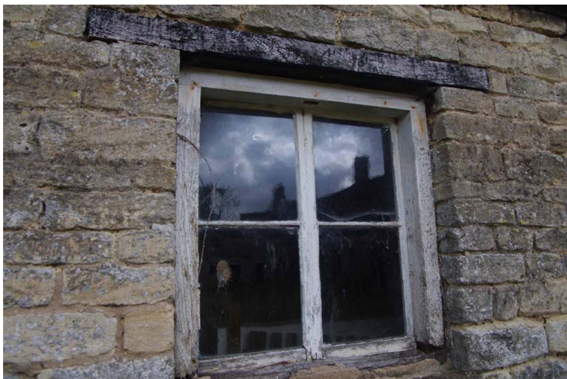
Figure 88: East range, Building E window detail Looking south-west. Note pegged frame and mortice hole at top of frame and chamfered lintel
