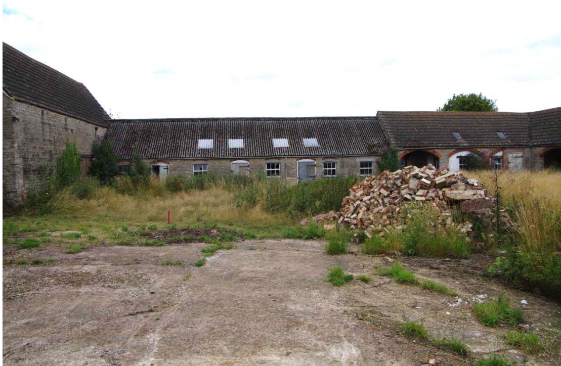
Figure 70: North range, south facing elevation Looking north
