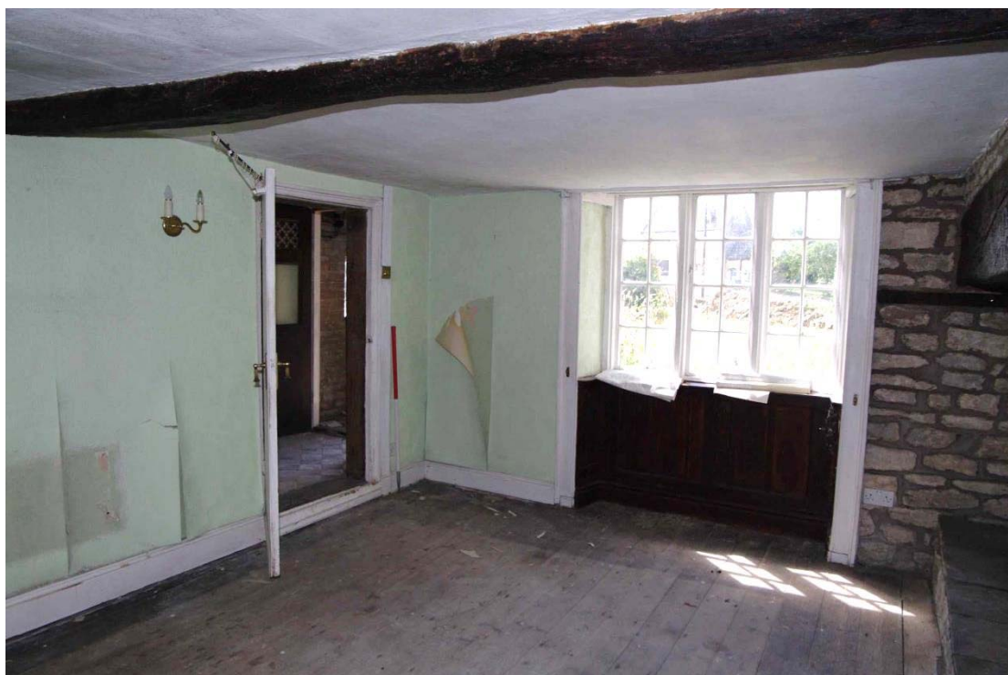
Figure 22: Ground floor, Room G1 Looking south-west, 1m scale
