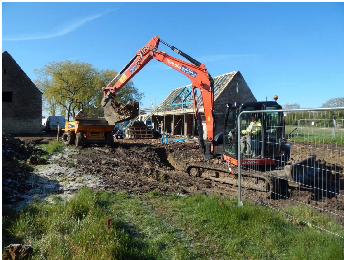
Figure 140: Work in progress on Unit 3, Building H, looking south
