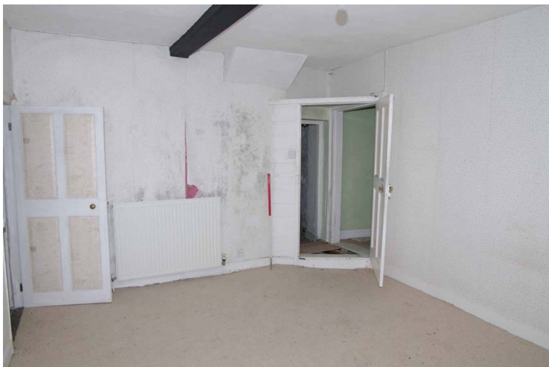
Figure 42: First floor, Room F1 Looking north-east, 1m scale
