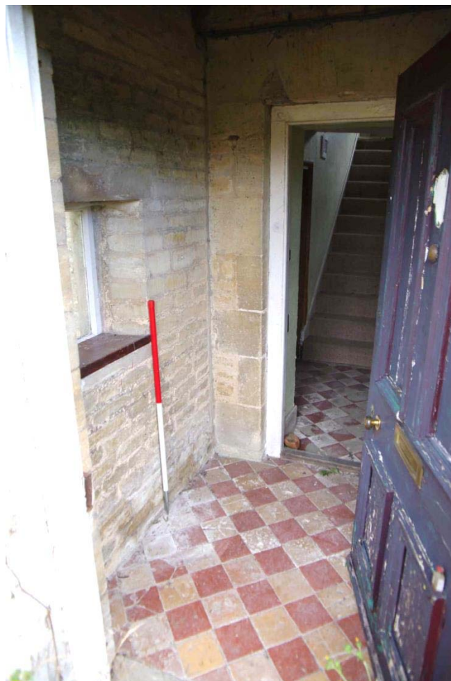
Figure 21: Porch and hall floors Looking north-west, 1m scale
