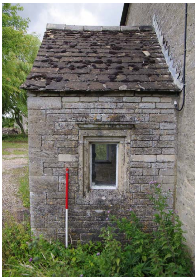
Figure 12: South facing elevation of porch Looking north, 1m scale
