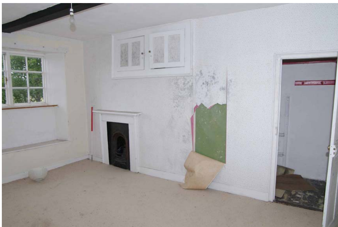
Figure 41: First floor, Room F1 Looking north-west, 1m scale
