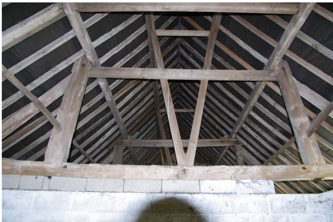
Figure 130: Cart shed (Building H), roof detail Looking north
