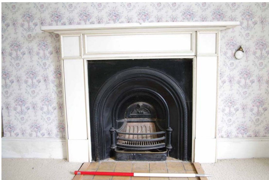
Figure 54: First floor, Room F5. Fireplace Looking west, 1m scale. Note bell pull to right of fireplace
