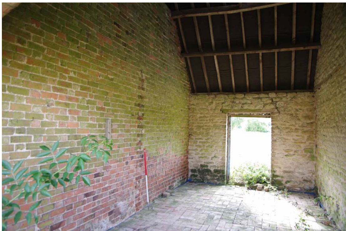
Figure 129: Cart shed (Building H), north end Looking west, 1m scale
