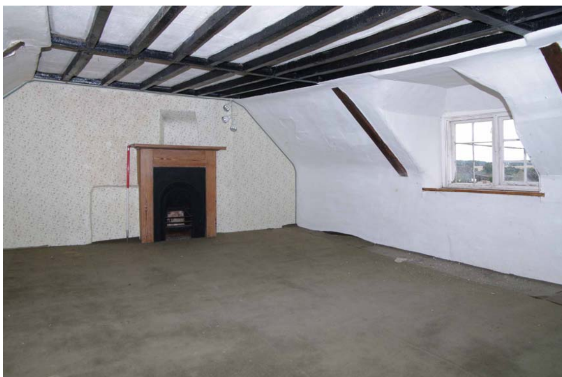
Figure 64: Second floor, Room S4 Looking south-west, 1m scale
