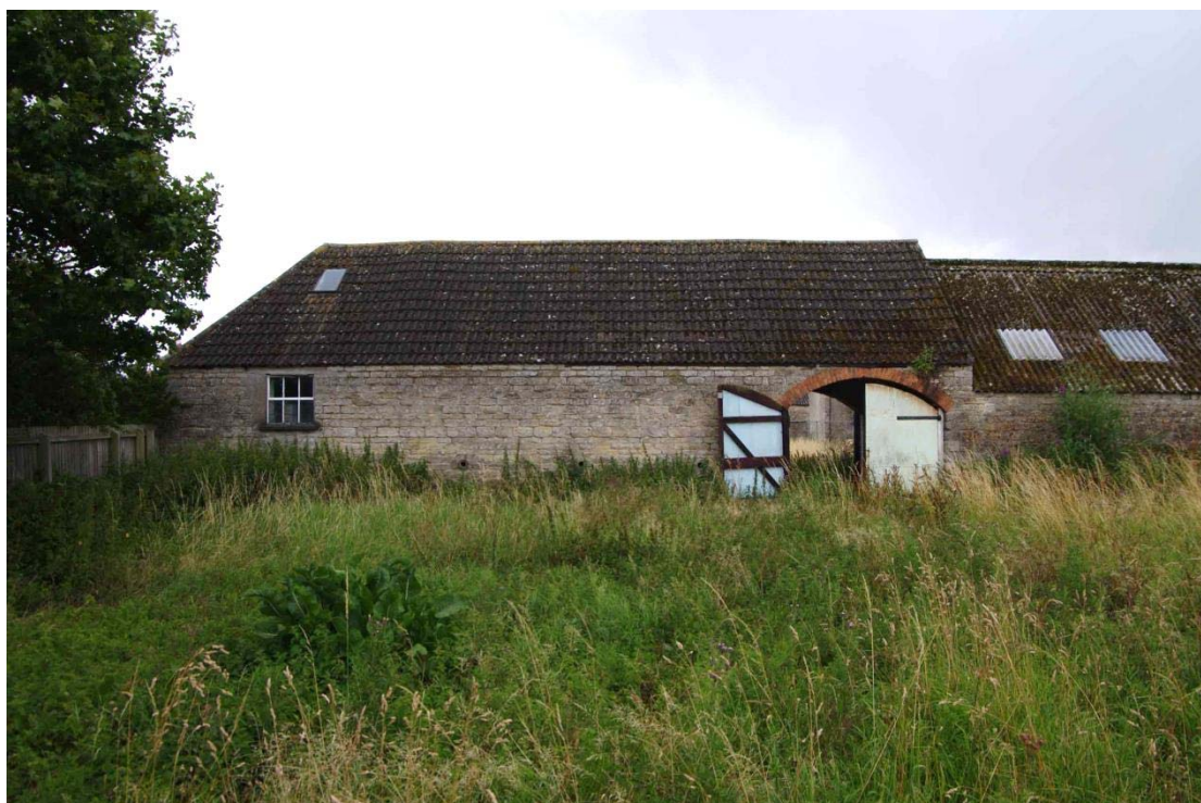
Figure 78: North range, north facing elevation, Building C Looking south
