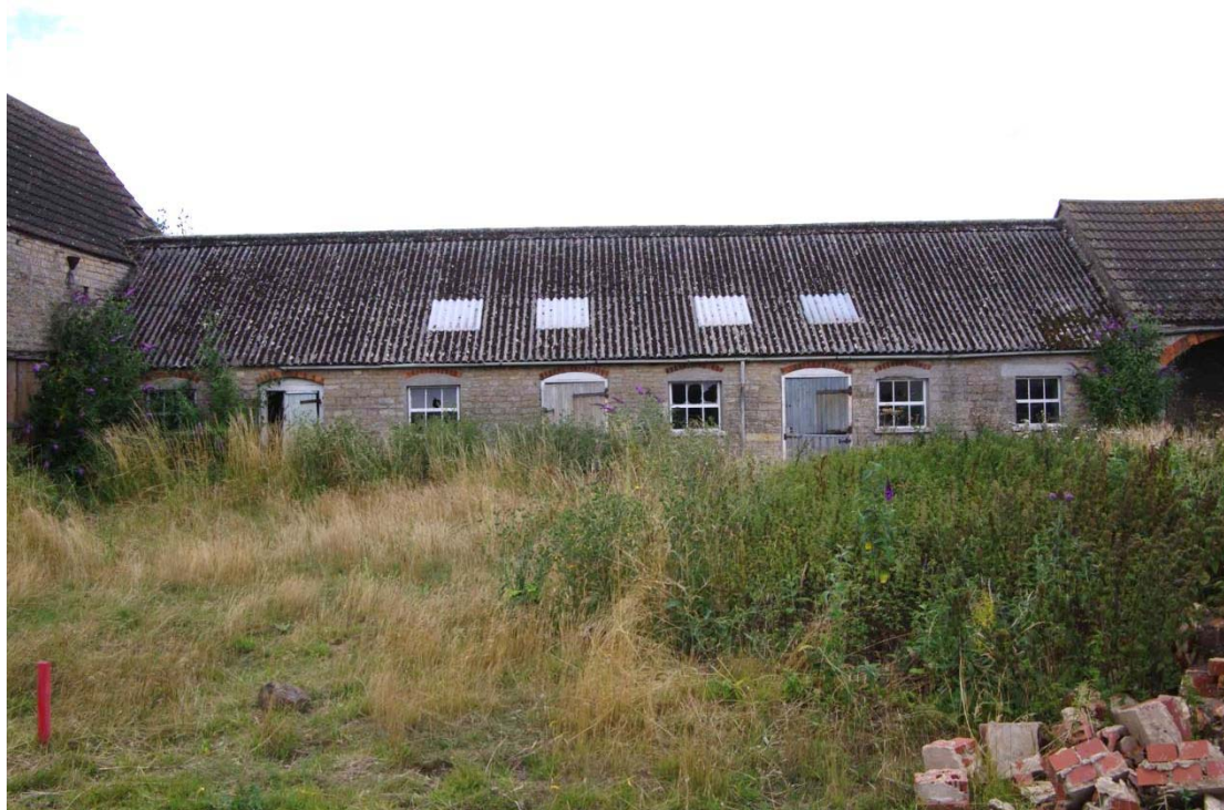
Figure 71: North range, western half of south facing elevation Looking north
