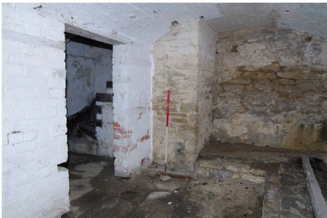
Figure 39: Cellar, north room Looking south-west, 1m scale
