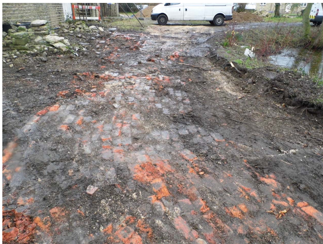
Figure 132: Stripped eastern arm of driveway, looking south
