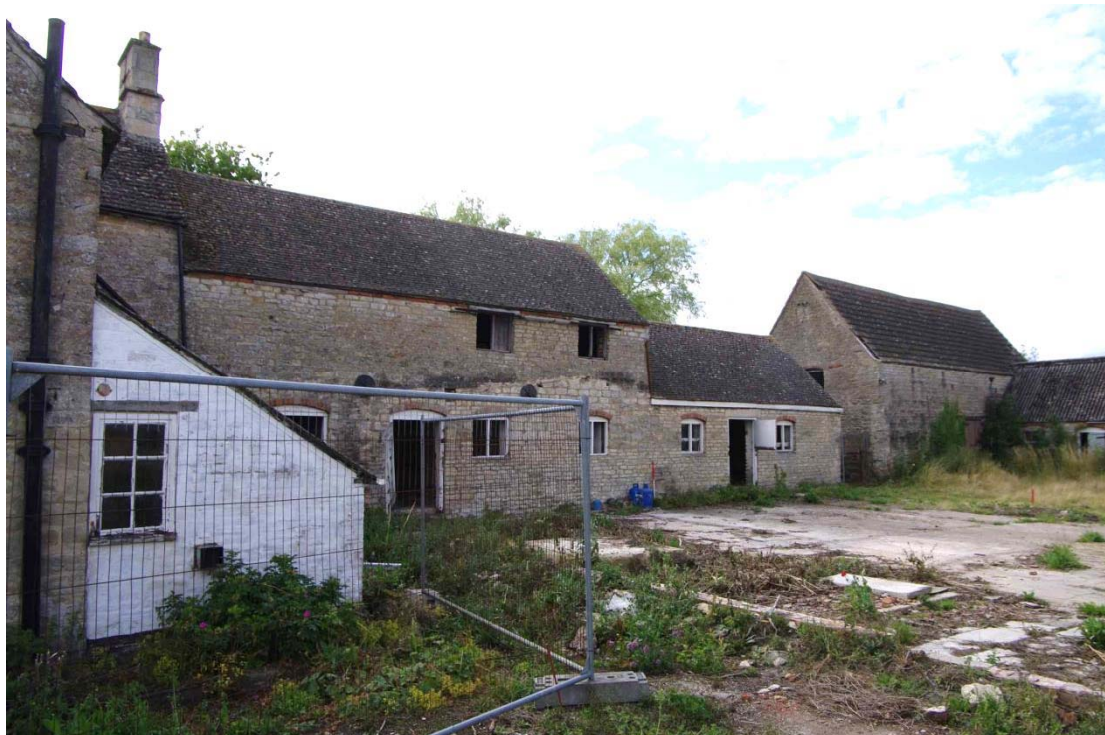
Figure 103: West range, east facing elevation Looking north-west, 1m scale
