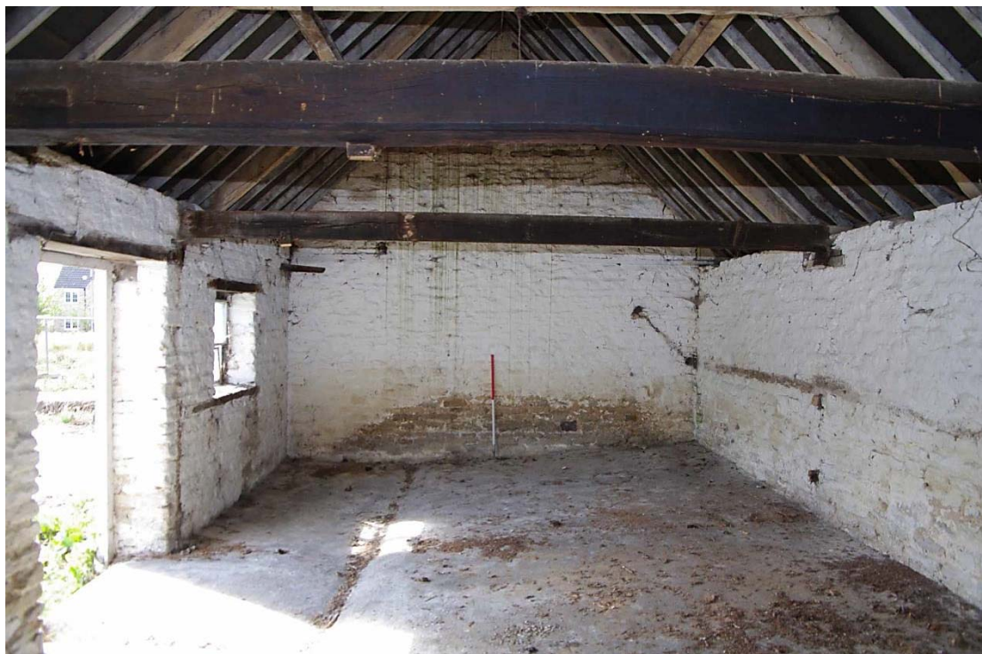
Figure 120: West range, north end of Building G Looking south, 1m scale. Note marks in paint showing position of byre on right
