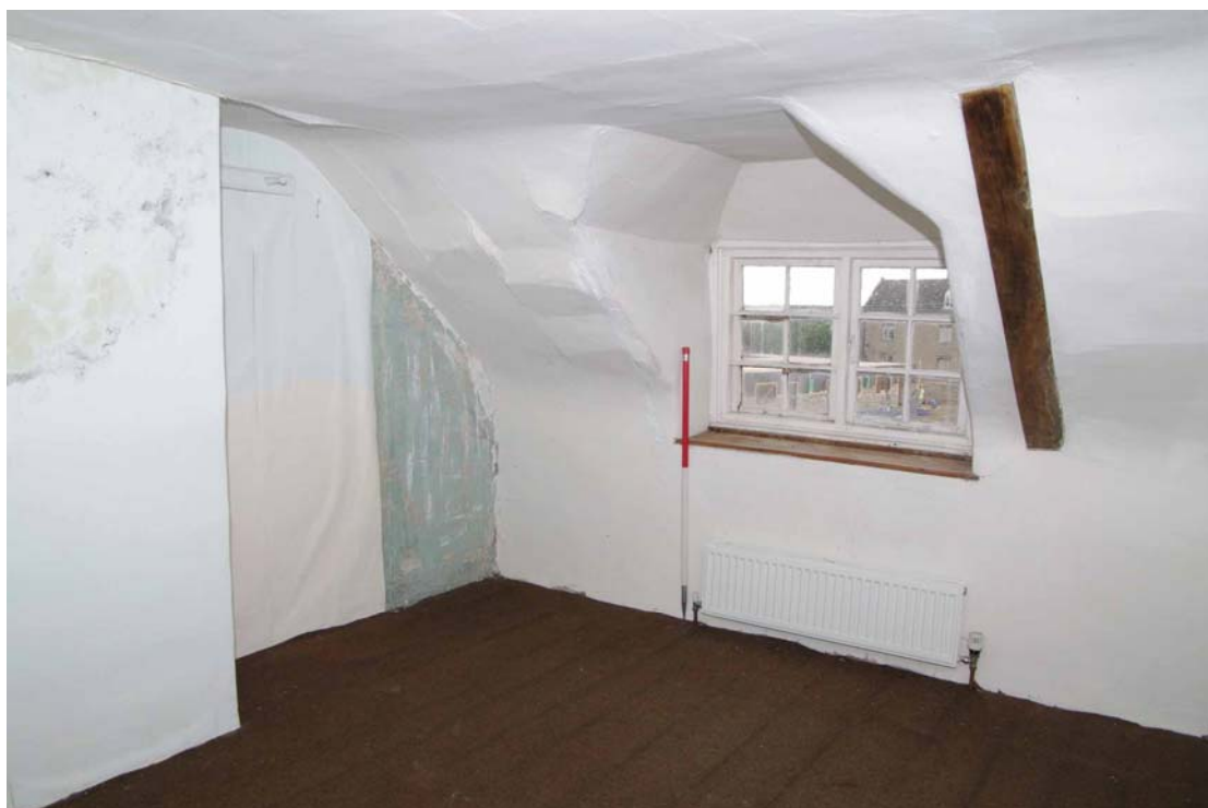
Figure 63: Second floor, Room S3 Looking south-west, 1m scale
