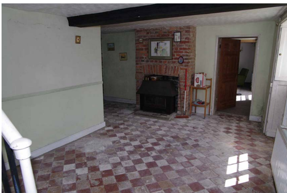
Figure 27: Ground floor, Room G2. Hall Looking south-east, 1m scale. Note inserted pantry on left of picture
