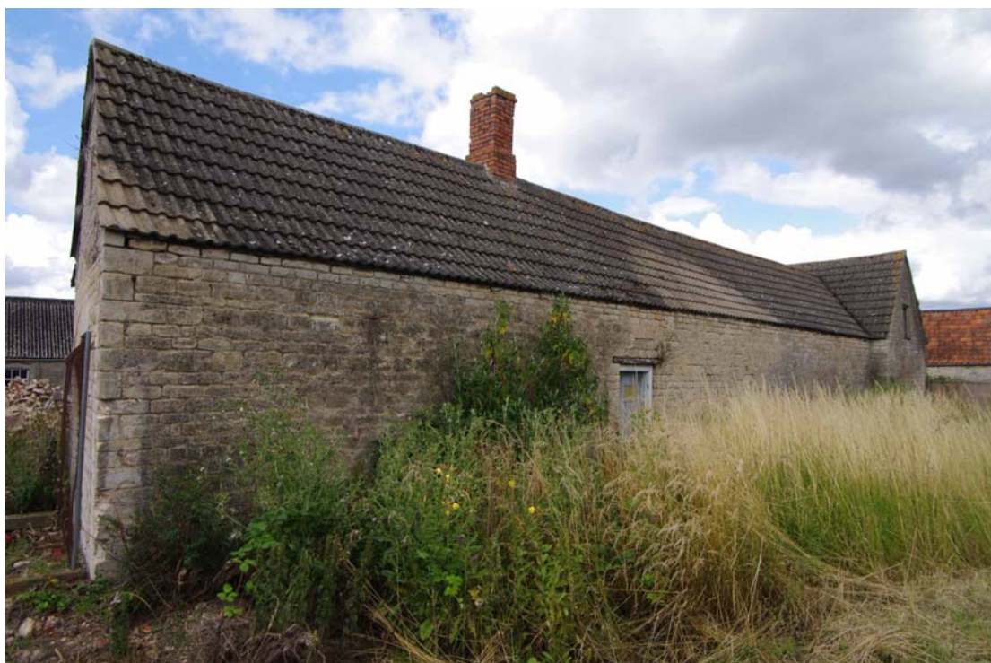
Figure 95: South range south facing elevation Looking north-east. Note slight projection of the east range gable at the right of the picture
