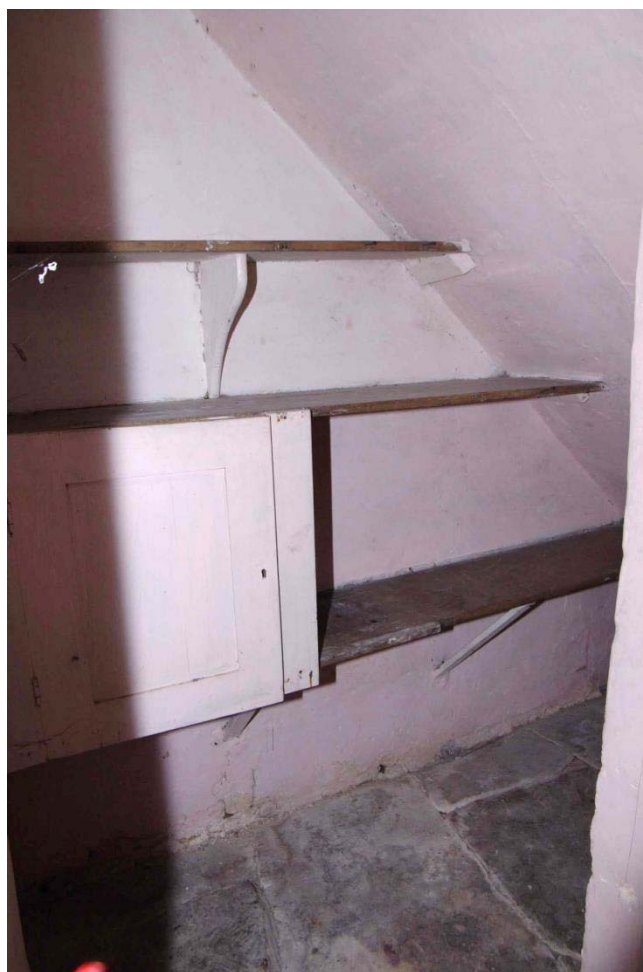
Figure 24: Ground floor, Room G1. Pantry below stairs Looking south-west
