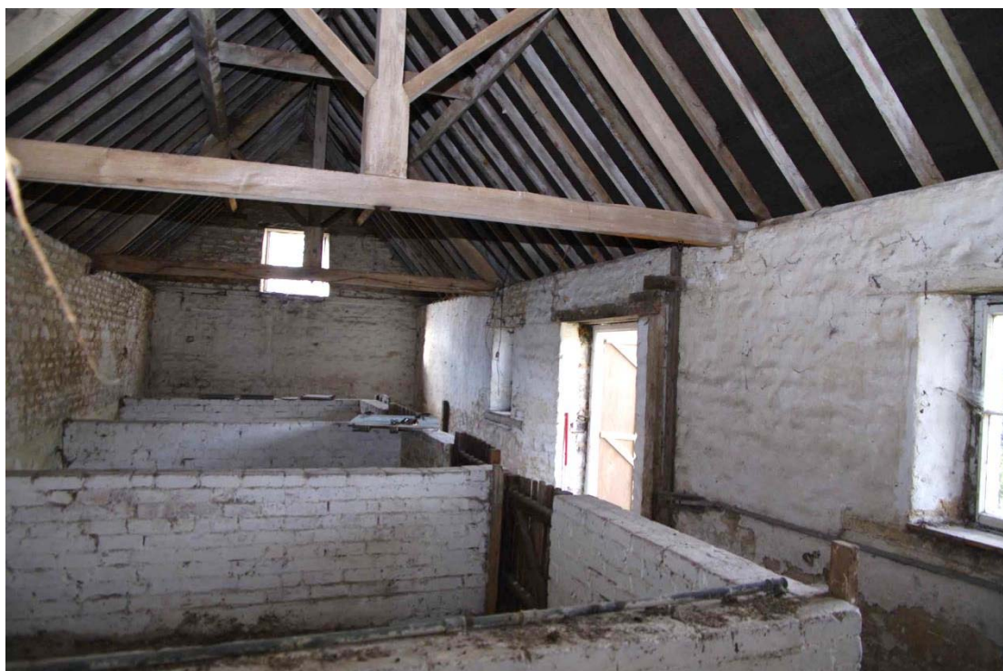
Figure 90: East range, Building E inside Looking south-west, 1m scale
