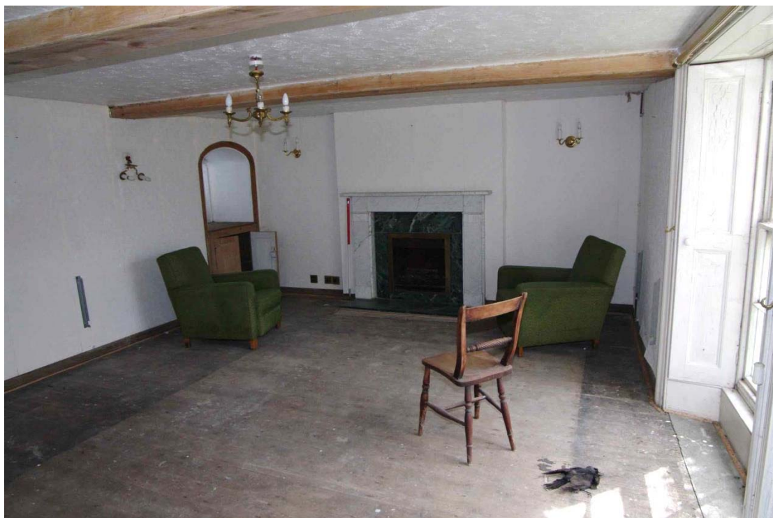
Figure 28: Ground floor, Room G3 Looking south-east, 1m scale
