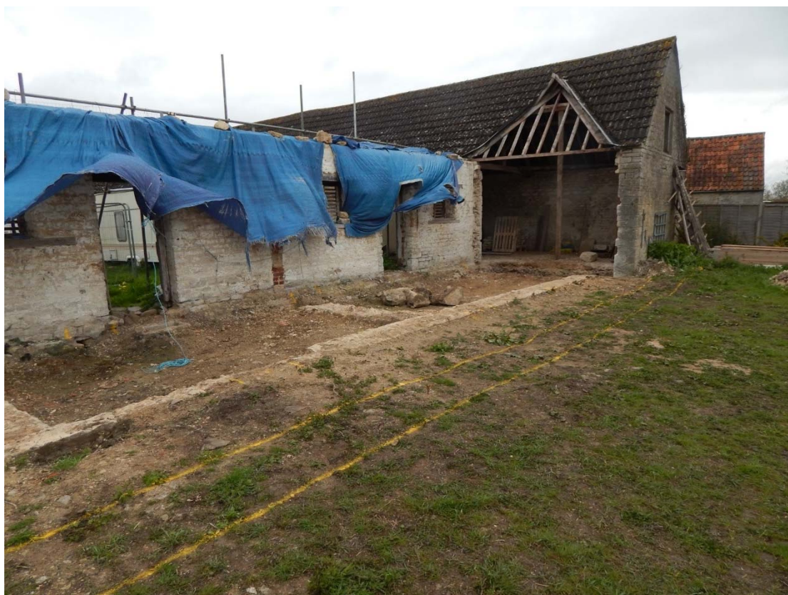
Figure 136: Post excavation view of Buildings E & F (Unit 1), looking east north-east
