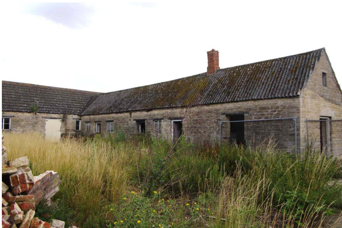
Figure 92: South range, north facing elevation Looking south-east
