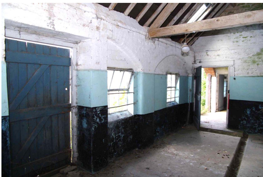
Figure 80: North range, Building C inside Looking south-west, 1m scale
