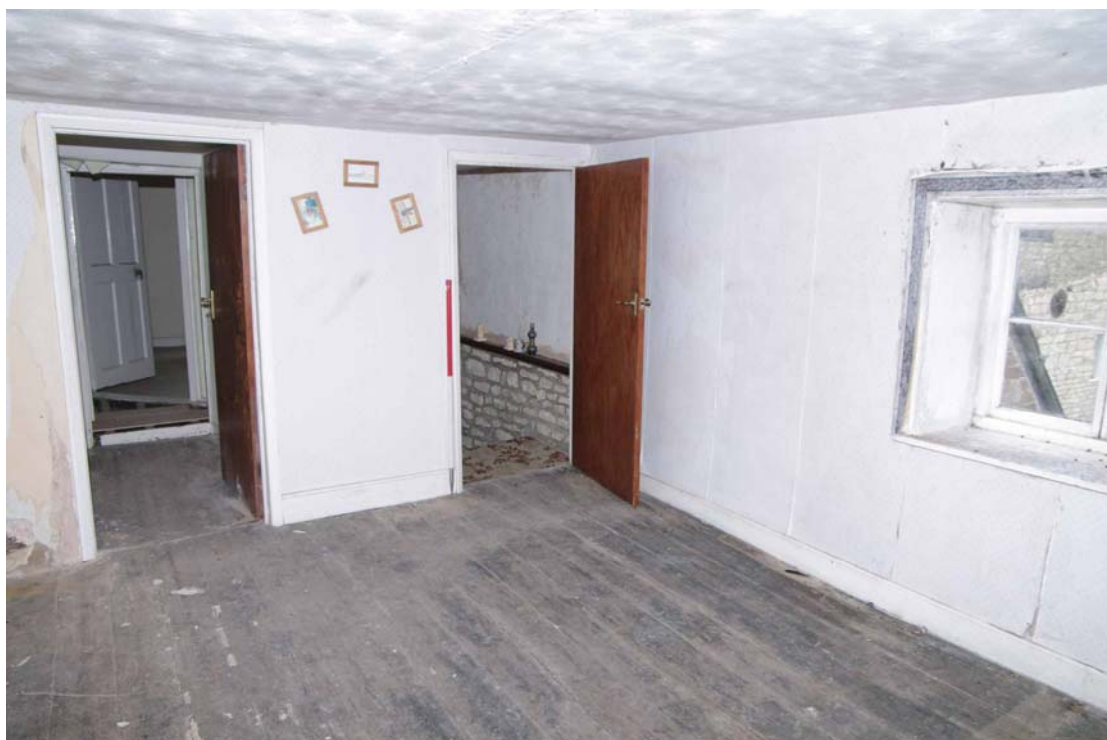
Figure 48: First floor, Room F3 Looking north-west, 1m scale
