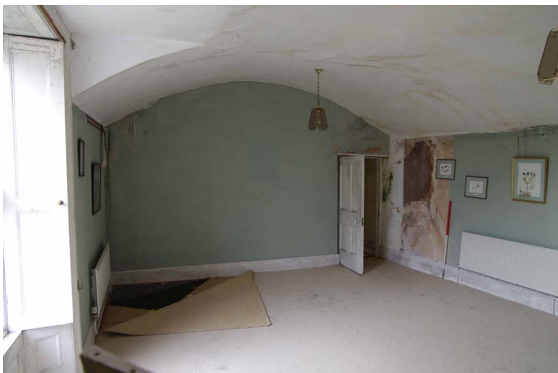
Figure 53: First floor, Room F5 Looking north-west, 1m scale
