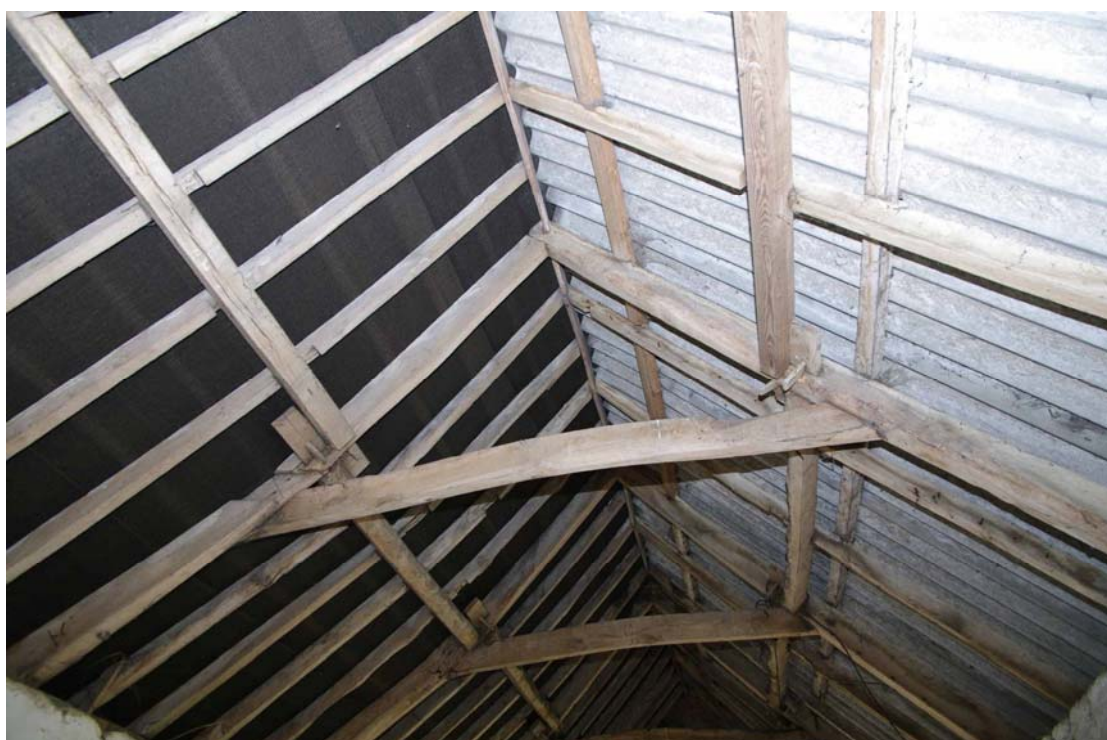
Figure 99: South range, west end roof detail
