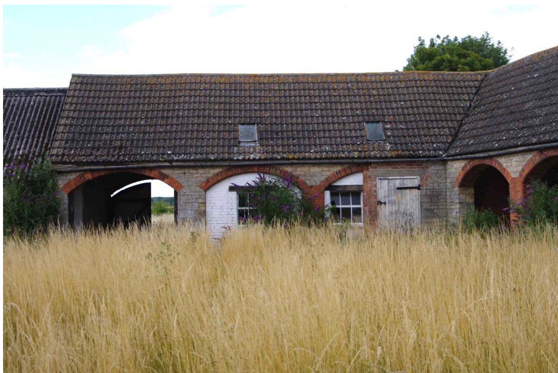
Figure 77: North range south facing elevation, Building C Looking north
