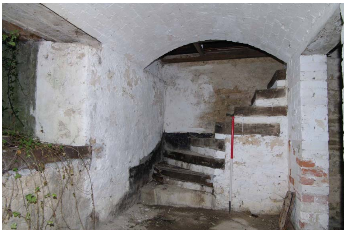
Figure 38: Cellar, south room Looking west, 1m scale
