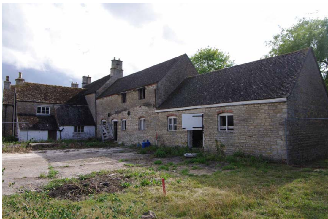
Figure 115: West range, east facing elevation of Building G Looking south-west towards house
