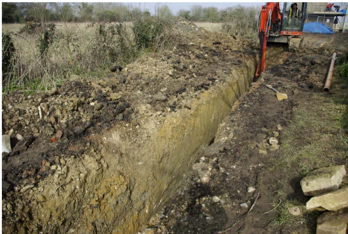
Figure 134: Partially finished trench, looking north north-west
