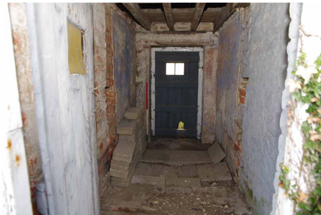
Figure 100: South range corridor Looking south, 1m scale
