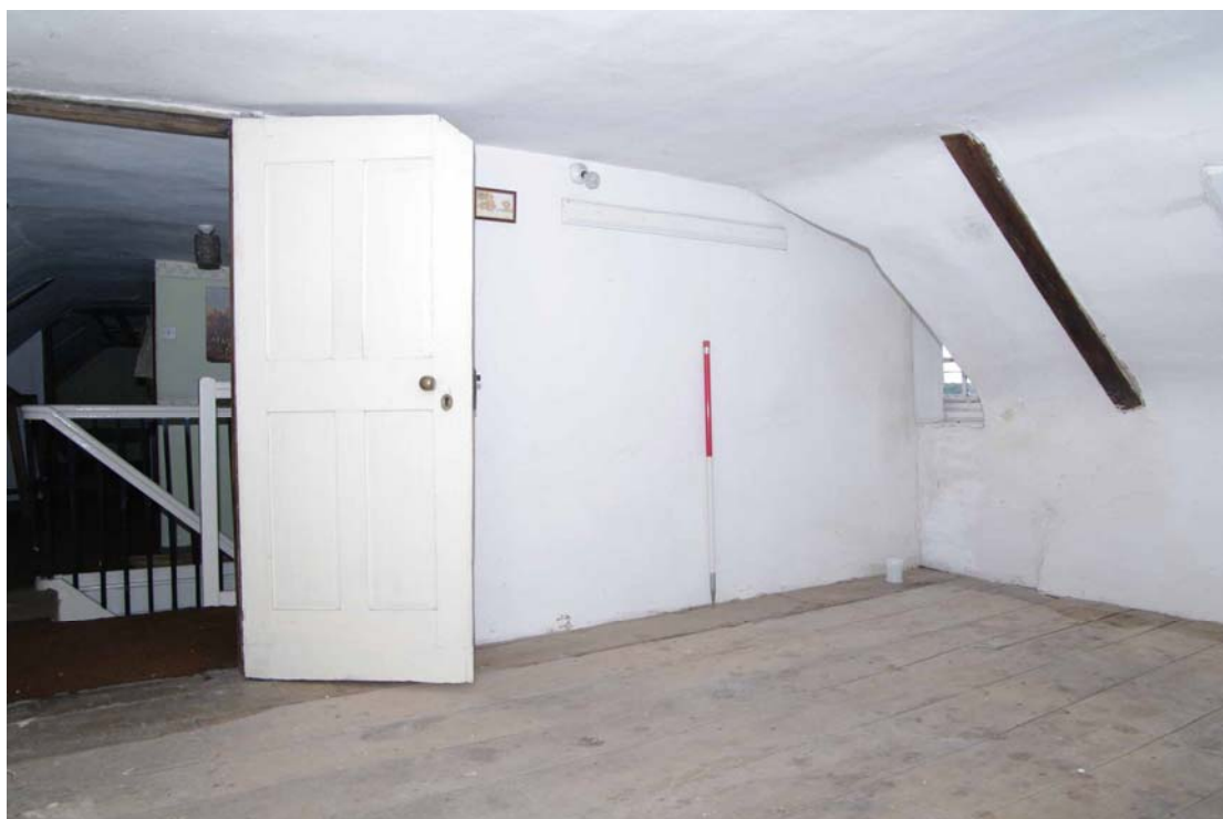
Figure 58: Second floor, Room S1
