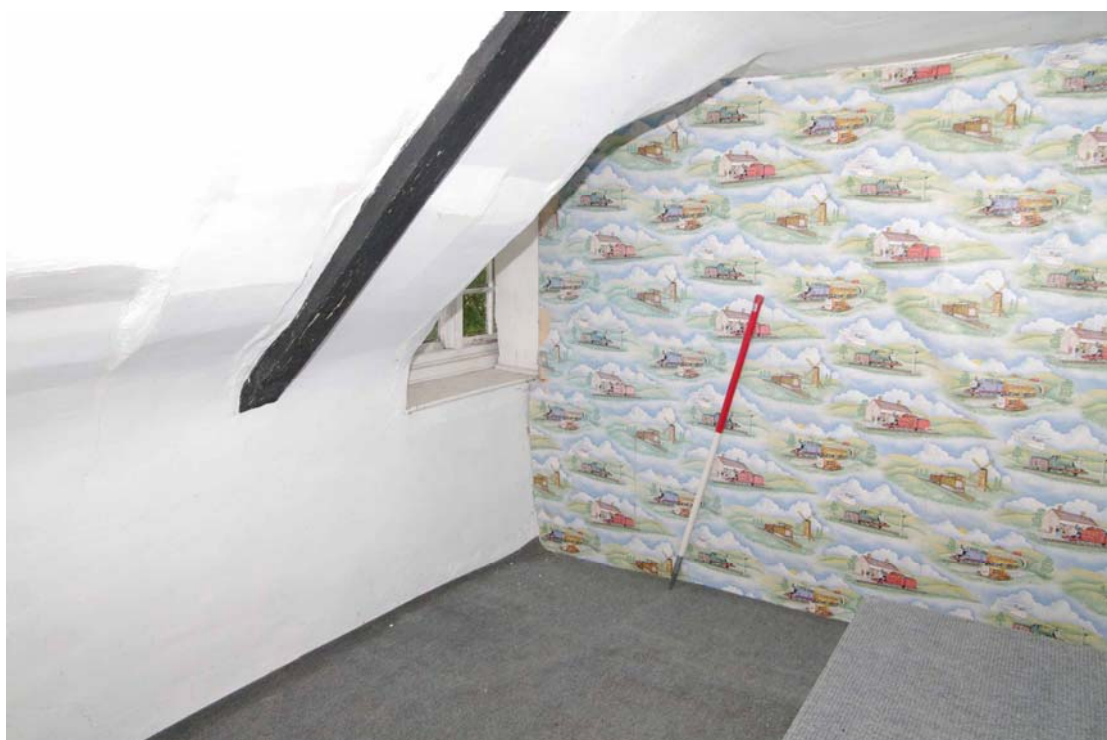
Figure 60: Second floor, Room S2 Looking north-west, 1m scale
