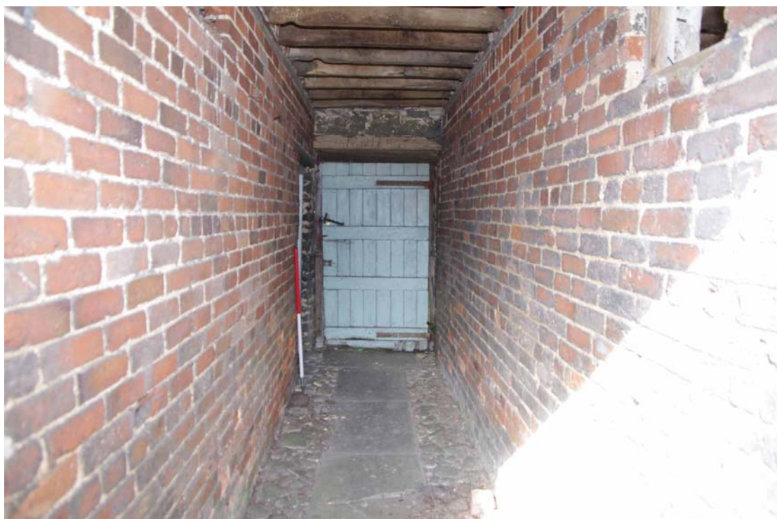
Figure 116: West range, passageway through Building G Looking west, 1m scale. Entrance to the coal store and north end wall of house just behind the 1m scale
