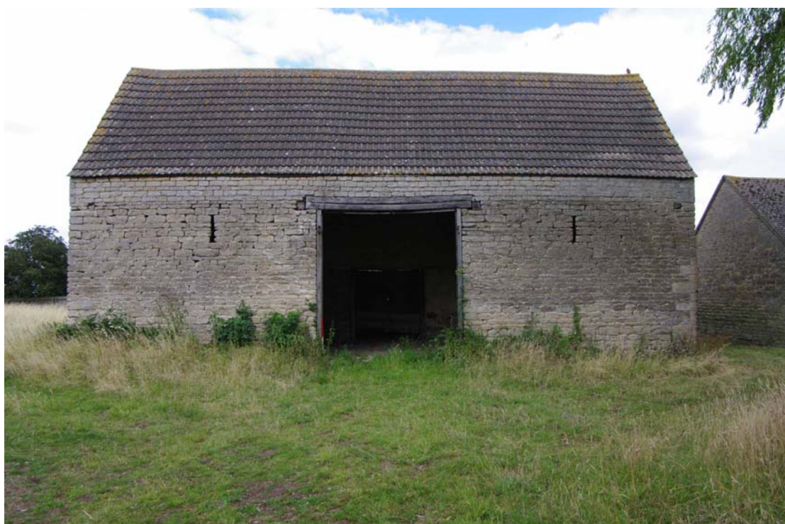
Figure 106: West range, west facing elevation of Building A Looking east
