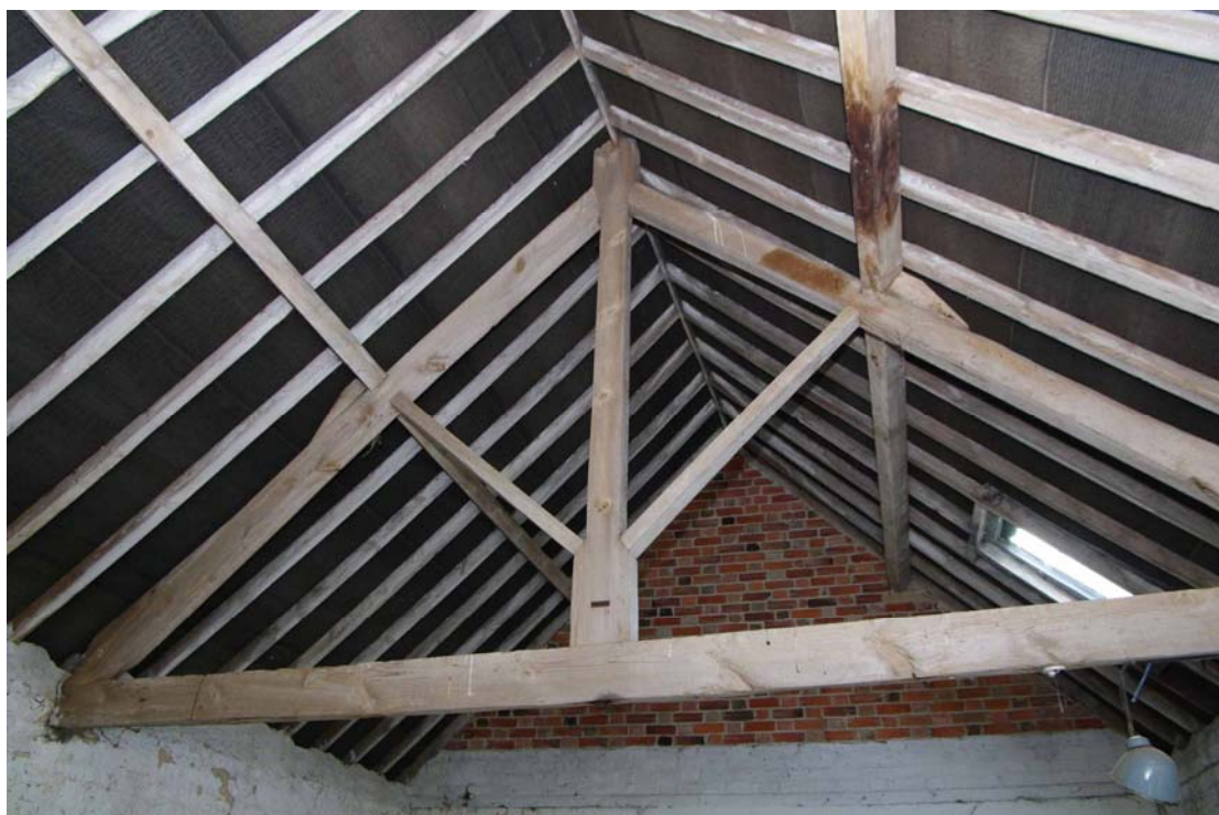
Figure 81: North range, Building C roof detail Looking north-east
