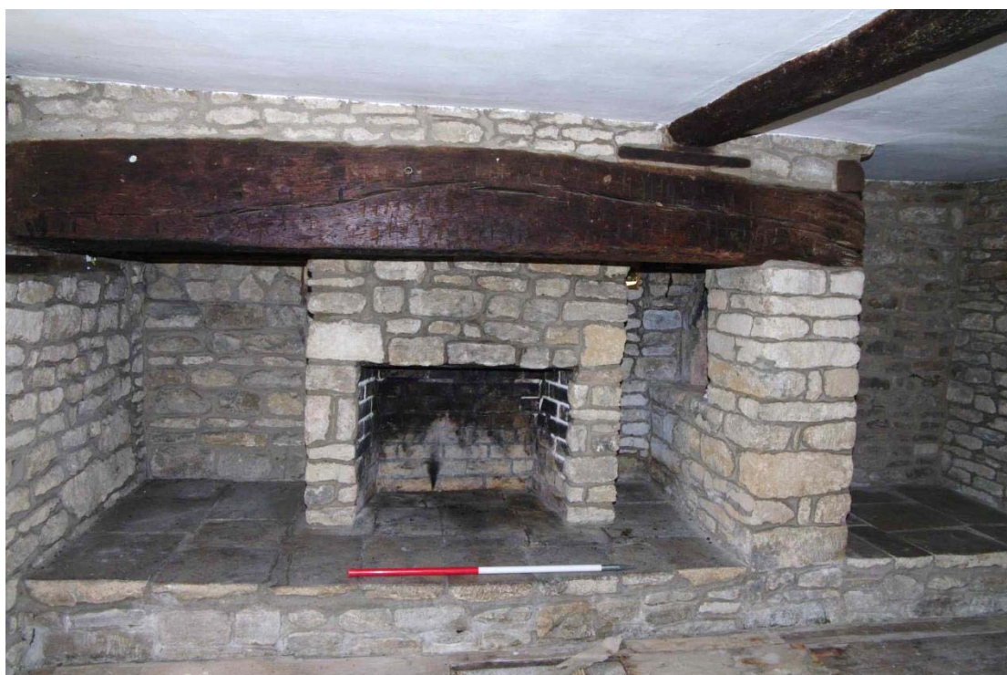
Figure 23: Ground floor, Room G1 fireplace Looking north, 1m scale
