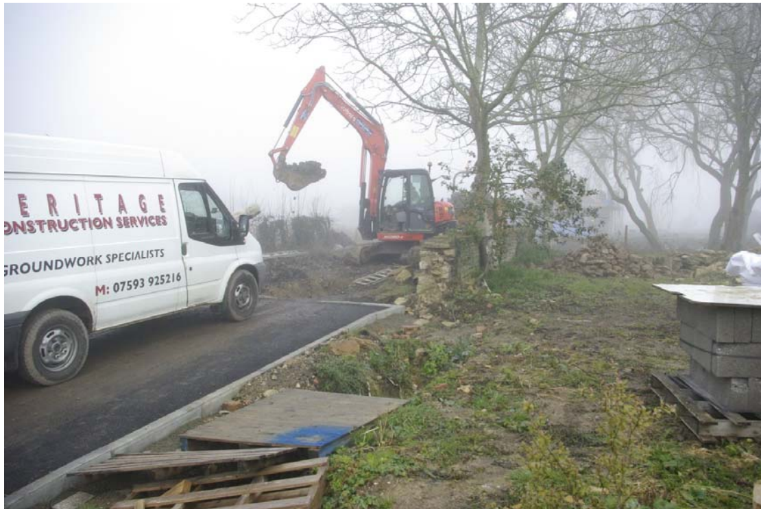
Figure 133: Work in progress on drain trench, looking north-west
