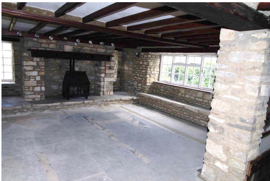
Figure 31: Ground floor, Room G4 Looking south-east, 1m scale. Cover to cellar steps just visible on right of picture
