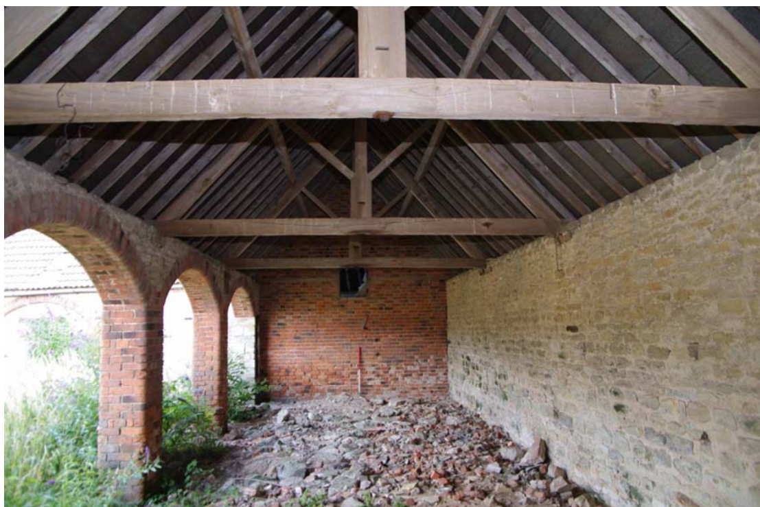
Figure 85: East range, Building D inside Looking north, 1m scale
