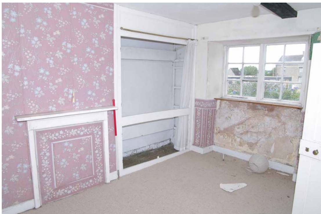
Figure 50: First floor, Room F4 Looking south-west, 1m scale
