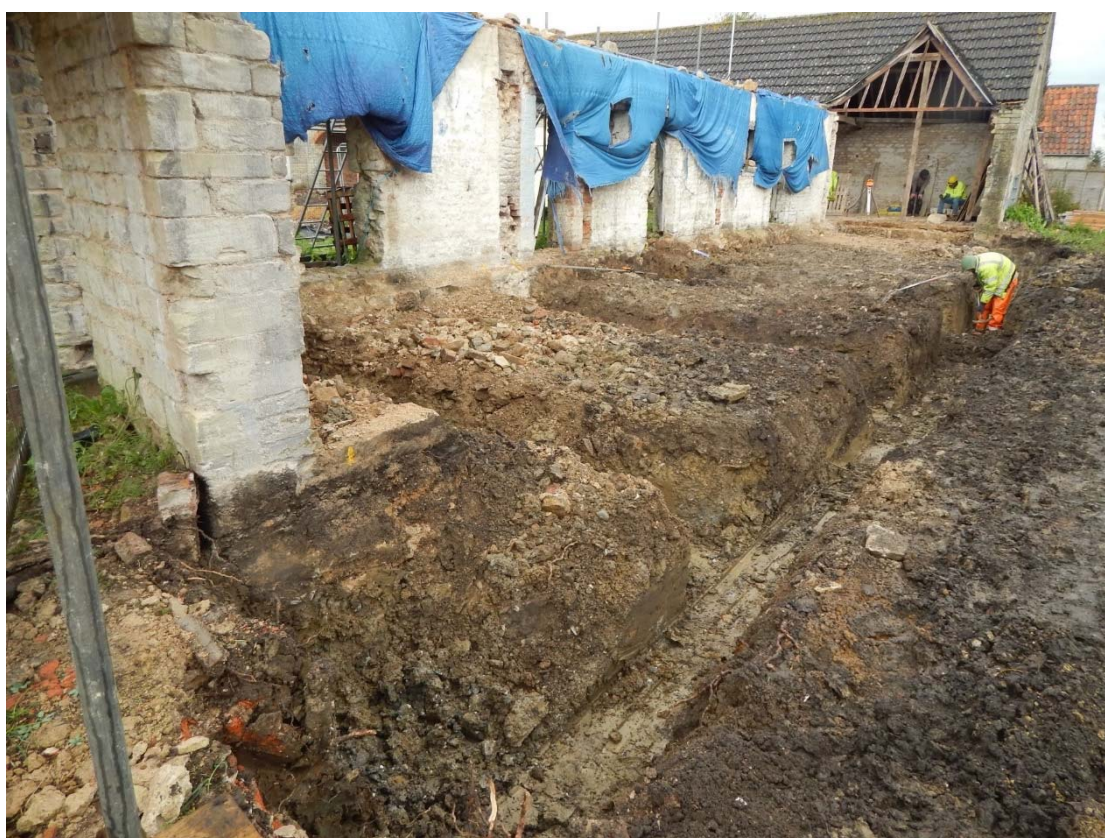
Figure 139: Completed foundation trenches Building F, looking east north-east
