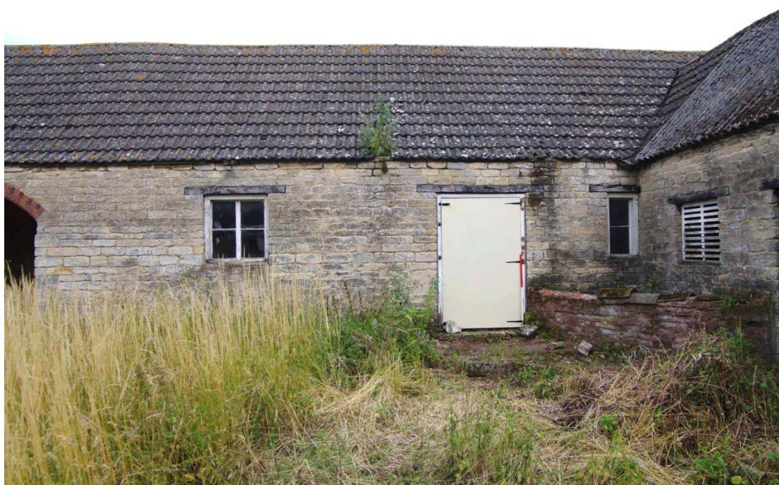
Figure 87: East range, Building E Looking east
