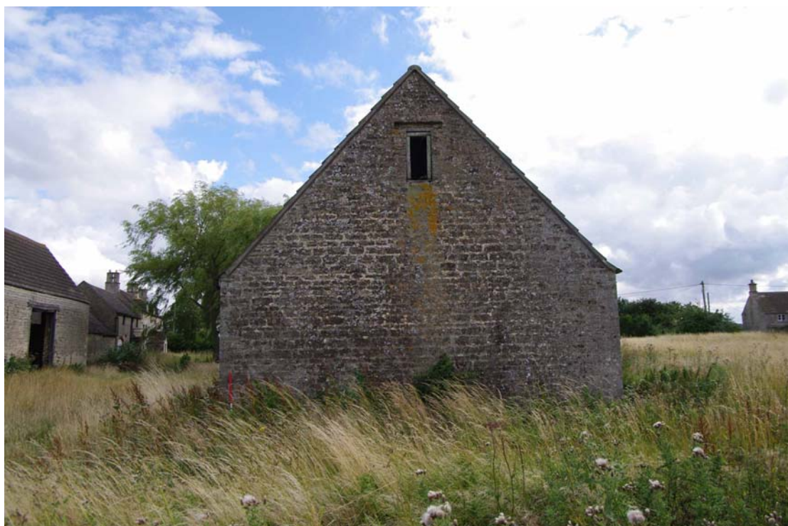
Figure 126: Cart shed (Building H), north facing elevation Looking south, 1m scale
