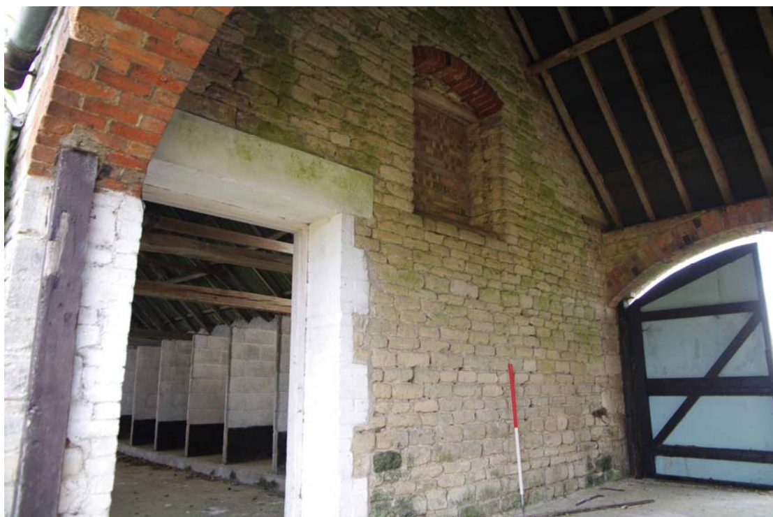
Figure 73: North range, east facing elevation of Building B Looking north-west, 1m scale. Note blocked window
