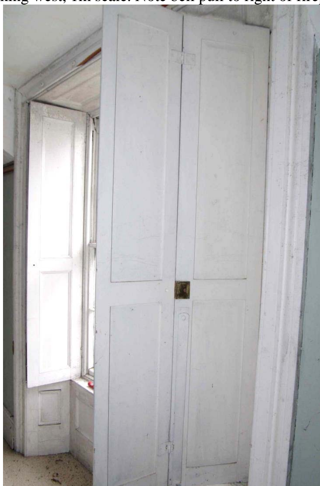
Figure 55: First floor, Room F5. Shutter detail
