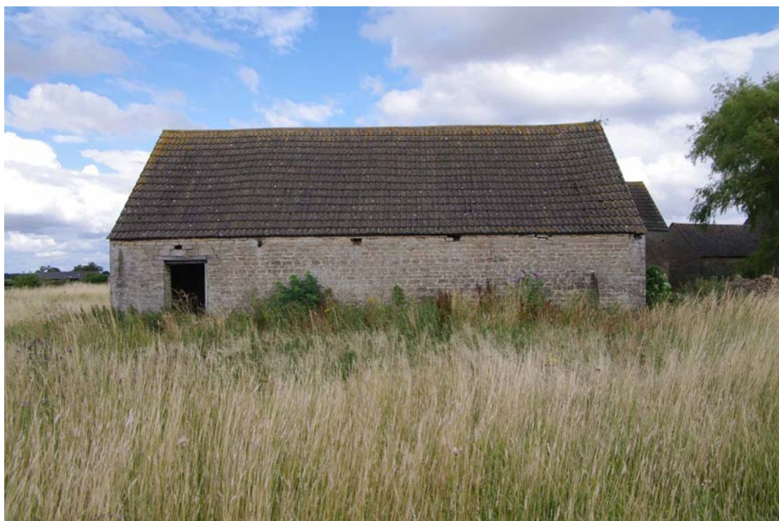
Figure 127: Cart shed (Building H), west facing elevation Looking east
