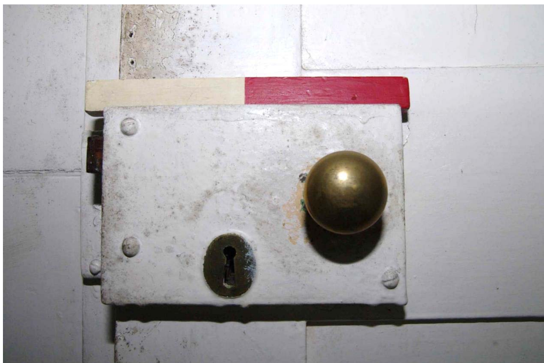
Figure 43: First floor, Room F1. Door lock detail 20cm scale
