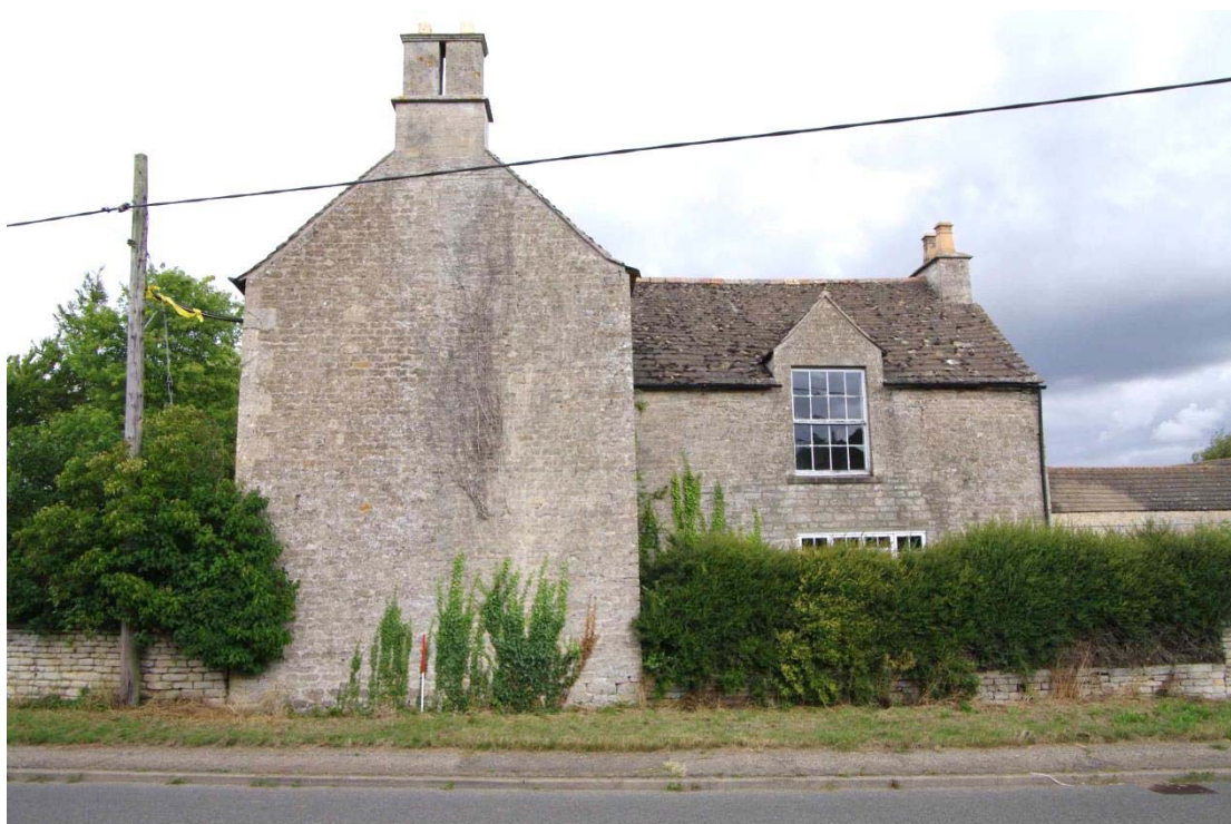
Figure 19: Farm House, rear south wing south facing elevation Looking north, 1m scale
