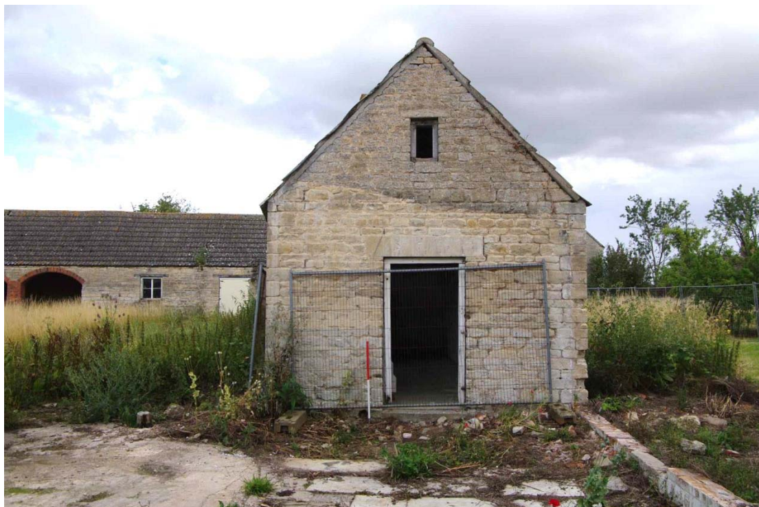
Figure 94: South range west facing elevation Looking east, 1m scale
