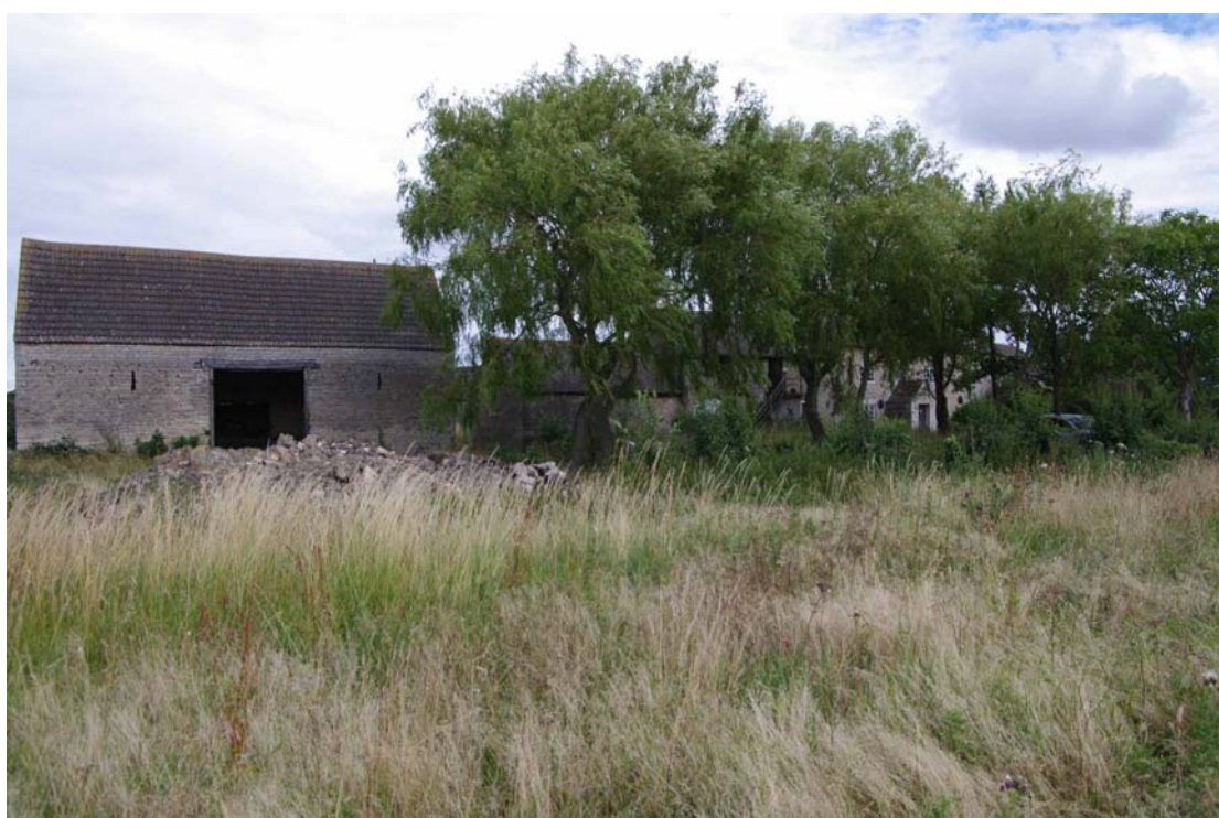
Figure 104: West range, west facing elevation Looking south-east. Pond in foreground
