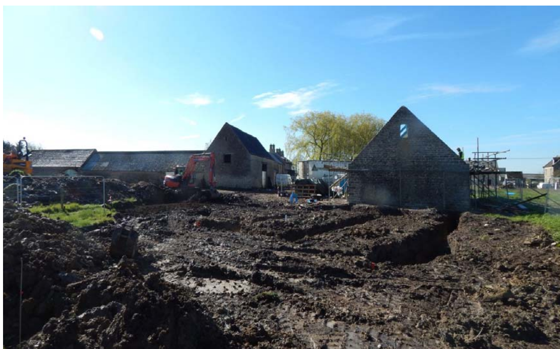
Figure 142: The finished trenches at Unit 3, looking south
