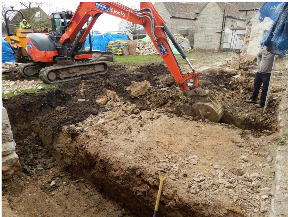
Figure 138: Work in progress on Building F, looking south-west
