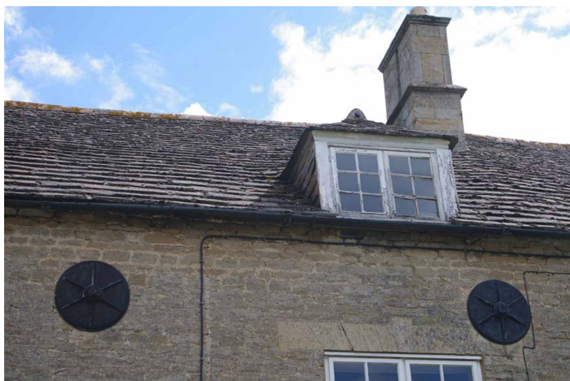
Figure 13: West facing elevation, dormer window detail
