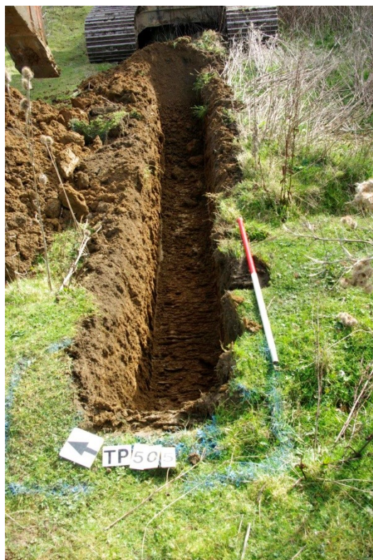
Figure 10 TP505 excavated to top of natural substratum Looking east. 1m scale
