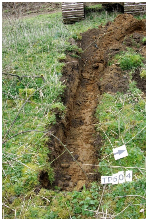
Figure 9 TP504 excavated to top of natural substratum Looking west. 1m scale
