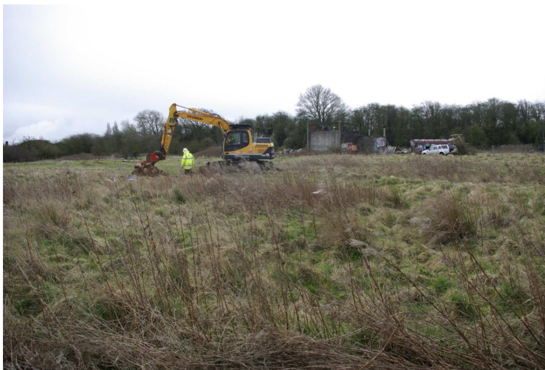
Figure 3 General view of site
