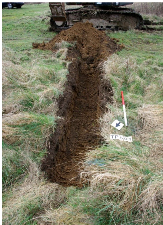
Figure 6 TP501 excavated to top of natural substratum Looking south-east. 1m scale
