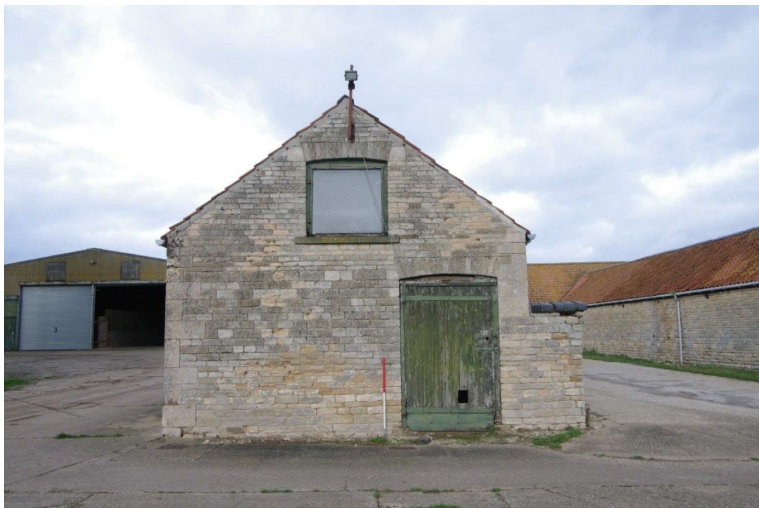
Figure 10 South facing gable end of western range Looking north. 1m scale
