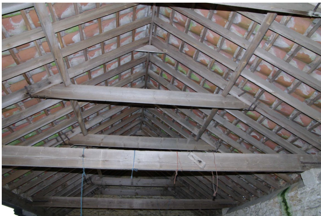
Figure 24 Barn roof structure The style is common throughout the building
