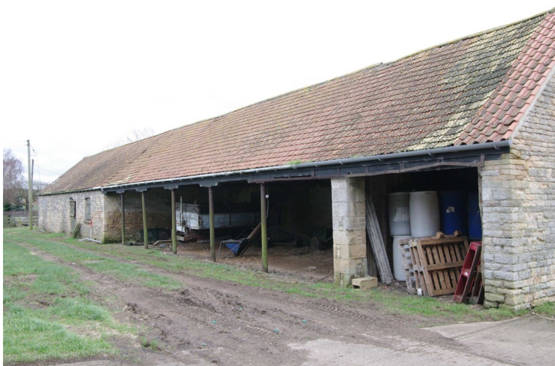
Figure 13 North facing elevation Looking south-east. 1m scale
