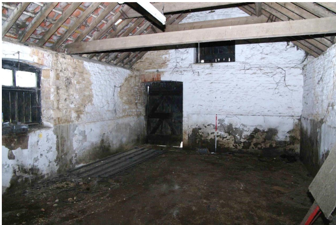
Figure 29 South room of centre range Looking south-east. 1m scale
