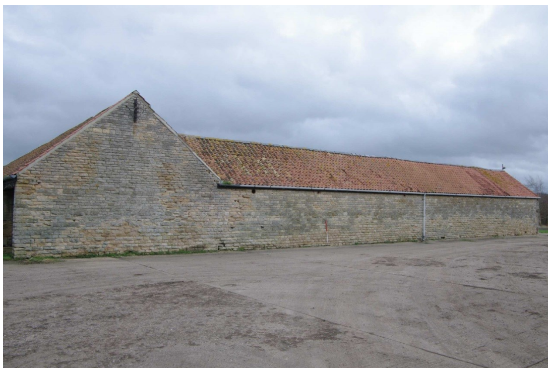
Figure 12 West facing elevation Looking south-east. 1m scale
