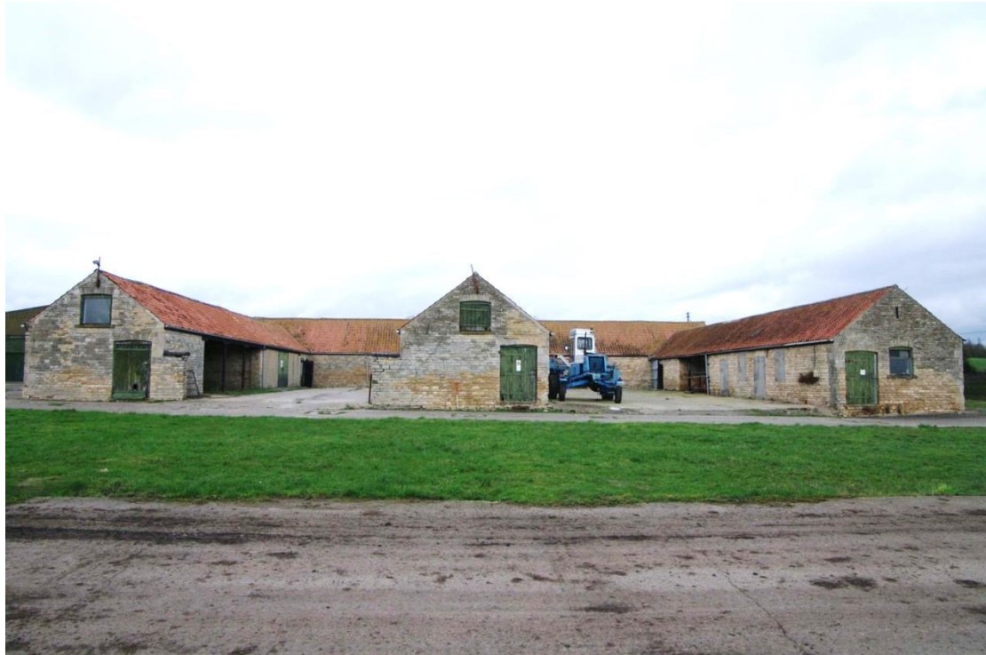
Figure 9 South facing elevation Looking north. 1m scale
