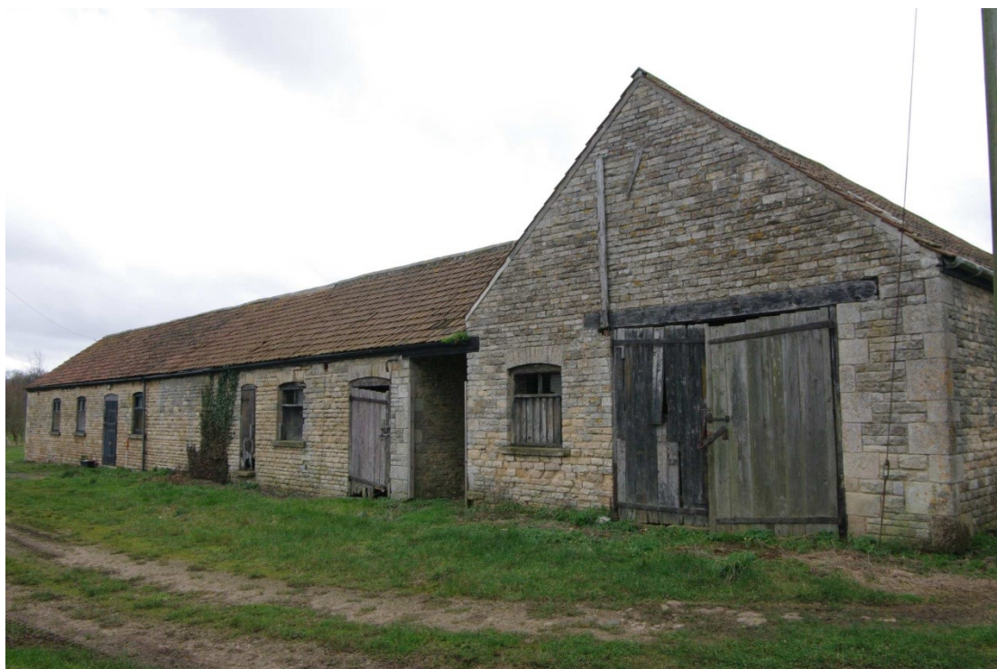
Figure 15 East facing elevation Looking south-west. 1m scale
