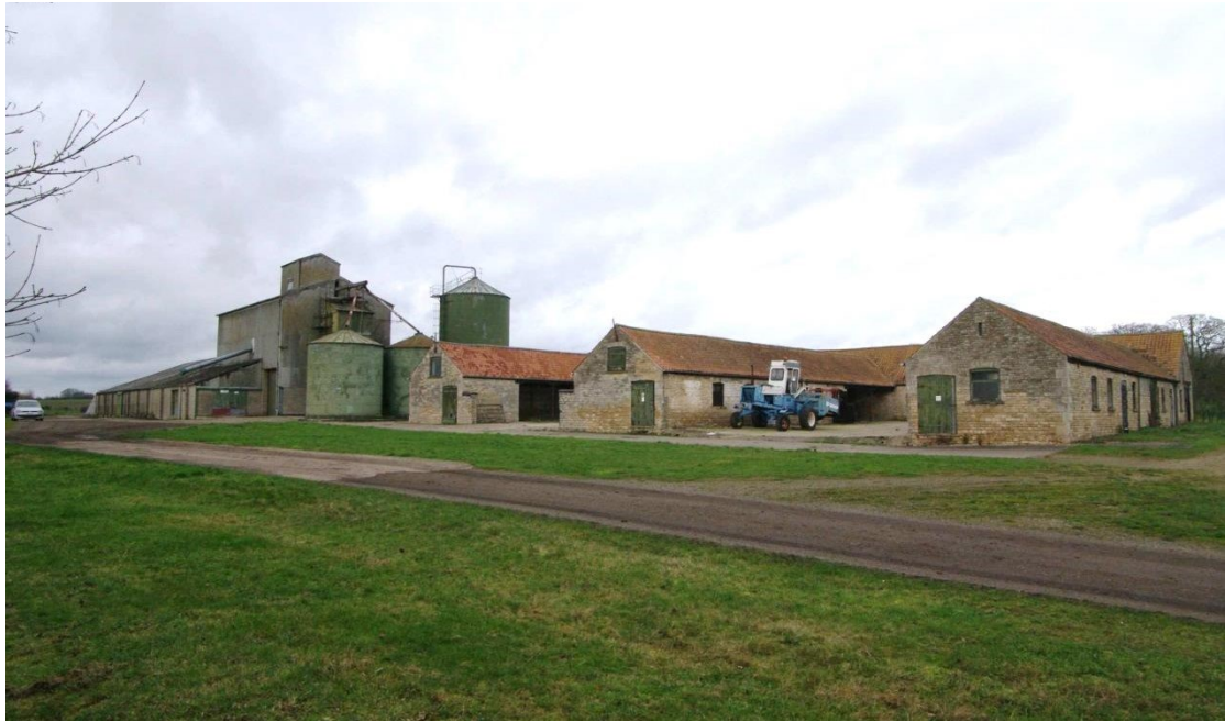
Figure 7 Barns and modern buildings Looking north-west
