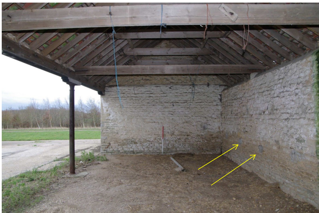
Figure 28 Open shed of west range Looking south. 1m scale. Yellow arrows point to locations of byres or stalls
