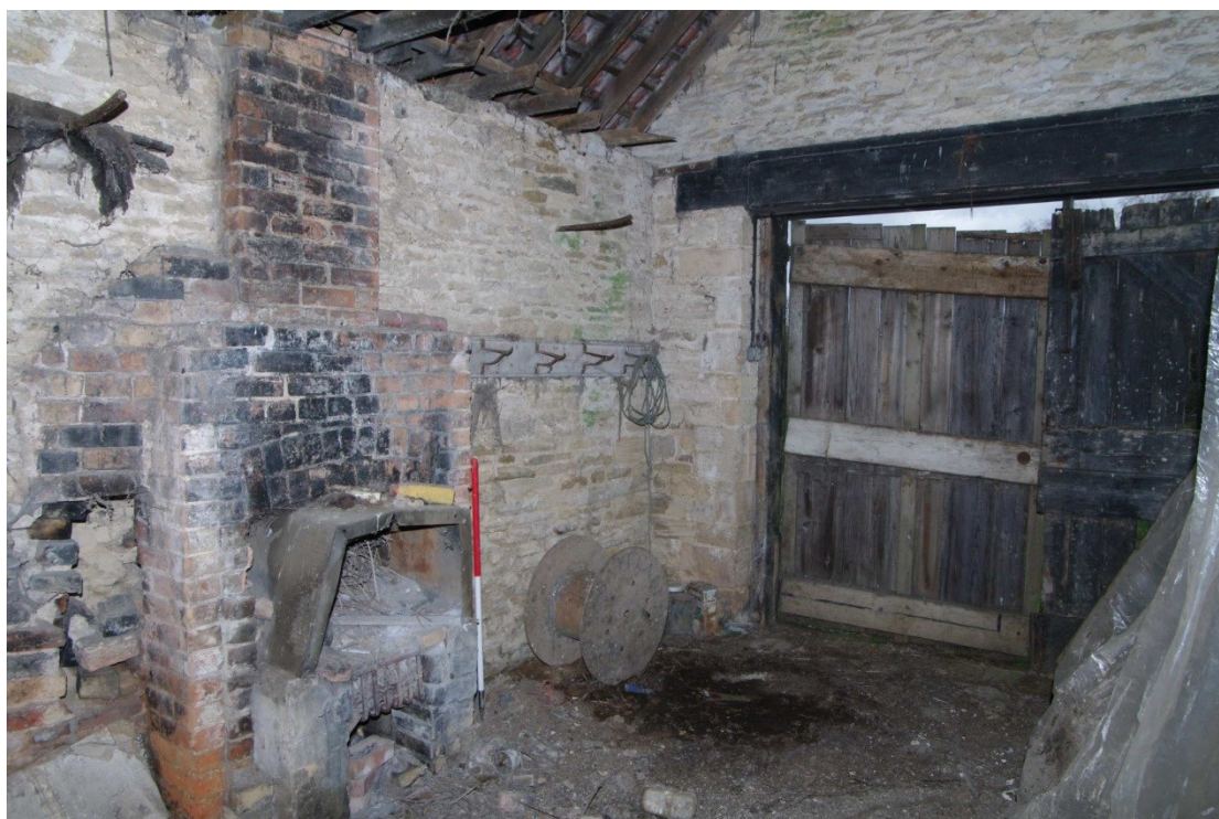
Figure 25 East room of north range Looking north-east. 1m scale
