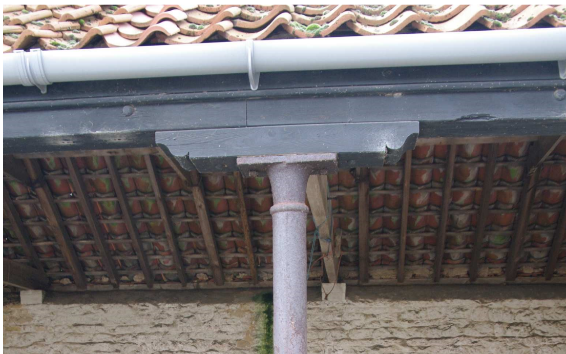
Figure 14 Column detail and woodwork on the open sheds
