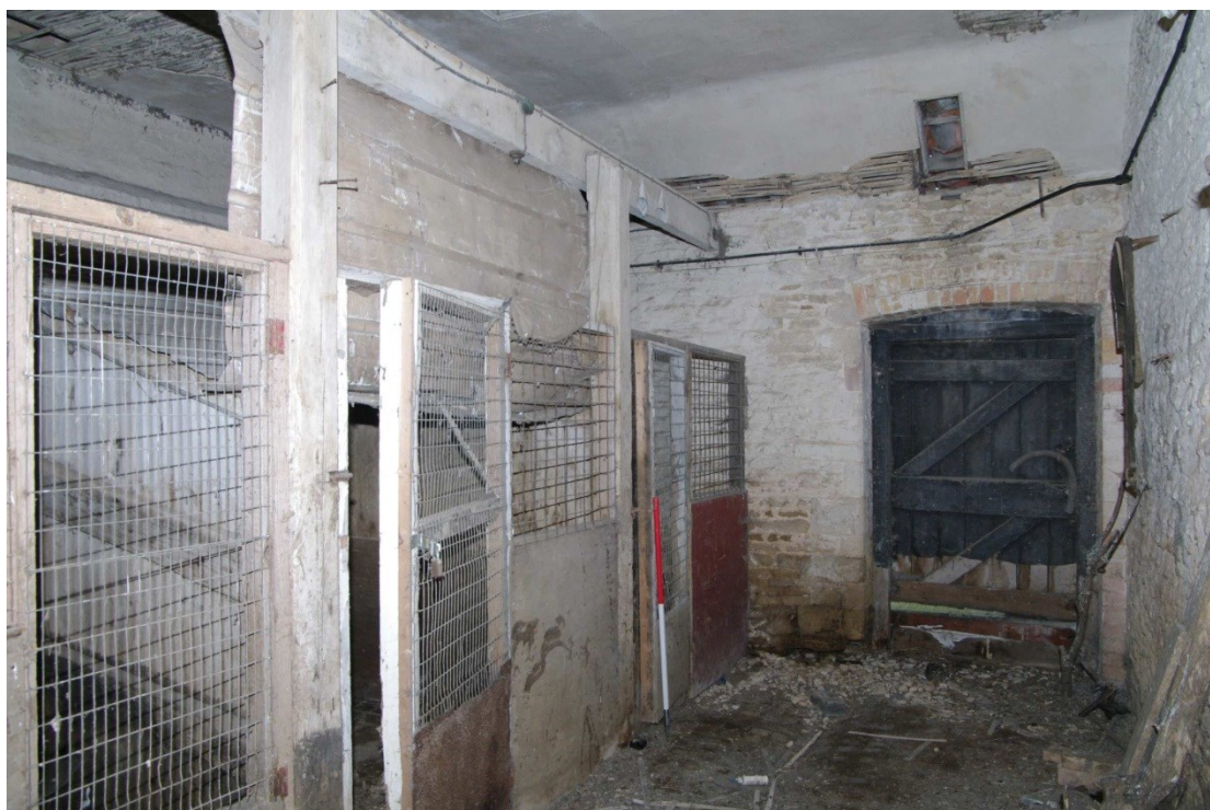
Figure 31 East range kennels Looking west. 1m scale
