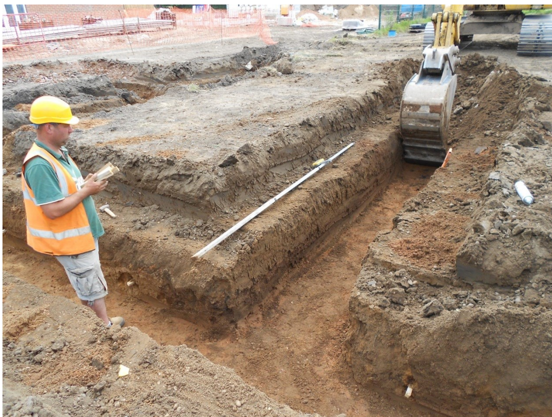
Figure 6: Work in progress on foundation trenches, looking south-west
