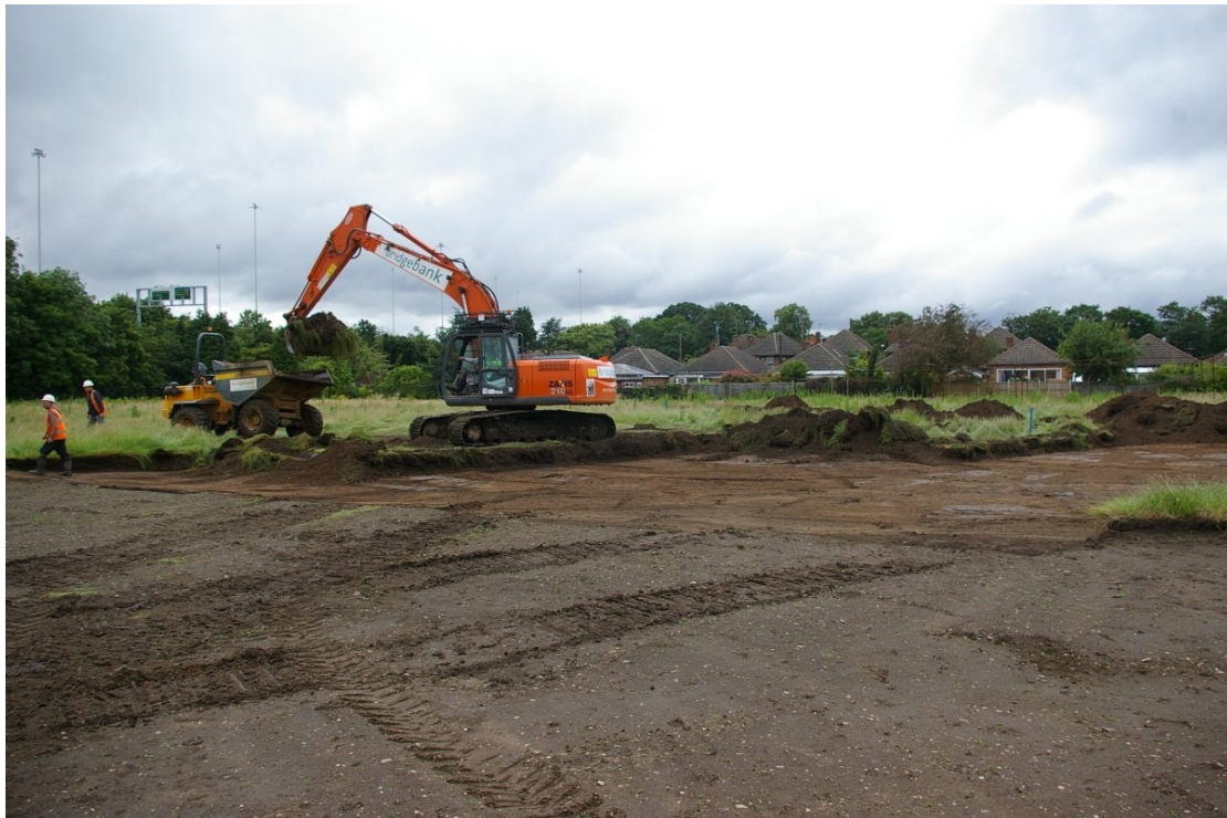
Figure 7: Stripping the northern part of site, looking north-west
