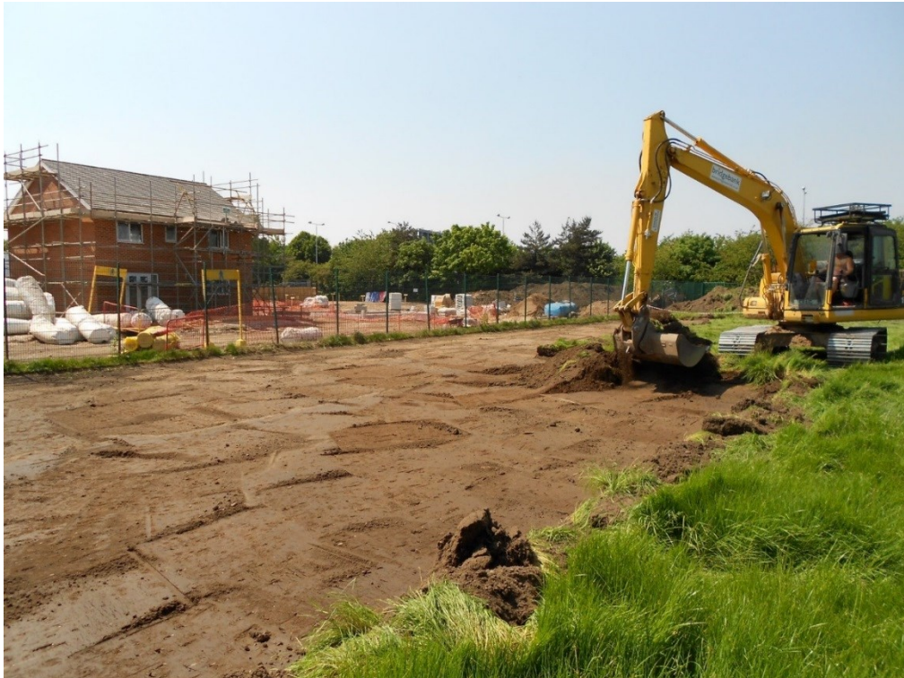
Figure 4: Work in progress on south-east edge of site, looking south-west
