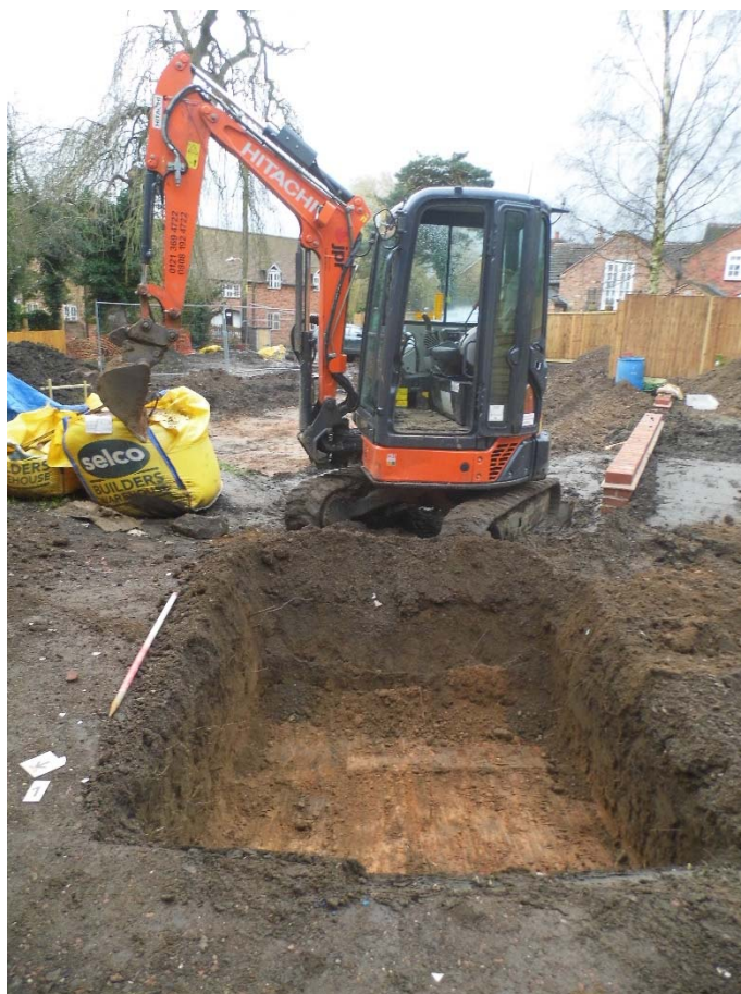
Figure 11: Excavation of the soakaway
