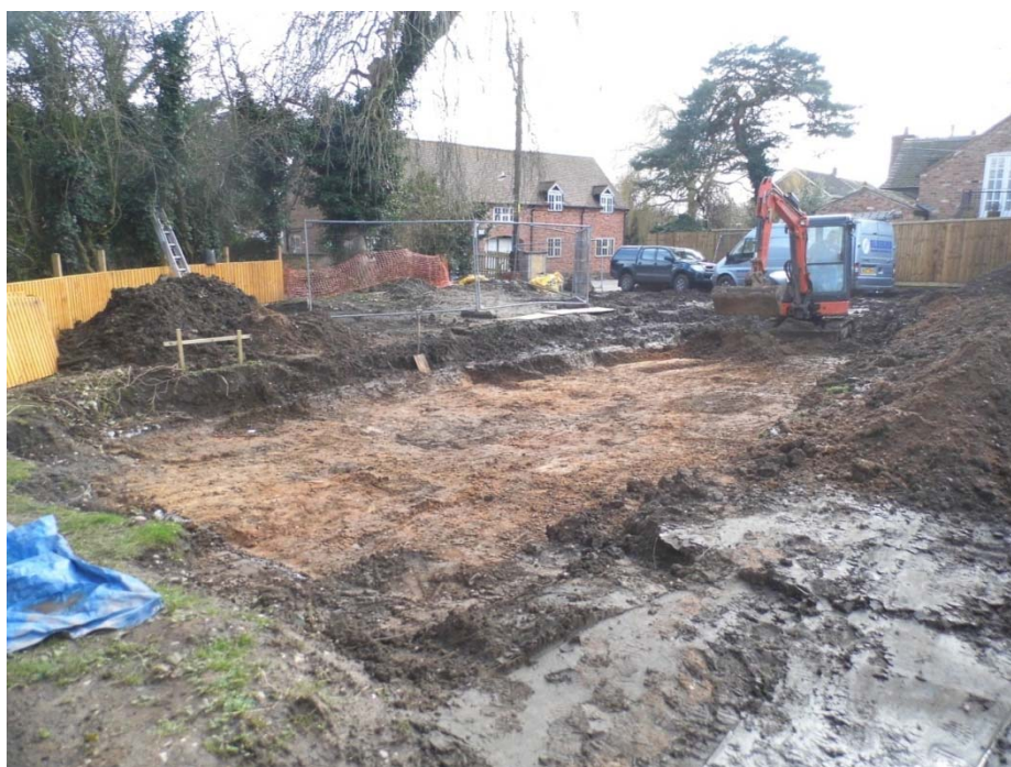
Figure 5: Excavating along building footprint, looking south-east
