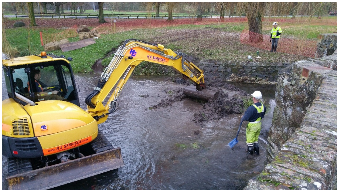
Figure 3: Dredging in progress; view southeast
