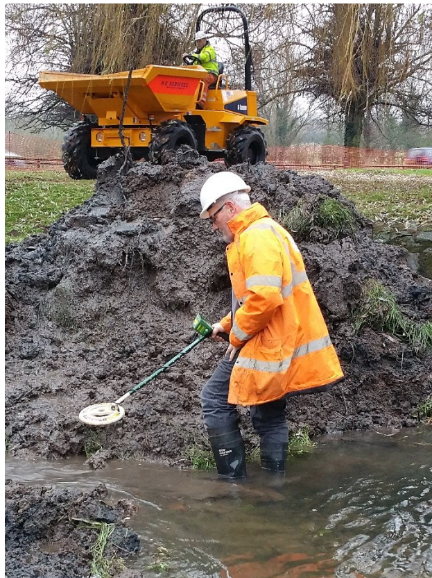
Figure 5: Metal detector scanning of river silts
