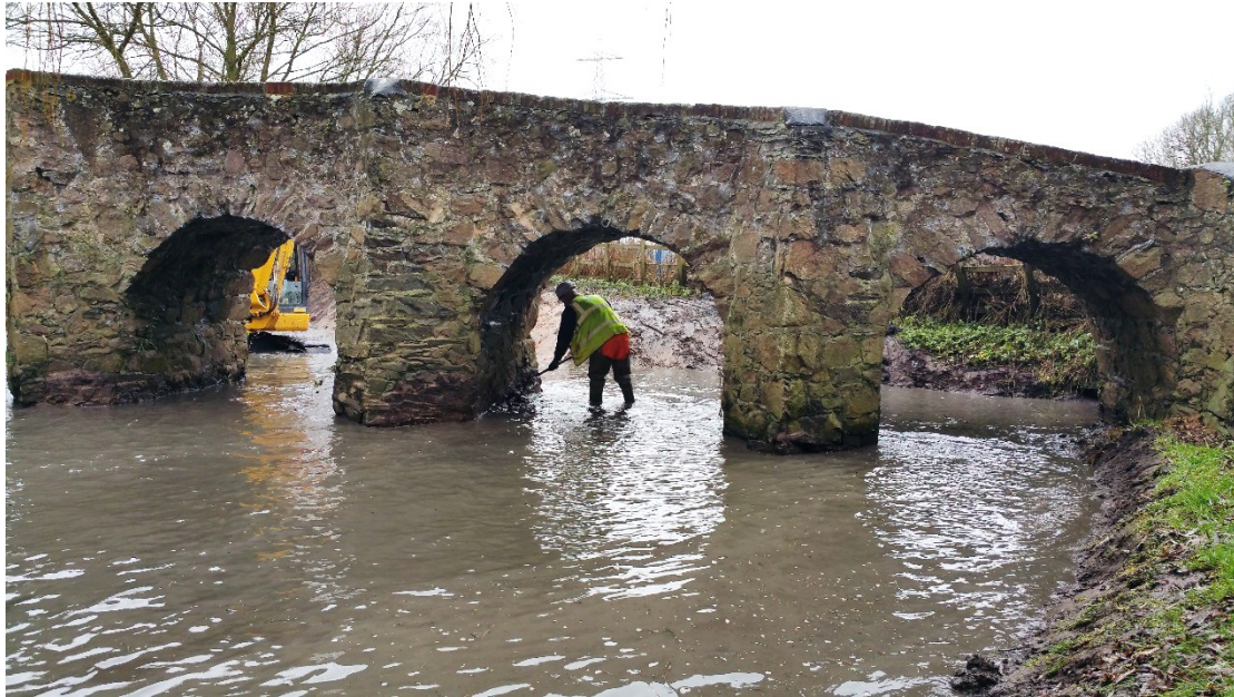
Figure 4: Hand clearance of river silts; view looking south-west
