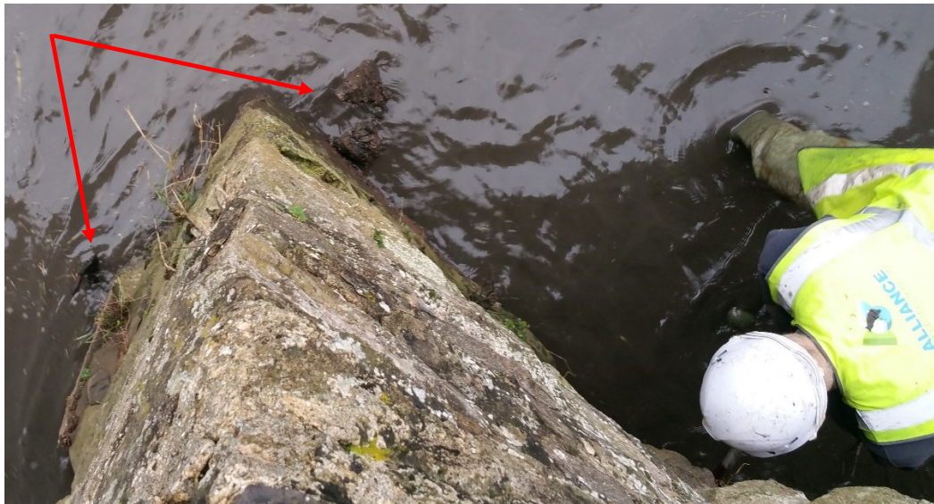
Figure 8: Pier 1 with timbers visible; view looking south-west
