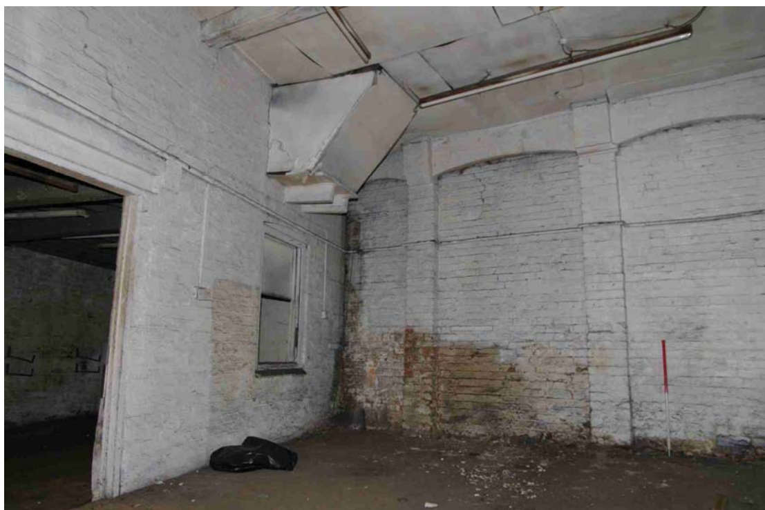
Figure 50 Building C ground floor, Room CG1 Looking north-west. 1m scale. Former door and window from Building B on left. Note moulded stone on the right brick pilaster and the corbelled brick on the left
