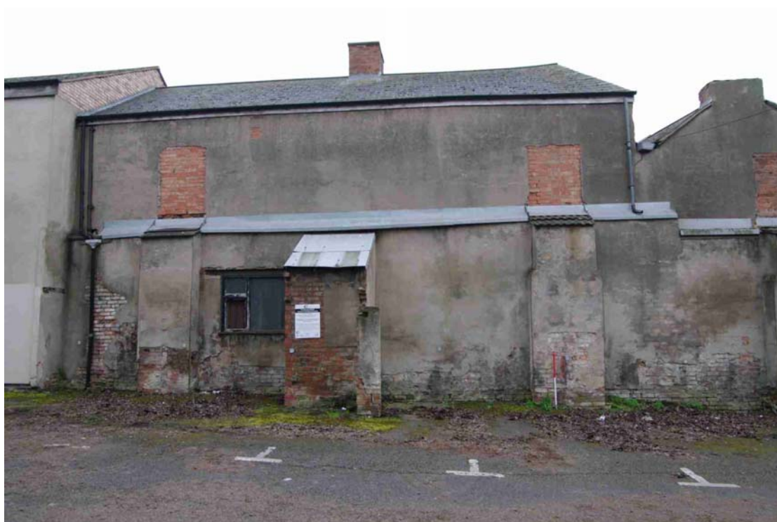
Figure 25 Building C north-east facing elevation Looking south-west. 1m scale. Note inserted ground floor window
