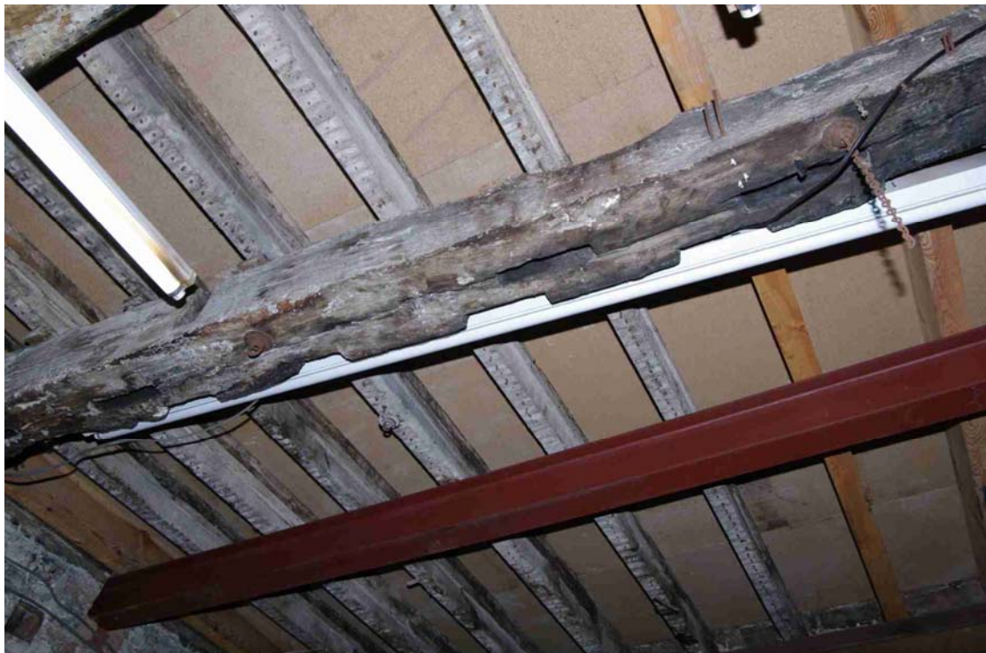
Figure 54 Building C ground floor, Room CG2 ceiling Southern area of ceiling with replacement steel beam and re-used joists
