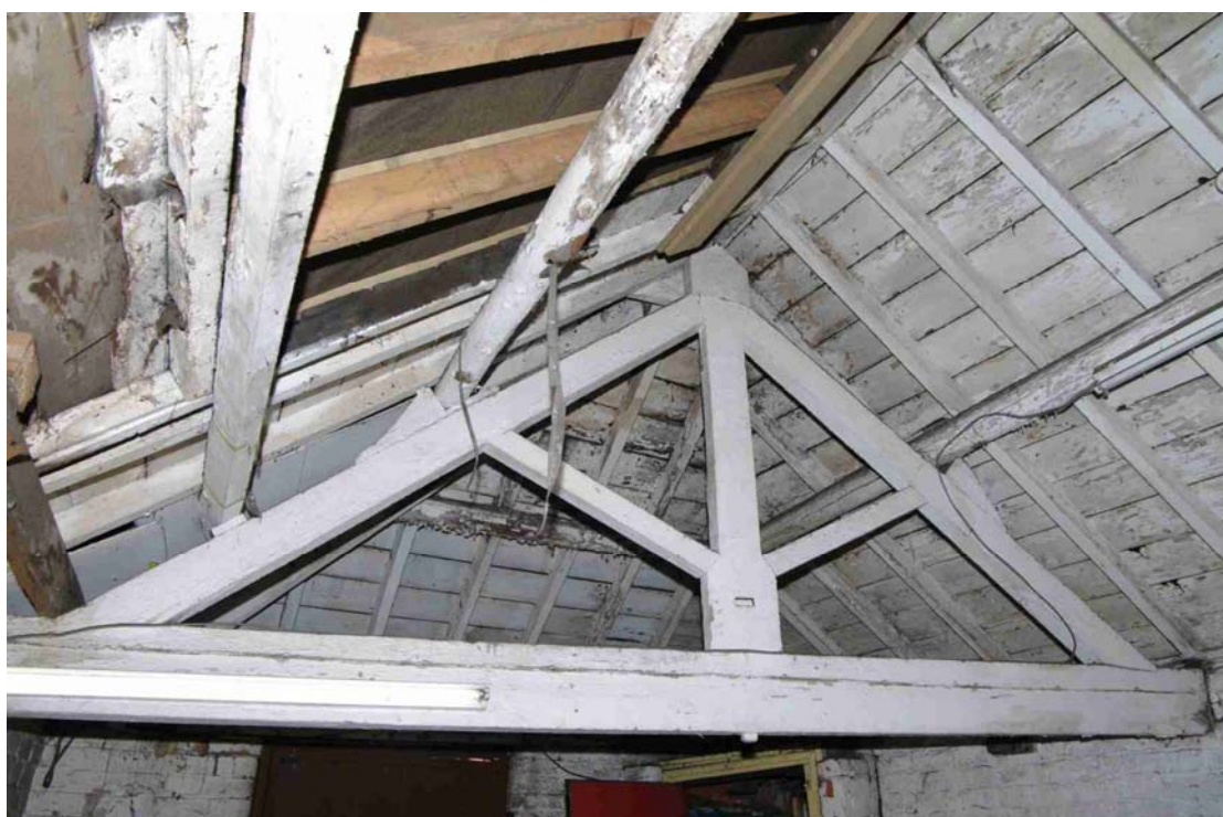
Figure 47 Building B first floor roof detail Looking south. Note round section purlins
