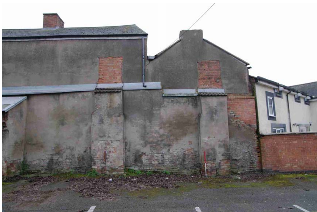
Figure 20 Building B north-east facing gable end Looking south-west. 1m scale. Building C on left. Note buttresses and remnant of outbuilding walls against the ground floor walls
