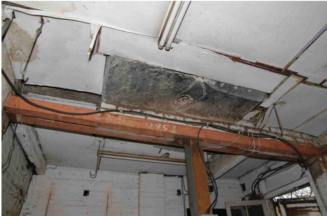
Figure 30 Building A ground floor, Room AG1 supported chimney stack Looking east
