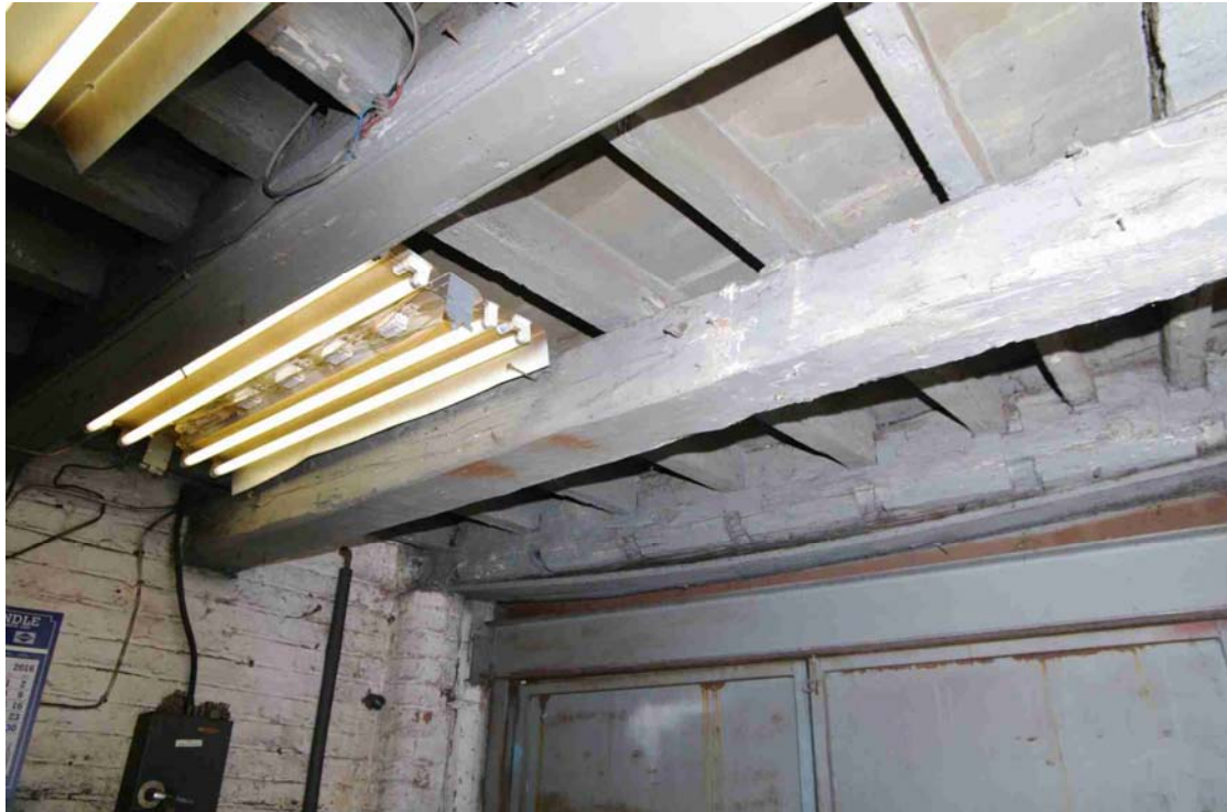
Figure 42 Building B ground floor, reused ceiling joists Looking east above main doorway
