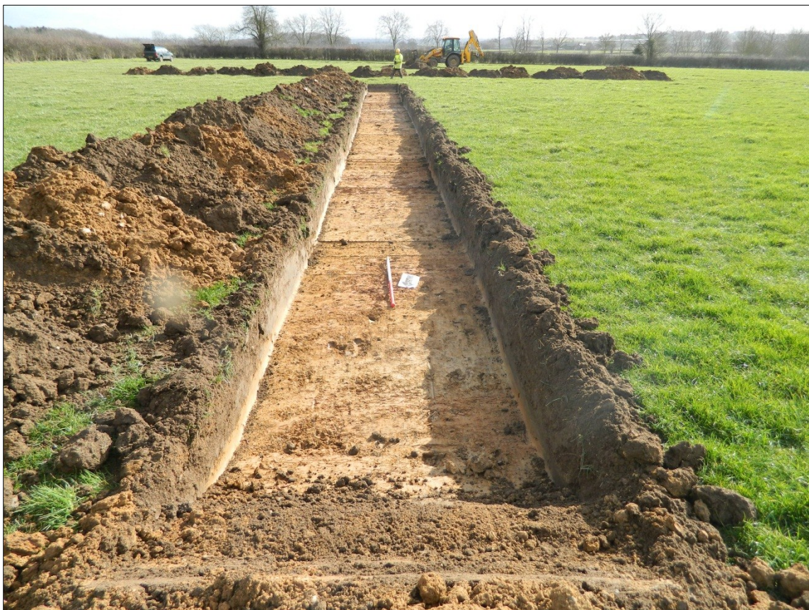
Plate 1: Trenching works being carried out
