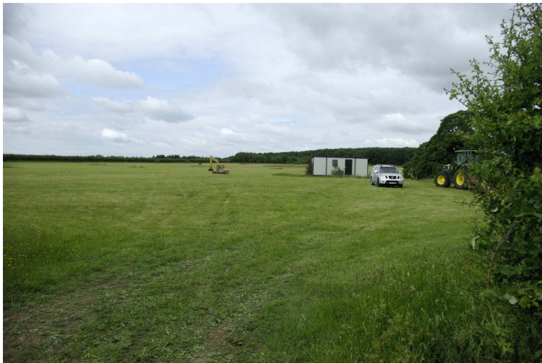
Figure 3 General view of site Looking south-west. Attenuation pond to be placed to the left of the digger, house to be in area of longer grass behind the cabin and before the woodland
