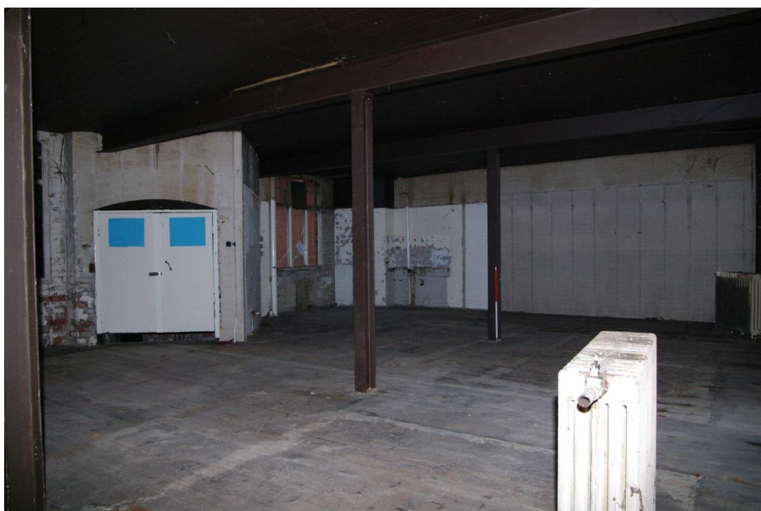
Figure 79 Second floor, rear range Looking south-east. 1m scale. Note goods lift on left
