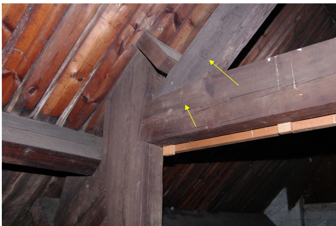
Figure 94 Fourth floor, carpenter's marks Roman numeral III arrowed
