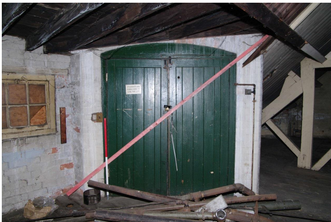
Figure 99 Fourth floor, goods lift Looking south-east. 1m scale
