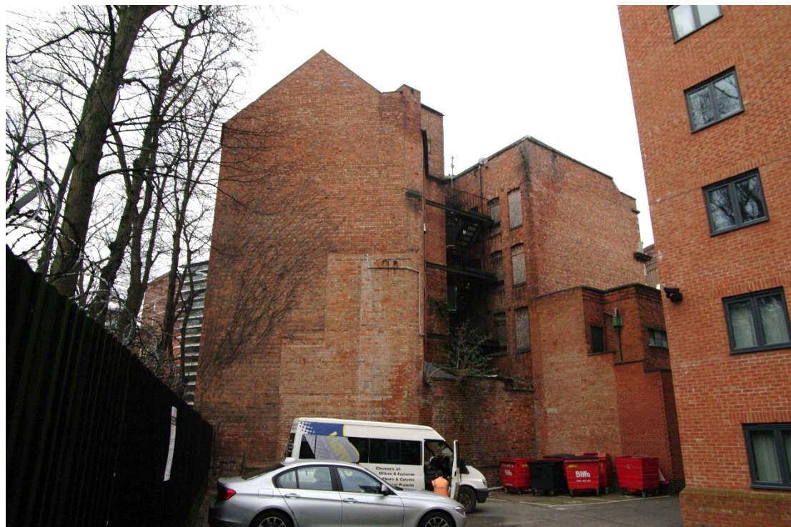
Figure 29 South-east facing elevation Looking north
