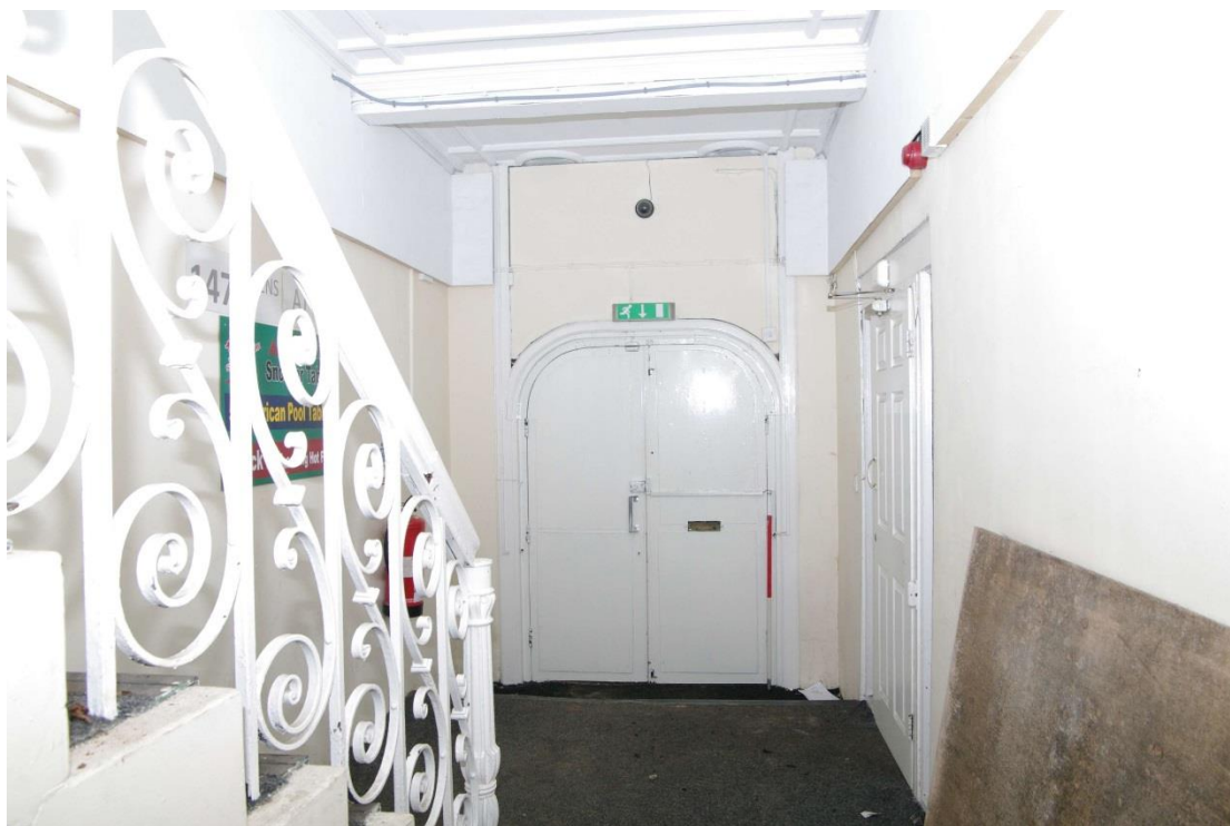
Figure 47 Ground floor, Tyler's principal entrance hall Looking north-west. 1m scale. Ornamental frieze protected behind boards at ceiling height
