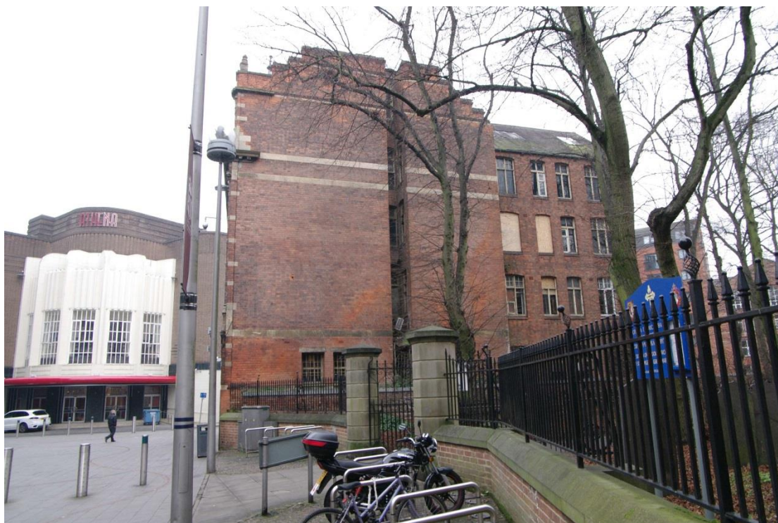
Figure 25 South-west facing elevation Looking east
