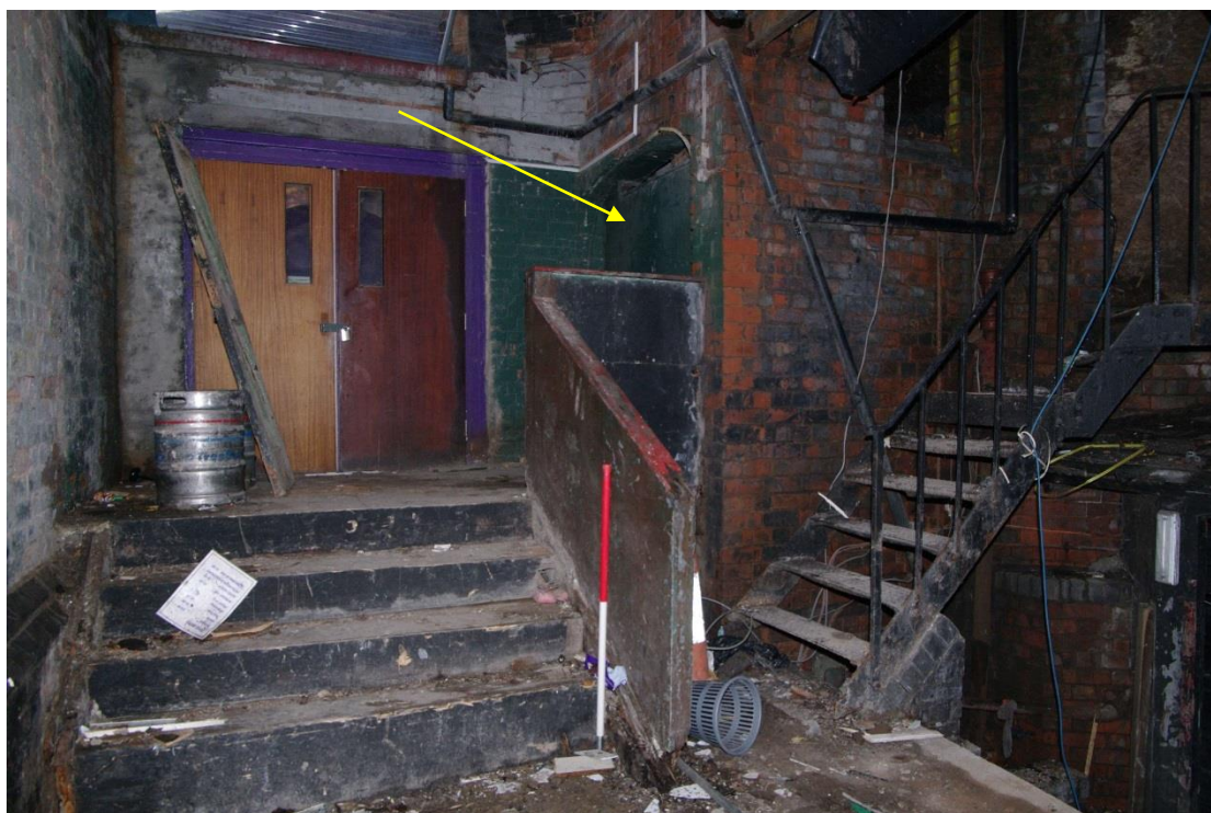
Figure 32 Open air loading bay
