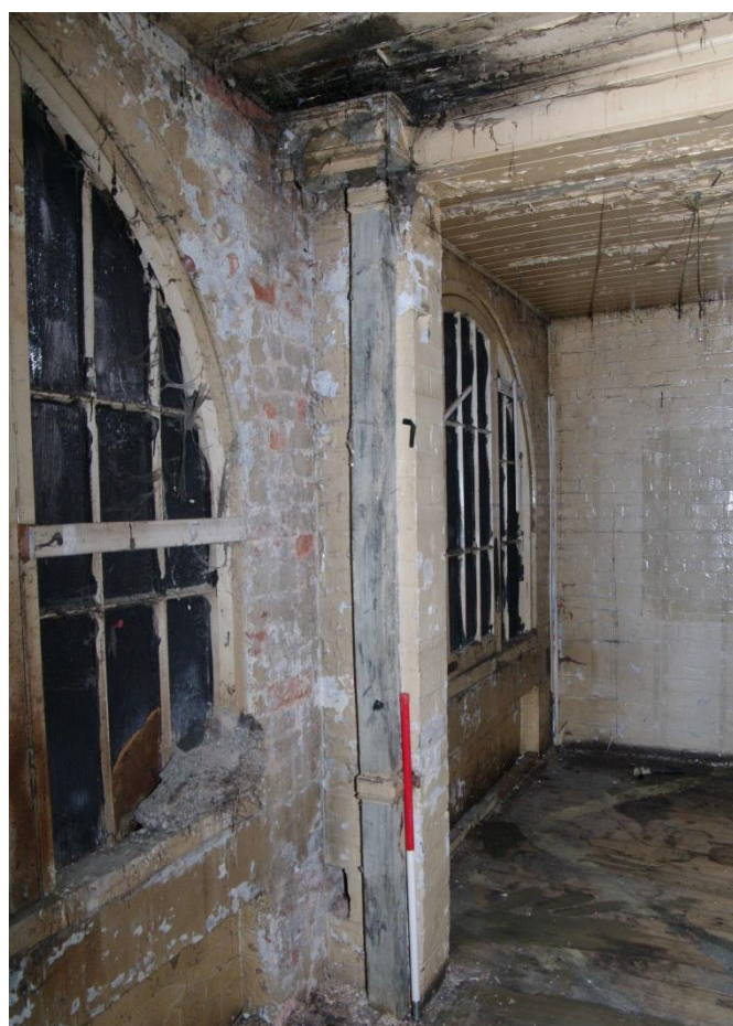
Figure 89 Third floor, internal lead downpipe and hopper Looking east. 1m scale
