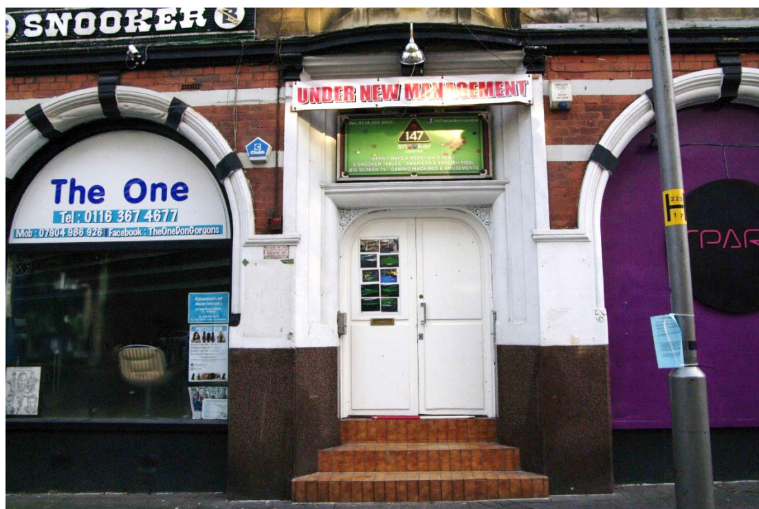
Figure 18 Ground floor entrance, north-west facing elevation Looking south-east. 1m scale
