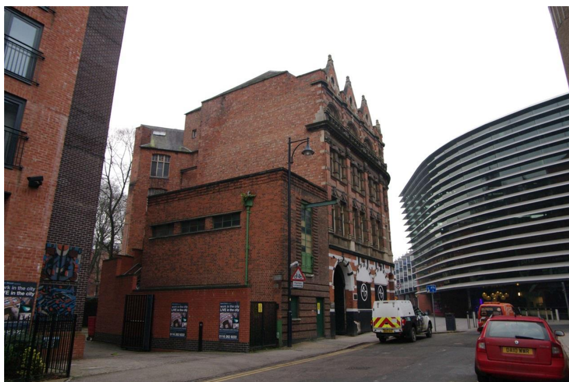
Figure 7 View from Queen Street looking west Curve Theatre on right
