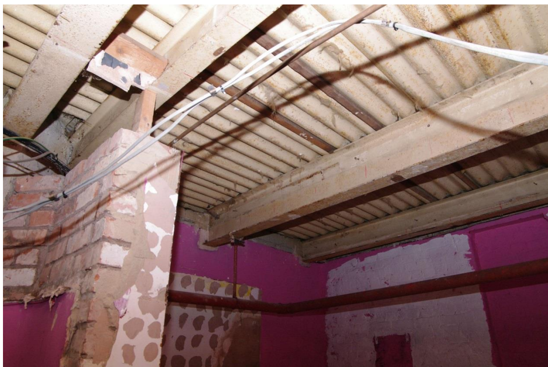
Figure 35 New basement ceiling and supports beneath rear range
