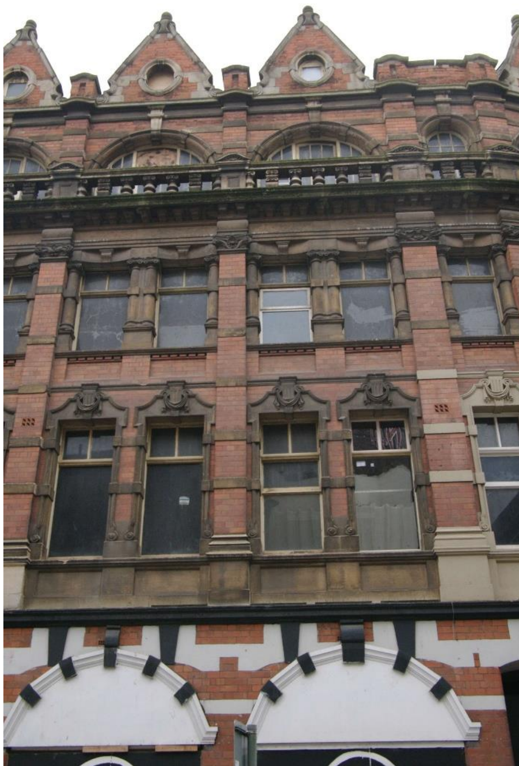
Figure 15 Upper floor details, NE facing elevation Looking south-east
