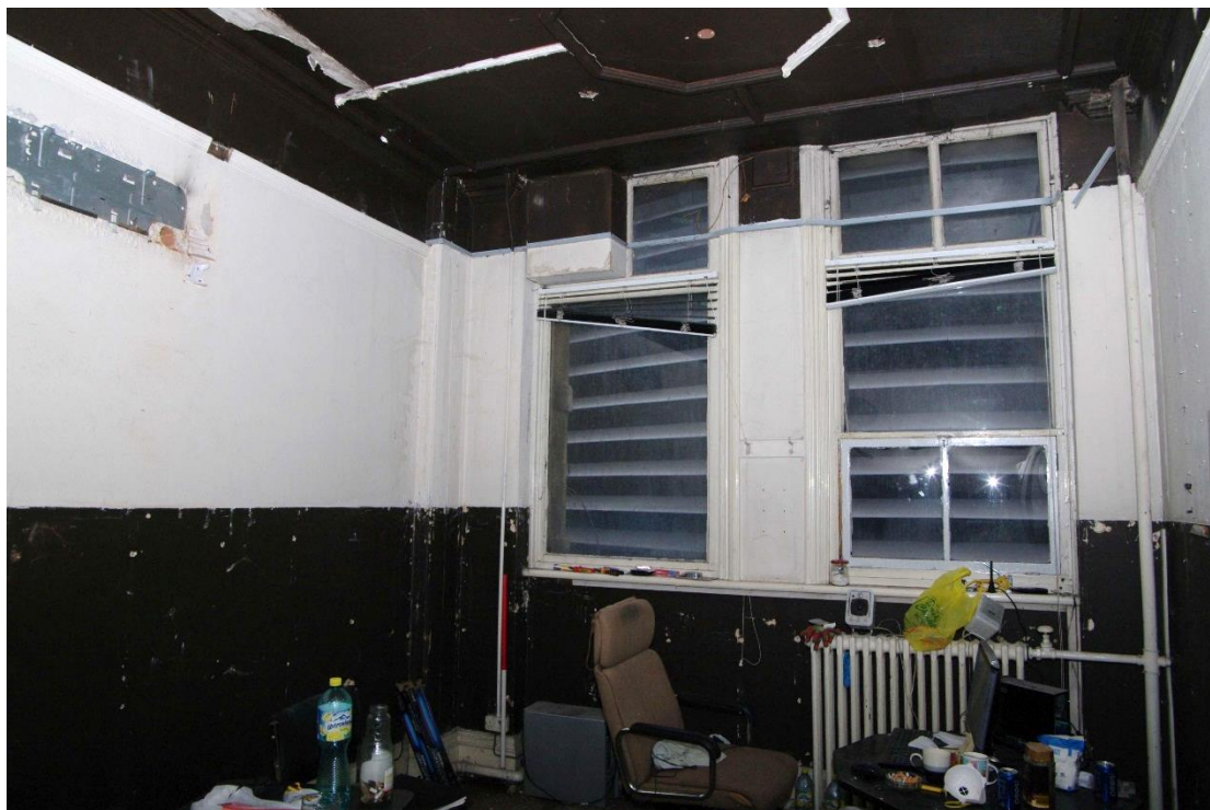
Figure 65 First floor, former reception room Looking north-west. 1m scale
