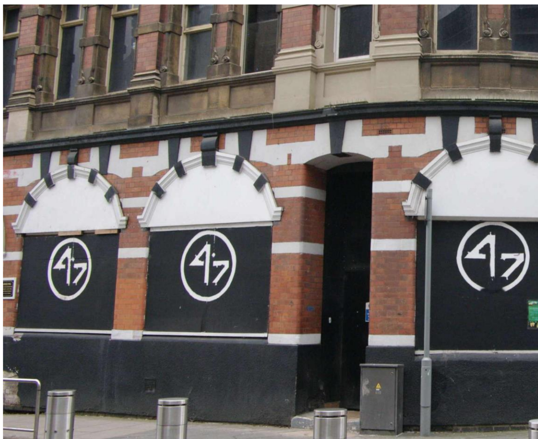
Figure 13 Ground floor detail, NE facing elevation Looking south-east
