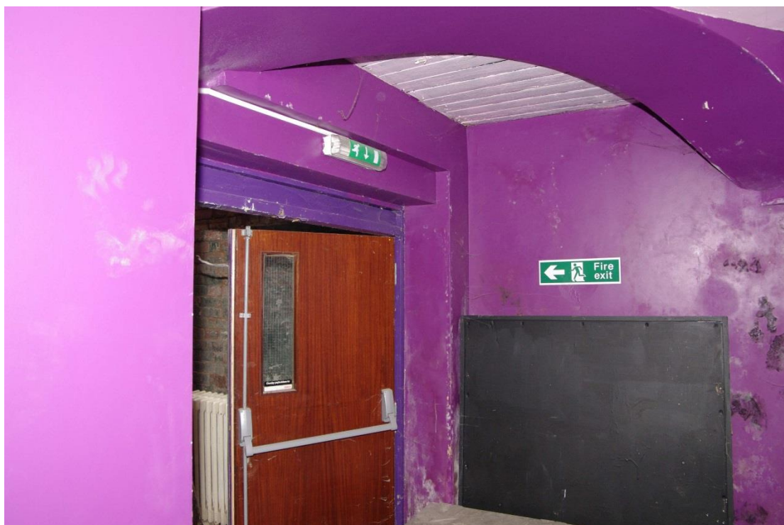
Figure 59 Ground floor, exit to the loading bay Looking east
