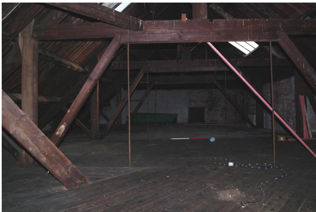
Figure 92 Fourth floor, above north-east facing range Looking east. 1m scale
