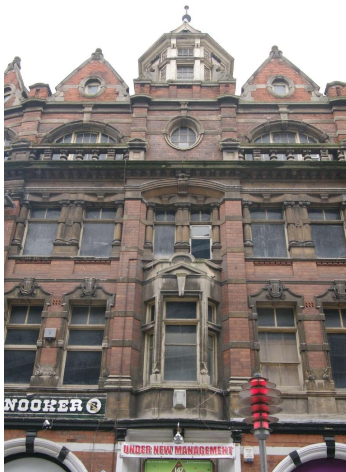
Figure 22 Upper floor detail, north-west facing elevation Looking south-east
