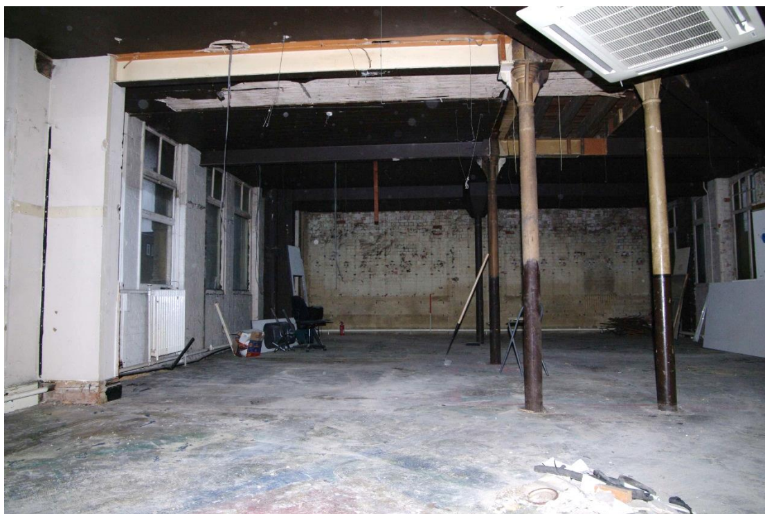
Figure 71 First floor warehouse behind north-east facing elevation Looking east. 1m scale
