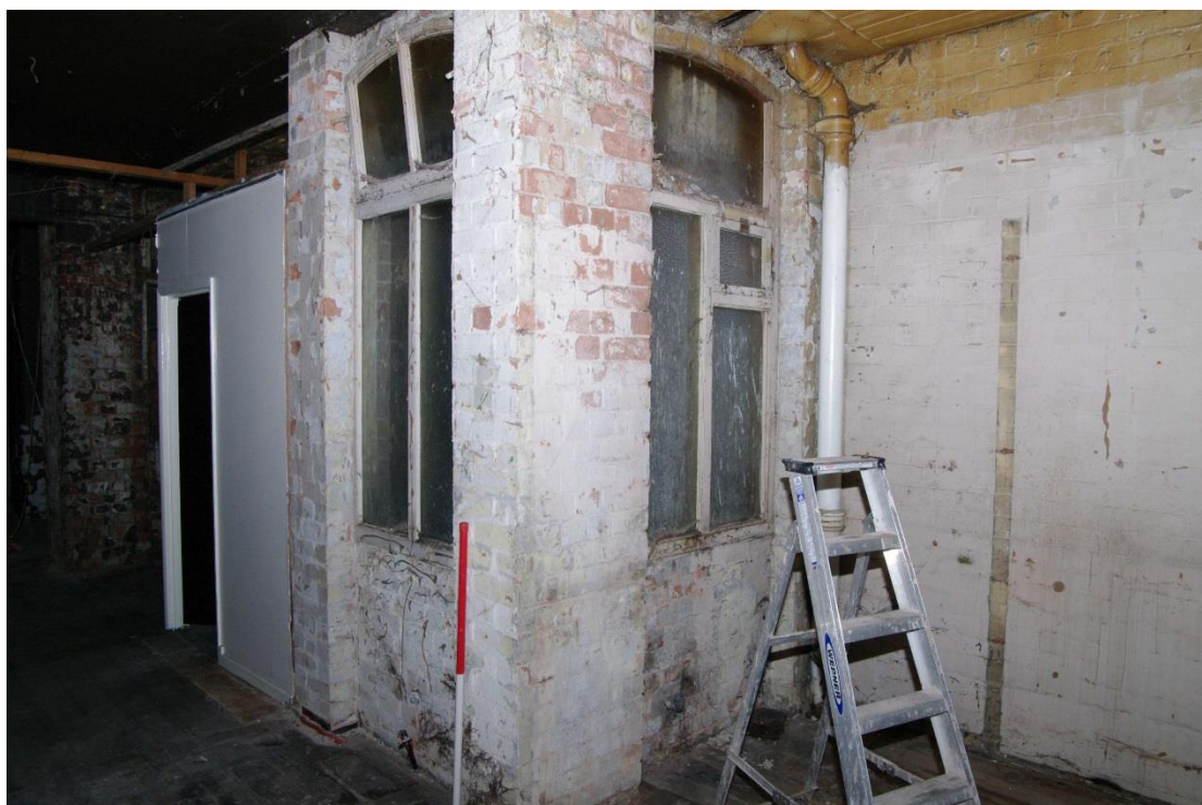
Figure 82 Second floor, north-west facing range toilet windows Looking south. 1m scale
