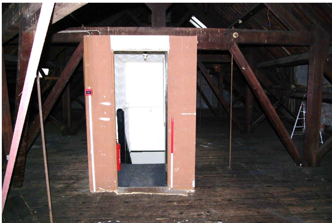
Figure 91 Fourth floor, stairs to lower floors Looking south-east. 1m scale
