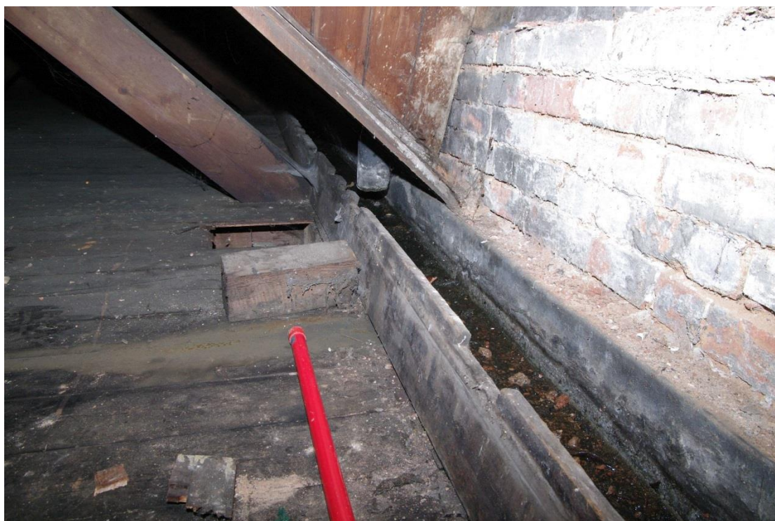
Figure 97 Fourth floor, internal rainwater gutter Looking west
