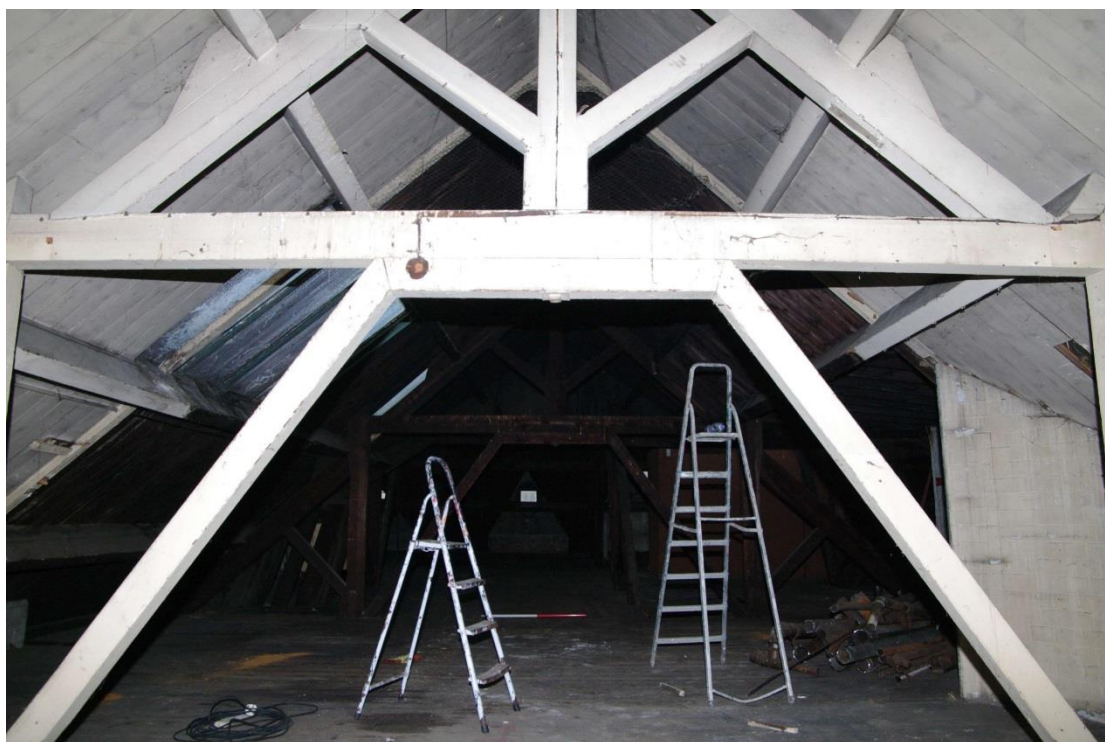
Figure 95 Fourth floor, roof structure Looking north from rear range
