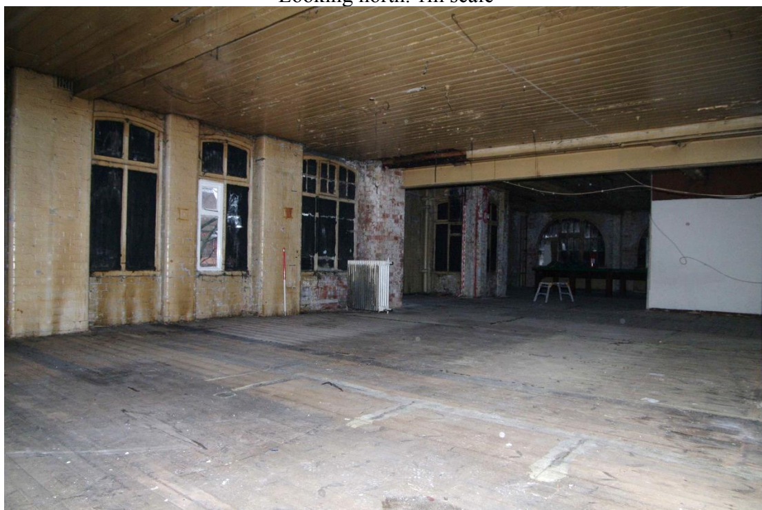
Figure 87 Third floor, rear range Looking north-west. 1m scale
