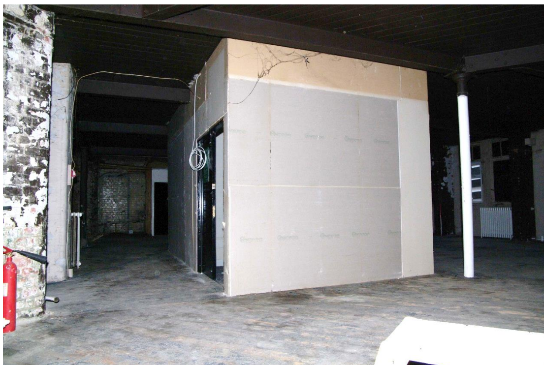
Figure 76 Second floor, stairwell Looking north-west
