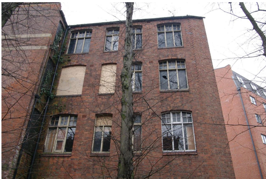
Figure 26 South-west facing elevation, rear range windows Looking north-east
