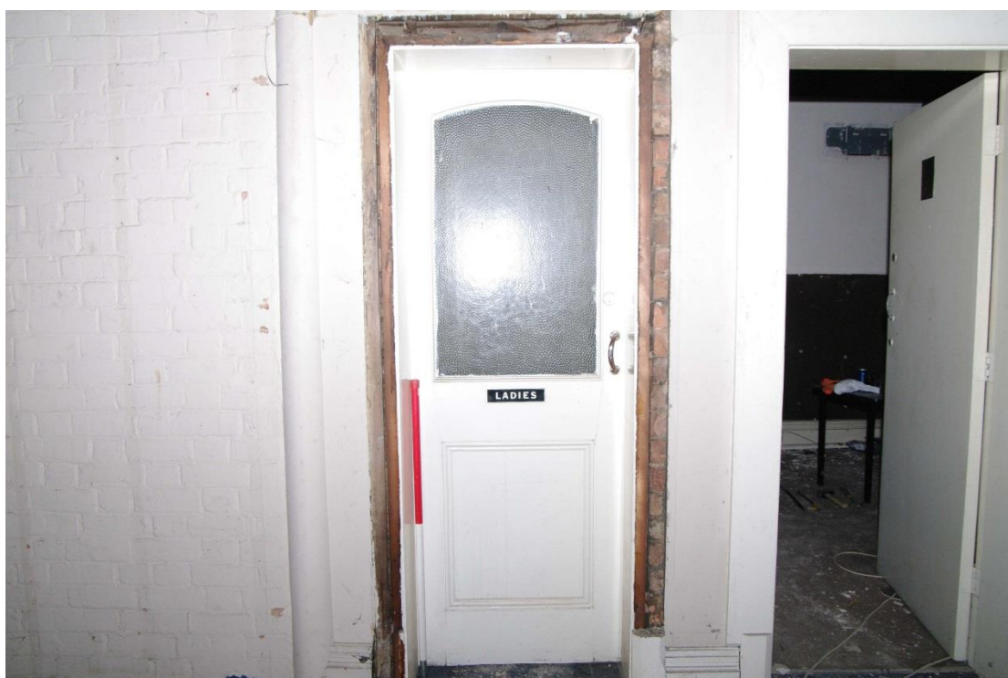
Figure 68 First floor, toilet door Looking south-west. 1m scale.
