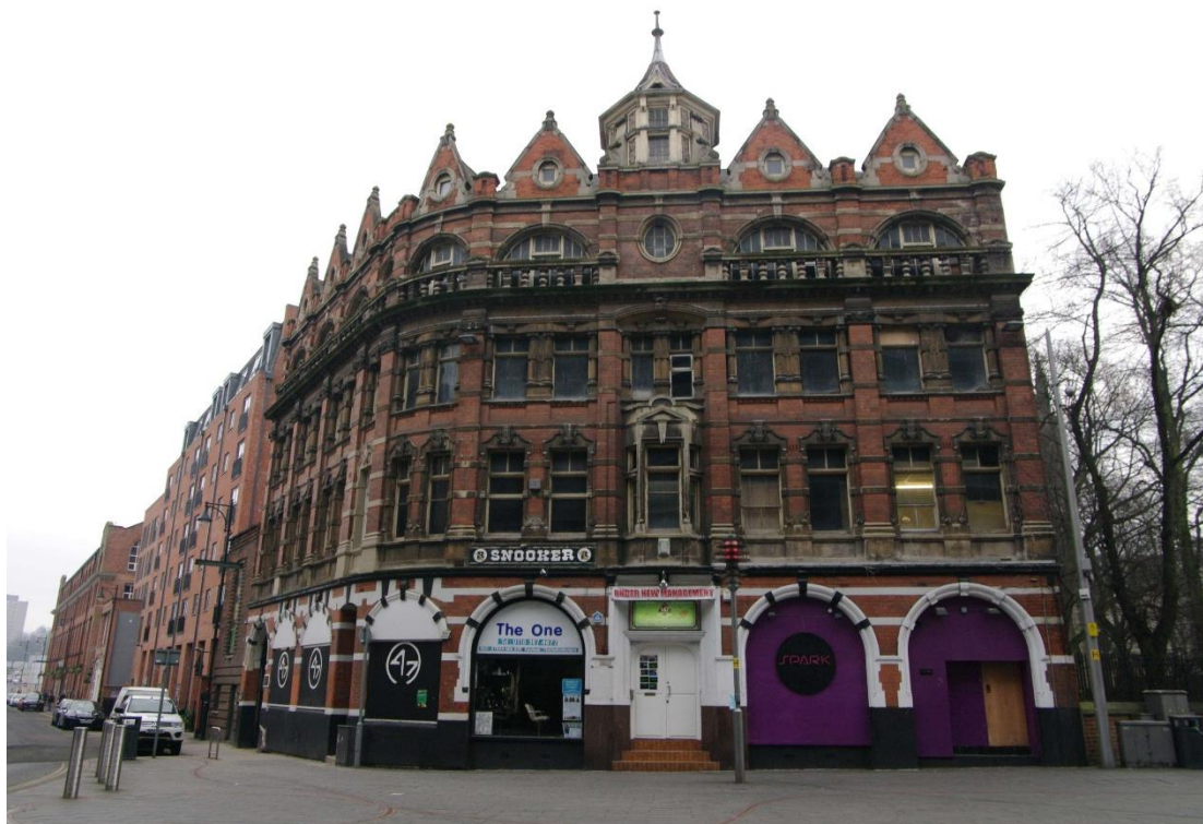
Figure 17 North-west facing elevation Looking south-east. Queen Street on left of picture
