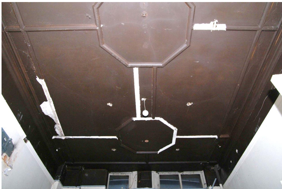
Figure 66 First floor, former reception ceiling Looking north
