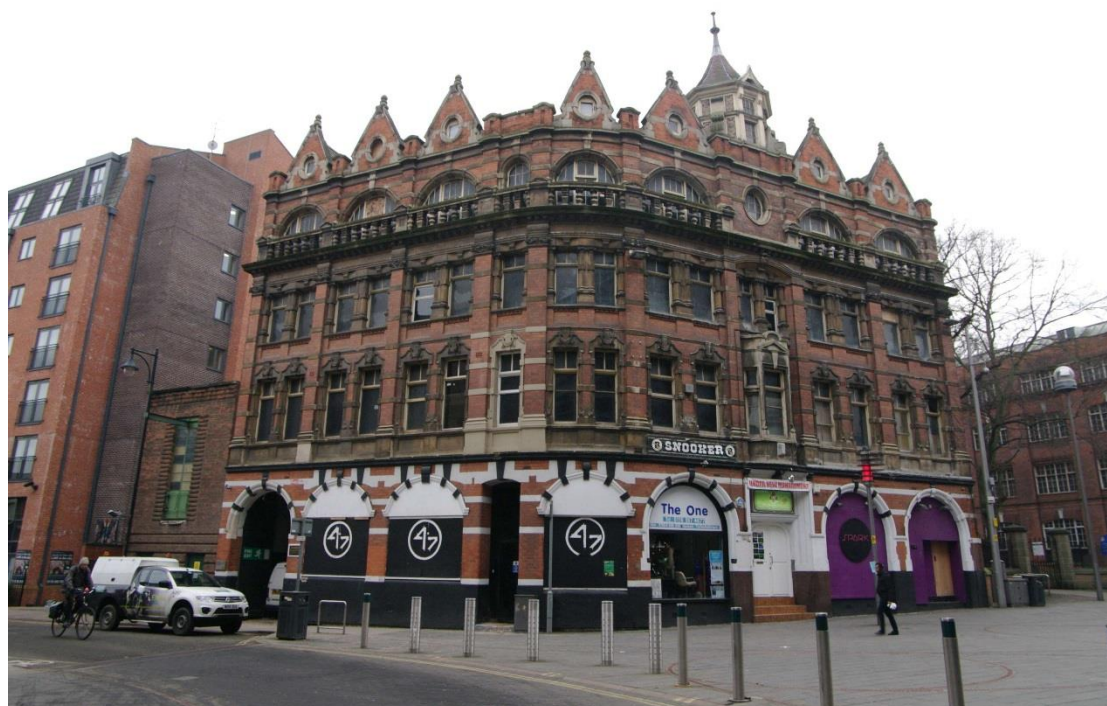
Figure 10 Principal façade, north-east and north-west facing elevations Looking south-west
