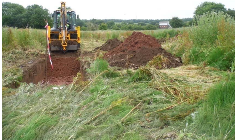
Figure 8: Excavating trench 13, looking east
