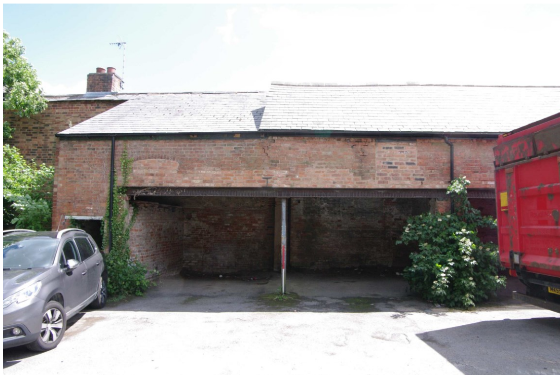
Figure 87 Outbuildings, north-west facing elevation, northern end Looking south-east
