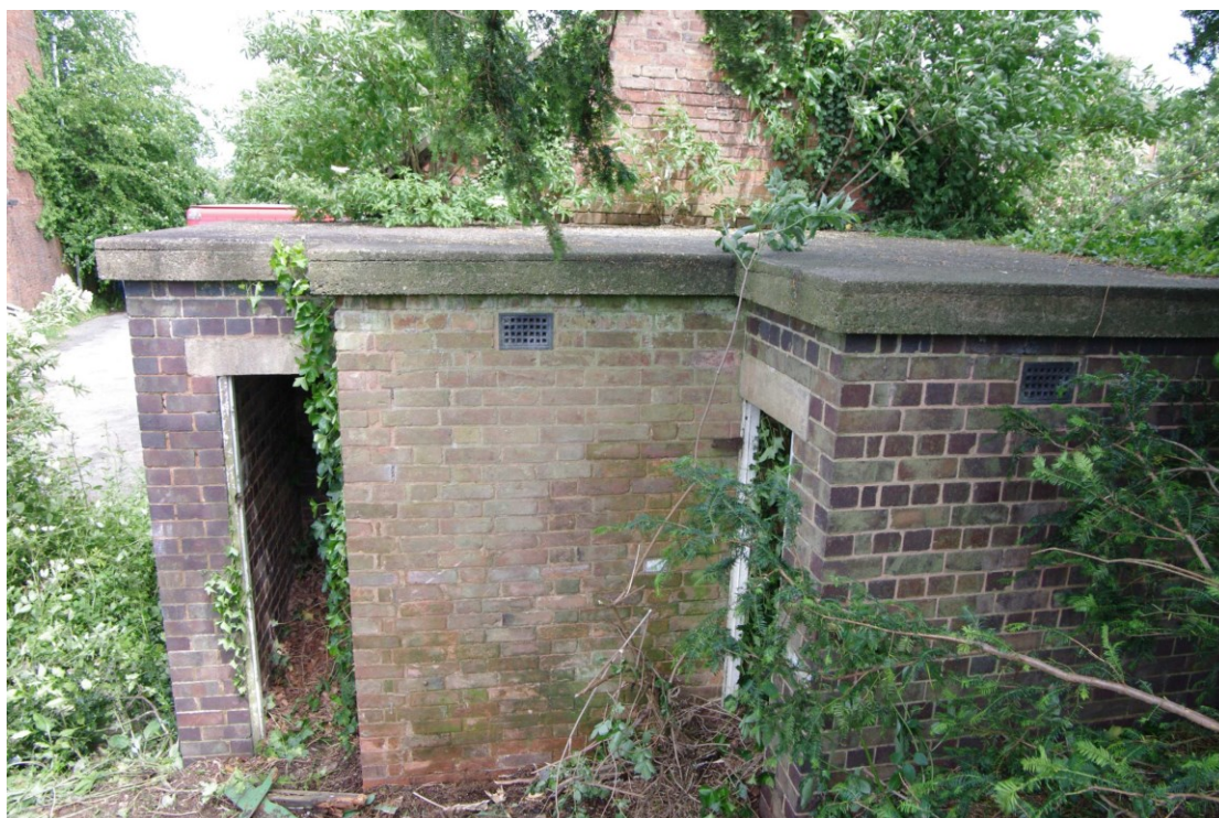
Figure 93 South-west facing elevation of air raid shelter Looking north-east
