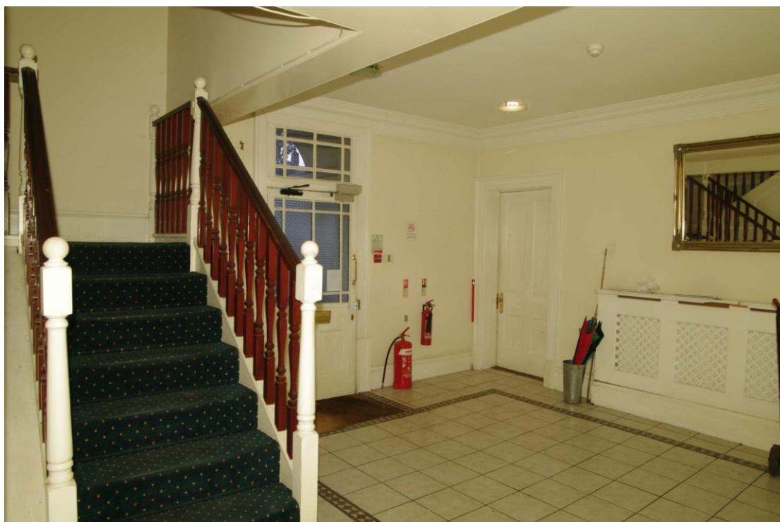
Figure 38 Room G1 Looking east. 1m scale
