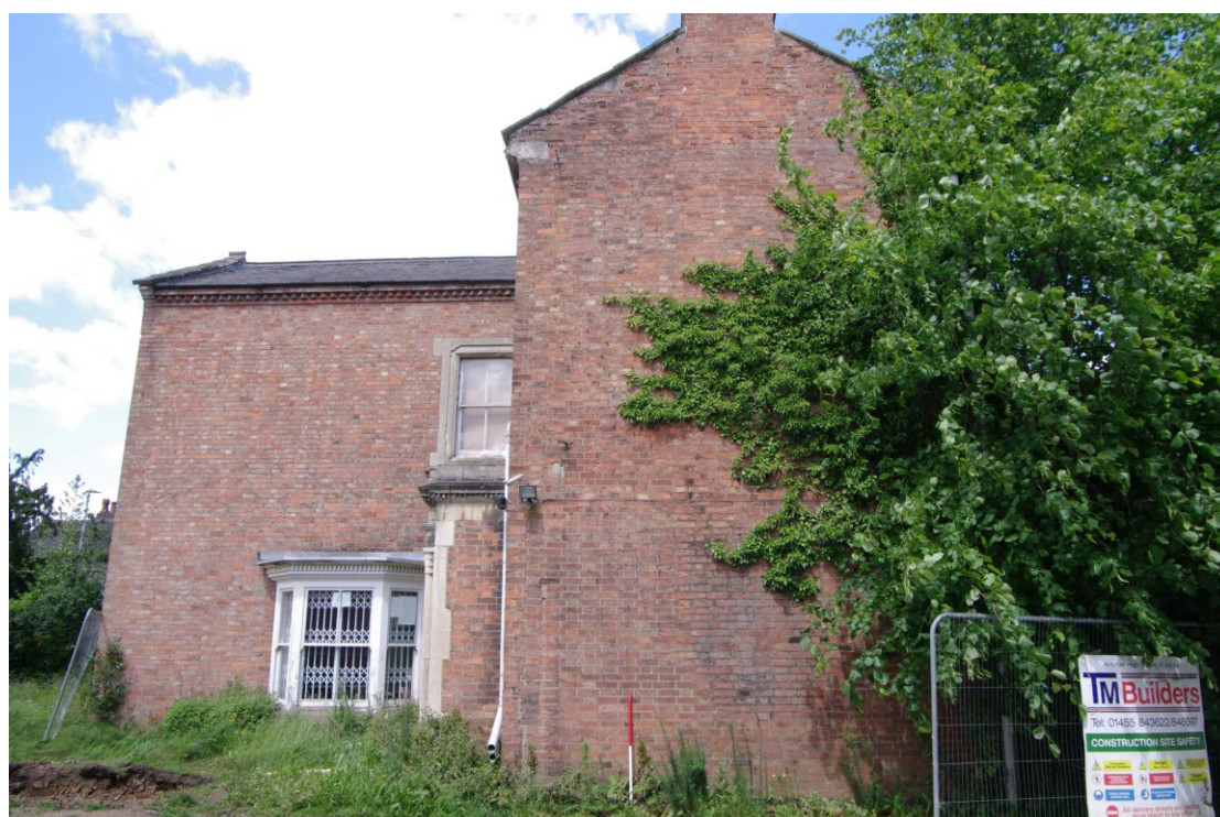
Figure 21 South-east facing elevation Looking north-west. 1m scale
