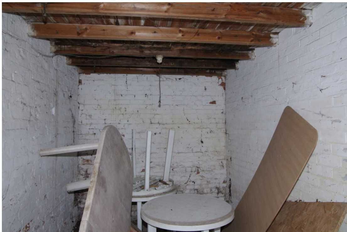
Figure 100 Outbuilding Room OB6 Looking south-east
