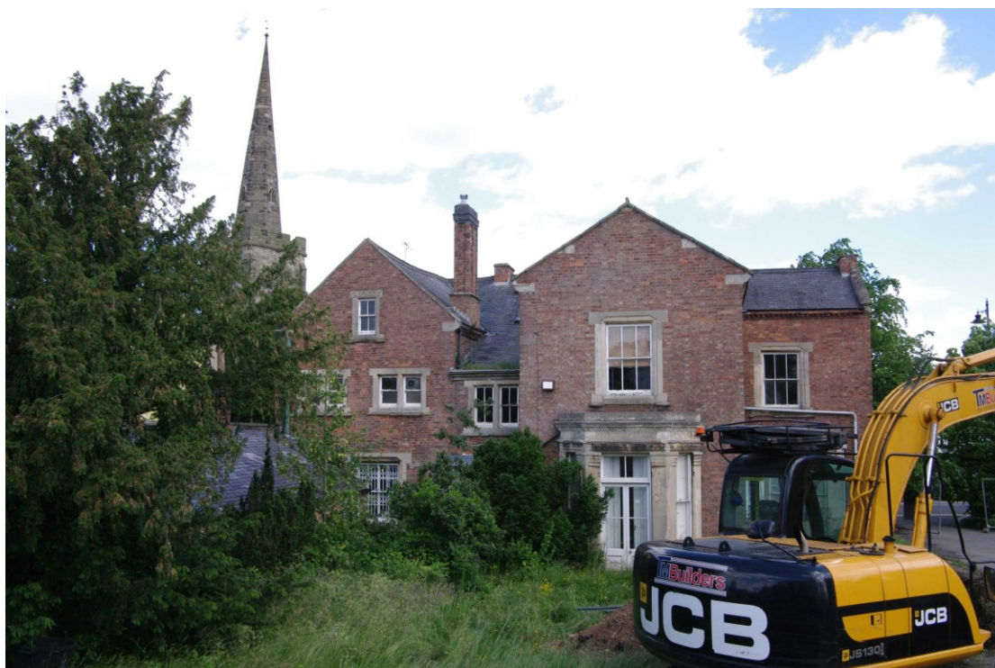
Figure 25 General view of south-west facing elevation Looking north-east
