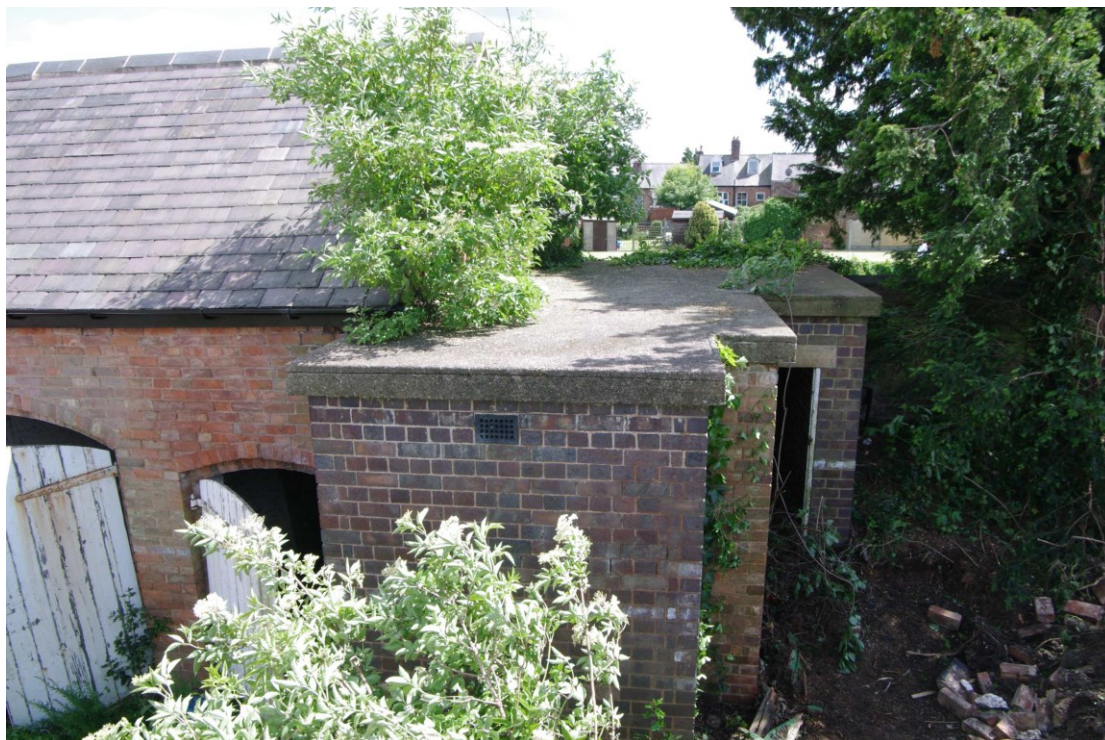
Figure 91 Air raid shelter at south-west end of outbuildings Looking south-east
