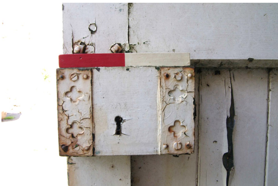
Figure 90 Door lock case on door of Room OB6 0.2m scale
