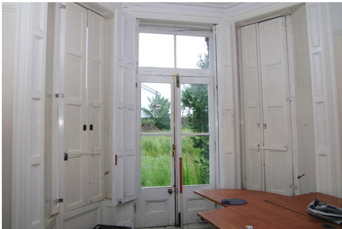
Figure 46 Room G3, doors to garden Looking west. 1m scale
