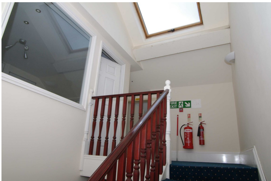
Figure 74 Room S1 Looking south-west. 1m scale. Door to S2 on left. Access to S4 corridor behind bannister
