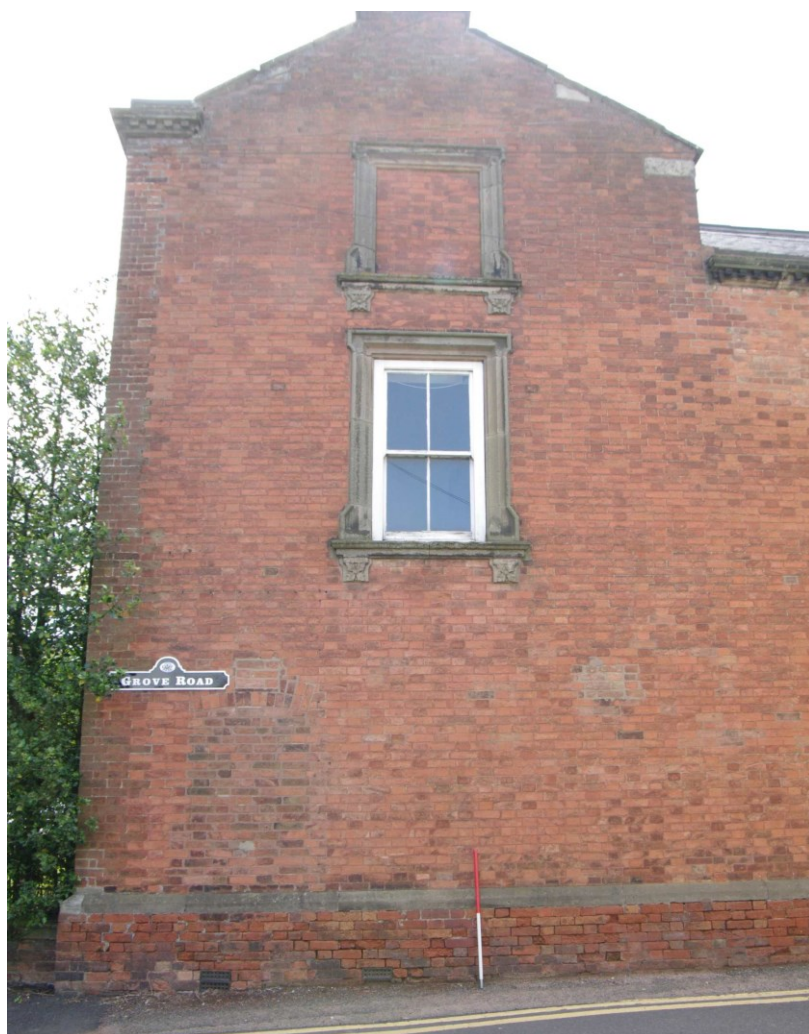
Figure 17 North-west facing elevation Looking south-east. 1m scale
