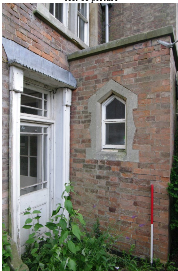
Figure 29 Infilled structure between the rear wings Looking north-east. 1m scale
