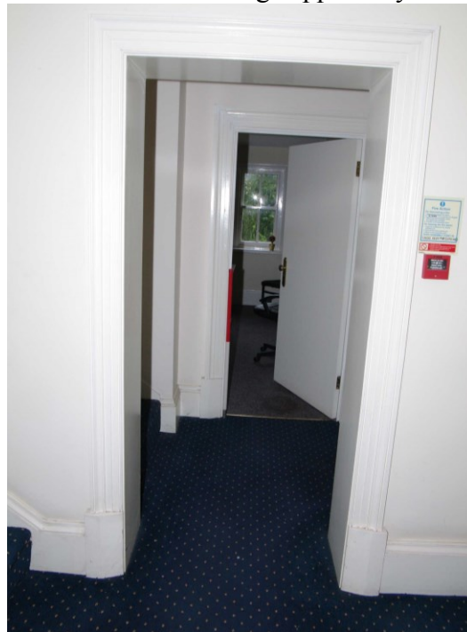
Figure 60 Room F1 doorway surround Looking south-west towards Room F2. 1m scale
