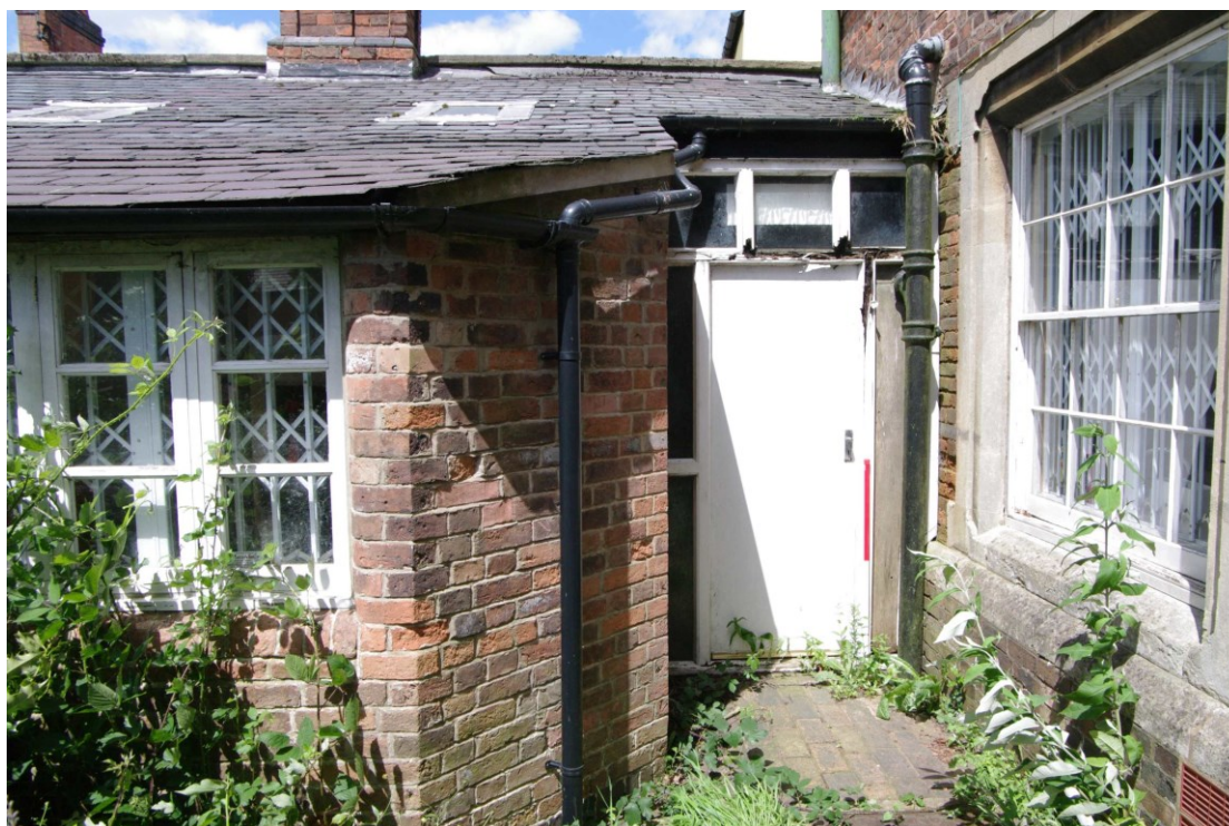
Figure 31 Single storey service range and junction with main house Looking north-west. 1m scale
