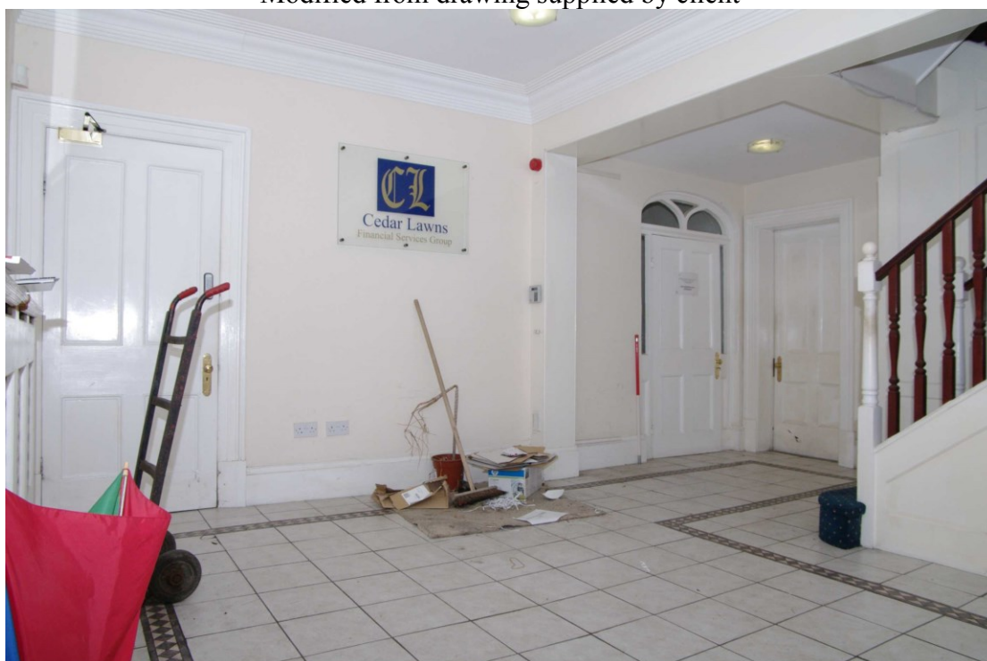
Figure 37 Room G1 Looking west. 1m scale
