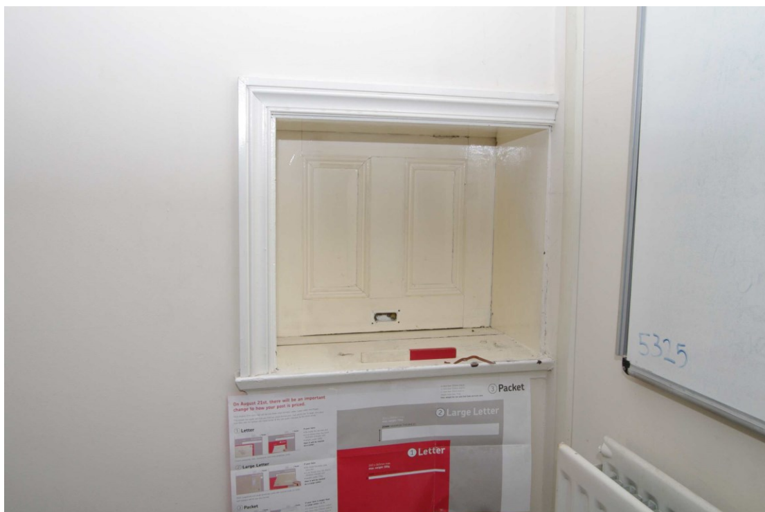
Figure 48 Room G3, serving hatch Looking north. 0.2m scale
