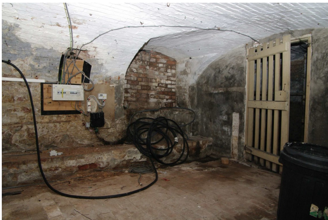
Figure 35 Cellar Looking north-east
