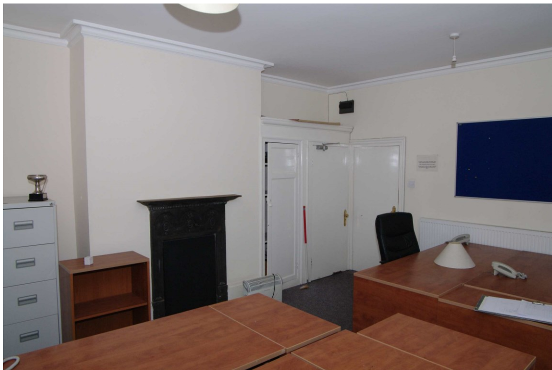
Figure 63 Room F4 Looking south. 1m scale. Right hand door goes to Room F3, middle door leads to room F1 landing, door to the side of the fireplace is the linen cupboard
