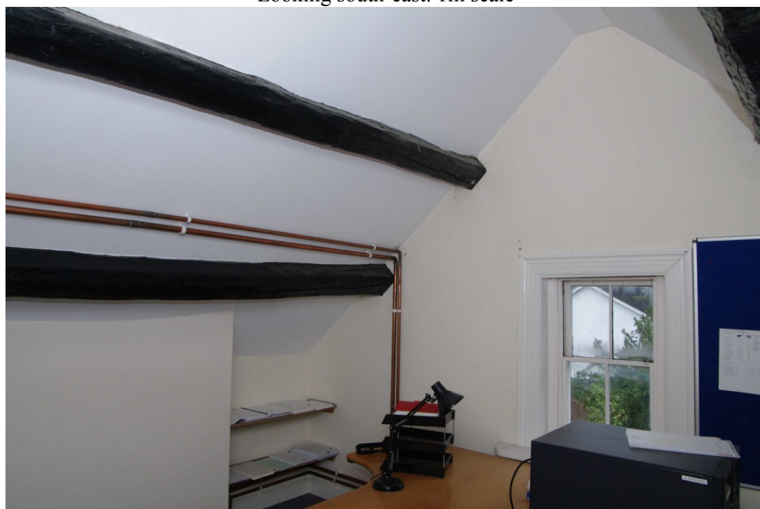
Figure 79 Room S5 Looking south
