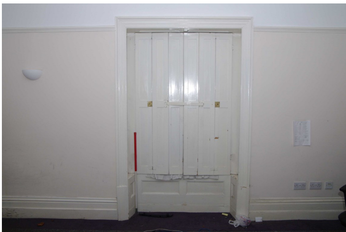
Figure 43 Room G2 window shutters Looking north-east. 1m scale
