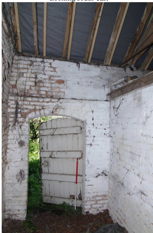
Figure 101 Outbuilding Room OB7 Looking south-west. 1m scale
