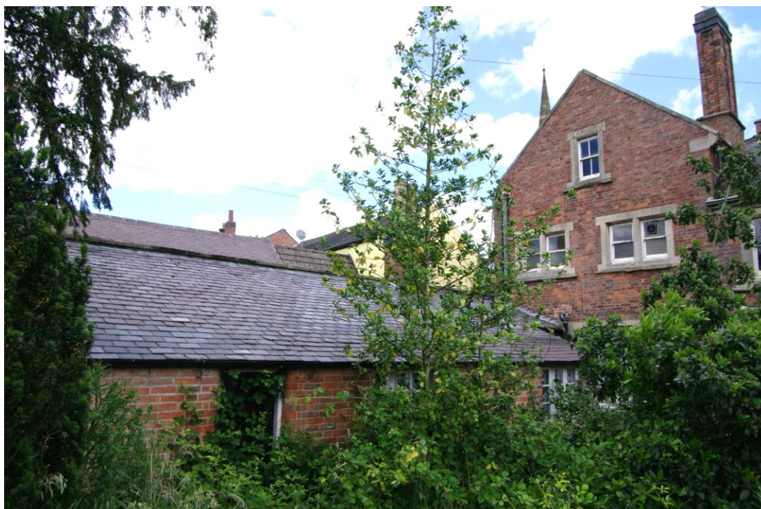
Figure 32 Single storey service range Looking north
