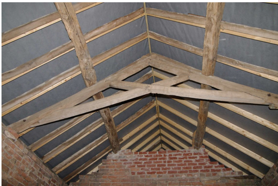
Figure 98 Roof structure of OB4 Looking south-west
