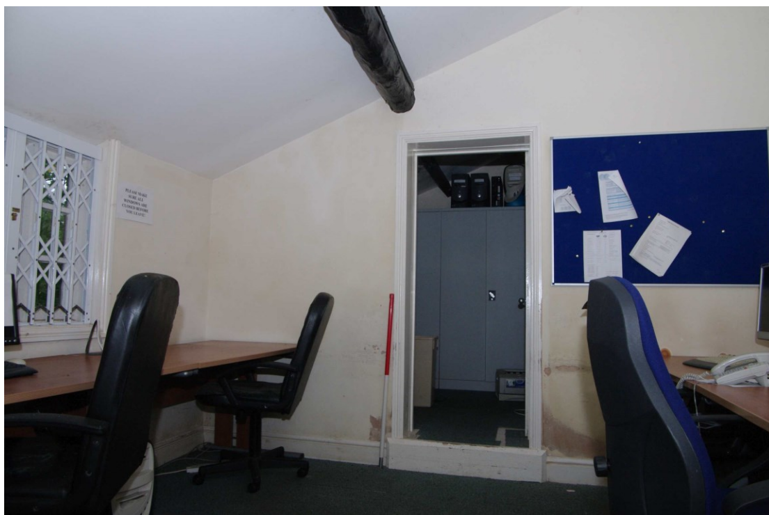
Figure 58 Room G8 Looking south-west. 1m scale. Note round section purlin
