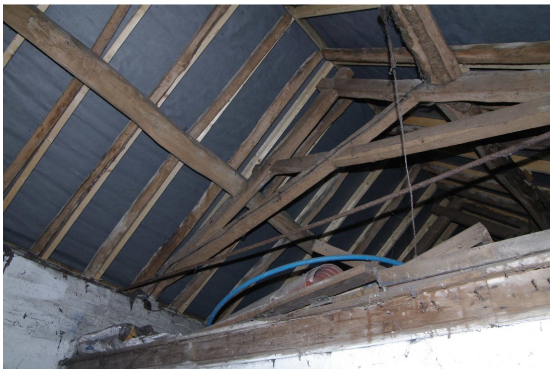
Figure 102 Roof support over Rooms OB5, 6 and 7 Looking north-east from Room OB7
