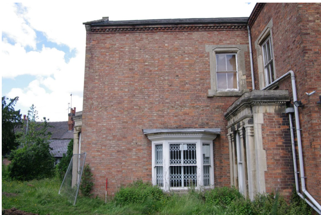
Figure 22 South-east facing elevation of rear south-east wing Looking north-west. 1m scale
