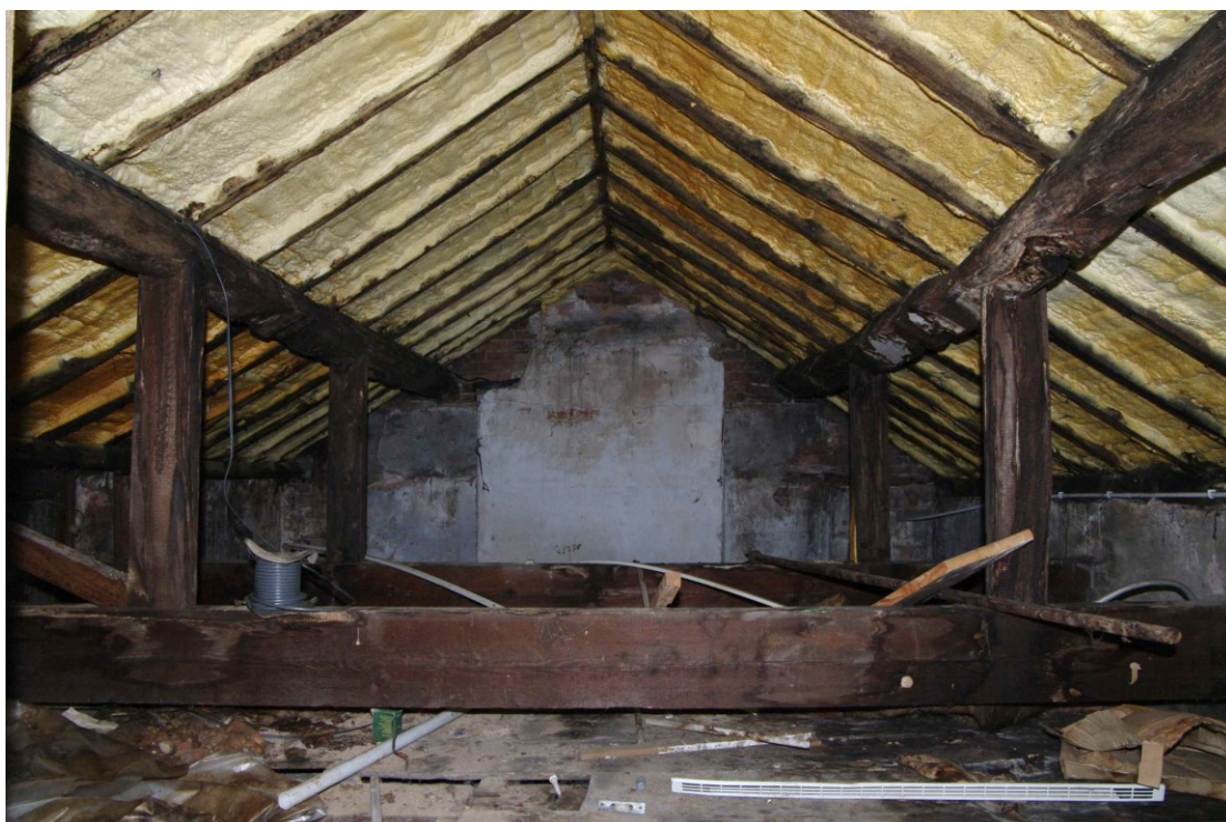
Figure 76 Room S3 Looking south-east through hatch from Room S2
