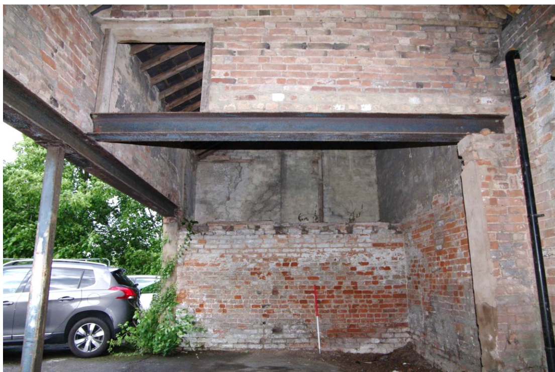
Figure 95 Outbuilding Room OB2 from OB3
