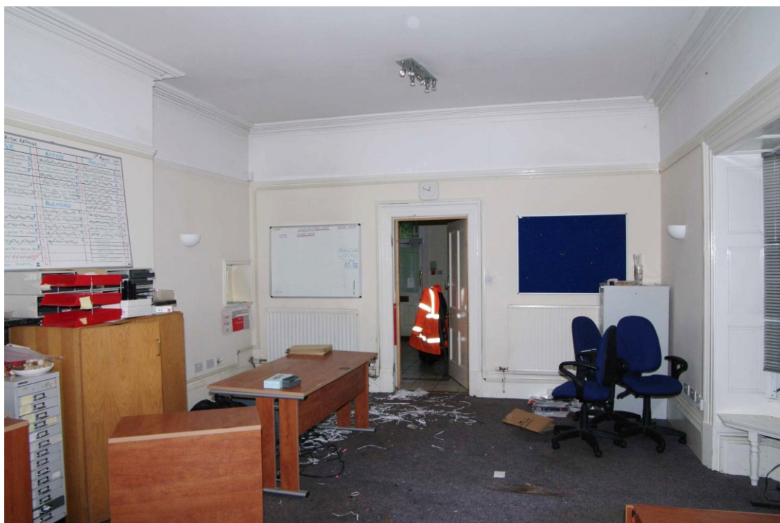
Figure 45 Room G3 Looking north-east. 1m scale
