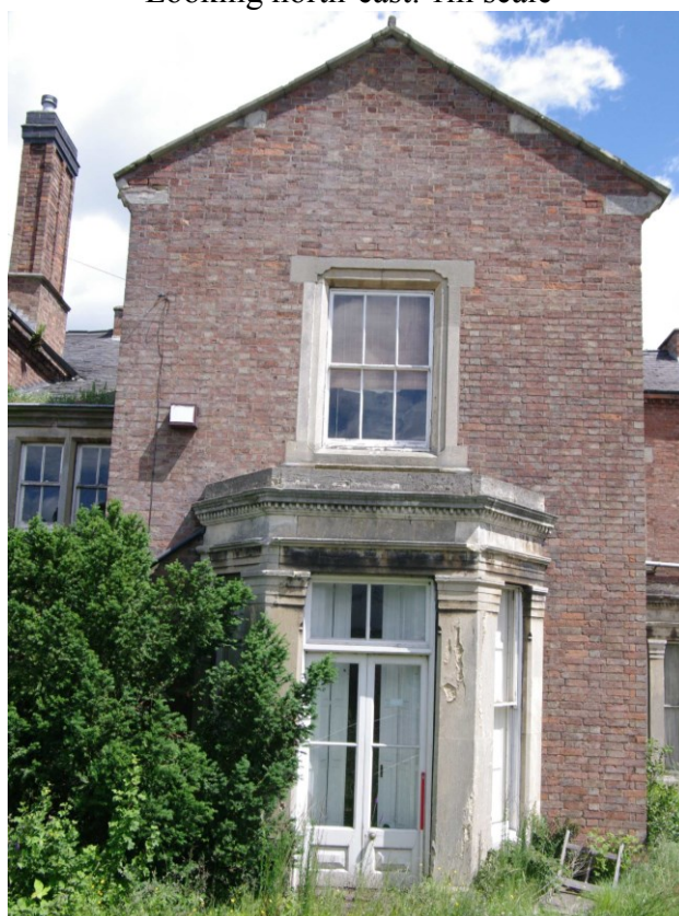
Figure 27 South-west facing elevation of SE rear wing Looking north-east. 1m scale
