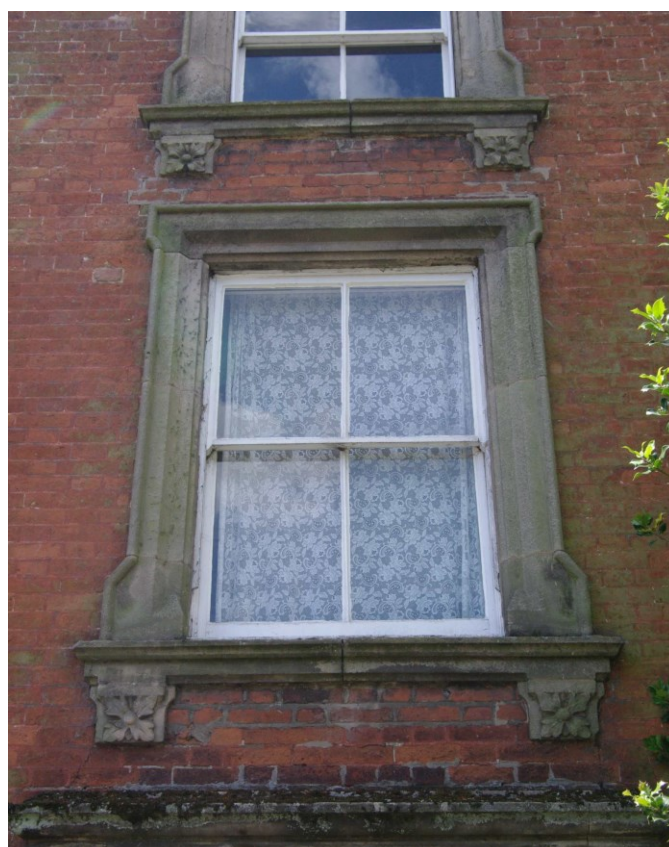
Figure 12 North-east facing elevation, first floor window detail
