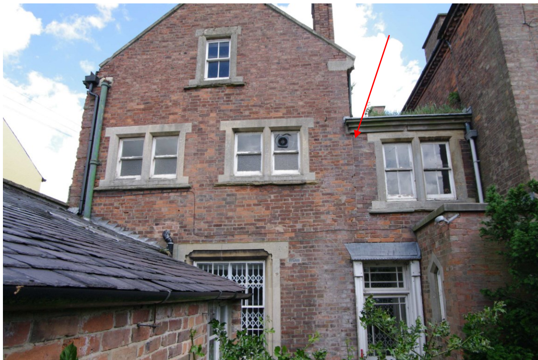
Figure 28 South-west facing elevation of SW rear wing and infill between wings Looking north-east. Note brick joint of infill (arrowed). Single storey service range on left of picture
