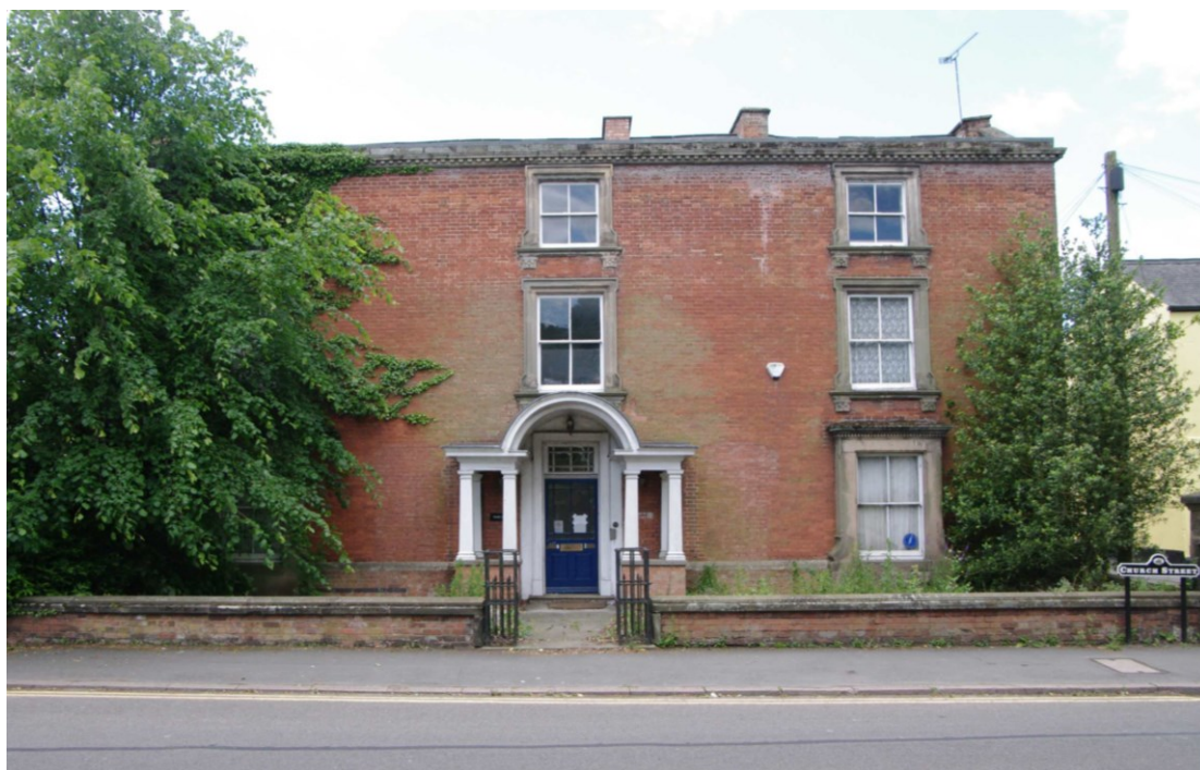
Figure 11 North-east facing elevation of main house Looking south-west
