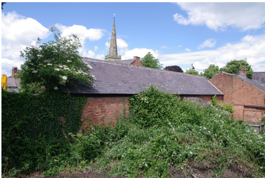
Figure 94 Outbuildings, south-east facing elevation Looking north
