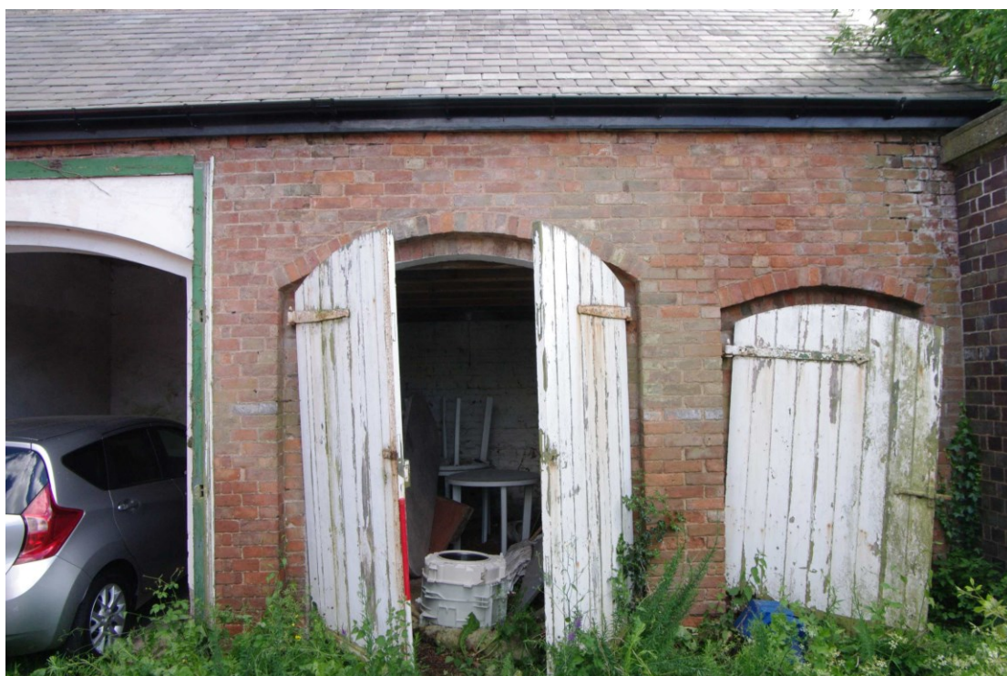
Figure 89 Outbuildings, north-west facing elevation, southern end Looking south-east. 1m scale
