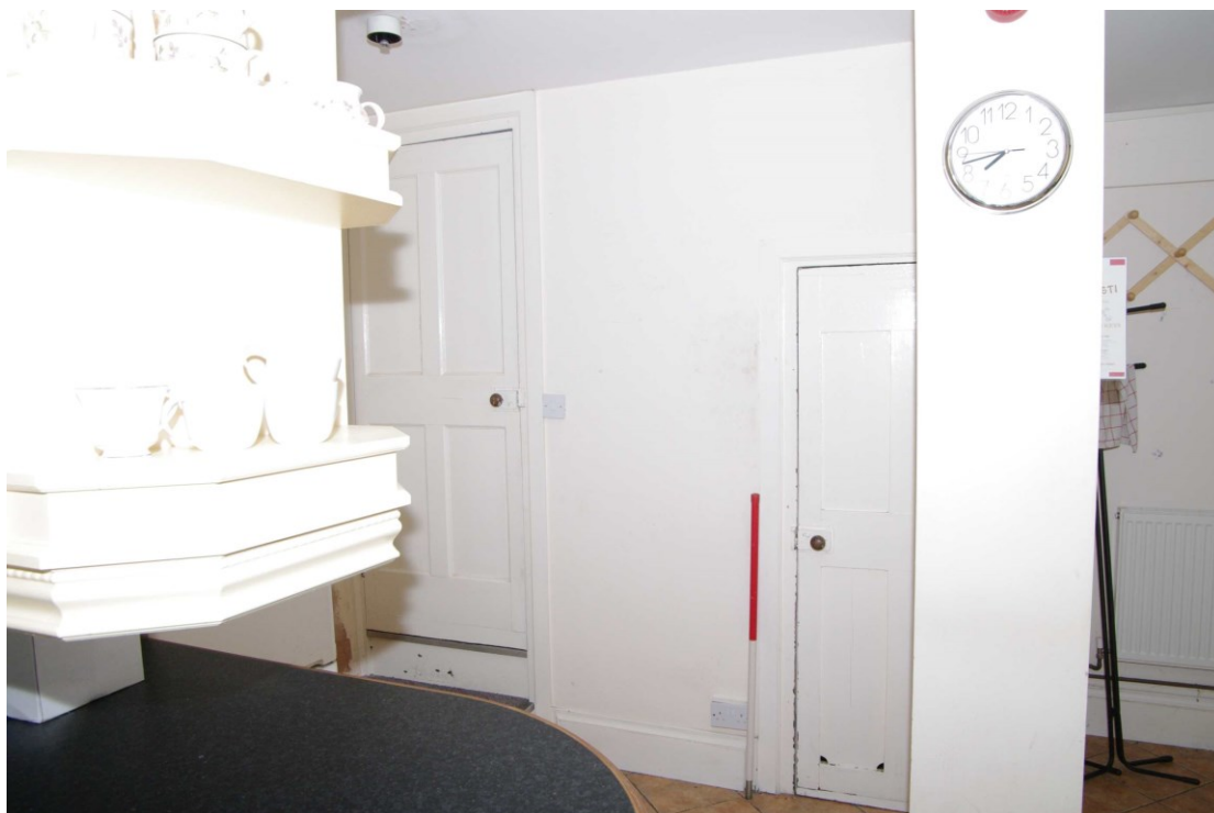
Figure 54 Room G6 Looking north. 1m scale. Doors to service stairs on left
