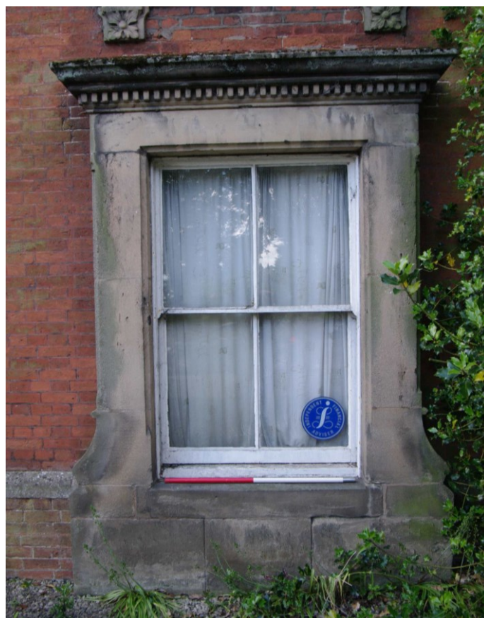
Figure 13 North-east facing elevation, ground floor window 1m scale
