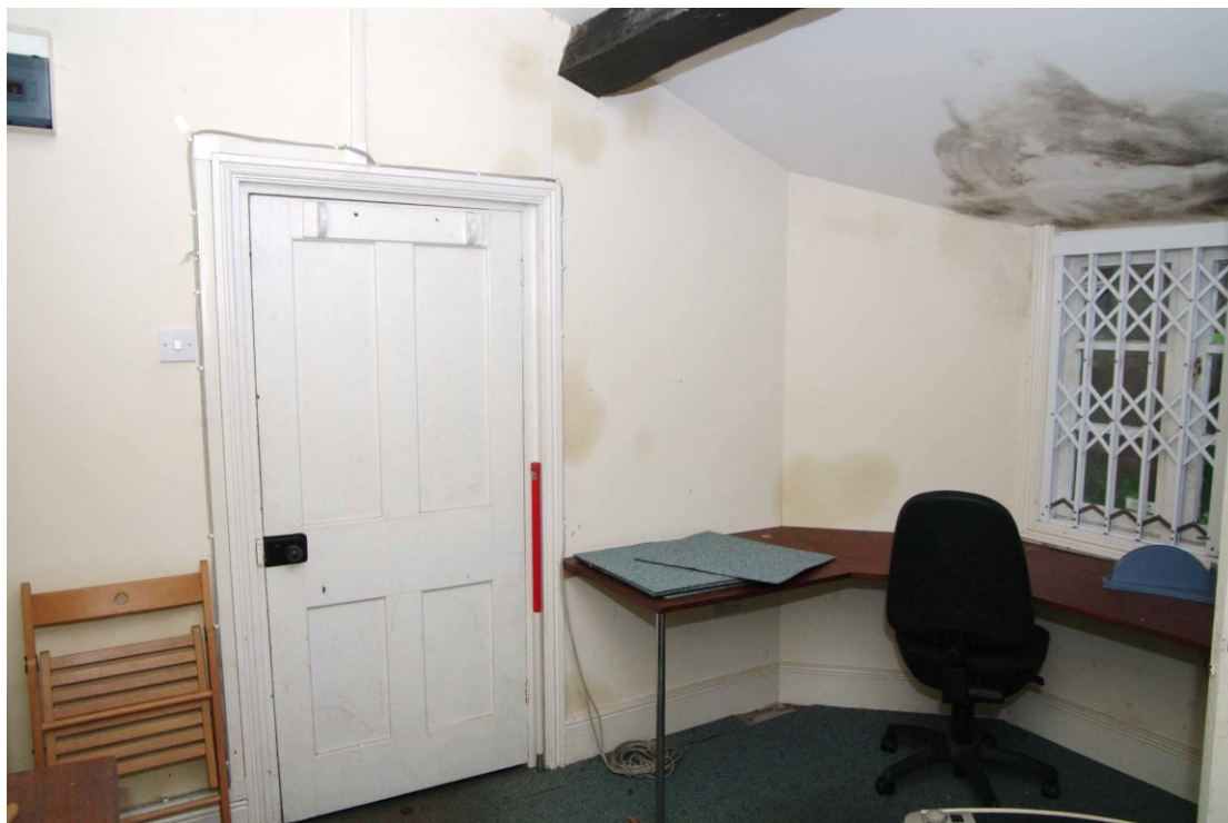
Figure 56 Room G7 Looking north-east. 1m scale
