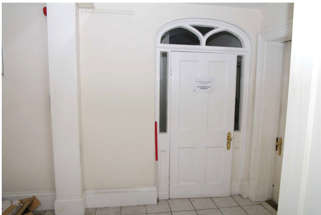
Figure 40 Room G1 door to service range Looking south-west. 1m scale
