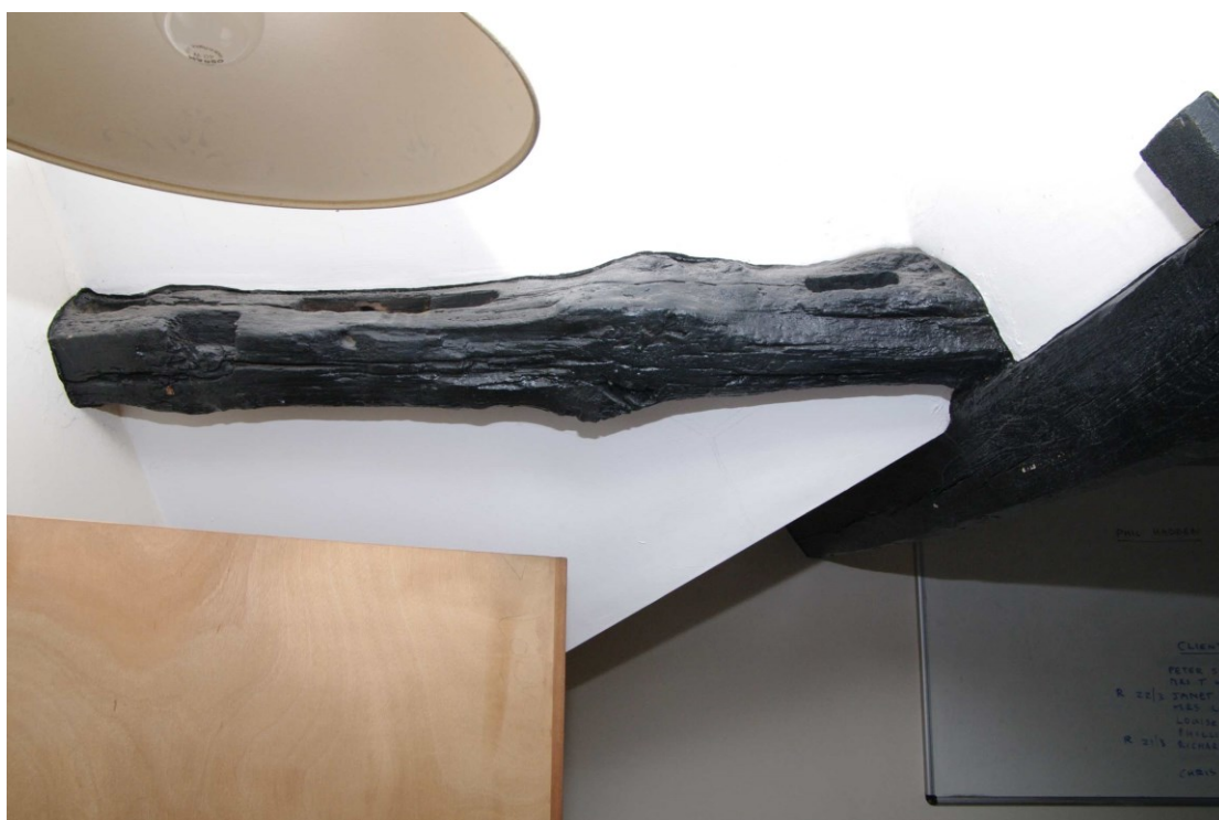
Figure 83 Purlins in Room S6 Looking north-west
