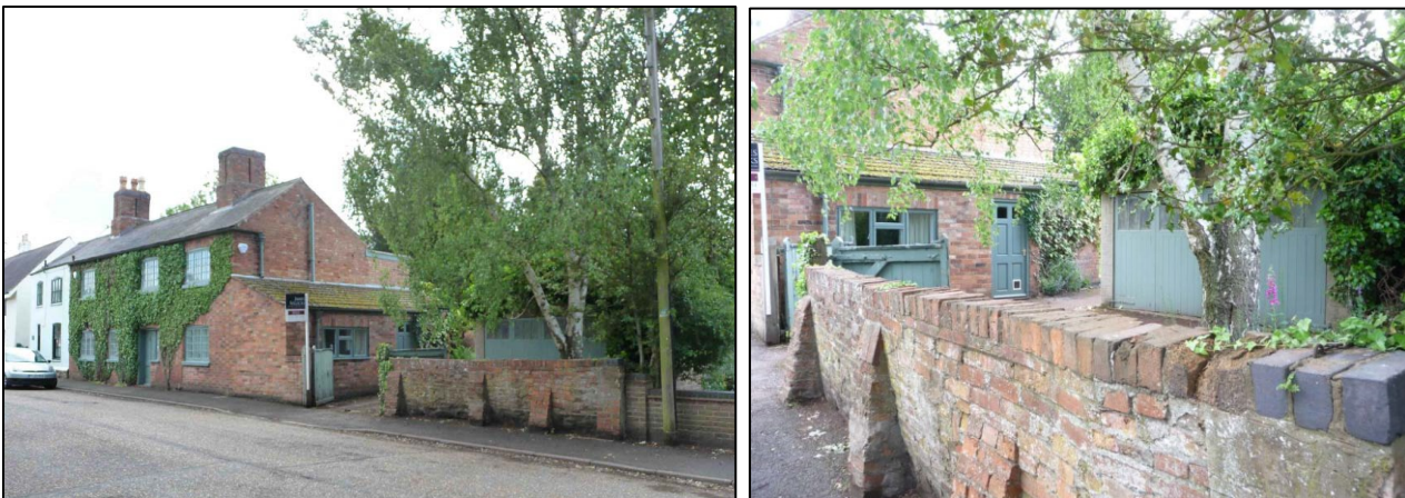
Figure 8. Photographs of the development site taken in 2011
