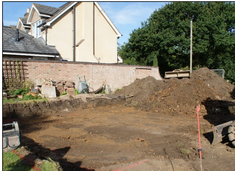
Figure 10. Footprint of the new building after removal of overburden, looking west.
