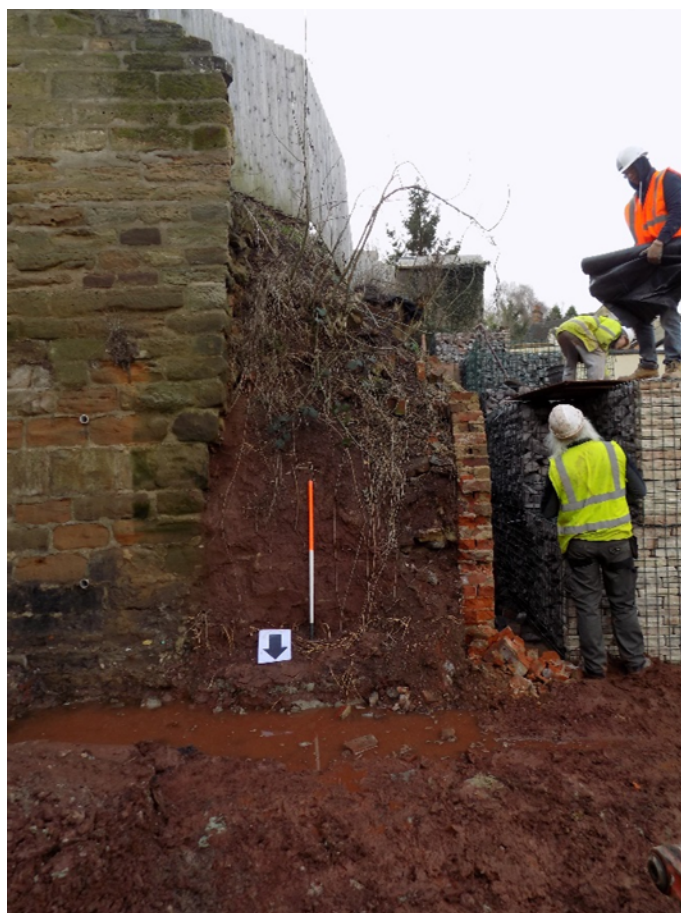
Figure 22: Area of bank and wall to be removed prior to excavation.
