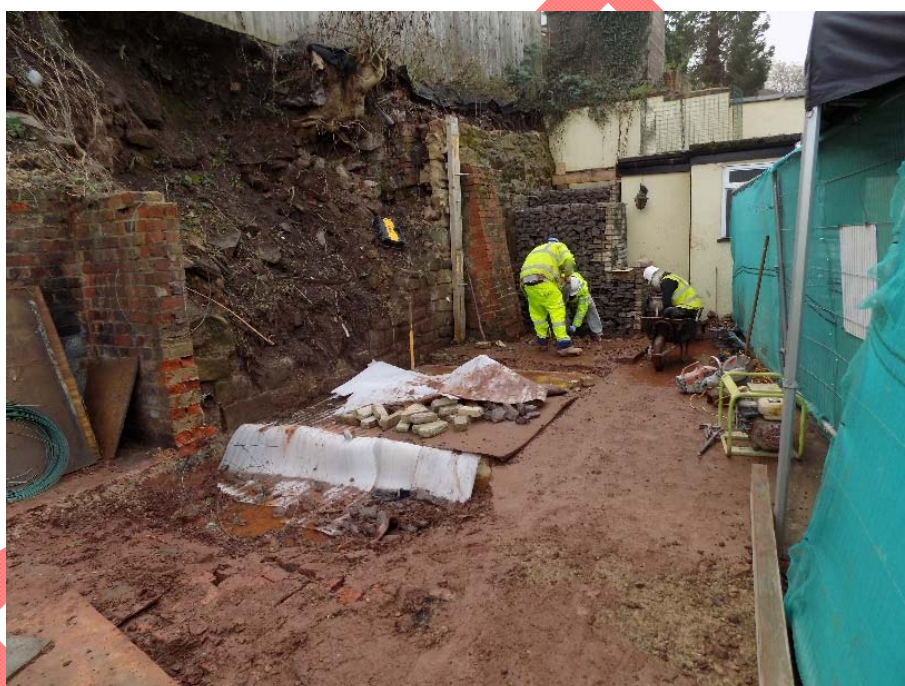
Figure 19: Area for excavation for the positioning of retaining gabions
