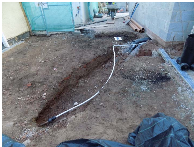
Figure 16: Excavated ground to the western side of the new cellar building.
