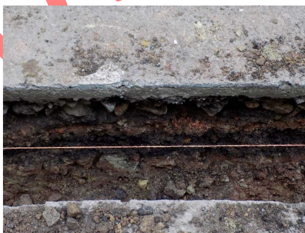
Figure 18: Trench showing the truncated top layer of ground excavated for drainage to the north of the existing public house.
