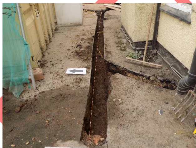
Figure 17: Trench excavated to the northern side of the existing public house for drainage.
