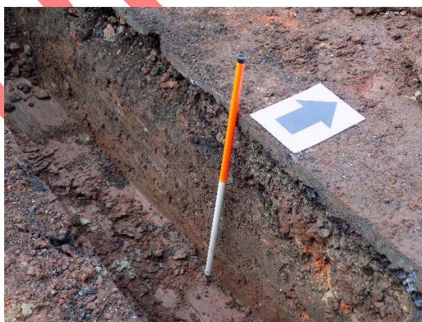
Figure 8: Northernmost foundation trench for the proposed new cellar building, post excavation. Photograph clearly showing how the disturbed top layer overlays the natural red clay substratum.
