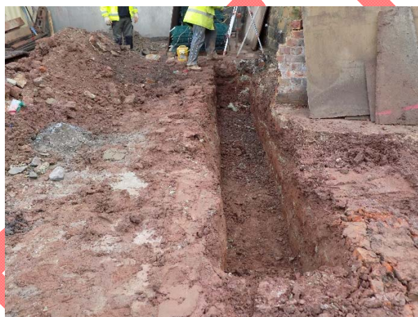
Figure 7: Southernmost Foundation trench for the new cellar building during excavation.
