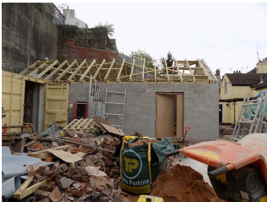
Figure 13: New cellar block under construction.
