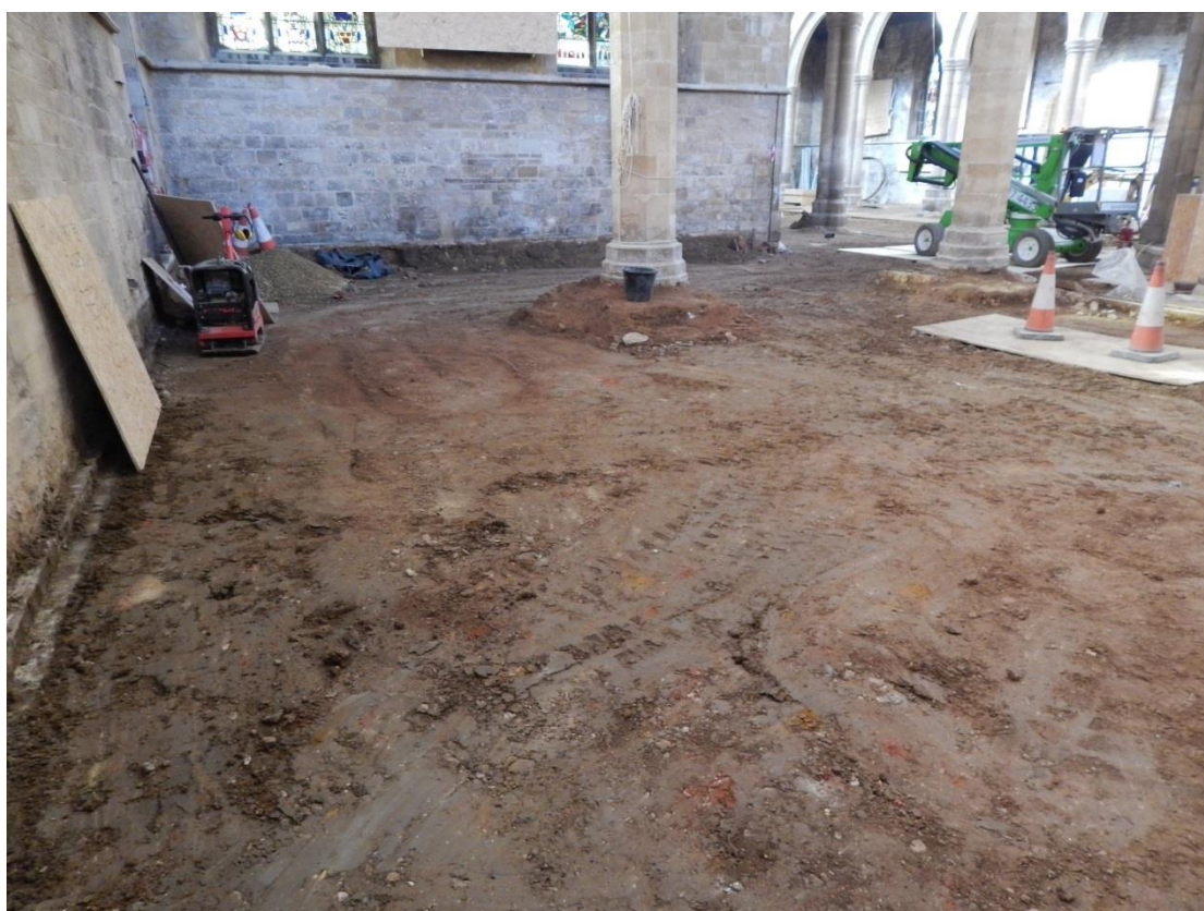
Figure 18: The south transept area after stripping and compacting, looking north-west
