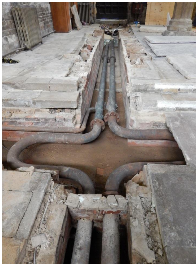
Figure 4: Ledgers removed over heating system in north transept, looking north
