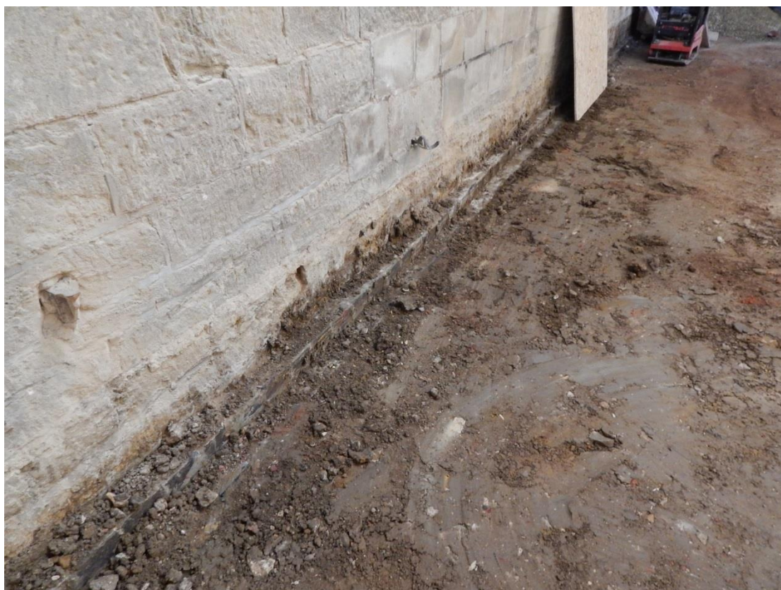
Figure 17: Blue bricks underpinning south wall of south transept, looking south-west
