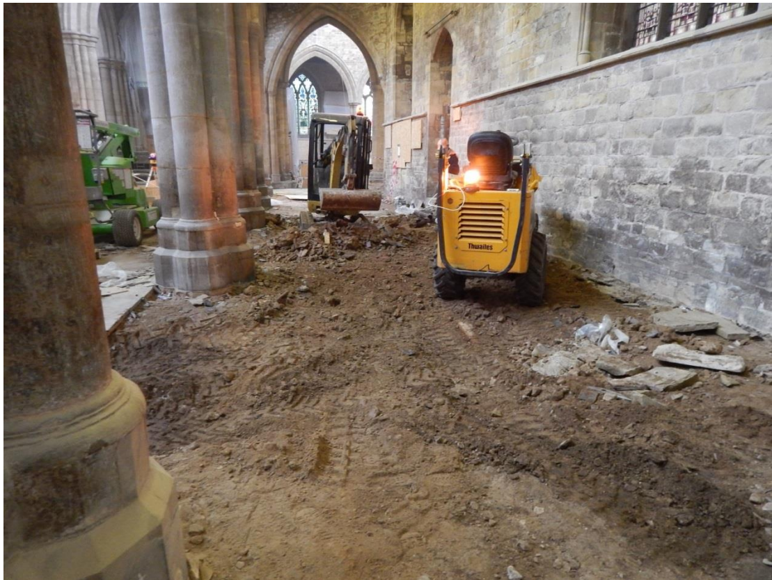
Figure 5: Work in progress within the nave, south aisle, looking east
