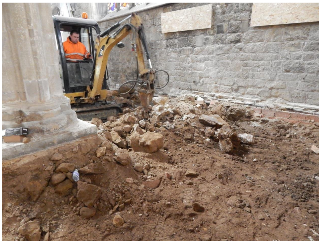
Figure 37: Work in progress on removal of screen foundation, looking north-west
