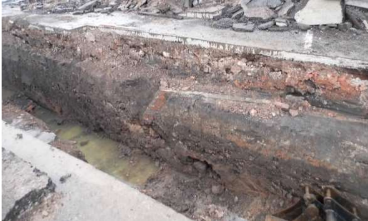
Figure 5: Trench 1: Terraced house boundary wall, looking north
