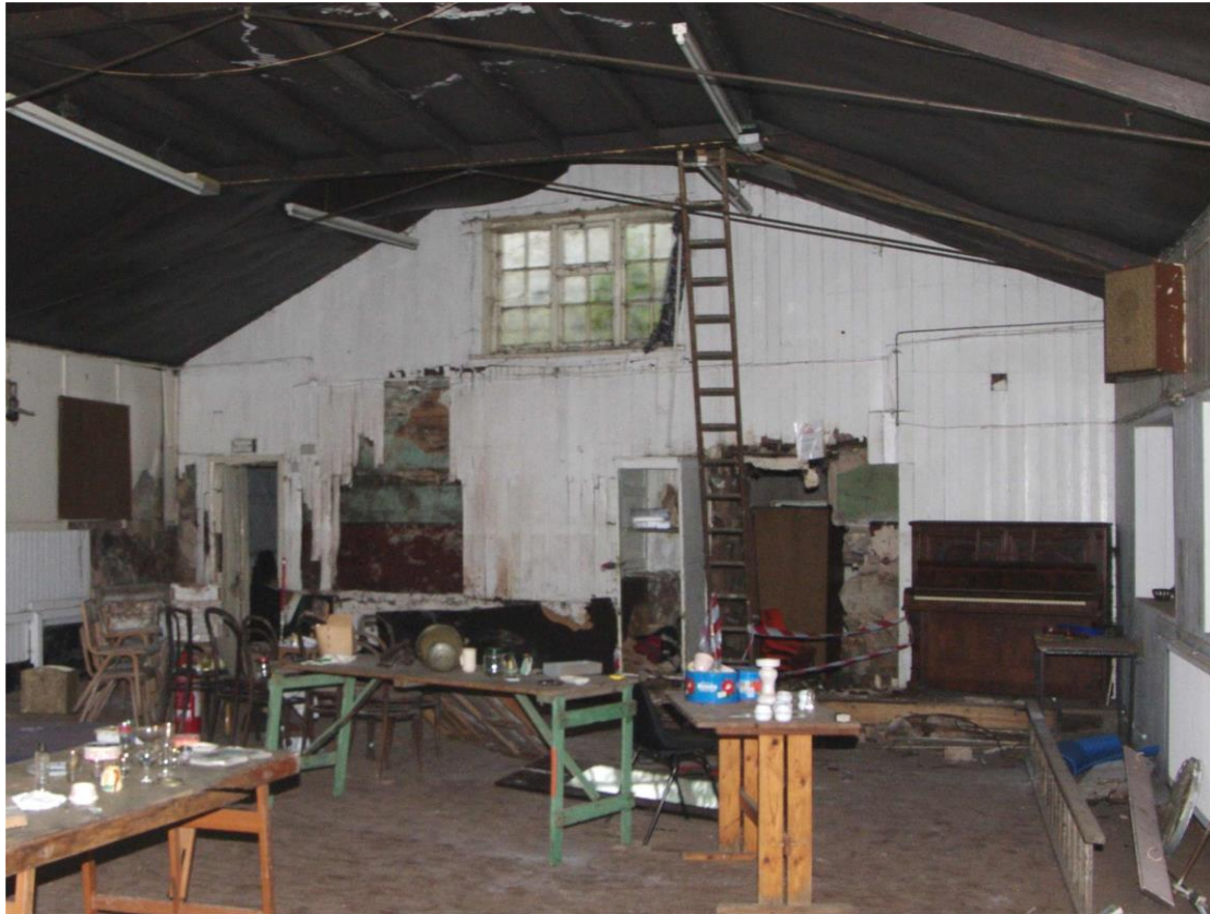
Figure 27 East end of hall Looking east.
