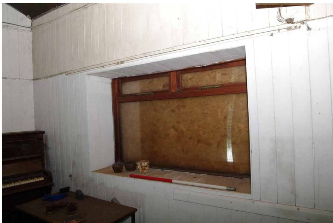
Figure 24 Main hall, south windows Looking south-east. 1m scale
