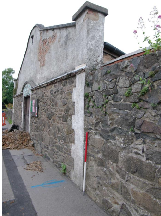
Figure 9 Decorative quoins applied to the west facing wall Looking north-east. 1m scale
