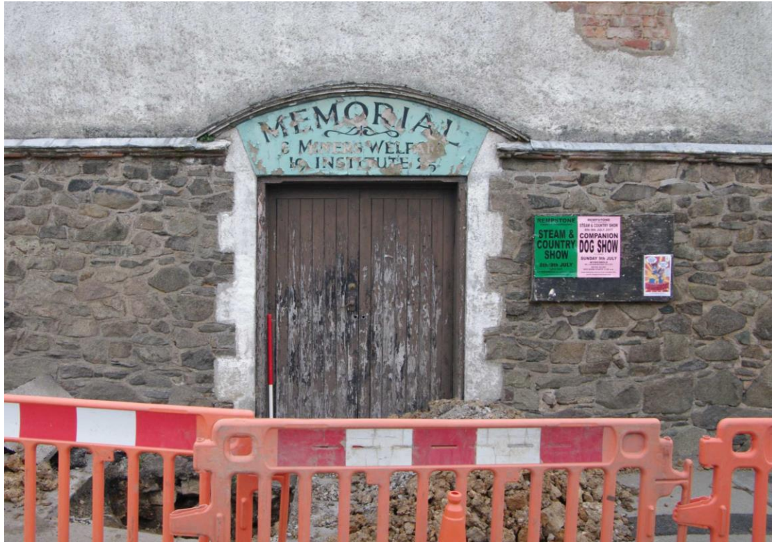
Figure 10 West facing elevation front doors Looking east. 1m scale
