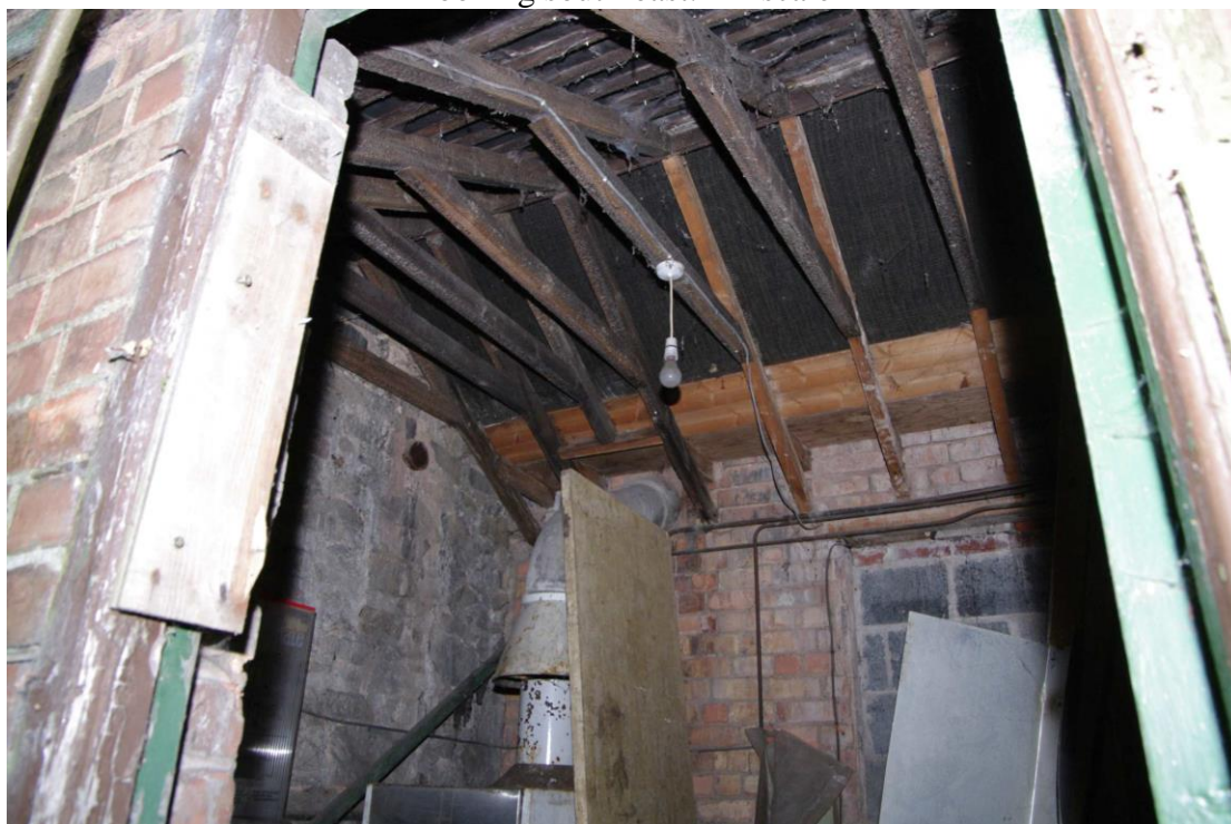
Figure 17 Inside the boiler house Looking north-east
