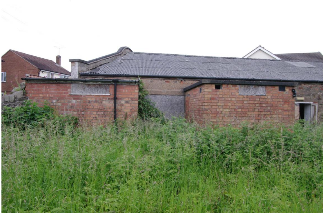
Figure 14 Toilet block extensions Looking north
