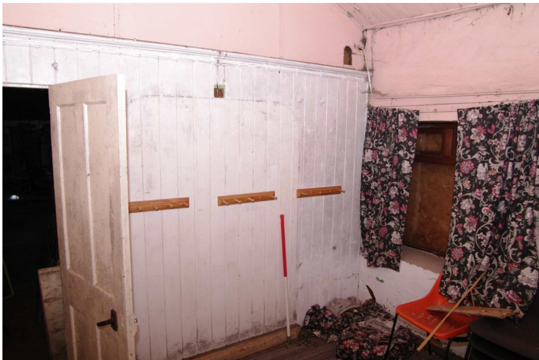
Figure 26 Cloakroom at west end of hall Looking south-east. 1m scale
