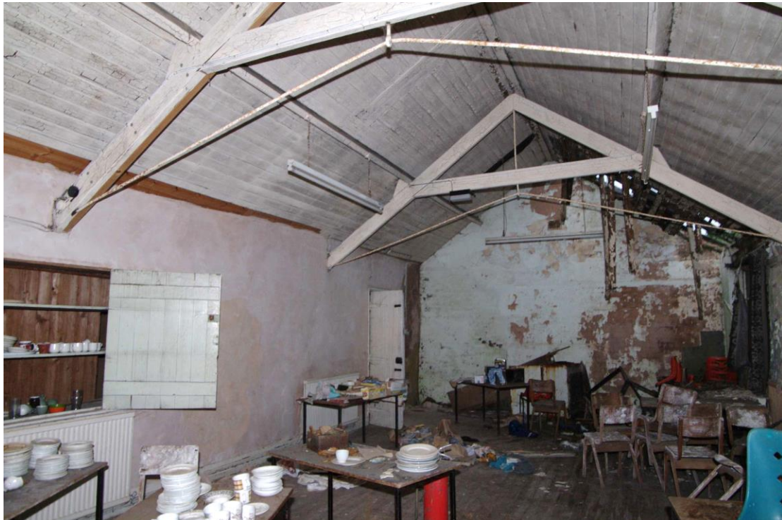
Figure 31 Canteen Looking north. Doorway to storeroom in left hand corner
