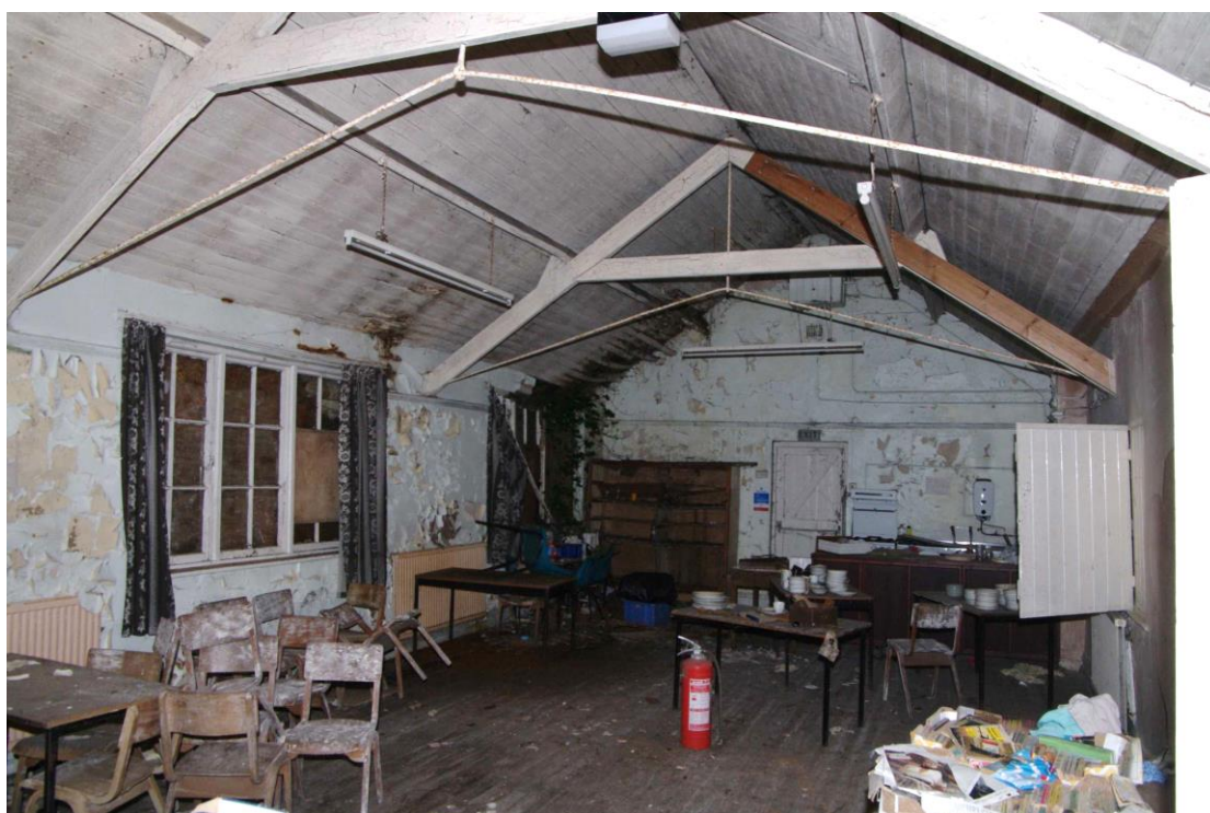
Figure 30 Canteen Looking south. Door to car park in centre of picture
