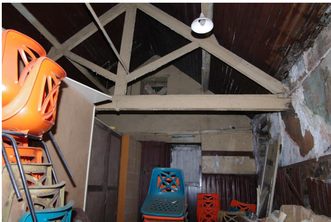
Figure 29 Storeroom, main room Looking south
