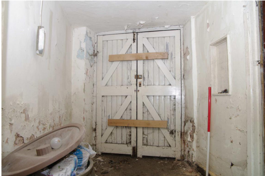
Figure 19 Entrance vestibule Looking west towards external doors. 1m scale
