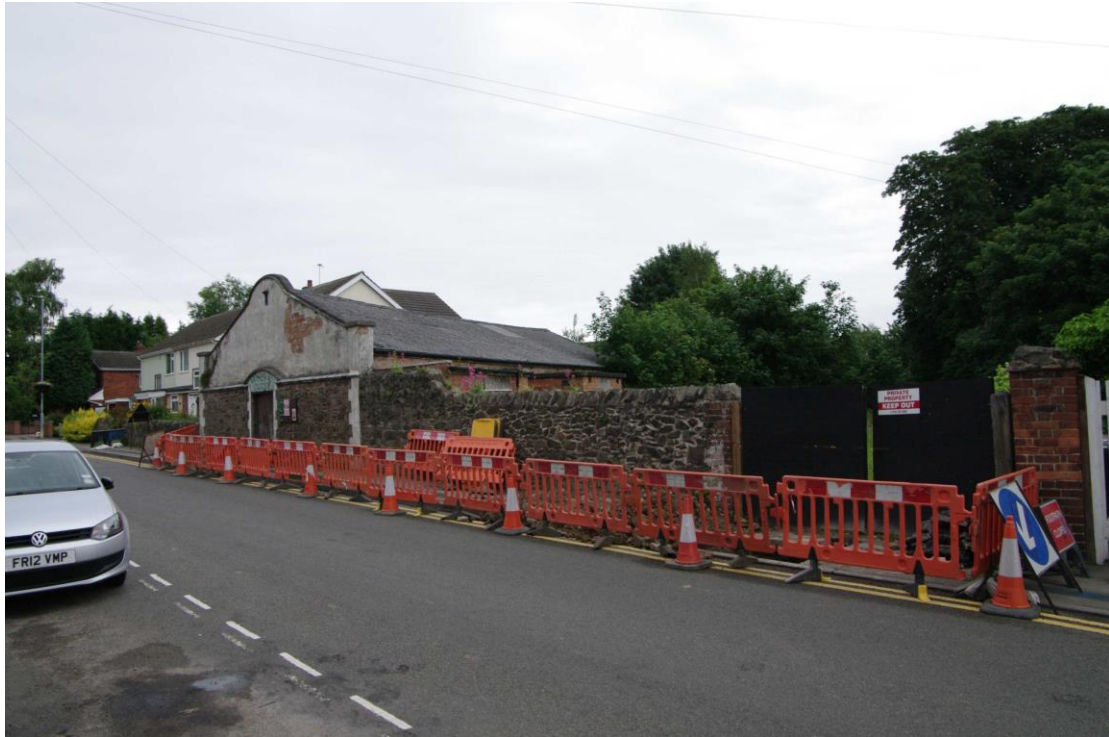
Figure 8 West facing elevation and boundary wall Looking north-east
