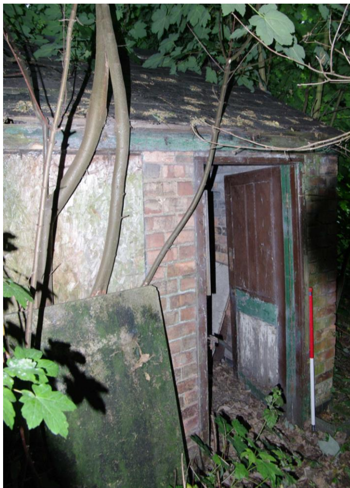
Figure 16 Boiler house Looking south-east. 1m scale
