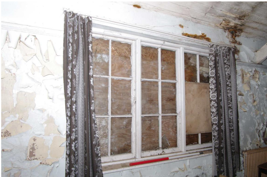
Figure 32 Canteen window detail Looking south-east. 1m scale
