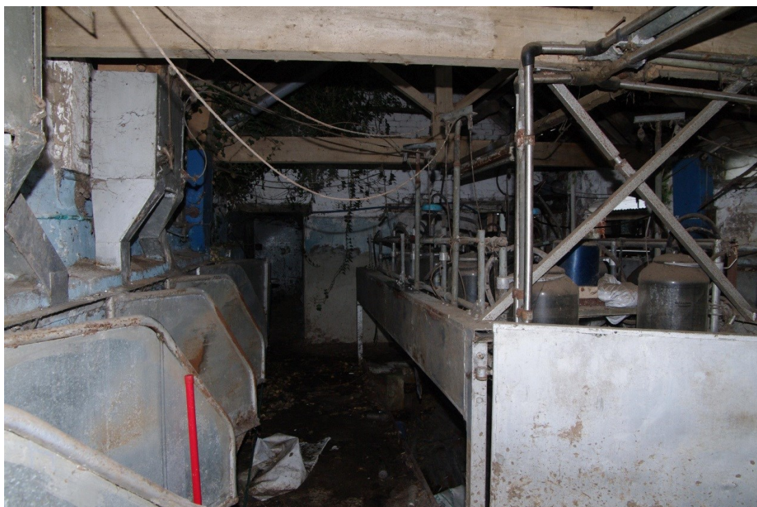
Figure 21: Barn A, milking parlour Looking east
