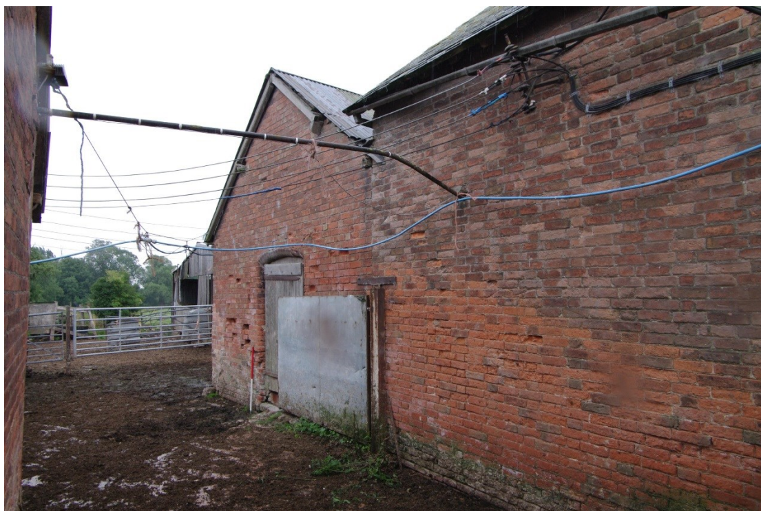
Figure 32: Barn B, north facing elevation (east end) Looking south-east. 1m scale
