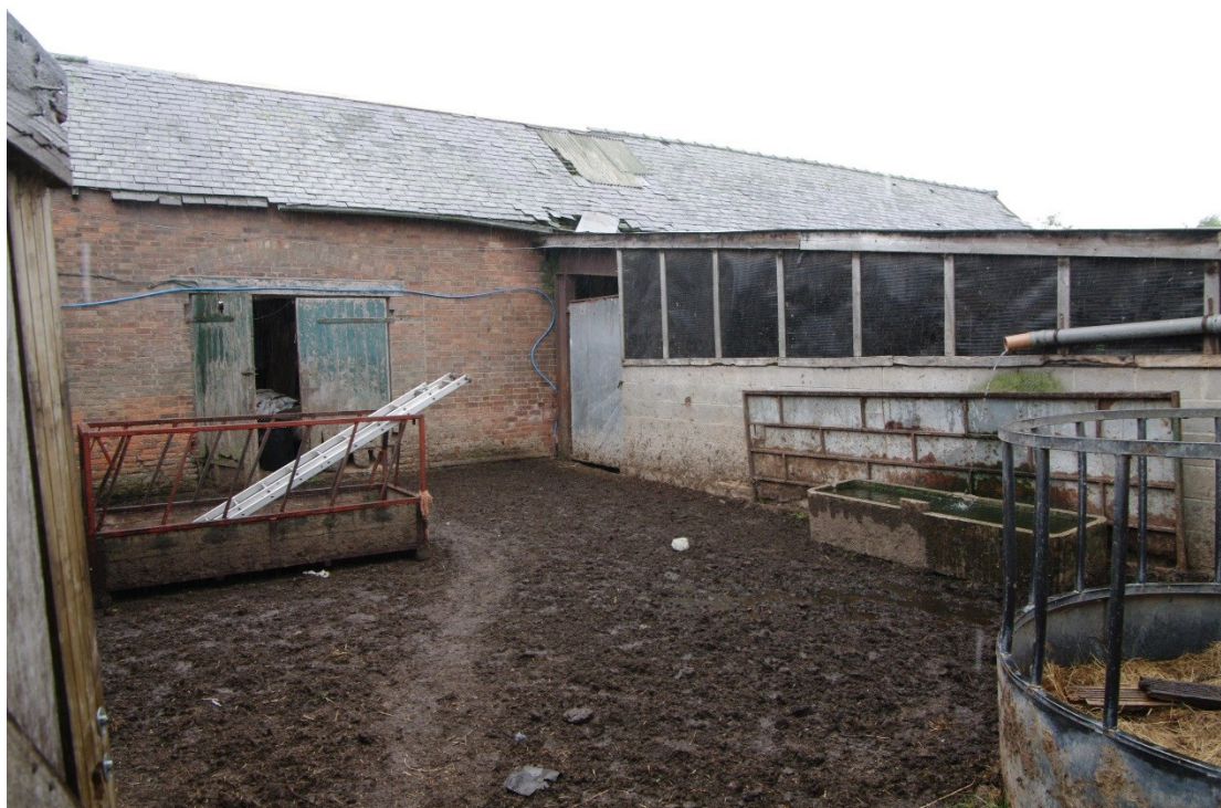
Figure 33: Barn B, north facing elevation (centre portion) Looking south-east
