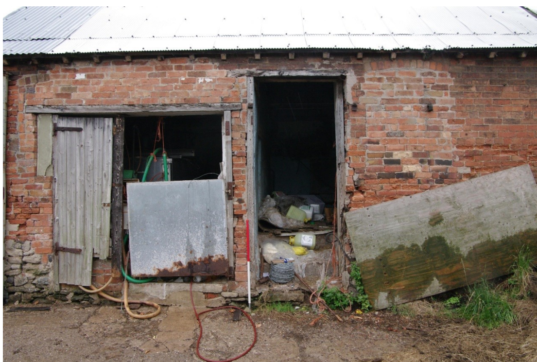
Figure 12: Barn A, western doors on south facing elevation Looking north. 1m scale. Note modified doors and blocked windows
