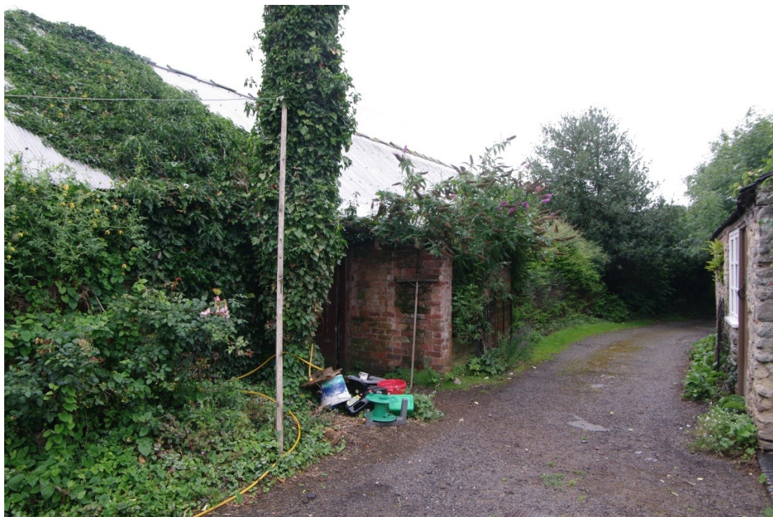
Figure 19: Barn A north facing elevation Looking south-west
