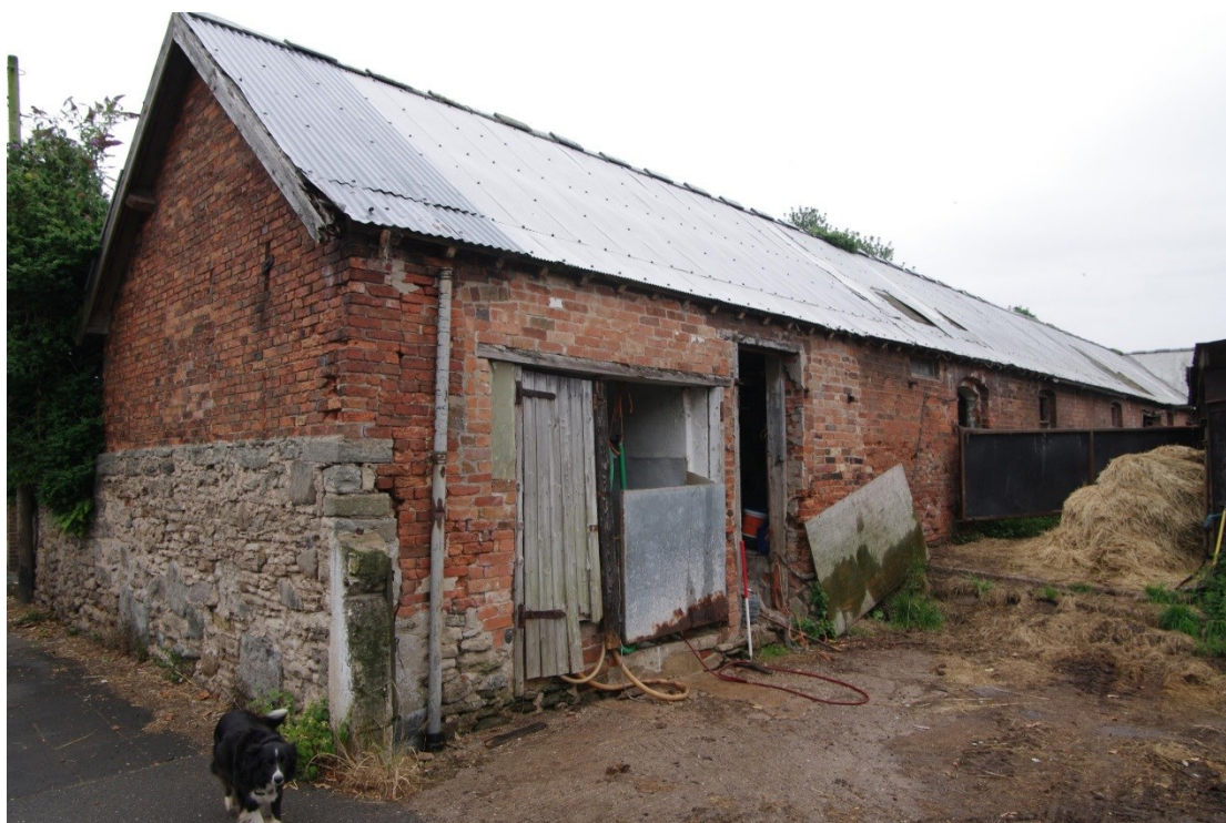
Figure 11: Barn A west and south facing elevations Looking north-east. 1m scale
