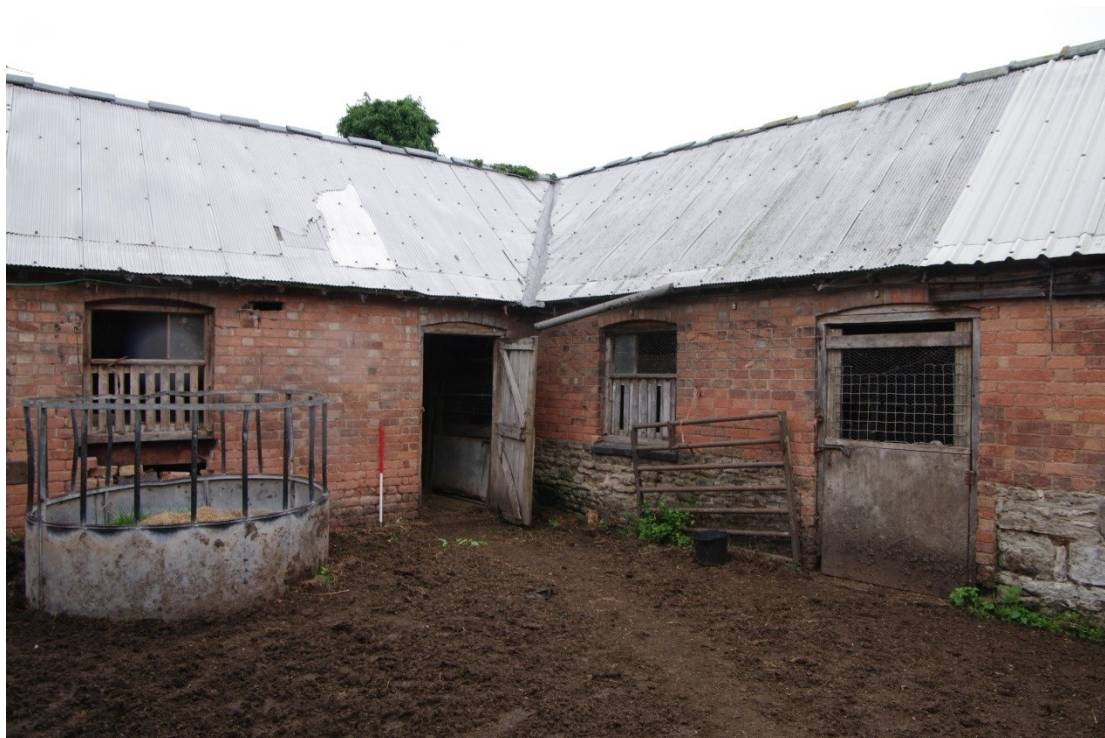
Figure 15: Barn A east end Looking north-east
