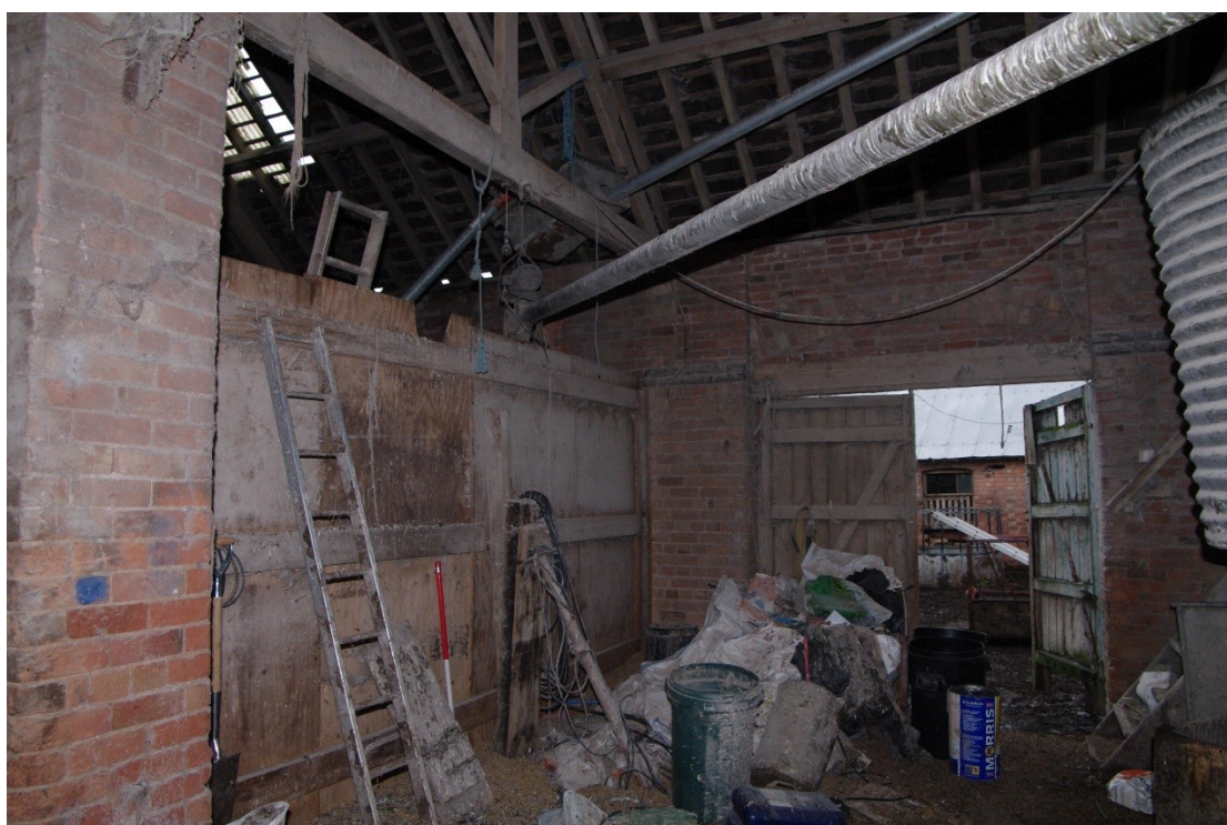
Figure 38: Barn B, northern double doorway Looking north. 1m scale
