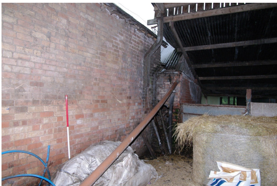
Figure 30: Barn B, south facing elevation (east end) Looking north-east. 1m scale
