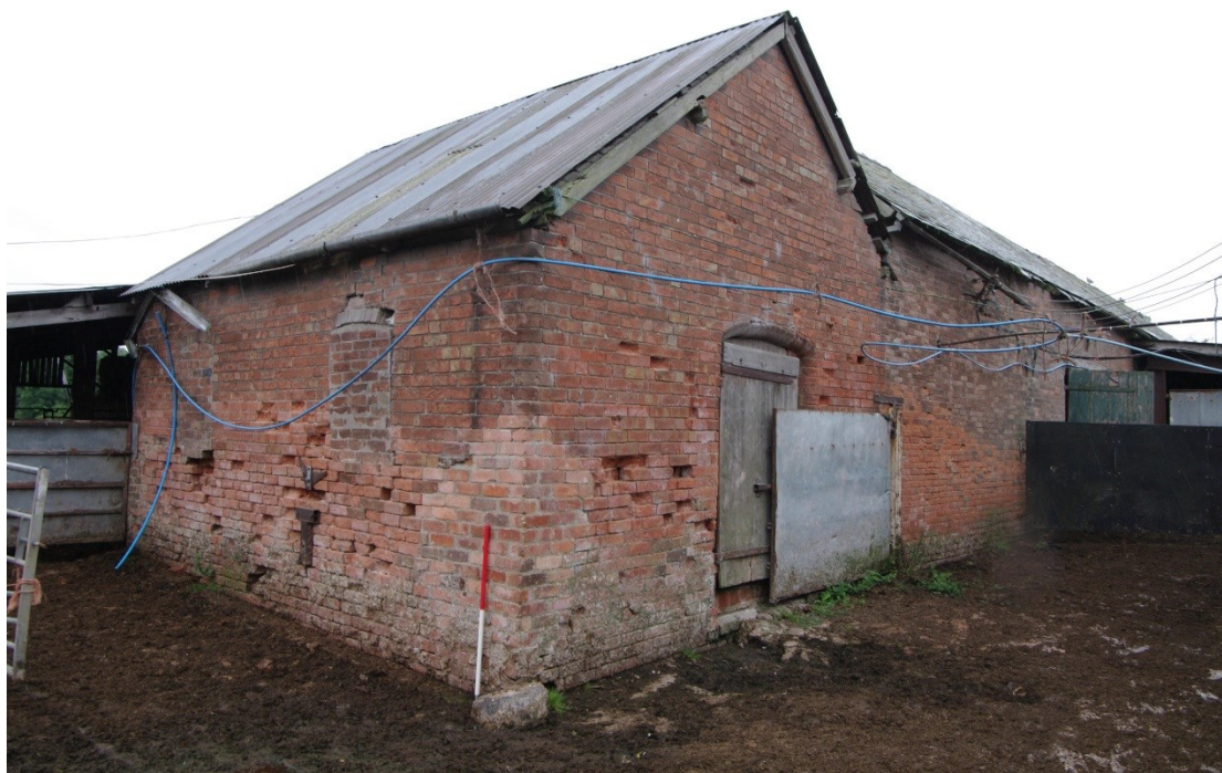
Figure 31: Barn B, east and north facing elevations Looking south-west. 1m scale
