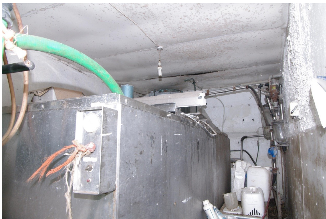
Figure 20: Barn A, westernmost room Looking north from doorway
