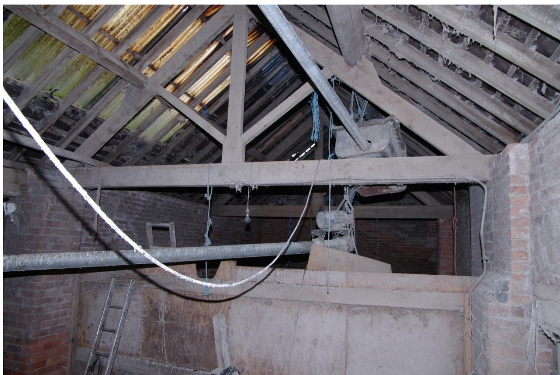
Figure 37: Barn B, centre room Looking west over partition wall
