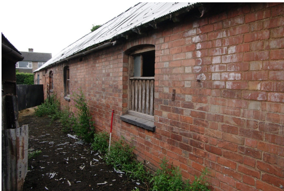
Figure 13: Barn A, south facing elevation Looking north-west. 1m scale
