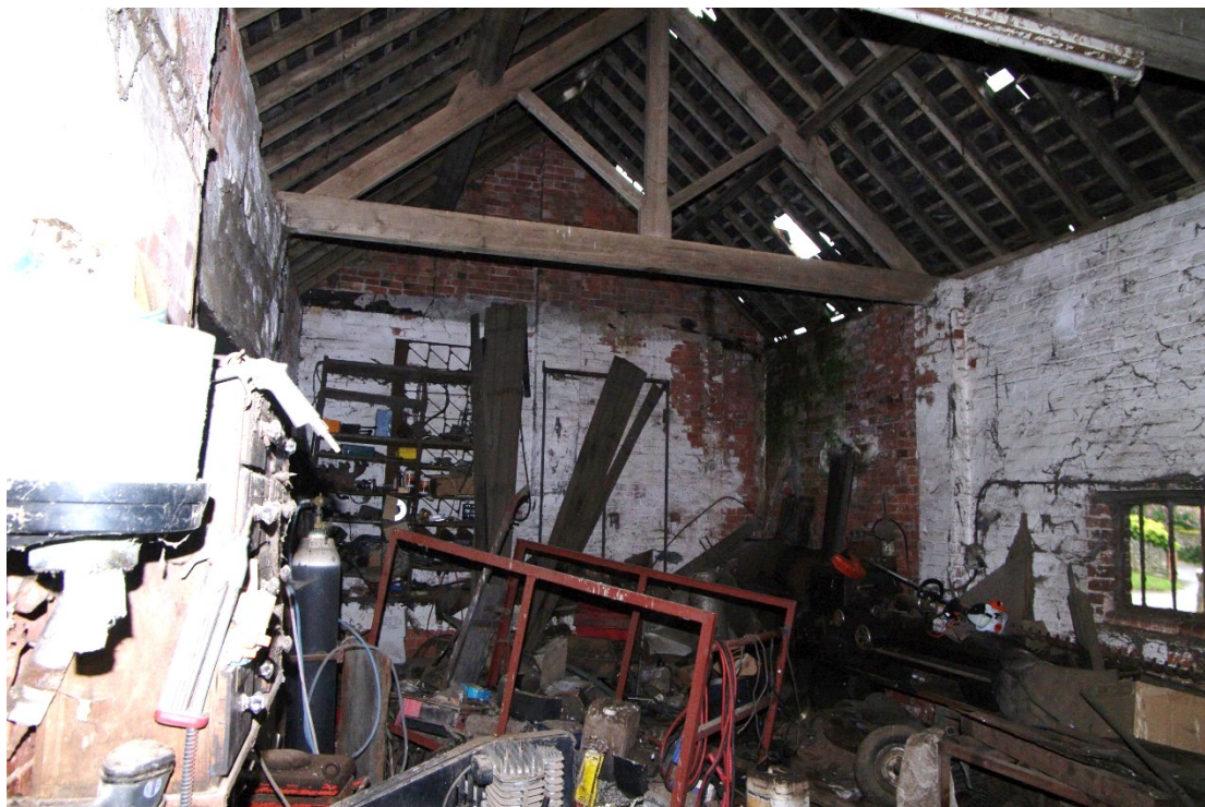
Figure 35: Barn B, western room/workshop Looking north-west
