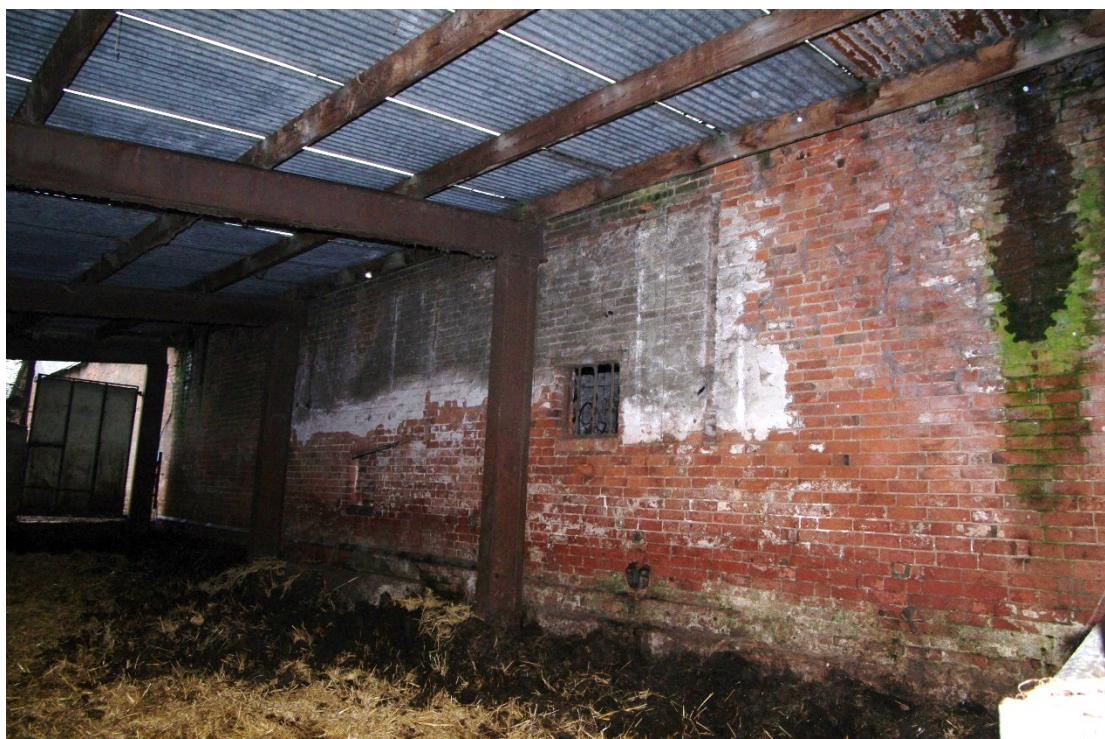
Figure 34: Barn B, north facing elevation (west end) Looking south-east
