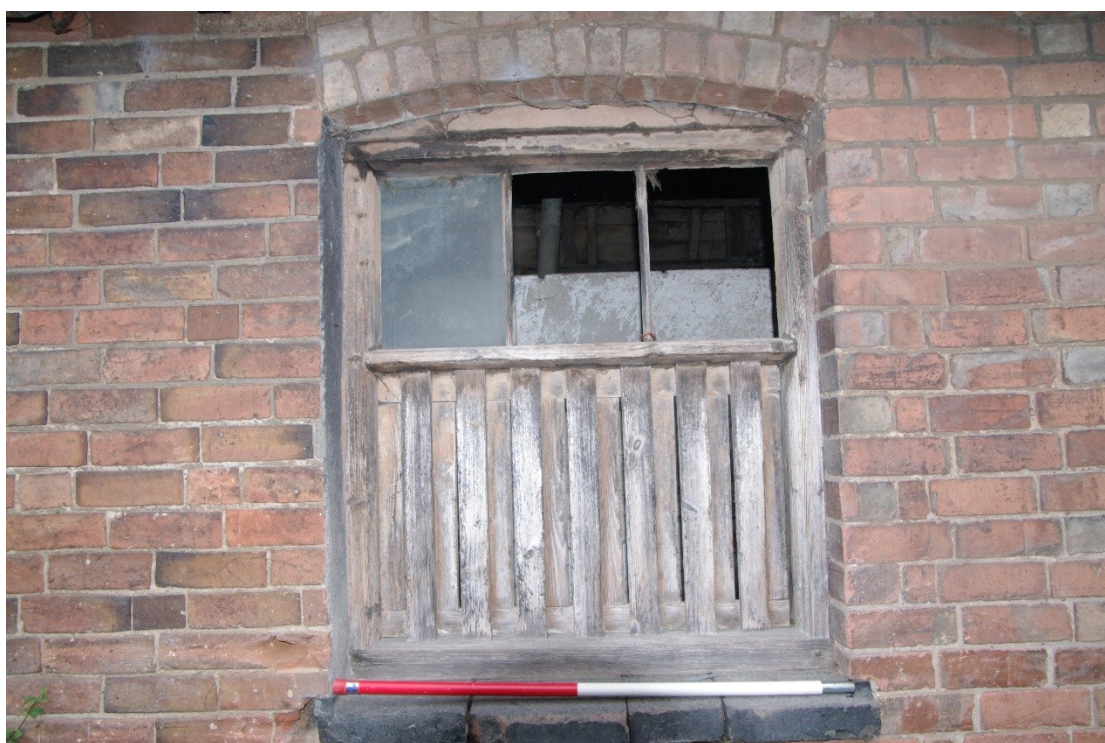
Figure 14: Barn A, south facing elevation window detail Looking north. 1m scale
