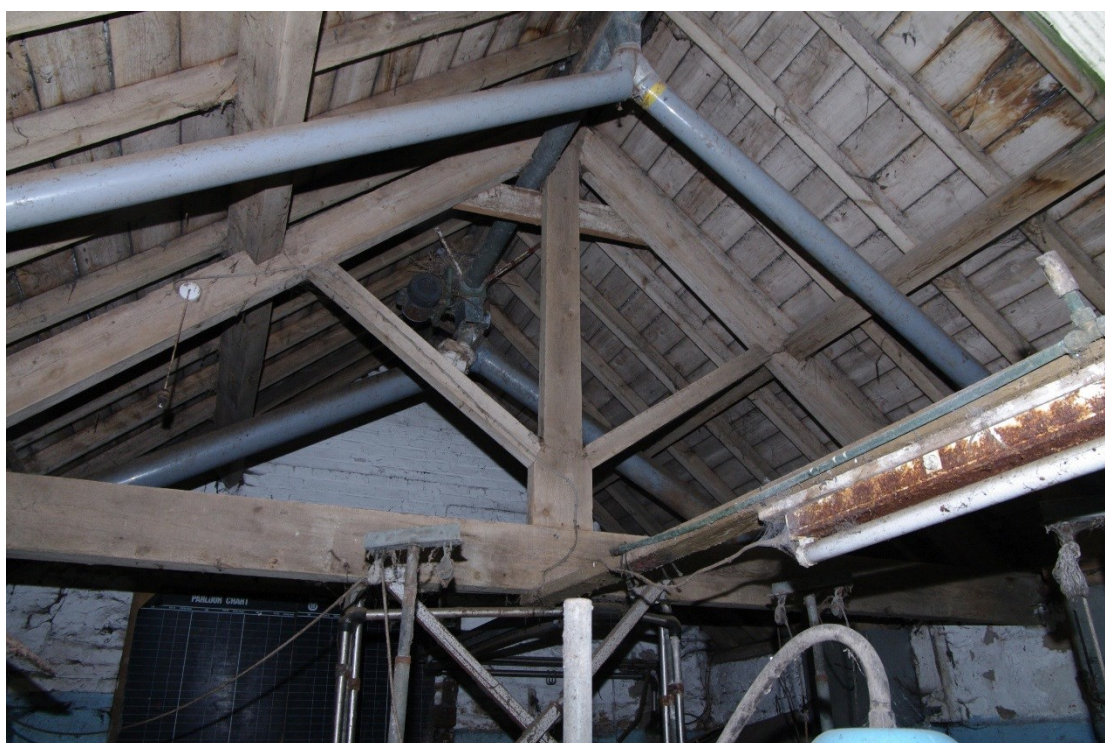
Figure 22: Barn A roof structure in milking parlour Looking west
