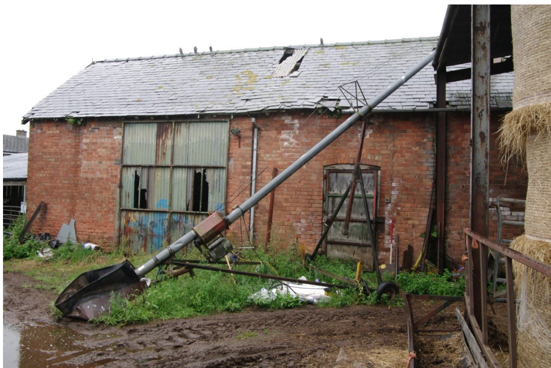
Figure 28: Barn B, south facing elevation (west end) Looking north. 1m scale
