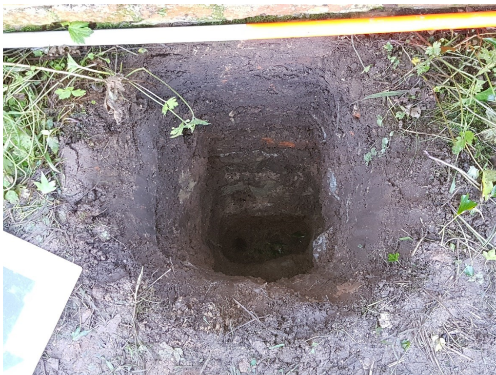
Figure 8: T1, Looking into the investigation pit. The stonework of the original wall is visible close to the base.
