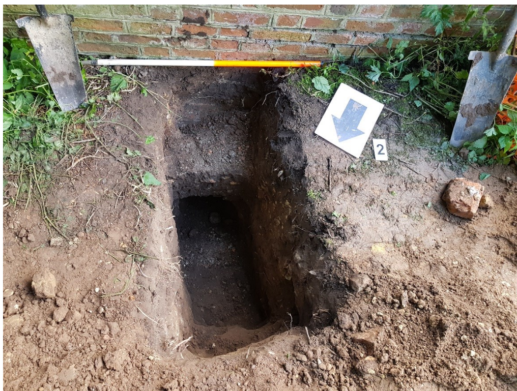
Figure 9: T2, Looking down into the investigative pit. Wall shows signs of repair.
