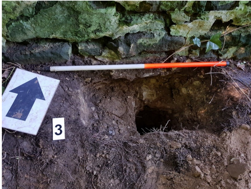
Figure 11: Looking down into T3. Photograph shows the lack of footing to the wall.
