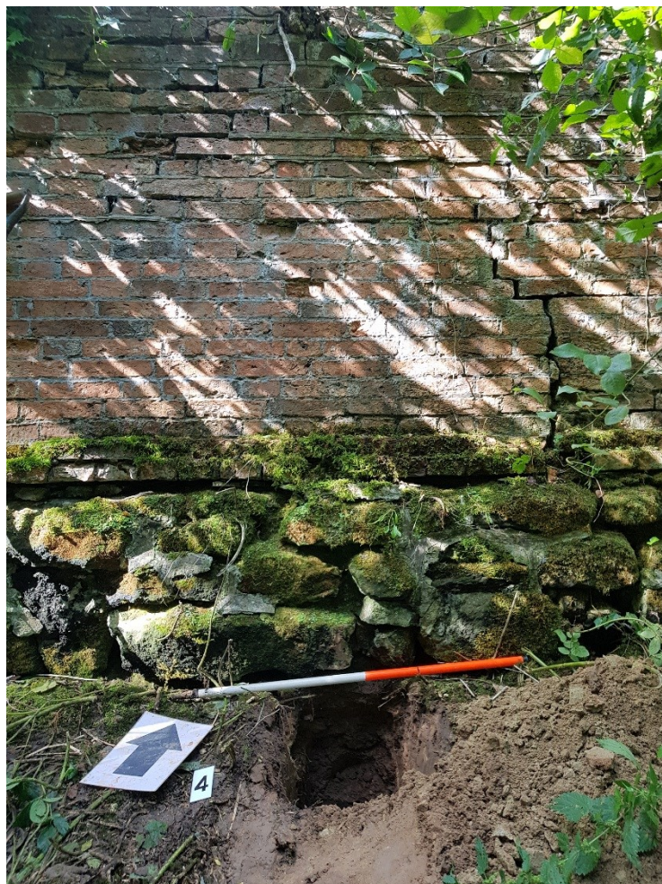
Figure 12: T4 surface of the investigative pit. Photograph showing lack of footing for the wall and also the poor state of the wall.
