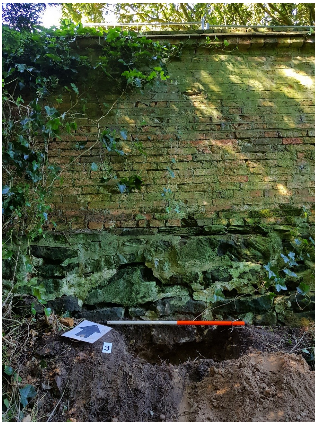
Figure 10: T3, Looking at the investigative pit surface. Photograph shows the lack of footing to the wall.
