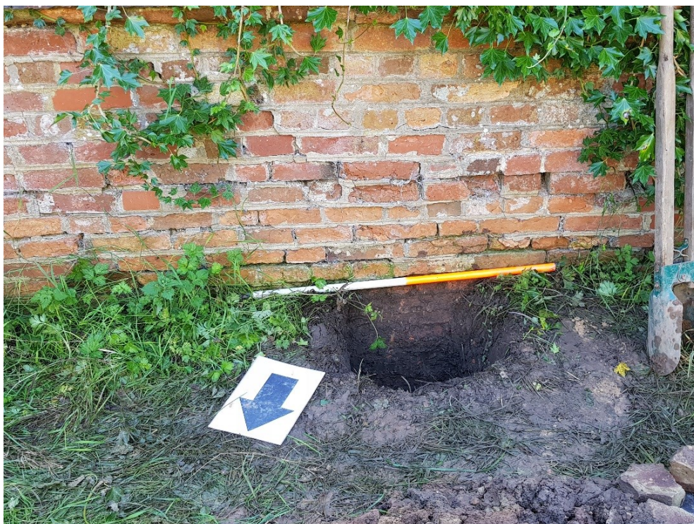
Figure 7: T1 – Investigative pit after excavation. Shows the brickwork of the wall running down to the base of the pit where the stonework of the old wall is visible.
