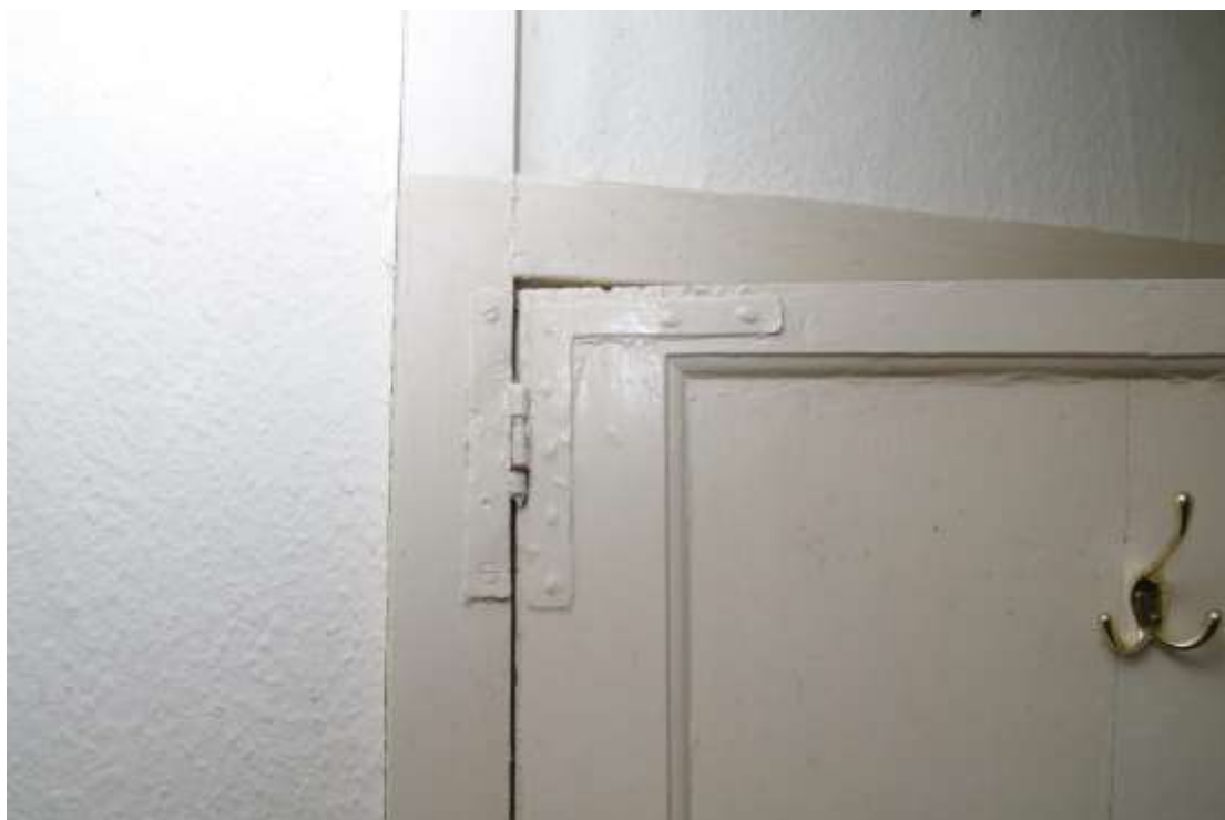
Figure 44 First floor, east room door L-hinge detail Looking west
