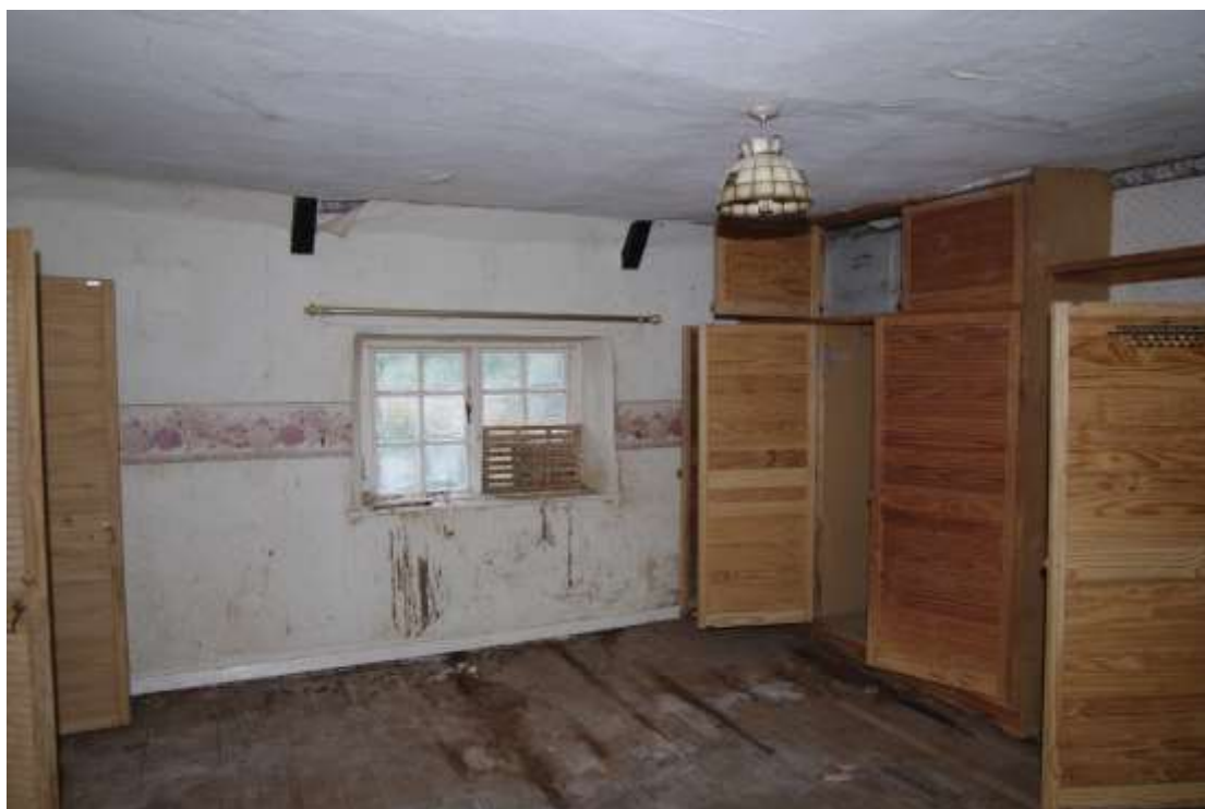
Figure 36 First floor, west room Looking south-west
