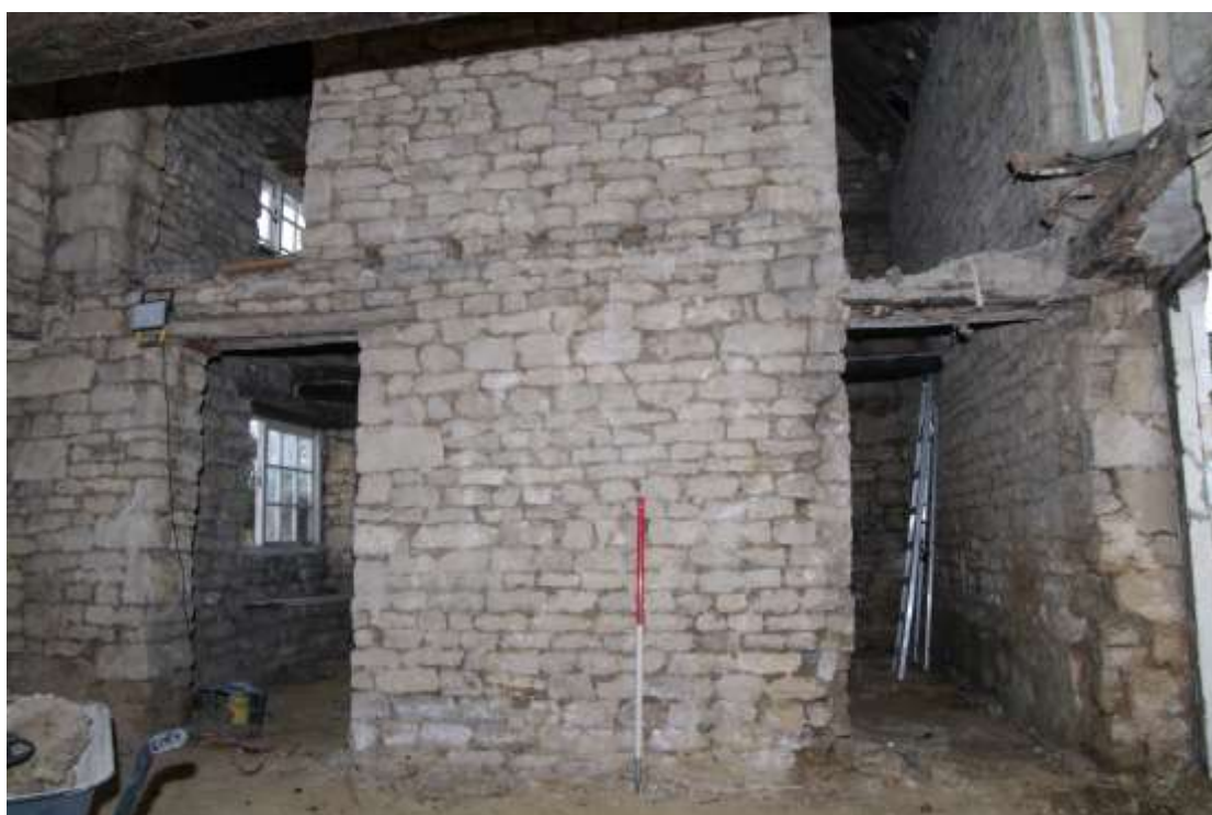
Figure 48 Doorways into western rooms Looking west. 1m scale. Former blocked door from G1 beneath stairs is bottom right. Door to outside is partially shown on right of picture
