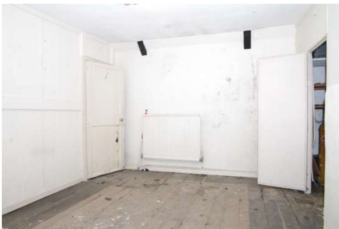
Figure 41 First floor, east room Looking north-west. 1m scale
