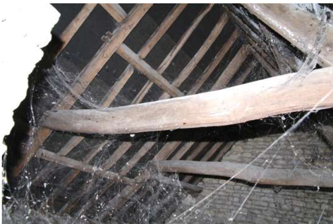
Figure 45 Roof structure Looking south-west
