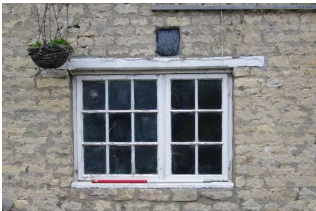
Figure 16 South-facing elevation, ground-floor window detail Looking north. 1m scale
