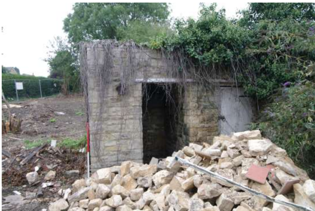
Figure 26 Outdoor privy Looking north. 1m scale
