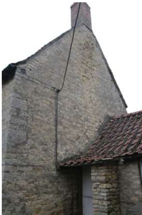
Figure 23 East-facing elevation Looking north-west
