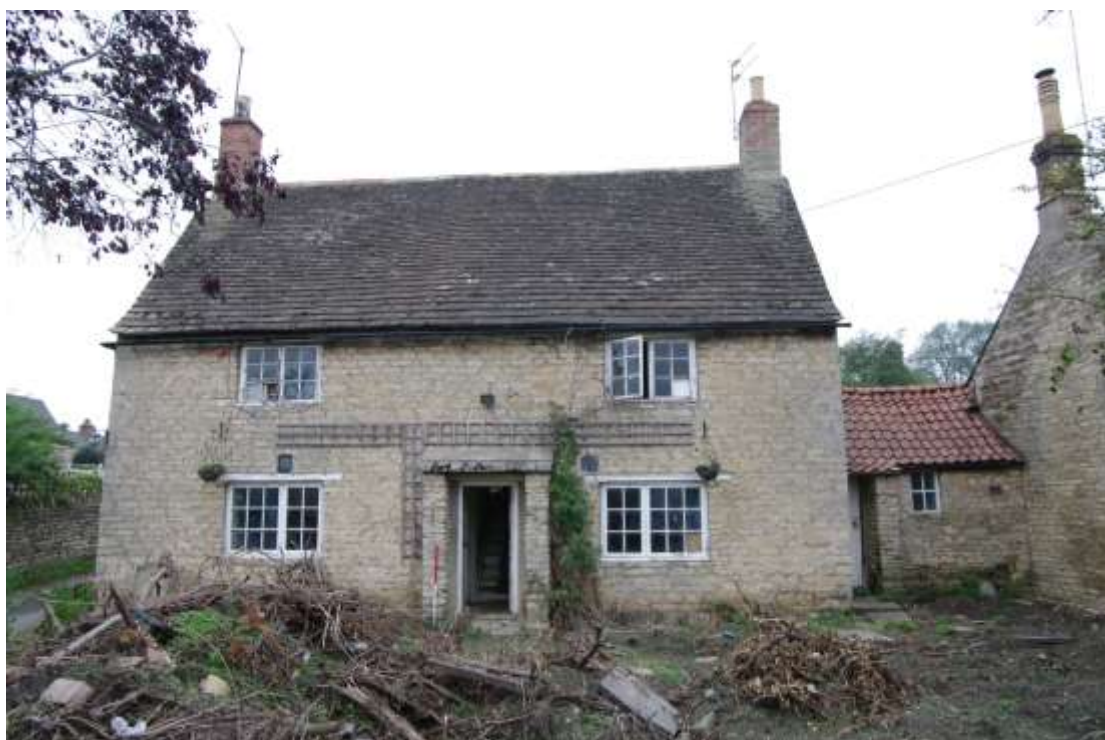
Figure 15 South-facing elevation Looking north. 1m scale
