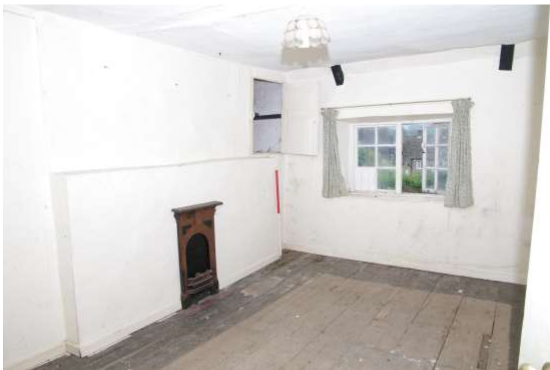
Figure 40 First floor, east room Looking south-east. 1m scale
