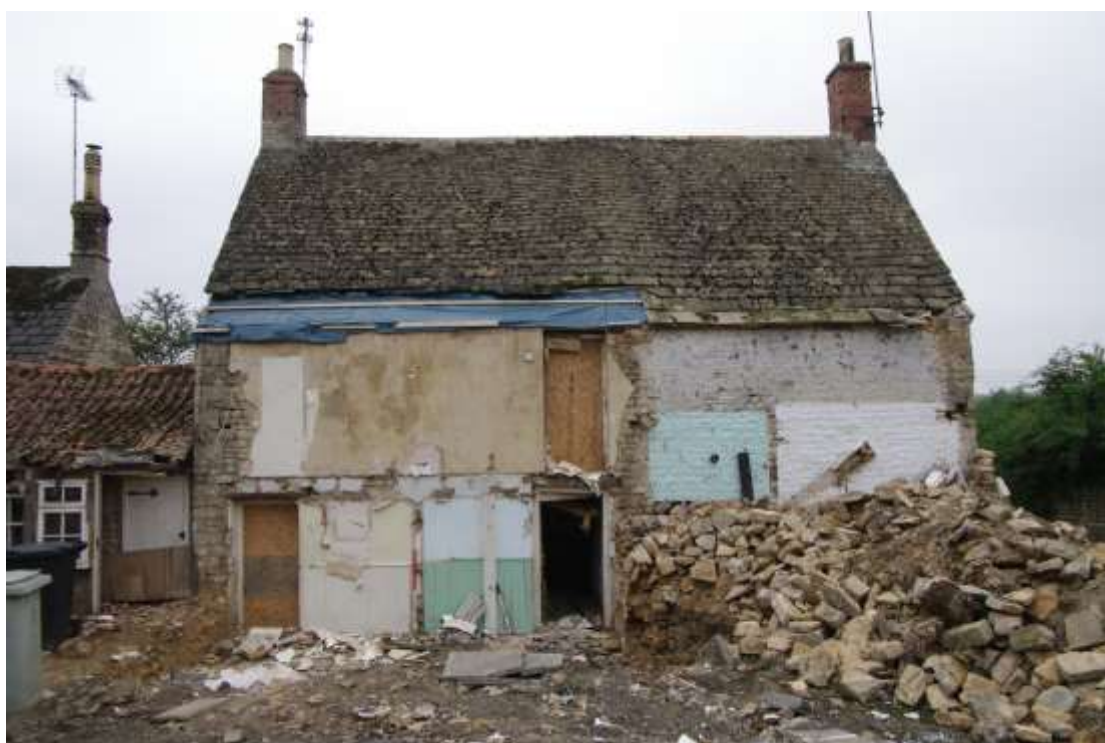
Figure 20 North-facing elevation Looking south. 1m scale
