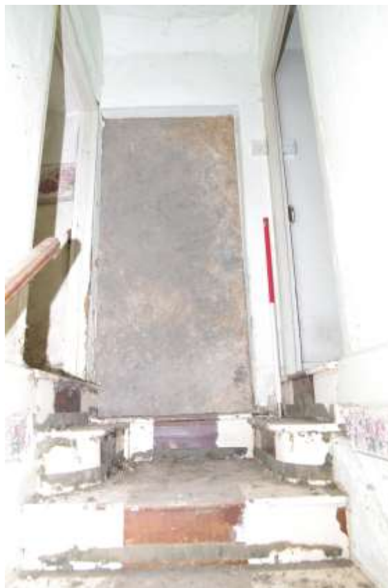
Figure 38 First floor, top of stairs Looking north. 1m scale
