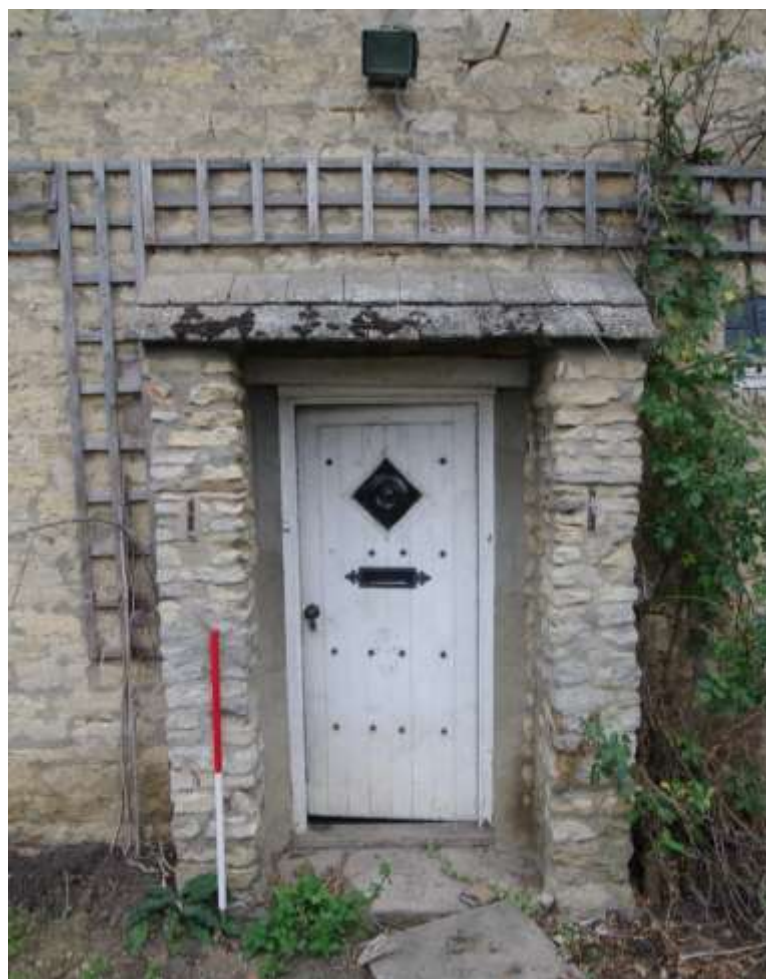
Figure 17 South-facing elevation, front door Looking north. 1m scale
