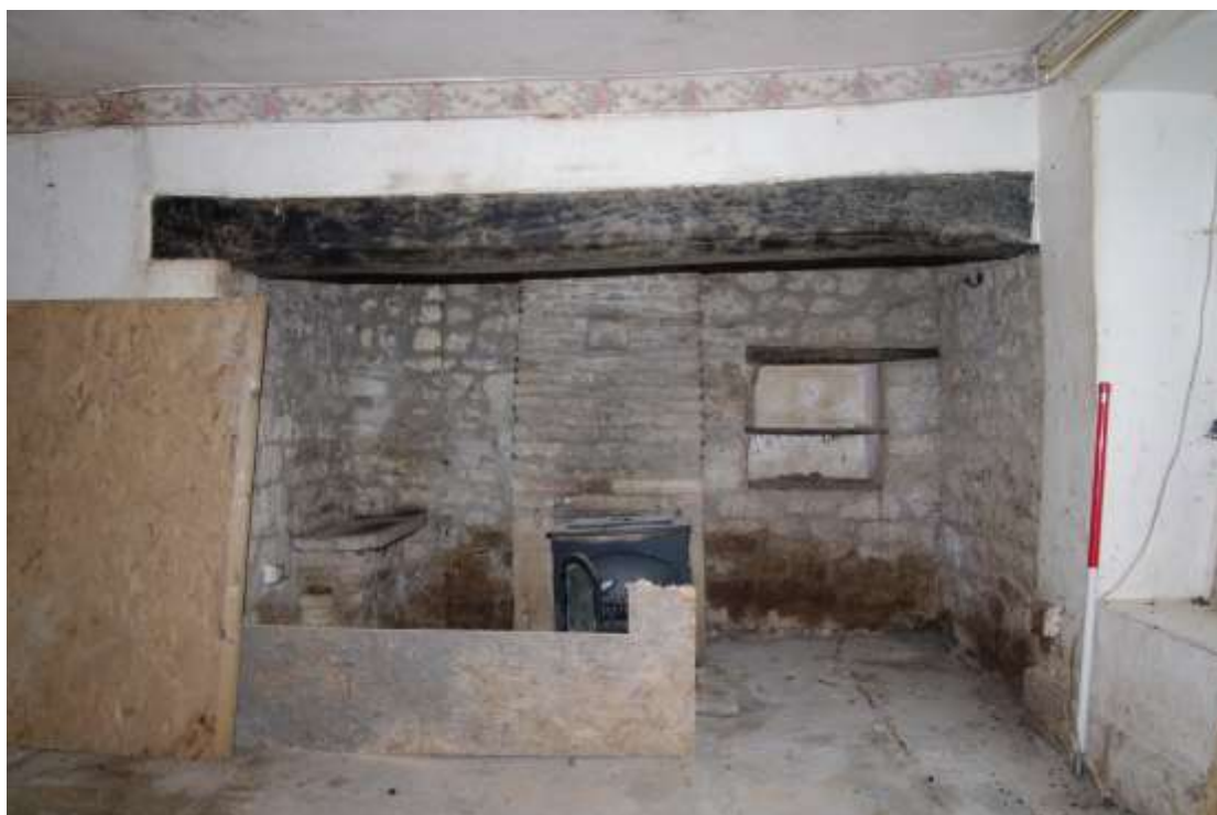
Figure 34 Room G3 fireplace Looking east. 1m scale
