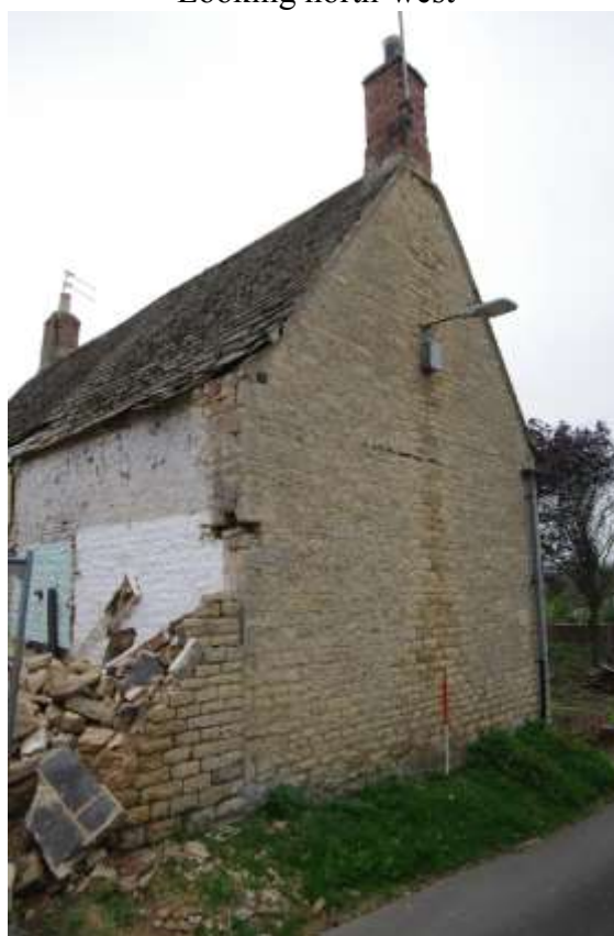
Figure 24 West-facing elevation Looking south-east from Kings Lane. 1m scale
