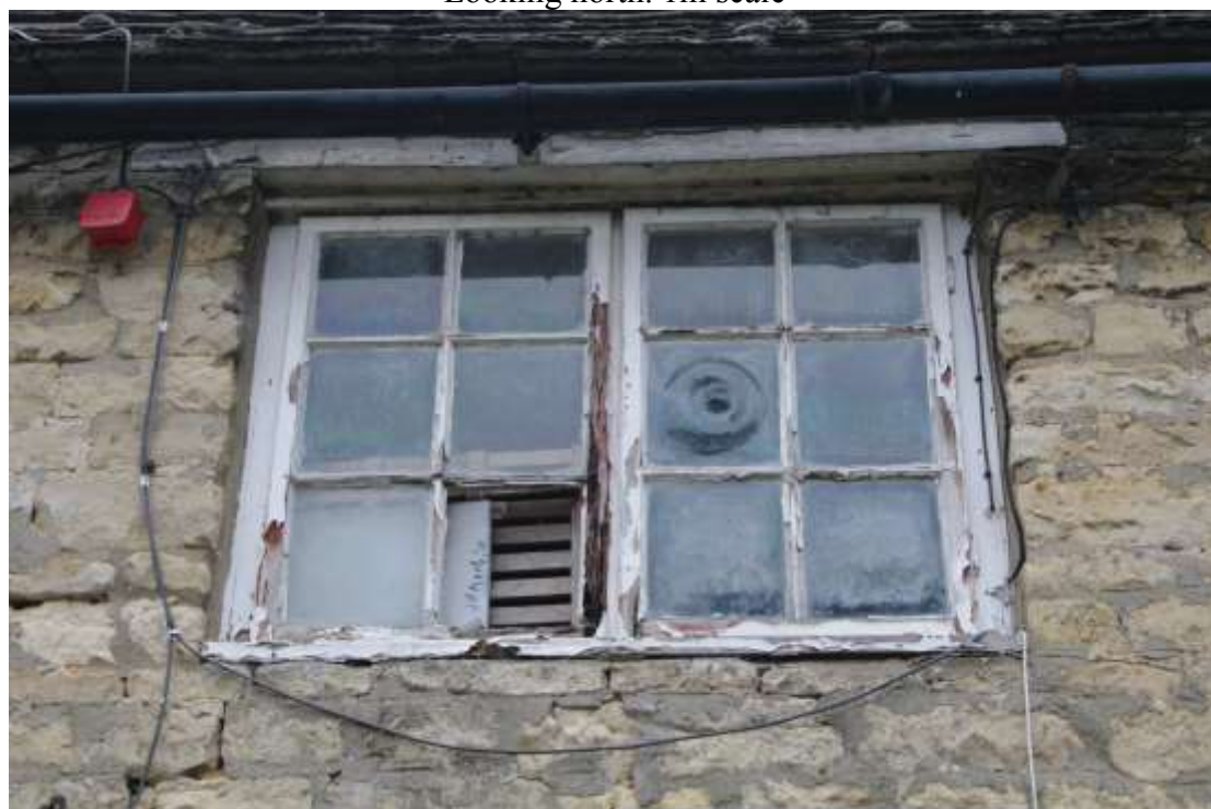
Figure 18 South-facing elevation, first-floor window detail Looking north
