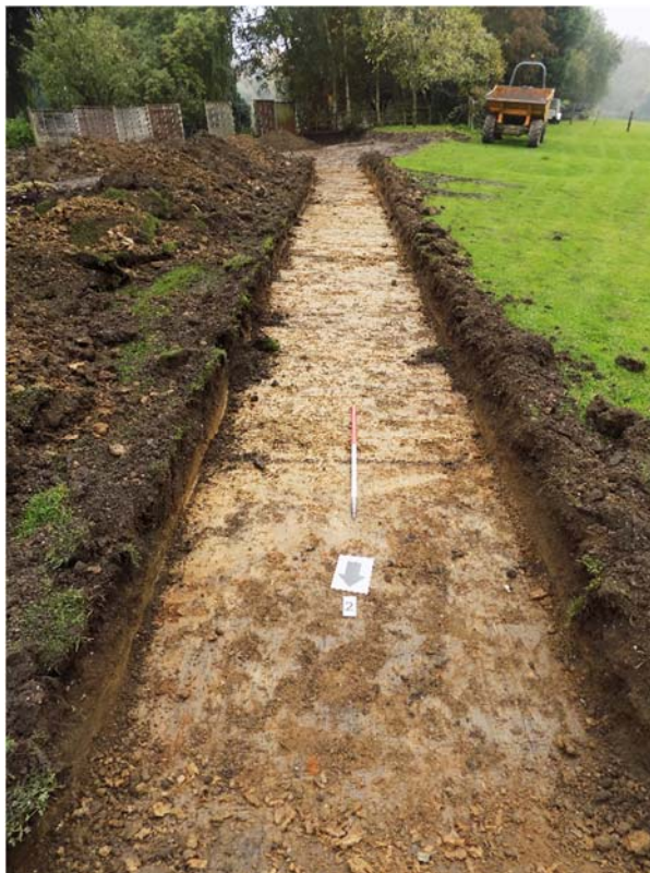
Figure 4: Trench 2: general view south towards Trench 3 & the area previously stripped of topsoil (1m scale)
