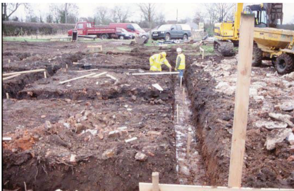
Plate 3. Foundations being excavated on Plot 2.
