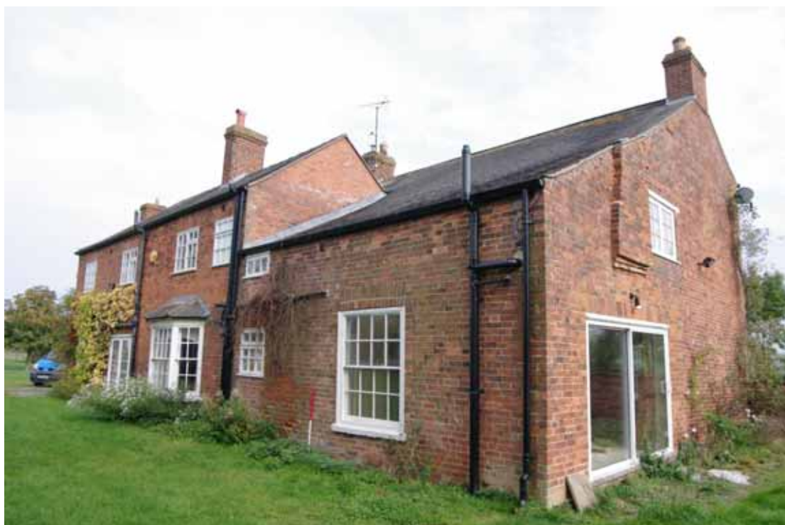
Figure 19 South-west and north-west facing elevations Looking east. 1m scale
