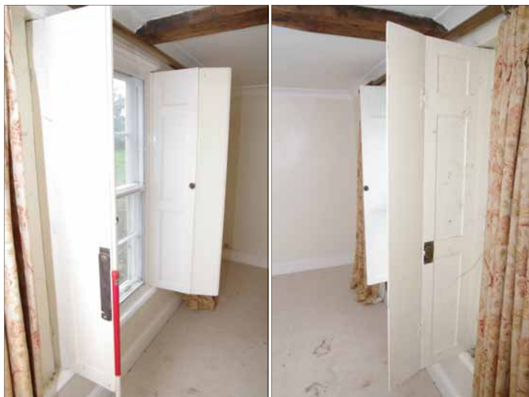
Figure 31 Room G1 window shutter detail Left: looking SW. Right: Looking NE
