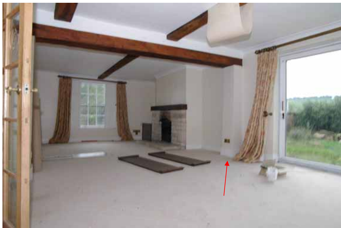
Figure 29 Room G1 Looking south from Room G2. Back wall line of original house is arrowed
