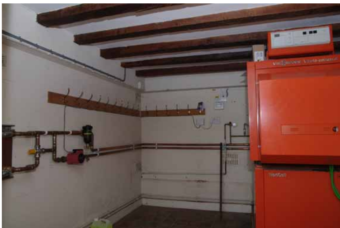
Figure 45 Room G9 boiler room Looking south-east from doorway
