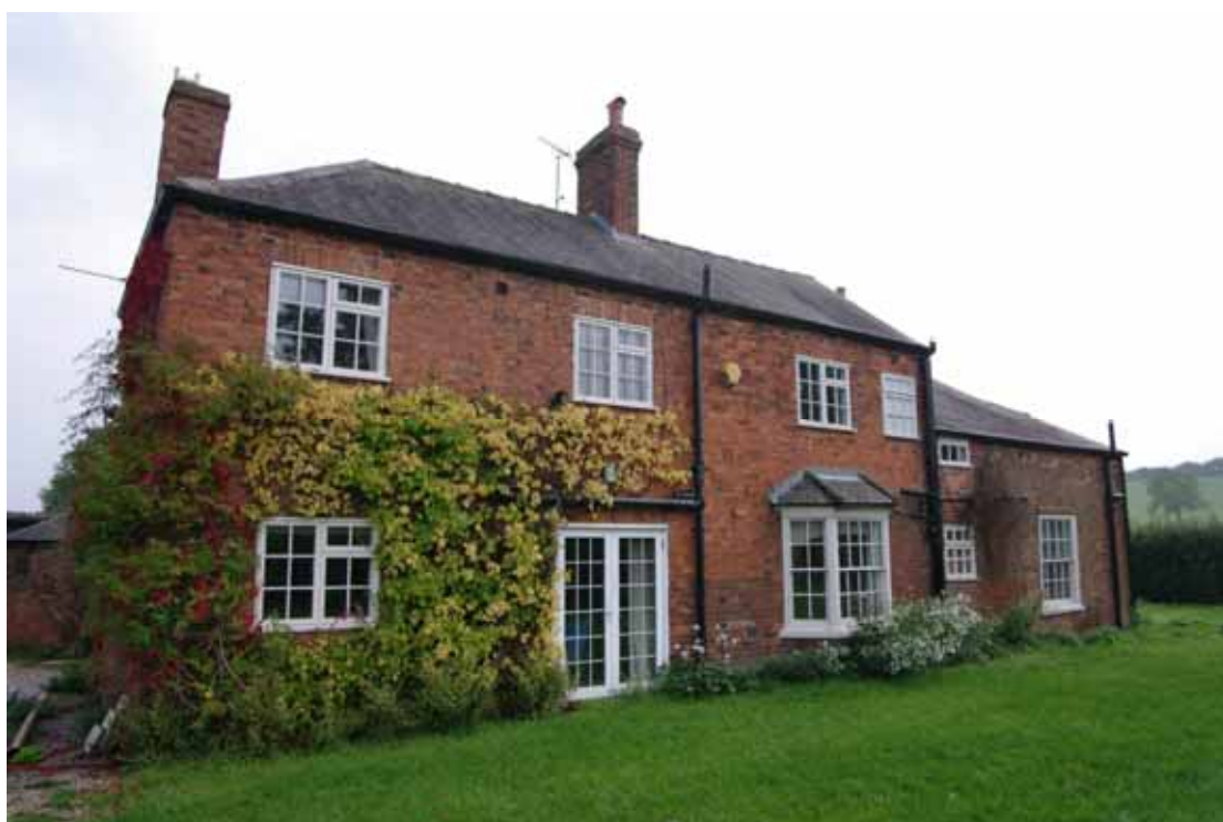
Figure 20 North-west facing elevation Looking south
