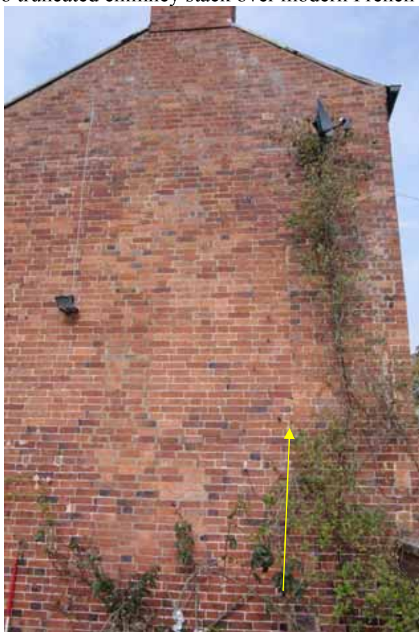
Figure 18 South-west facing elevation Looking north-east. Arrow points to joint/repaired brickwork
