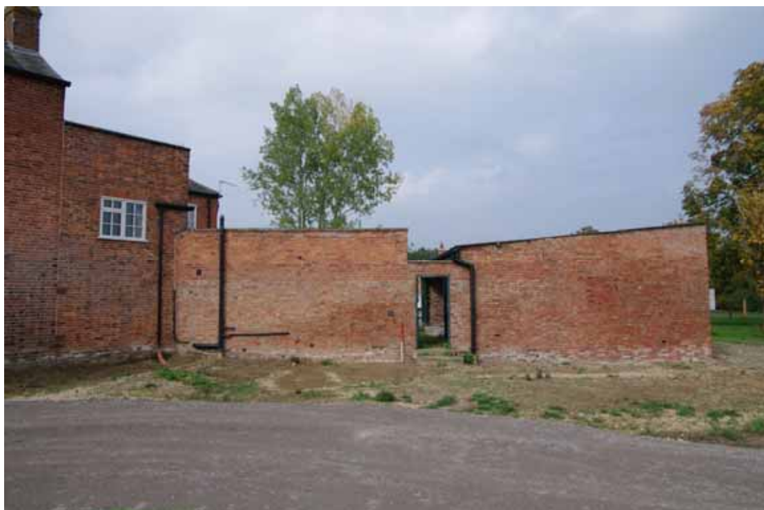
Figure 24 Outbuildings, south facing elevation Looking north. 1m scale. Garage building on right
