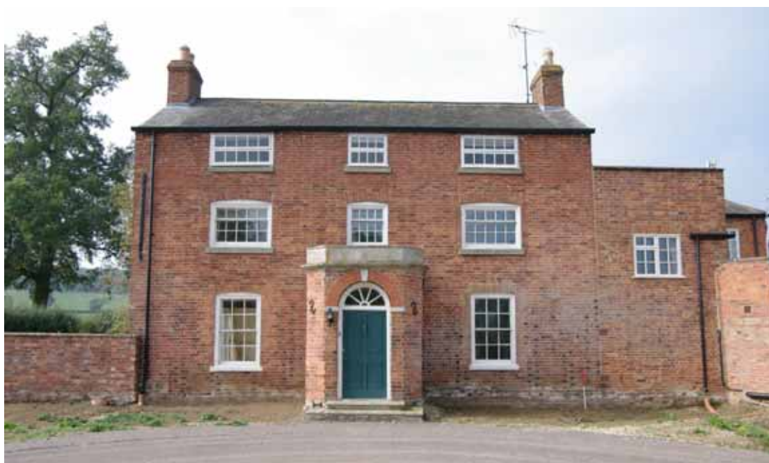
Figure 14 South-east facing elevation Looking north-west. 1m scale. Note butt joint of low two storey extension on right
