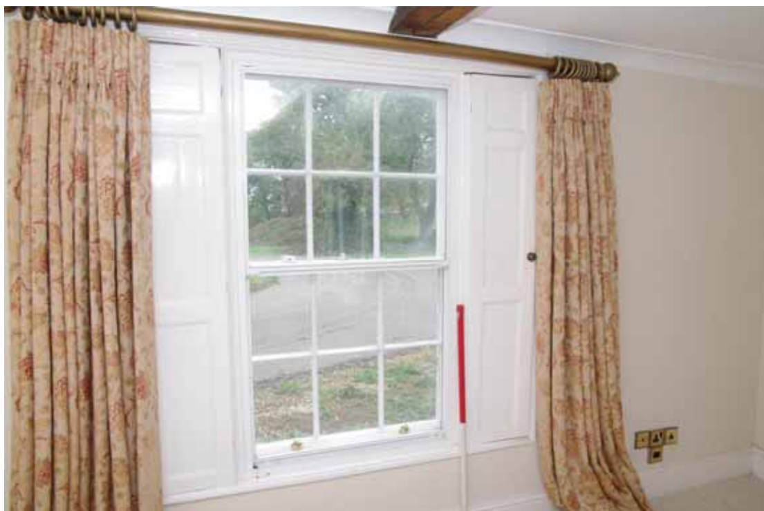
Figure 30 Room G1 window detail Looking south. 1m scale
