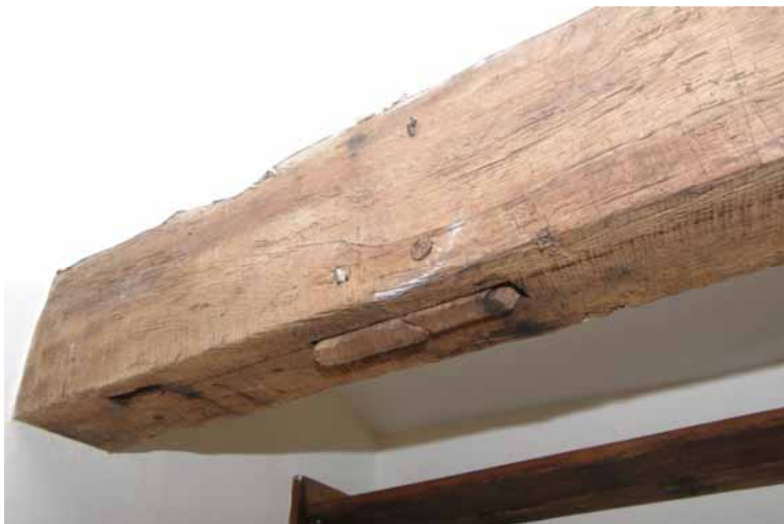
Figure 40 Room G6, underside of bressumer beam
