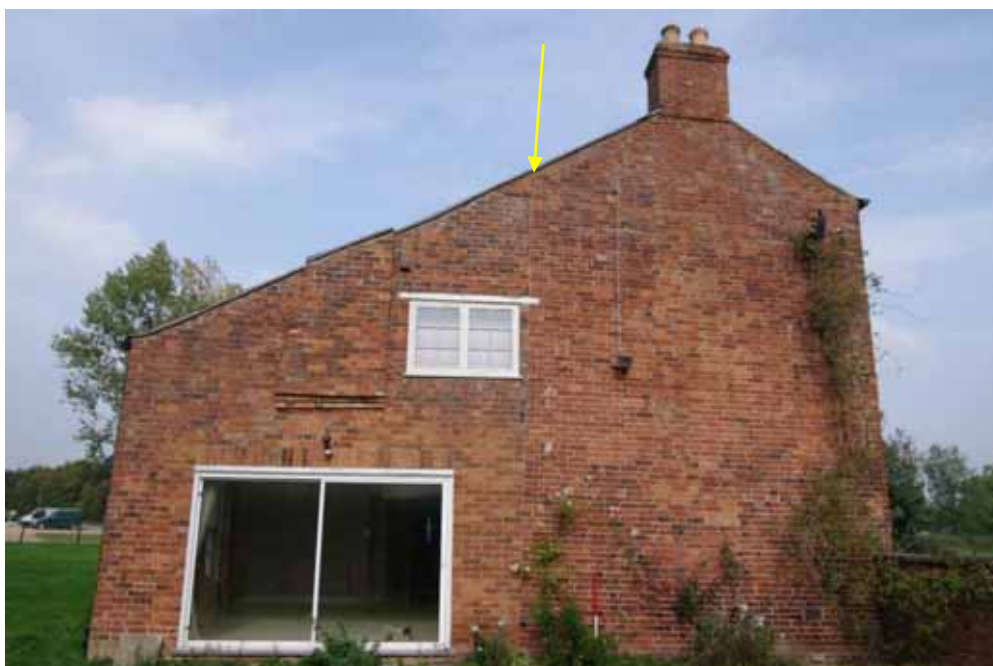
Figure 17 South-west facing elevation Looking north-east. 1m scale. Arrow marks joint of original house and rear extension. Note also truncated chimney stack over modern French windows
