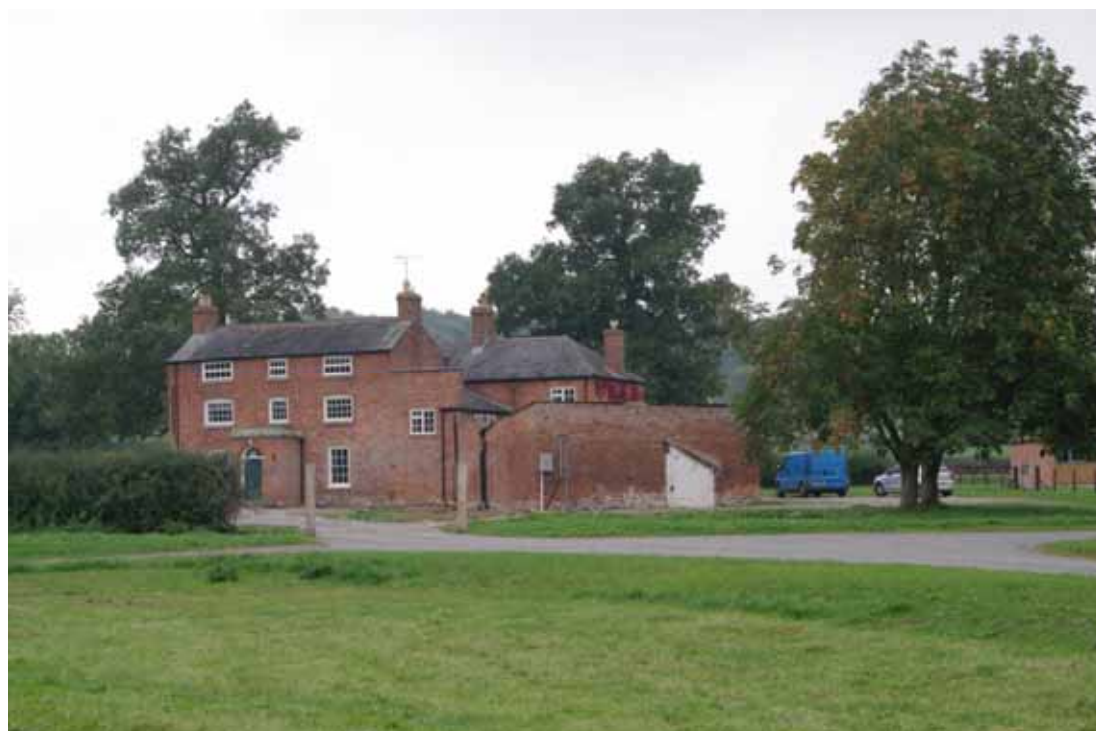
Figure 22 Relationship of house and outbuildings Looking north-west
