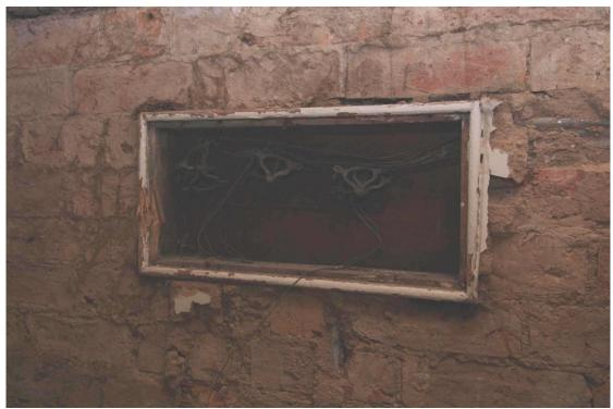
Figure 217 Bell-pull system on second floor
