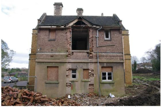
Figure 27 West facing elevation and demolished link to wards
