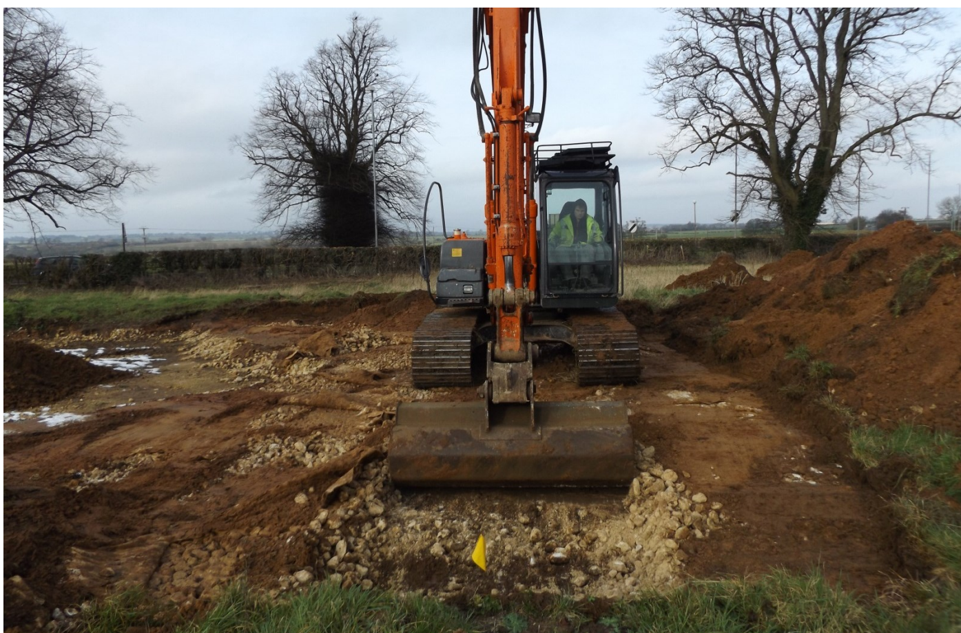
Plate 3: Machining the trenches
