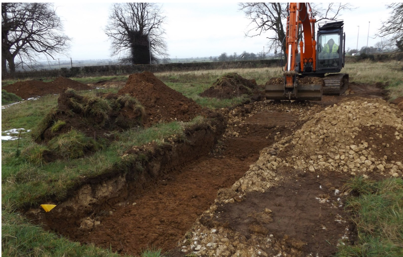
Plate 4: Machining the trenches
