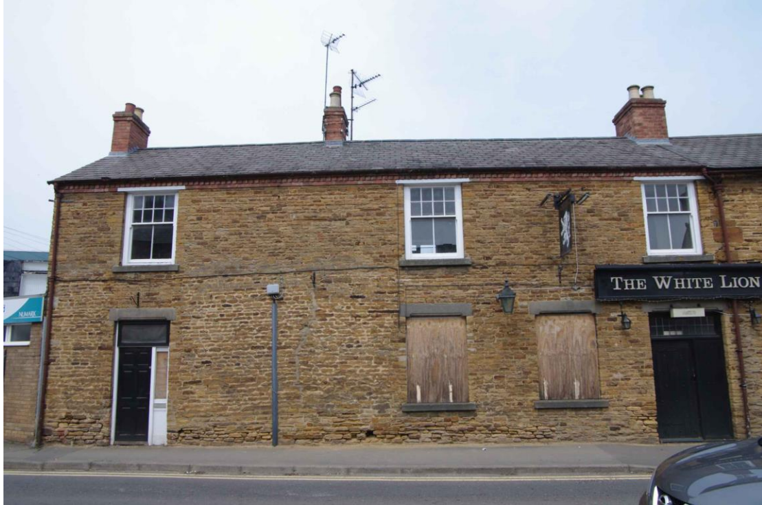
Figure 9 South facing elevation (west end) Looking north
