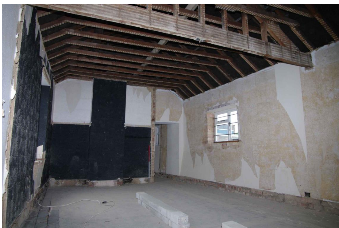
Figure 36 Room F2 Looking north-west. 1m scale
