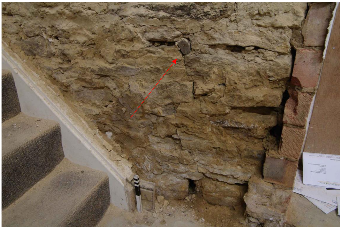
Figure 24 Room G1 sawn off peg on south wall Looking south-east. 0.2m scale. Note also remnant of skirting board
