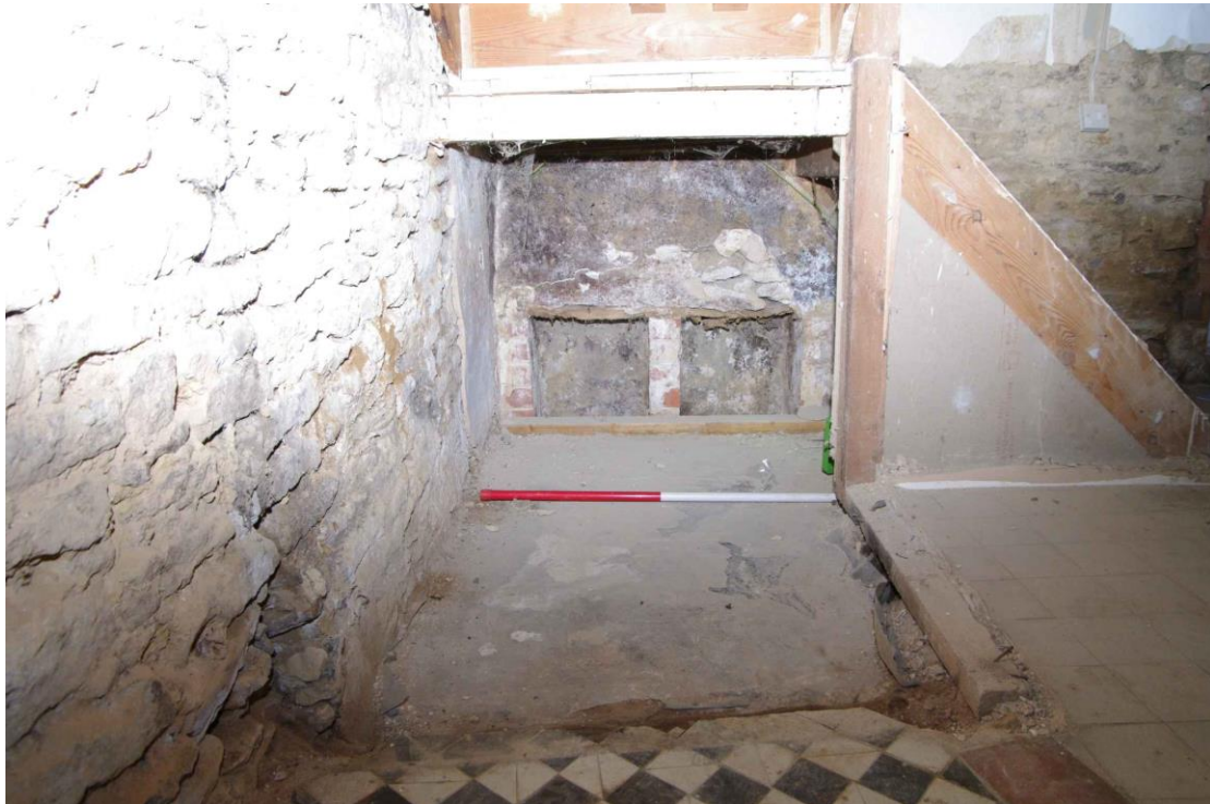
Figure 23 Room G1 former cellar below stairs Looking south. 1m scale
