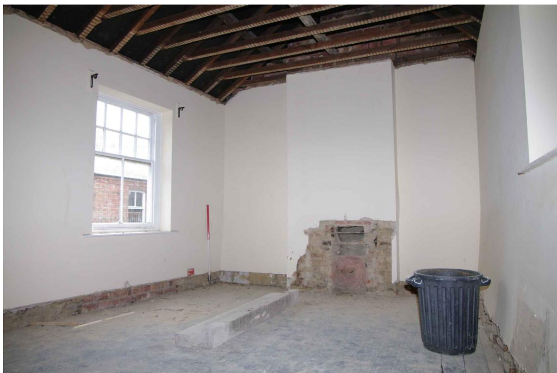
Figure 33 Room F1 Looking south-west. 1m scale
