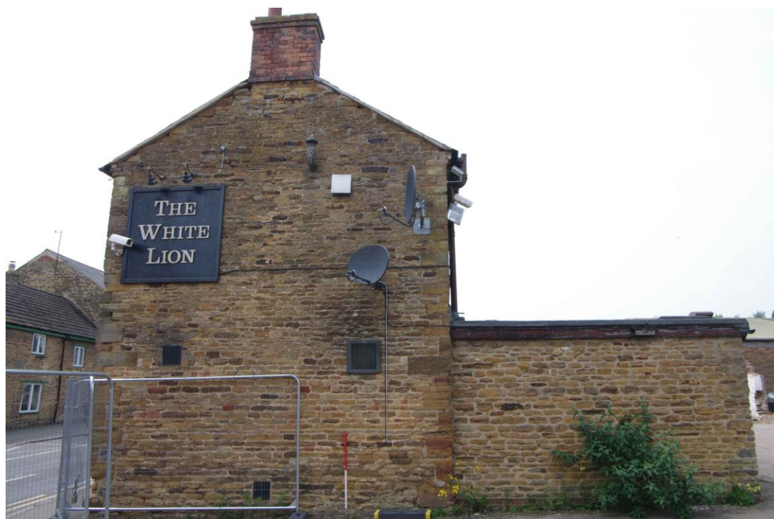
Figure 14 East facing elevation Looking west. 1m scale
