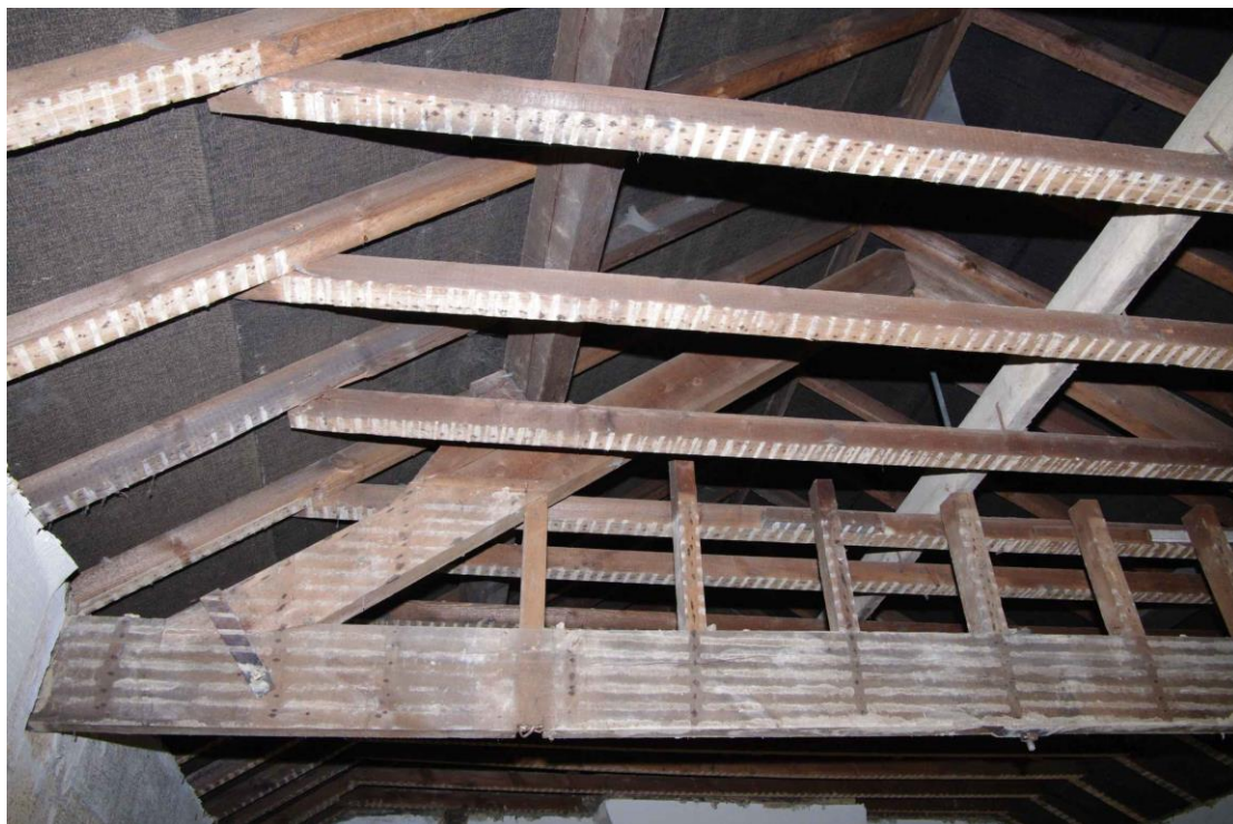
Figure 37 Room F2 roof detail Looking west. Note off-centre ridge and truss
