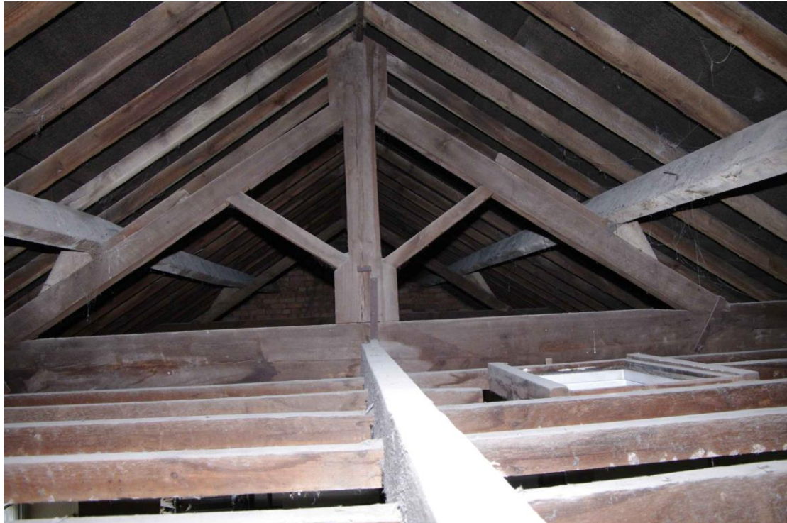
Figure 41 Room F3 roof detail Looking west
