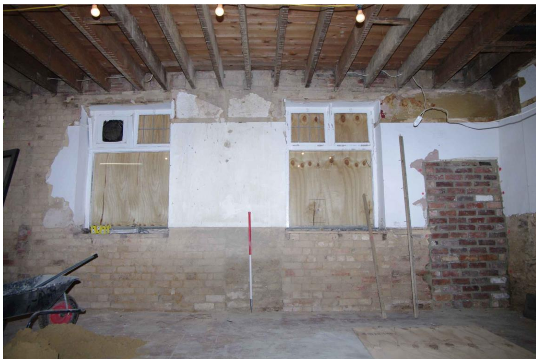
Figure 27 Room G2 south wall Looking south. 1m scale
