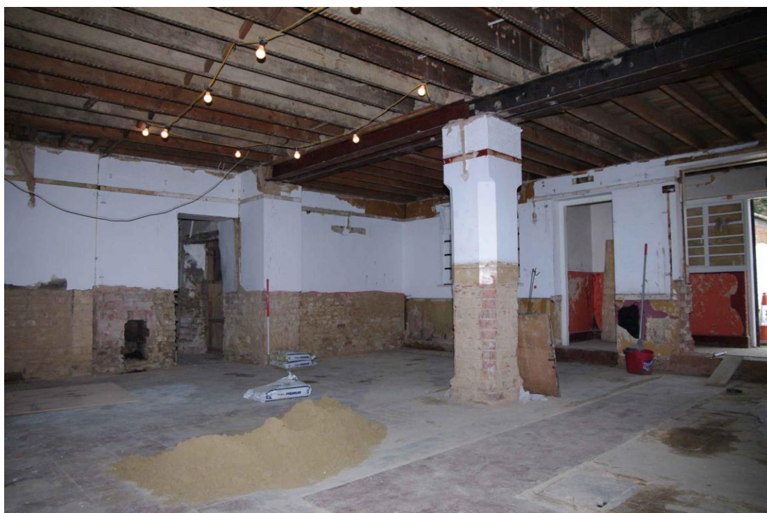
Figure 25 Room G2 Looking north-west. 1m scale
