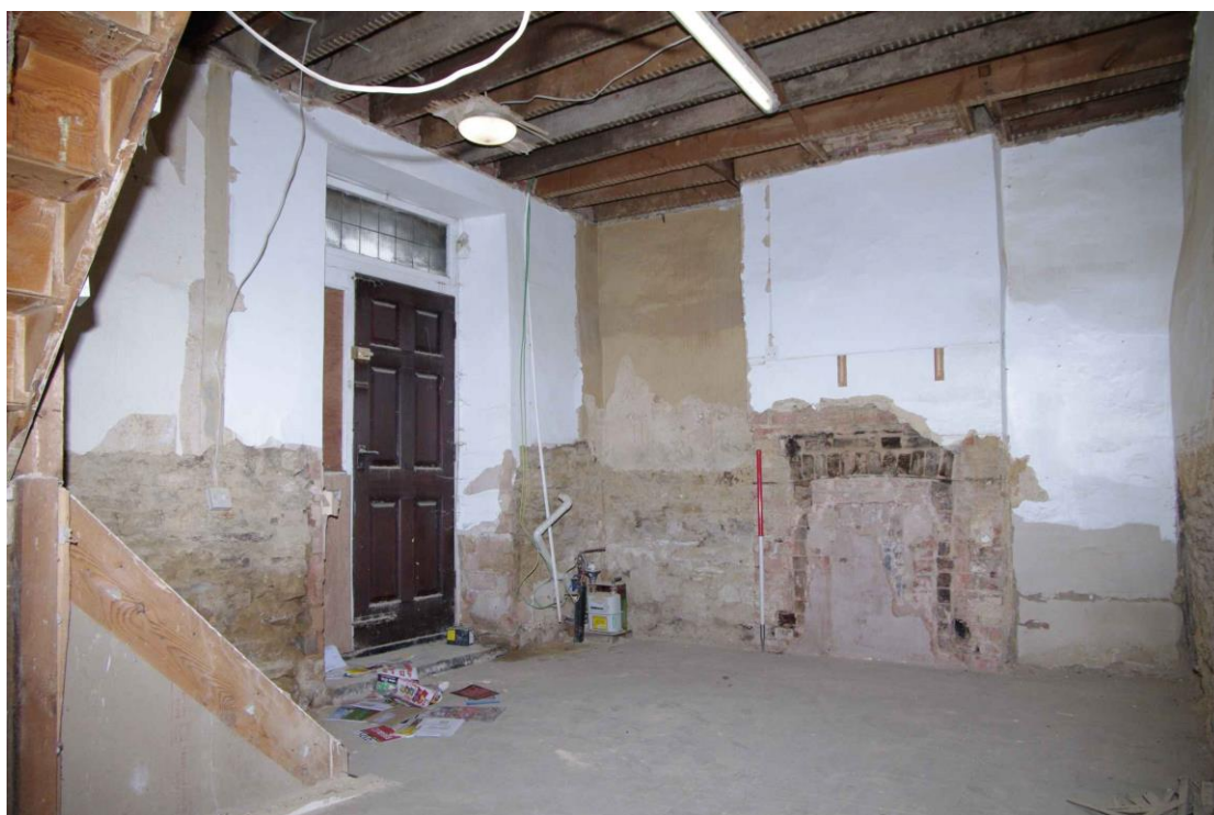
Figure 21 Ground floor room G1 Looking south-west. 1m scale
