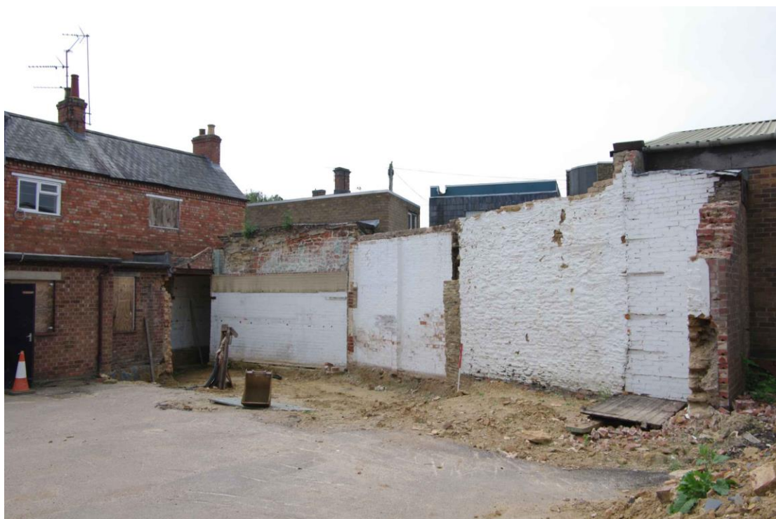
Figure 19 Demolished outbuildings in north-west corner Looking south-west. 1m scale
