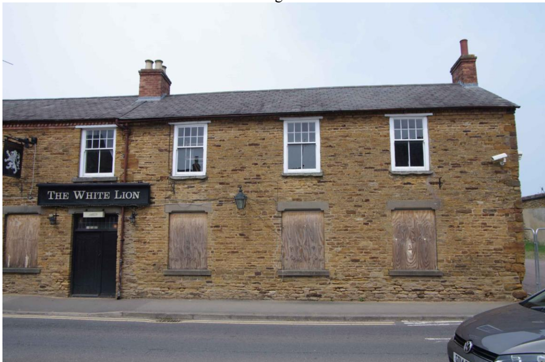
Figure 10 South facing elevation (east end) Looking north
