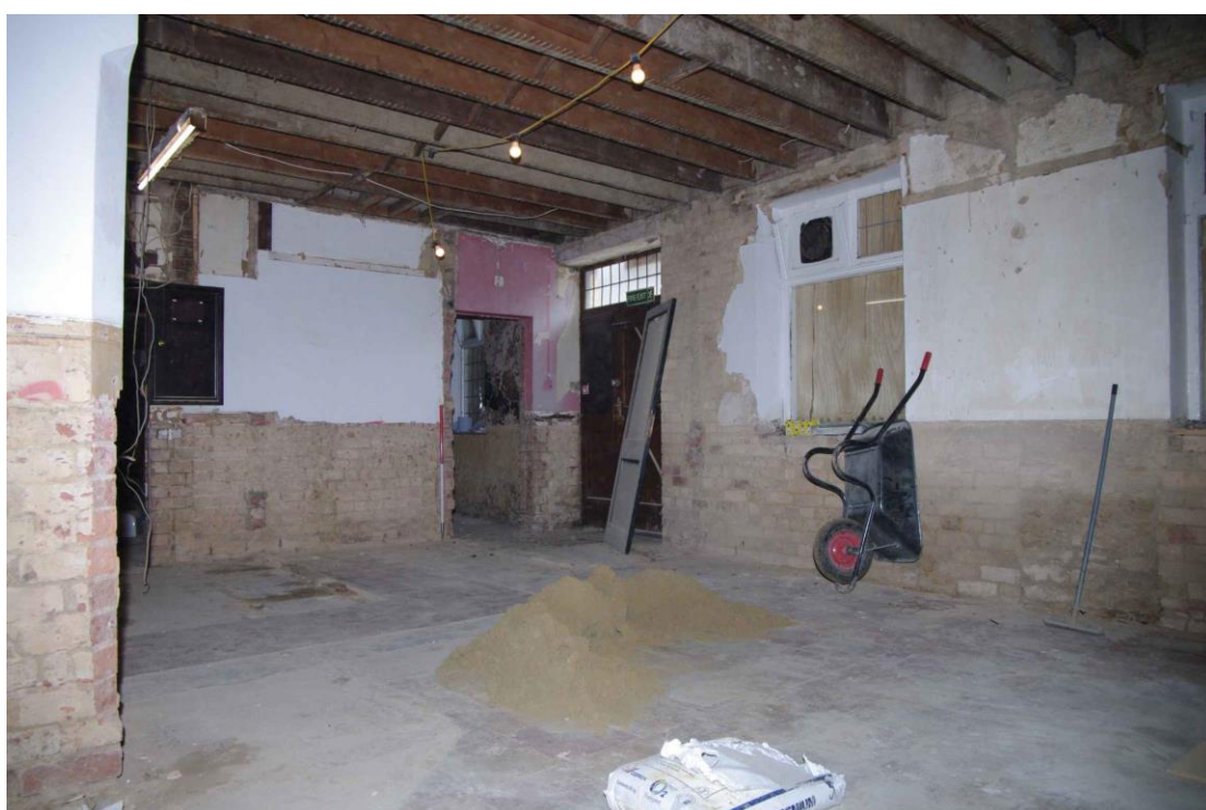
Figure 26 Room G2 Looking south-east. 1m scale
