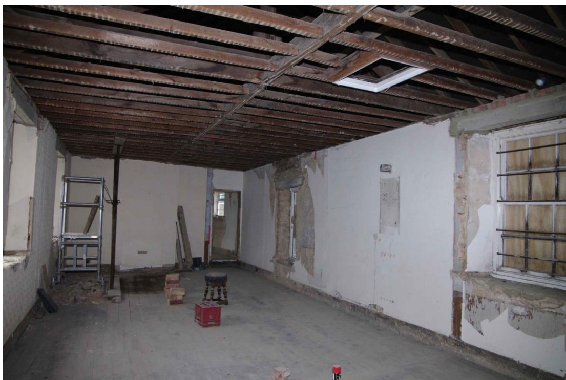
Figure 39 Room F3 Looking north-west. 1m scale
