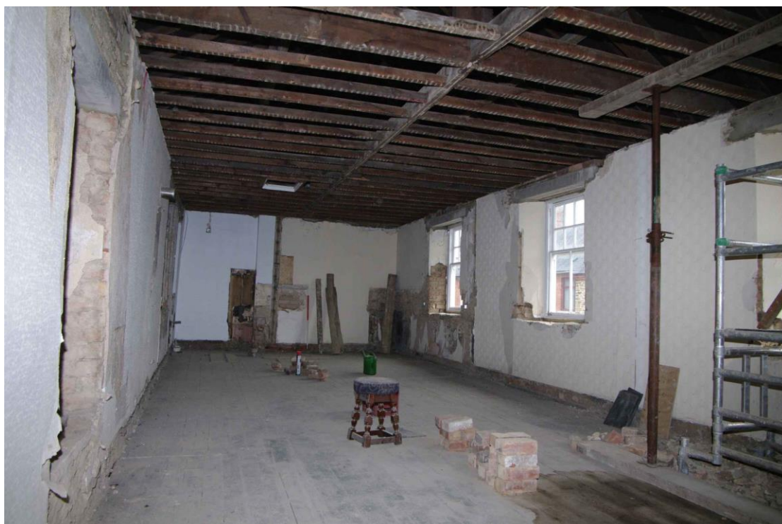
Figure 38 Room F3 Looking south-east. 1m scale
