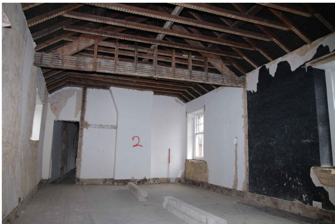
Figure 35 Room F2 Looking south-east. 1m scale
