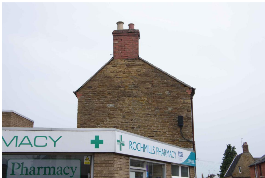
Figure 13 West facing elevation Looking east. Note trace of single storey gable end above the pharmacy building
