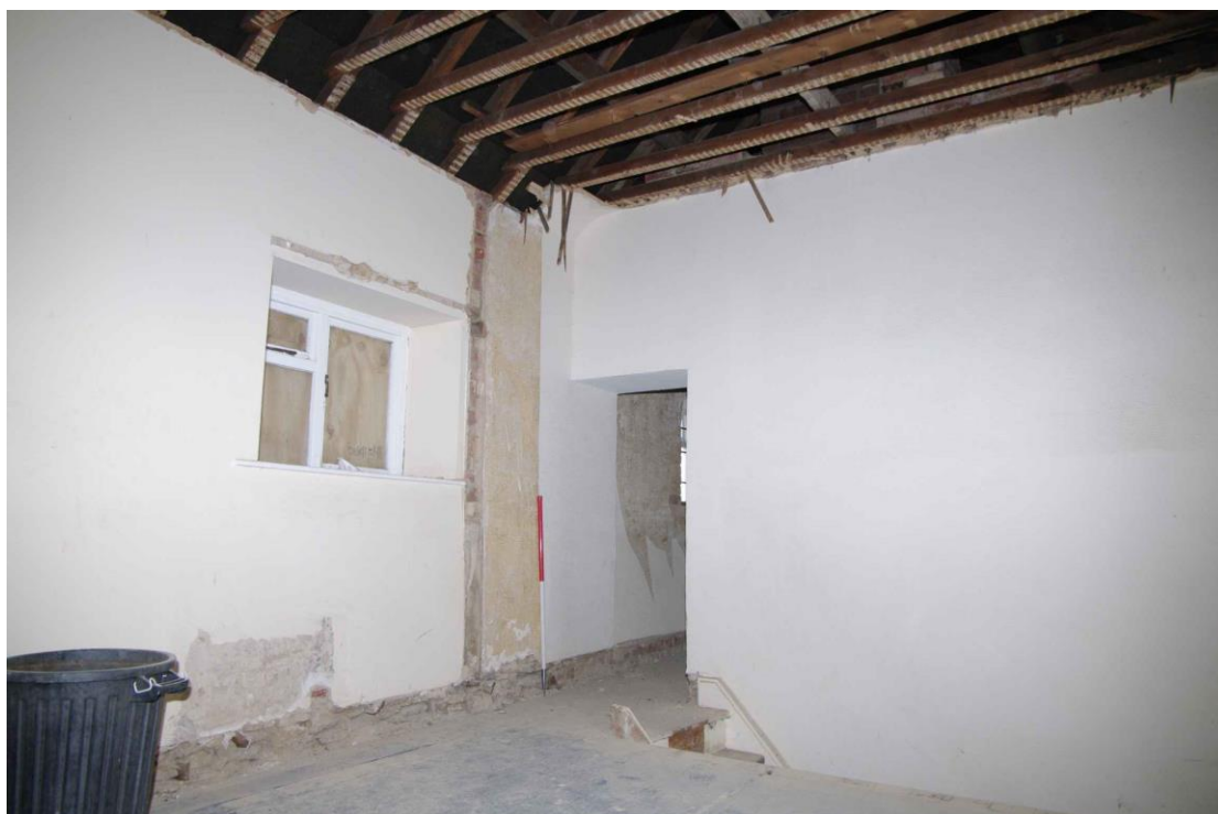
Figure 34 Room F1 Looking north-east. 1m scale
