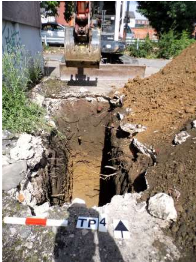
Figure 8 Test pit 4 fully excavated
