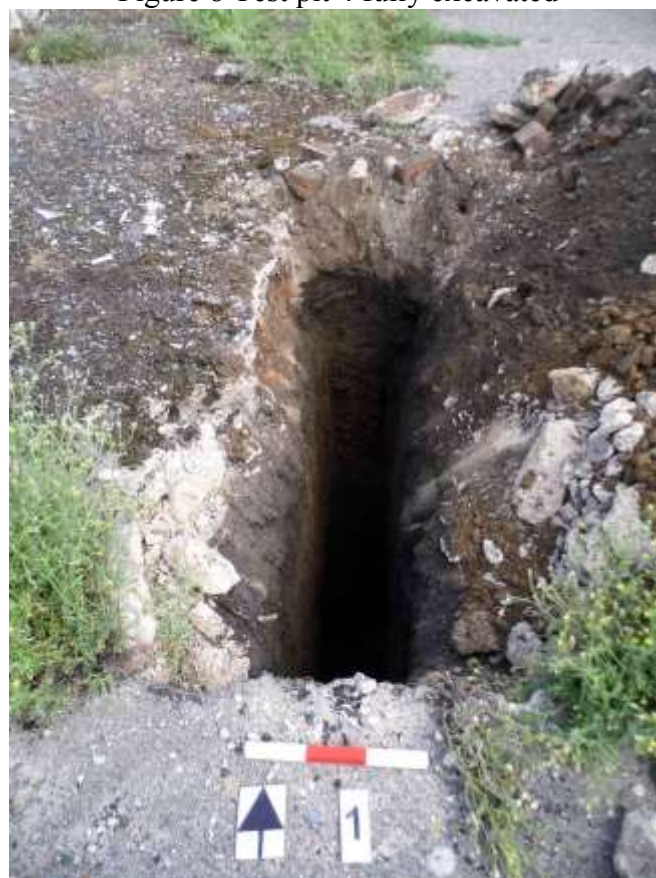
Figure 9 Soakaway pit 1 fully excavated
