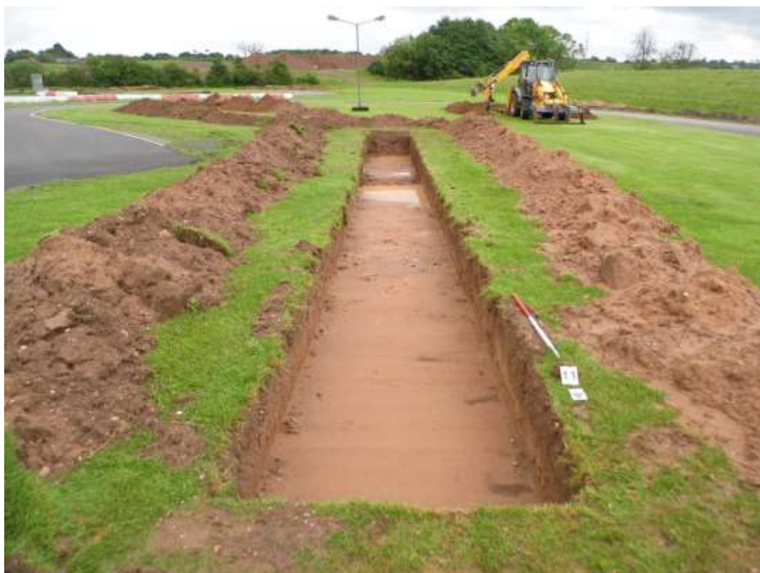
Figure 30: Trench 11, looking south
