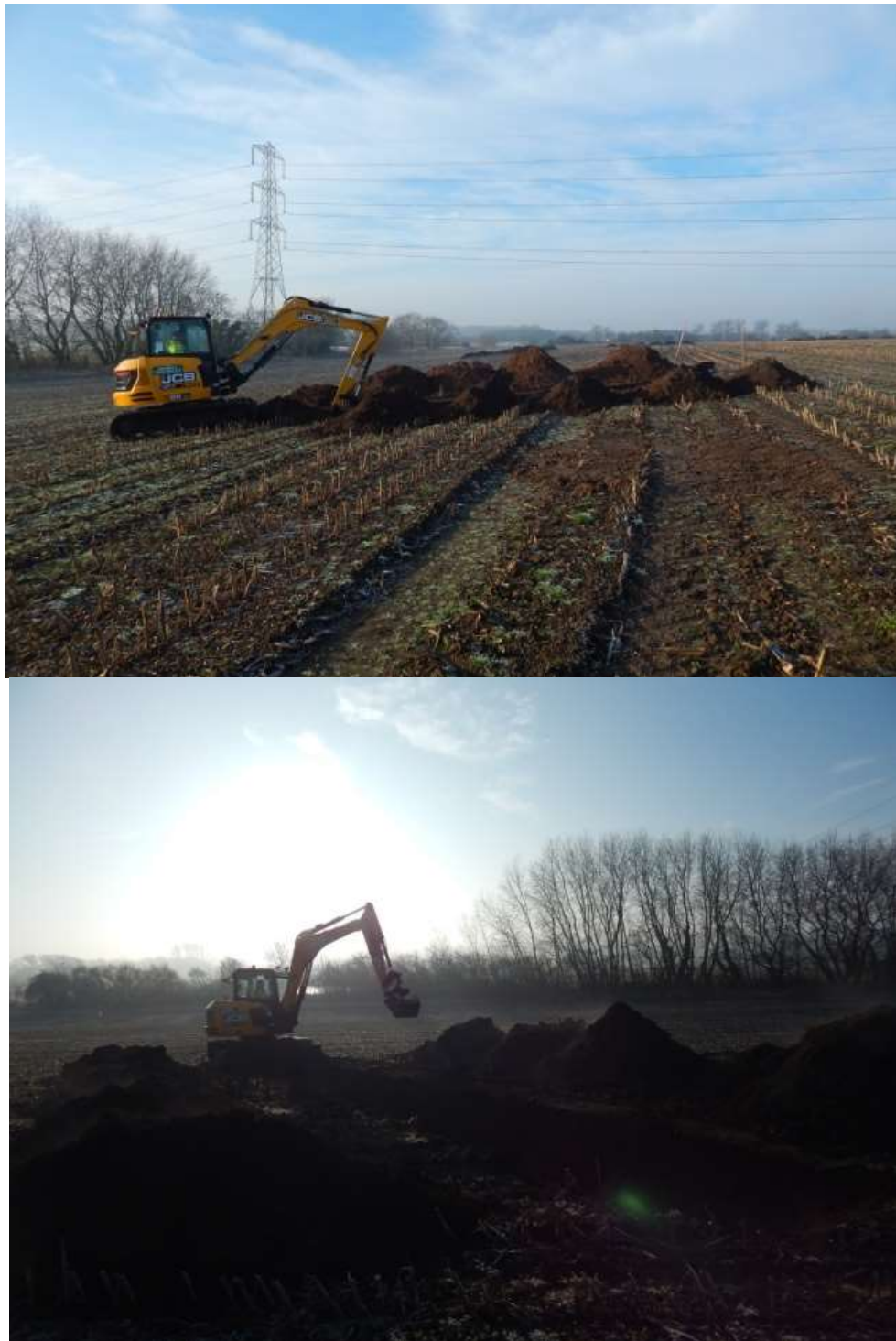
Figure 2: excavation of trenches in progress
