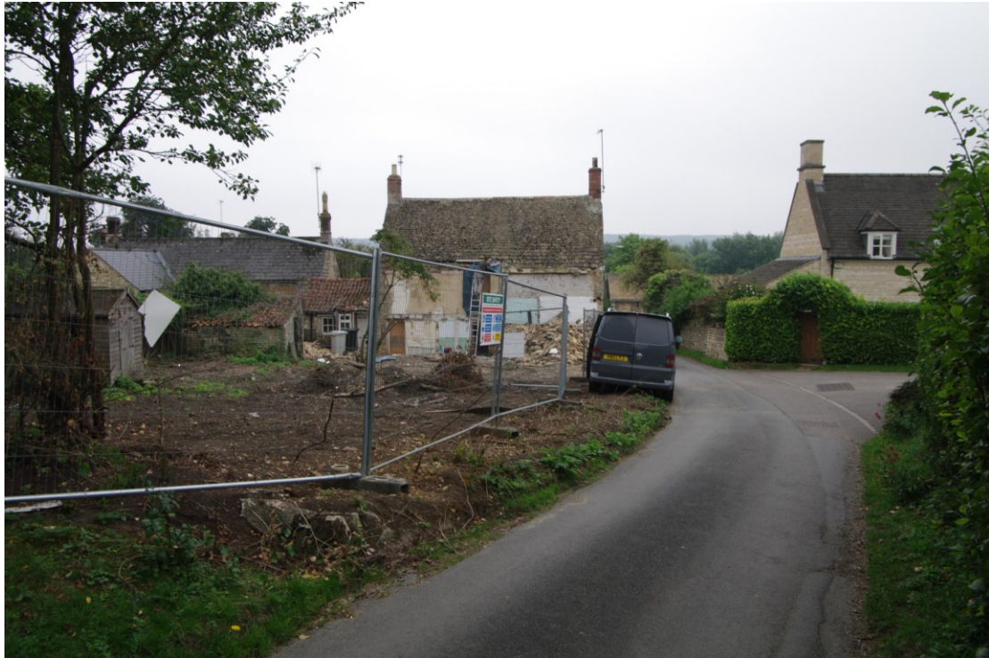
Figure 4: Rear garden of 2 Kings Lane Looking south down Kings Lane
