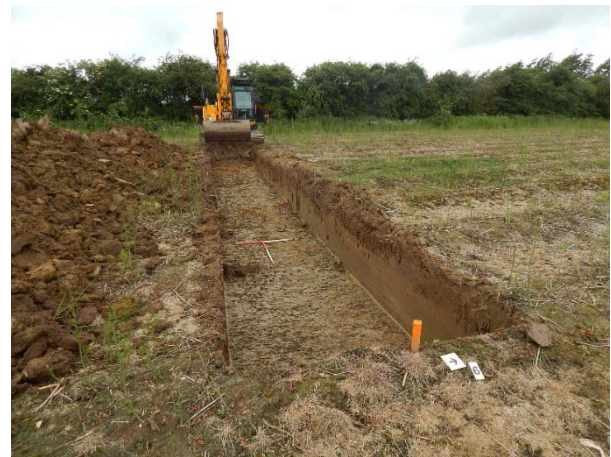
Figure 10: Trench 6 looking west
