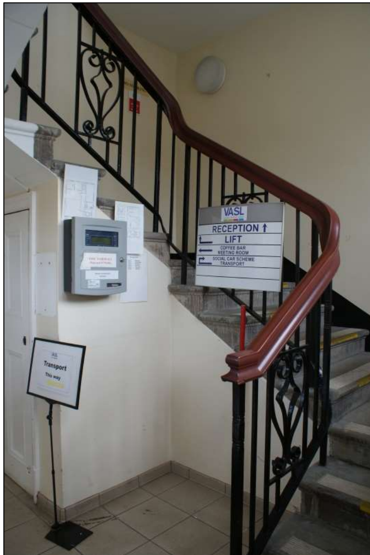
Figure 20: The entrance and stairwell with wrought iron balusters.
