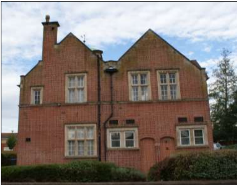
Figure 18: Photographs of the east facing elevation looking west with detail of the blocked doorways to the north
