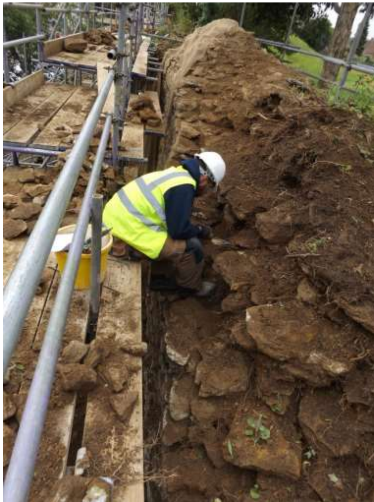
Plate 42: Work in progress of restoring curtain wall
