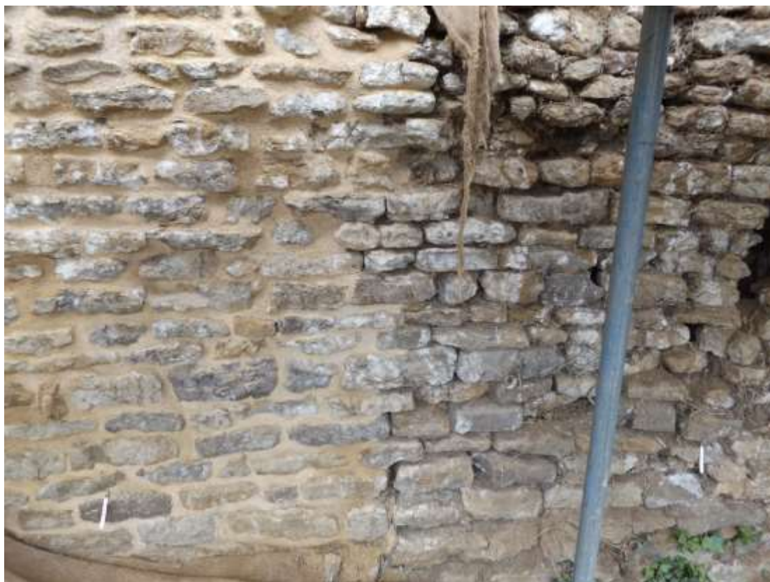
Plate 44: Section of wall showing before and after restoration
