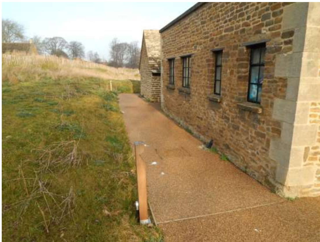
Plate 57: The new access path around the western side of the Great Hall, looking north
