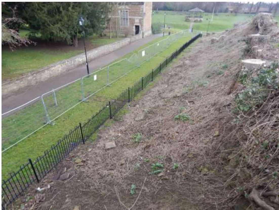
Plate 24: View of the completed perimeter fence, looking north from western rampart
