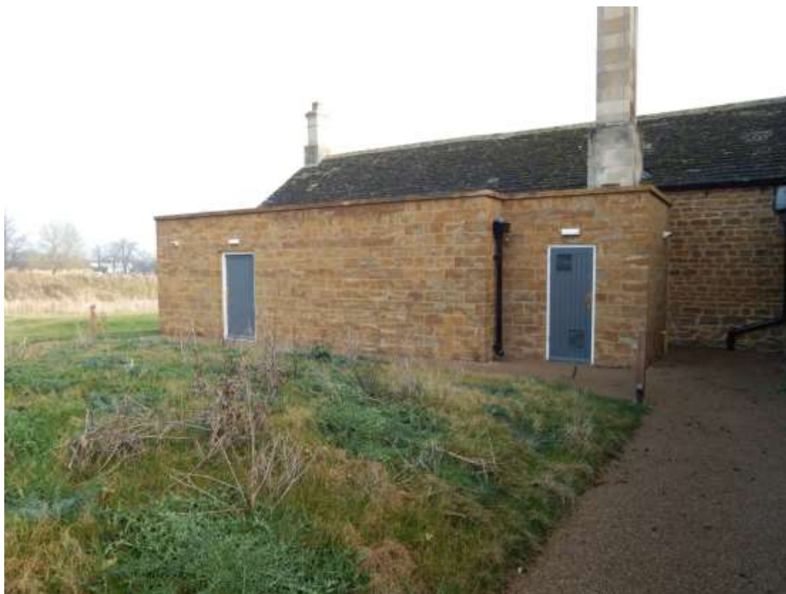
Plate 58: Completed new toilet block, looking east
