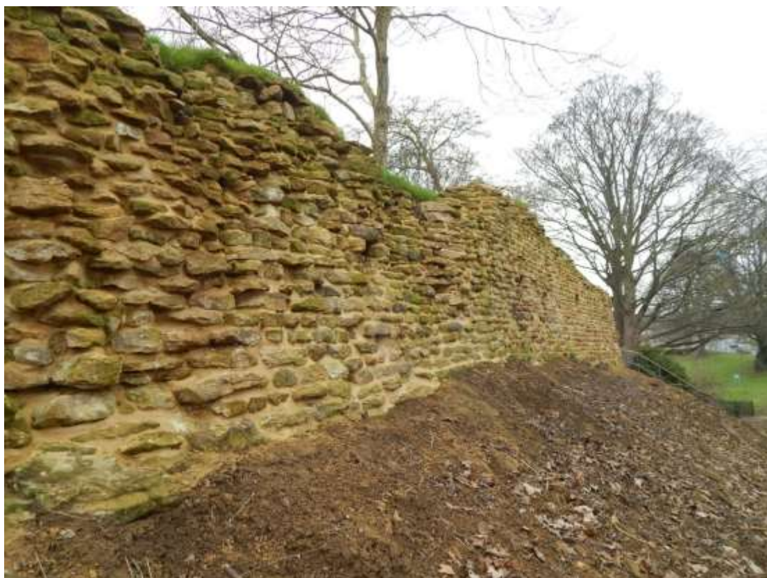
Plate 61: The restored east wall in 2017, looking north
