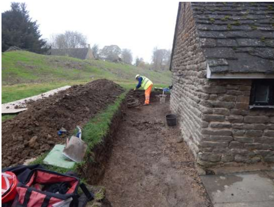
Plate 5: Work in progress on Test Pit 4- long section, looking north
