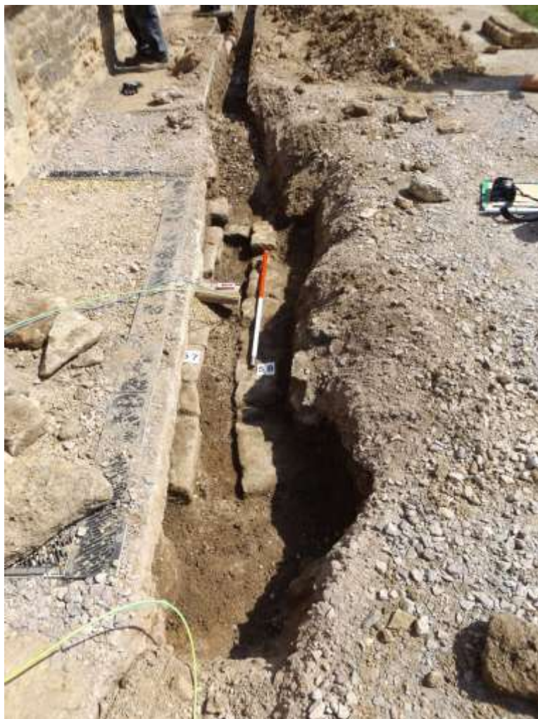
Plate 28: Stone drain in electrical trench, looking east
