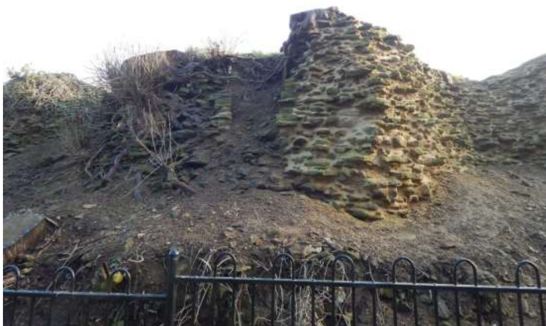
Plate 62: The restored postern gate in 2017, looking east
