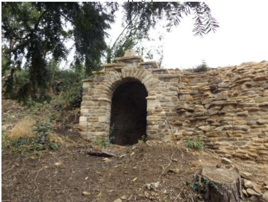
Plate 47: The restored grotto feature, looking west
