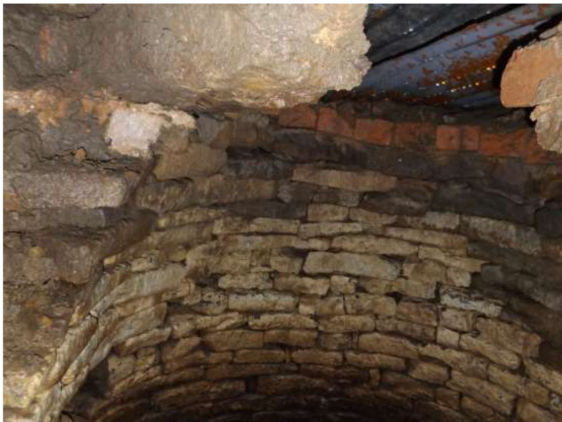
Plate 30: Internal shot of well, cap in place
