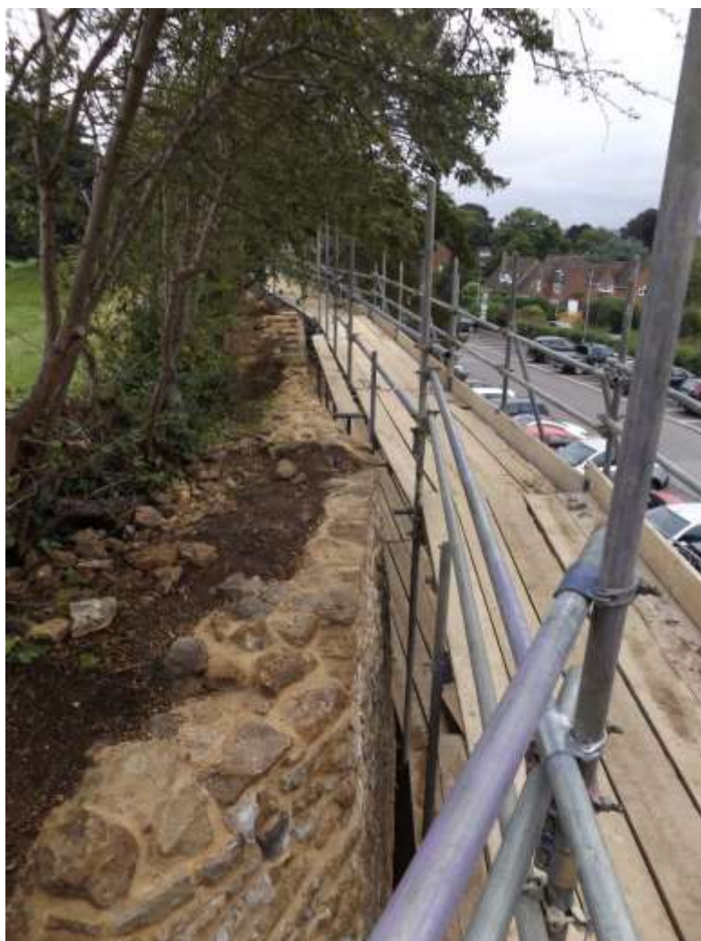
Plate 43: General shot of east side of walls, showing scaffolding, looking north
