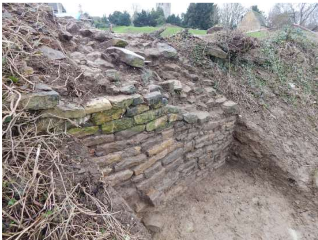
Plate 59: The curtain wall in the evaluation trench, looking south-west
