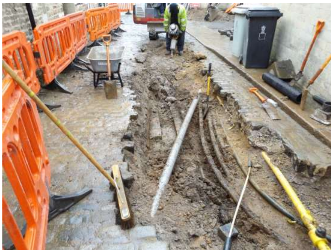
Plate 29: Work in progress Castle Lane, looking south
