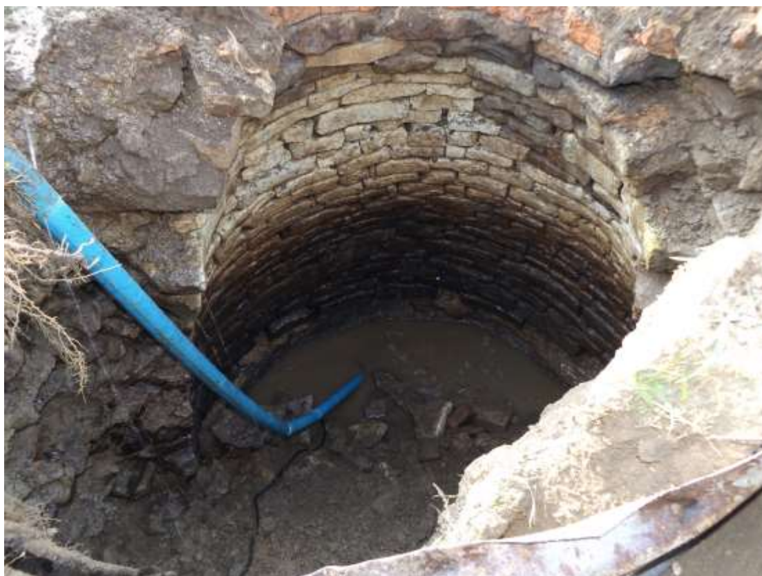
Plate 32: Well with cap removed and being pumped out
