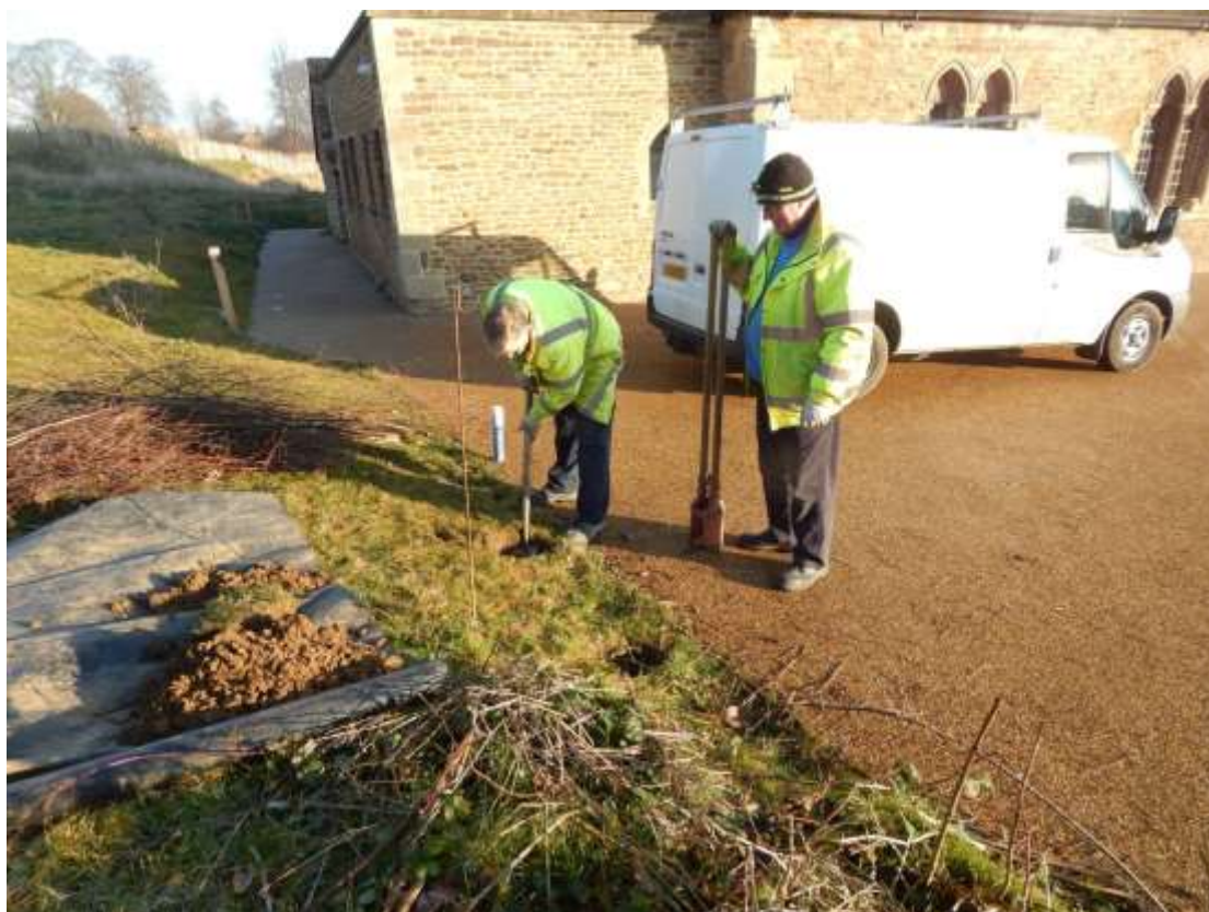
Plate 50: Work in progress on interpretation board holes
