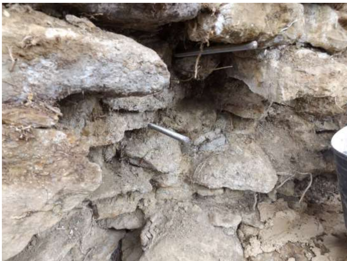
Plate 45: Metal pins inserted into wall structure for strength
