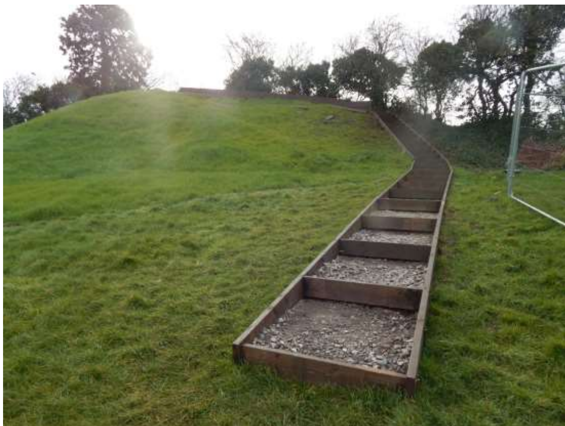
Plate 26: Steps to Motte partially constructed, looking east
