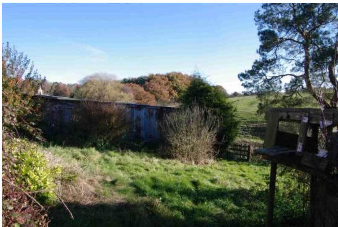
Figure 27: Shed 6 west facing elevation Looking south-east
