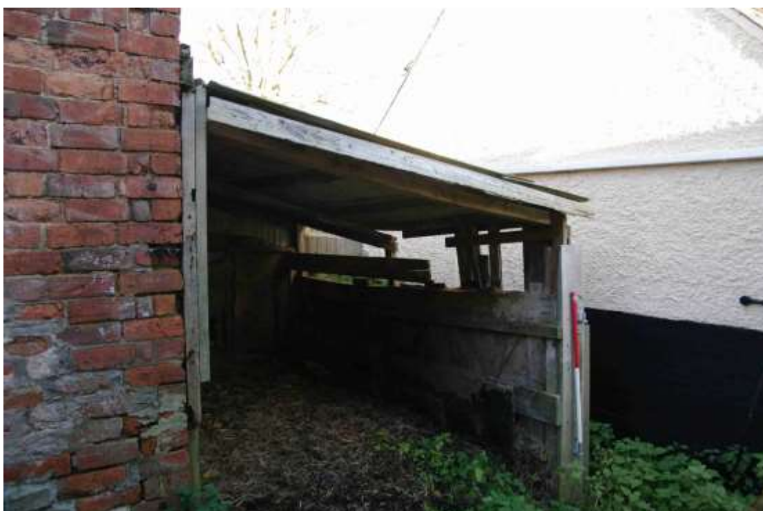
Figure 24: Shed 5 south facing elevation Looking north-east. 1m scale
