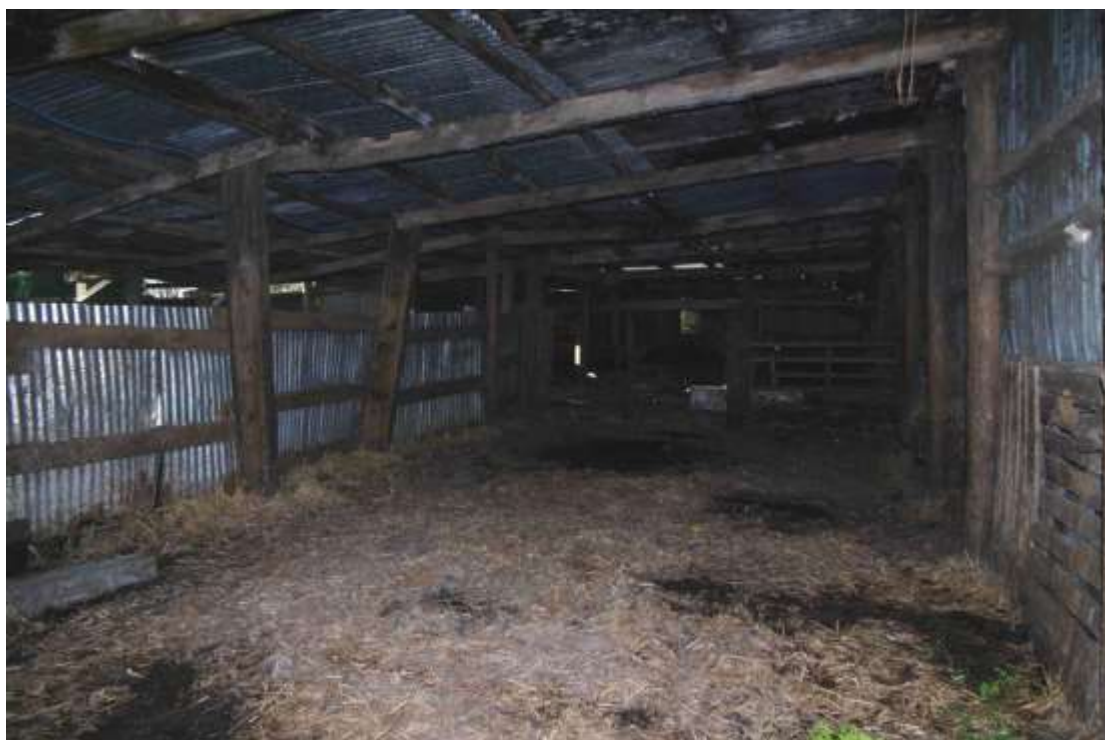
Figure 29: Shed 6, inside Looking west
