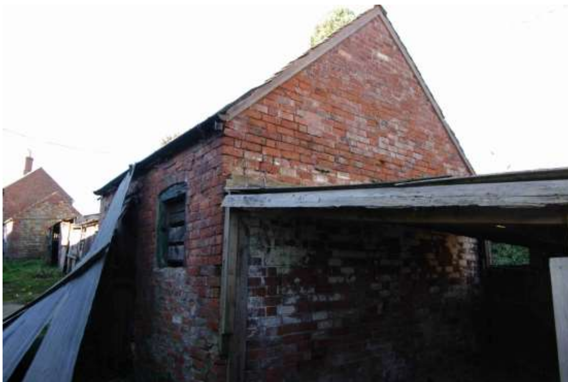
Figure 22: Shed 4 south and east facing elevations Looking north-west. Shed 5 on right
