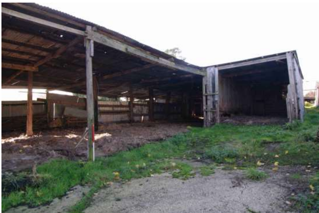
Figure 25: Shed 6 north facing elevation Looking south-west. 1m scale
