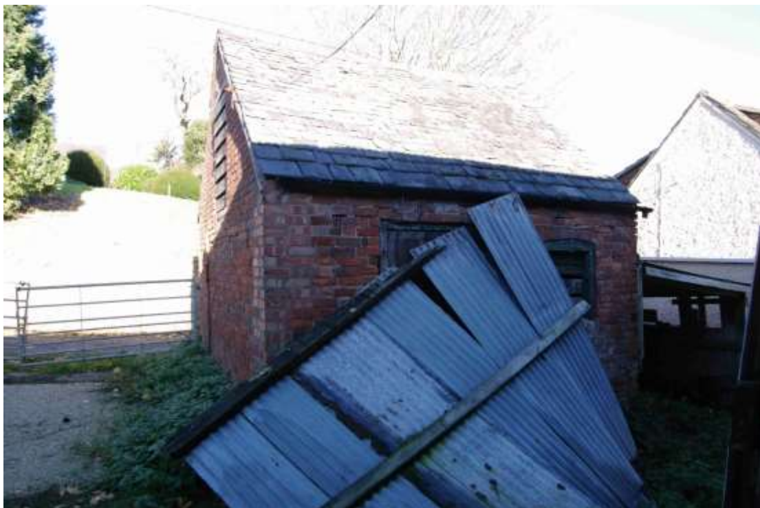
Figure 21: Shed 4 south facing elevation Looking north-east
