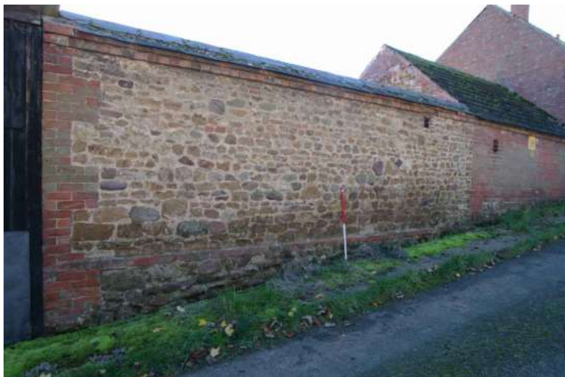
Figure 11: Shed 1 north facing elevation Looking south-west. 1m scale
