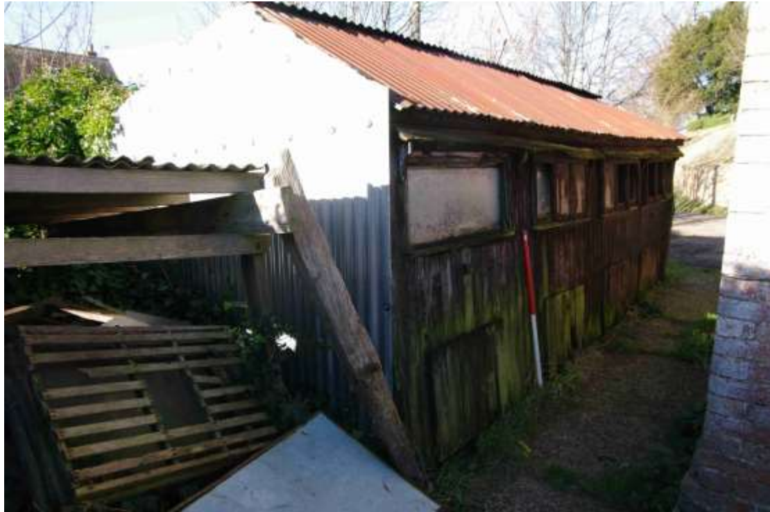
Figure 31: S34hed 7 south and east facing elevations Looking north-west. 1m scale
