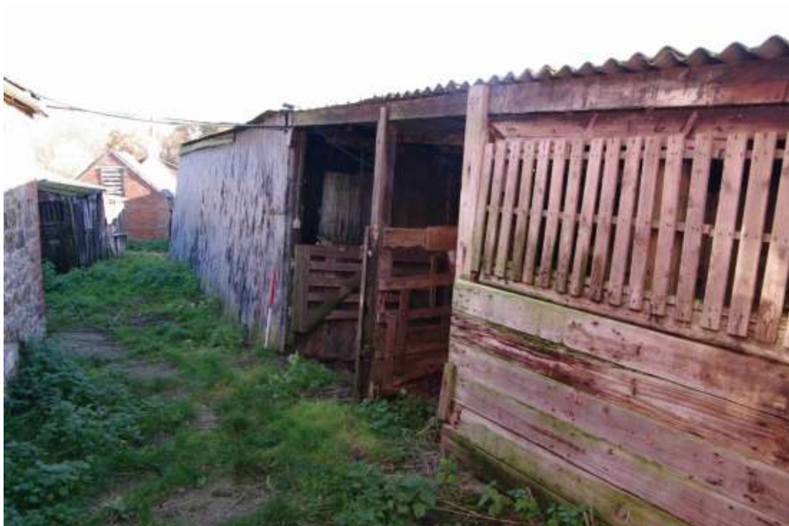
Figure 26: Shed 6 north-west corner Looking south-east. 1m scale
