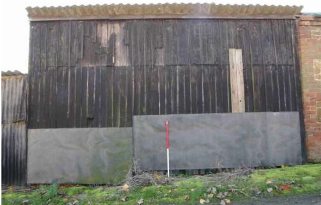
Figure 15: Shed 2 north facing elevation Looking south. 1m scale
