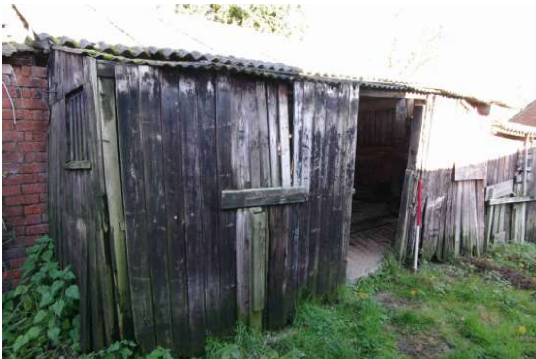
Figure 13: Shed 2 South facing elevation Looking north-east. 1m scale. Shed 3 on right
