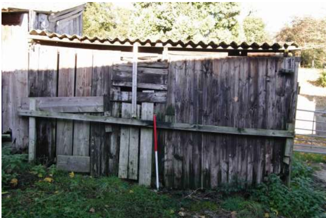
Figure 17: Shed 3 south facing elevation Looking north. 1m scale
