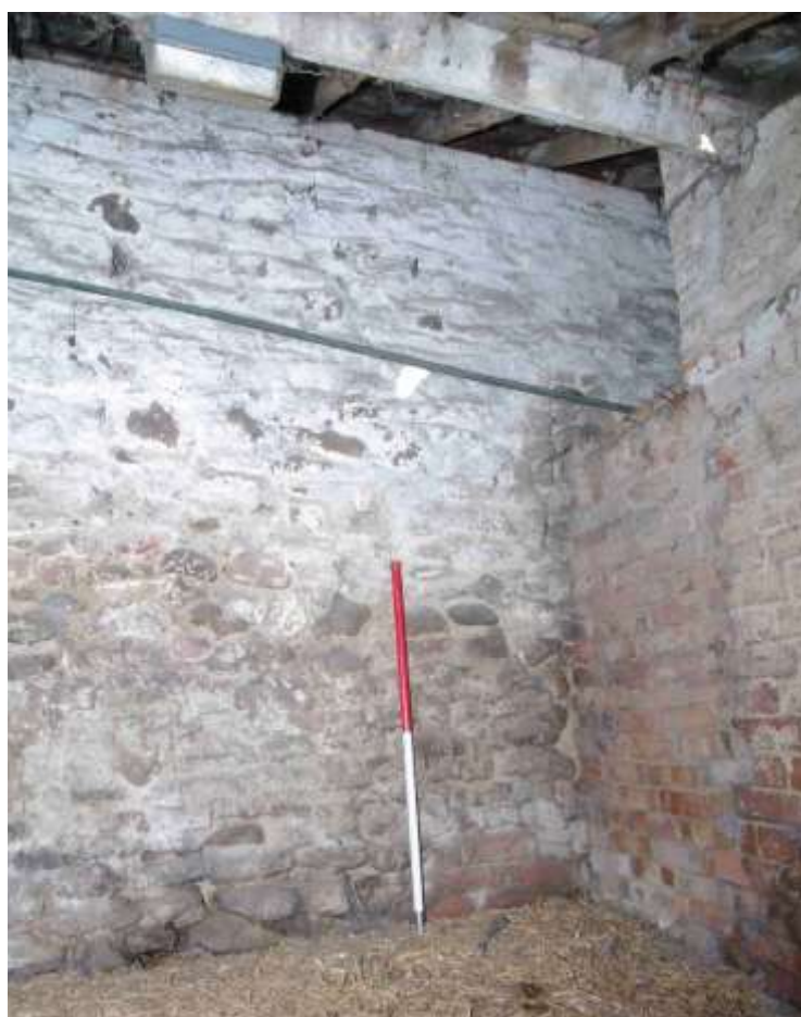
Figure 12: Shed 1, inside Looking north-east in middle sty. 1m scale
