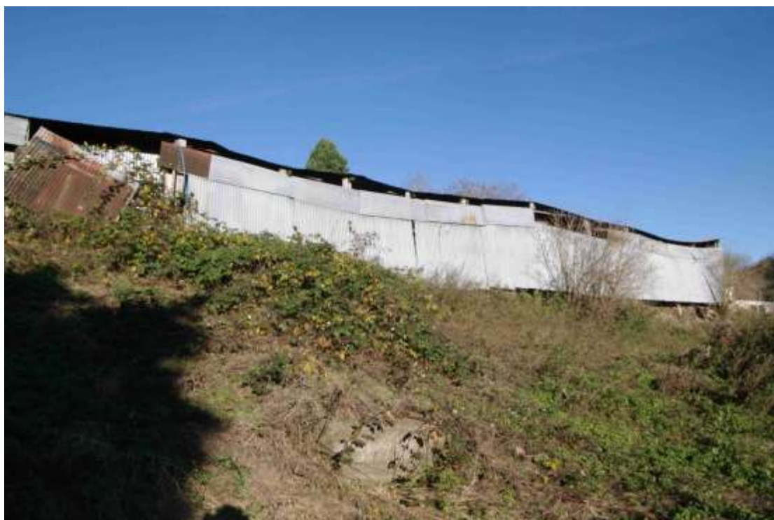
Figure 28: Shed 6 south facing elevation Looking north-east
