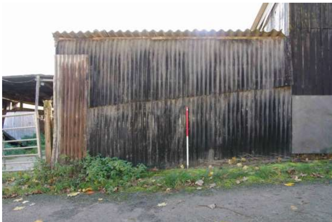
Figure 19: Shed 3 north facing elevation Looking south. 1m scale
