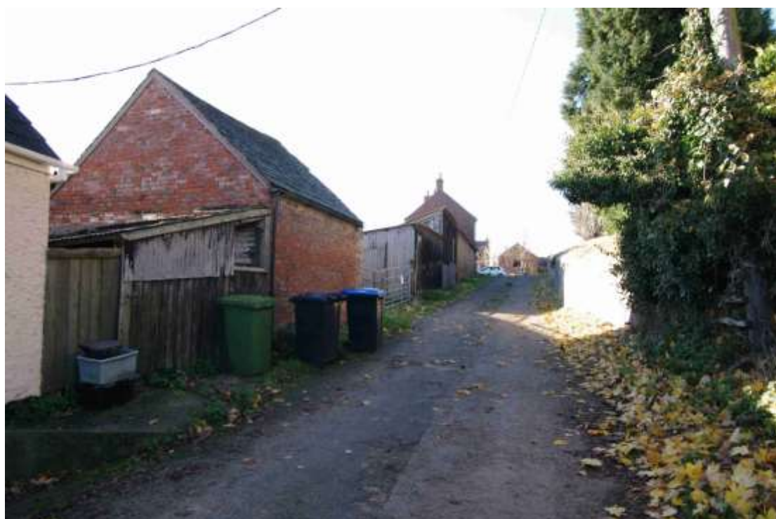
Figure 6: Buildings seen from Church Lane Looking south-west. The chimney and gable end belong to Ashby House Farmhouse. Shed 5 behind green bin, Shed 4 behind black bins, Sheds 1-3 beyond gate
