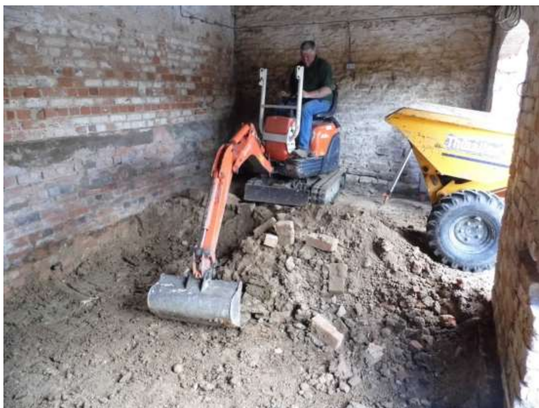
Figure 30: Work in progress inside former tack room, looking south
