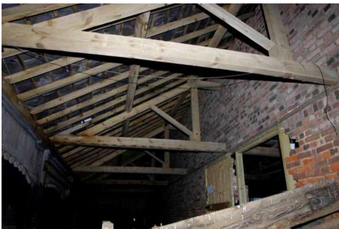
Figure 28 East range roof structure Looking north east
