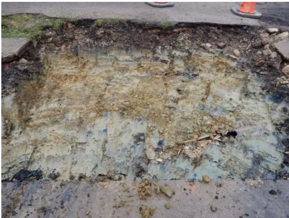
Figure 34: The trench excavated to the top of the clay, looking south-east
