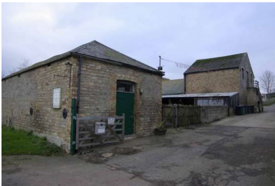
Figure 8 Courtyard buildings seen from entrance Looking north east
