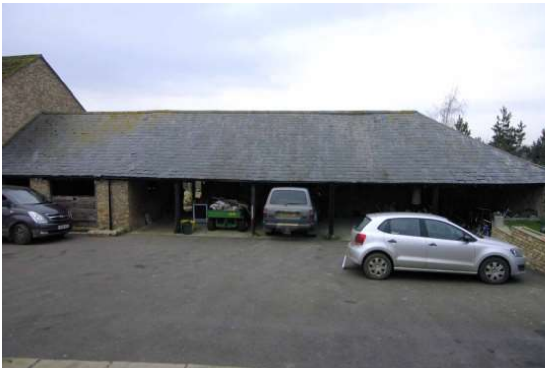
Figure 25 East facing elevation. Cart shed Looking north west. 1m scale
