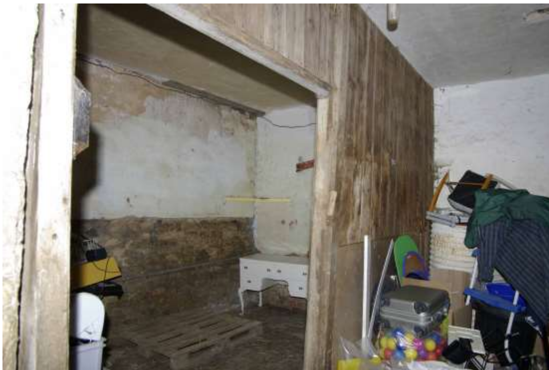
Figure 22 Hayloft building, ground floor, eastern room Looking south west
