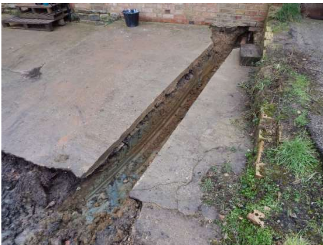
Figure 32: The drain leading from the tack room, looking east
