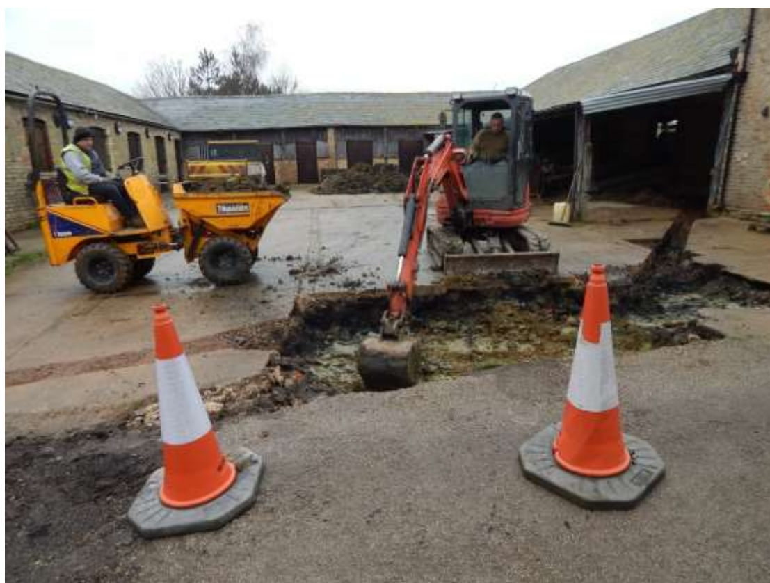
Figure 33: Work in progress on septic tank trench
