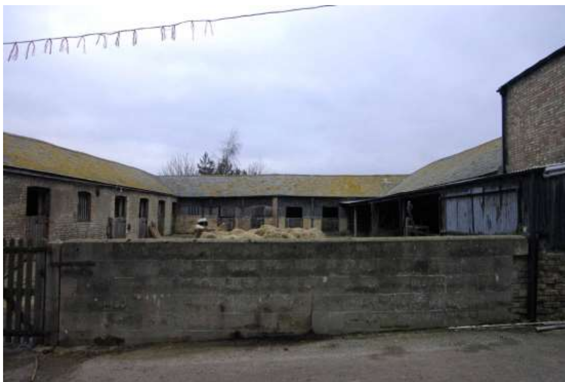
Figure 11 Main courtyard Looking north east
