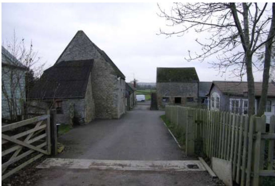
Figure 10 Courtyard and listed buildings Looking west
