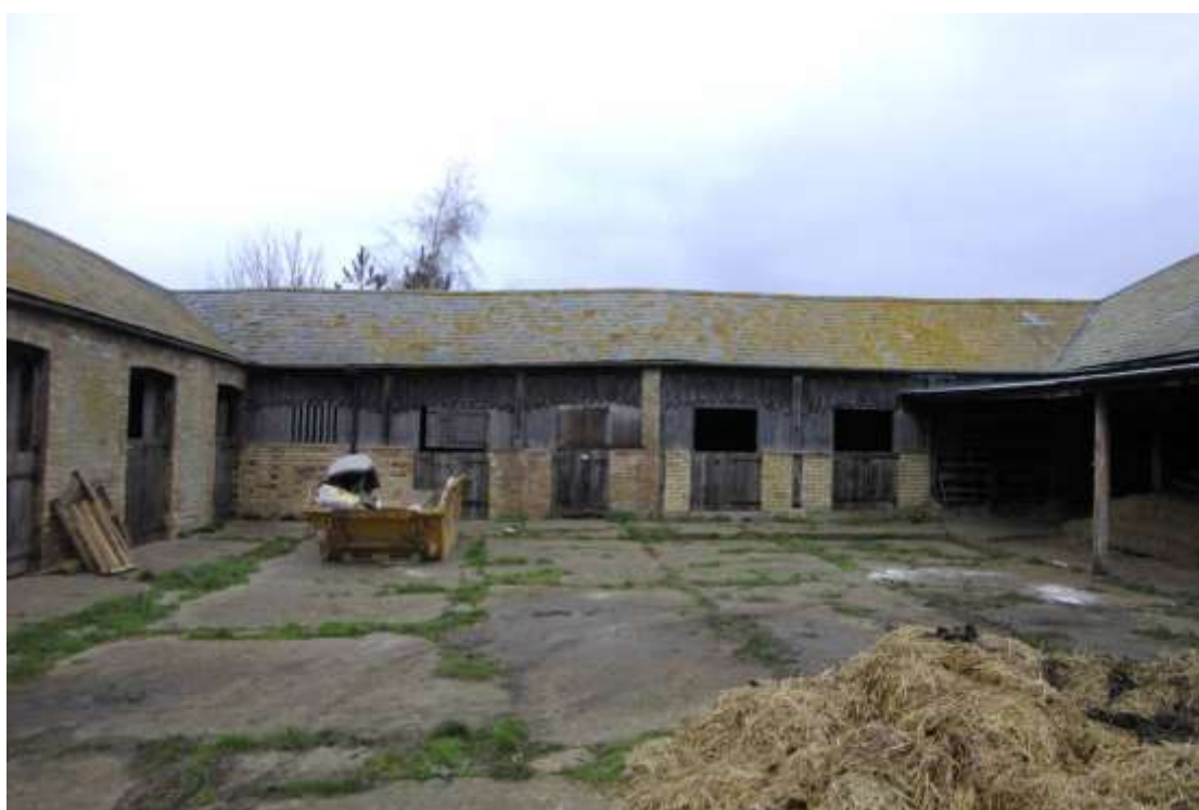
Figure 13 Main courtyard, north range Looking north east
