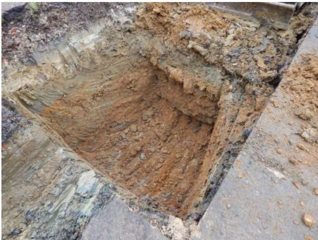
Figure 35: The trench excavated to full depth, looking south-west
