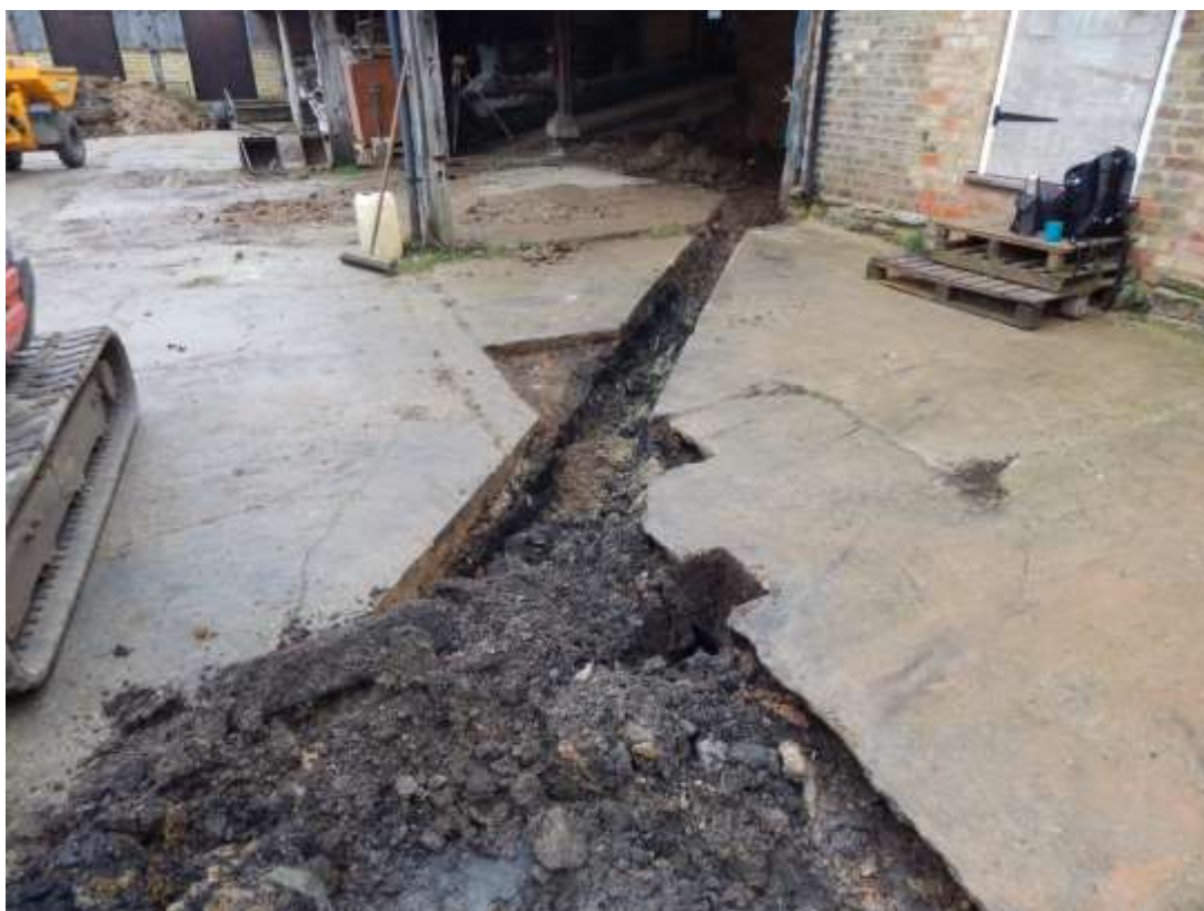
Figure 31: The drain leading from the former cart shed, looking east
