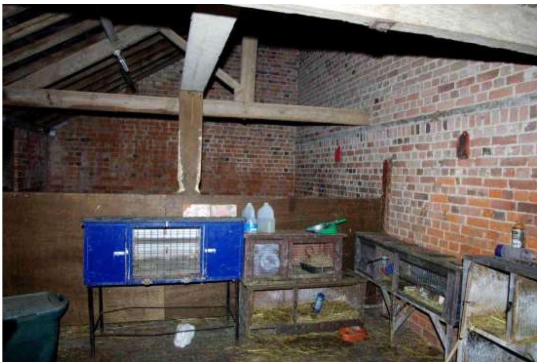
Figure 27 Internal view of added building under cart shed Looking south west
