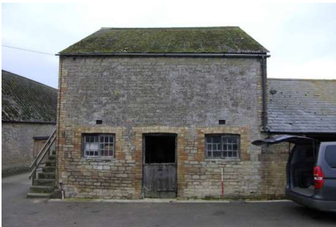
Figure 16 East facing elevation of hayloft building Looking north west. 1m scale
