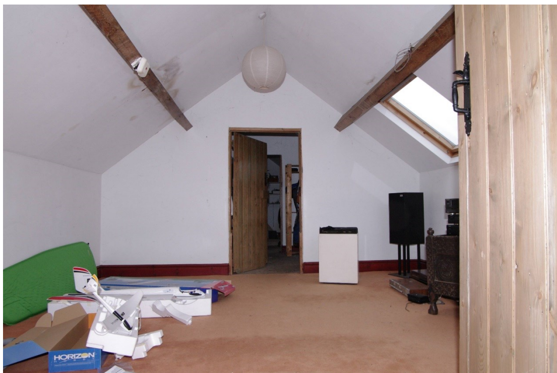
Figure 30 North range building, first floor Looking east
