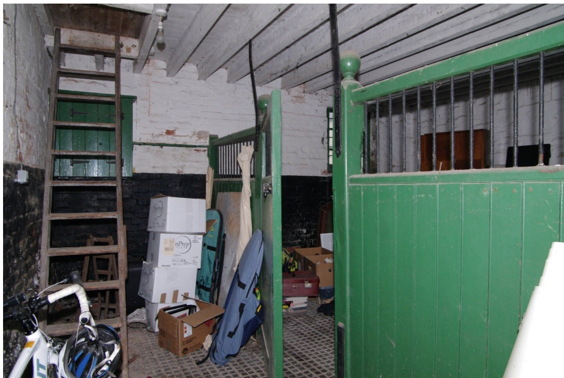
Figure 28 North range ground floor, east end room Looking north-east
