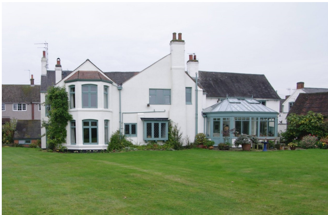
Figure 38 The White House, south facing elevation Looking north
