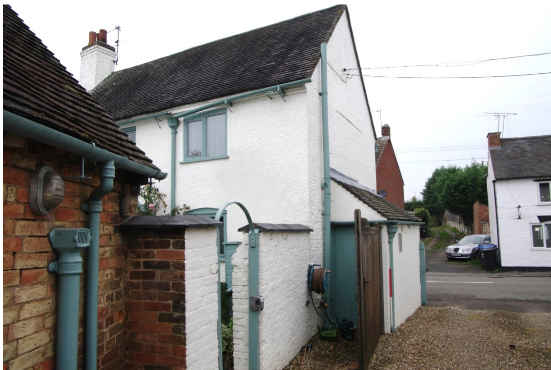
Figure 8 Lean-to which is to be demolished Looking north. 1m scale.
