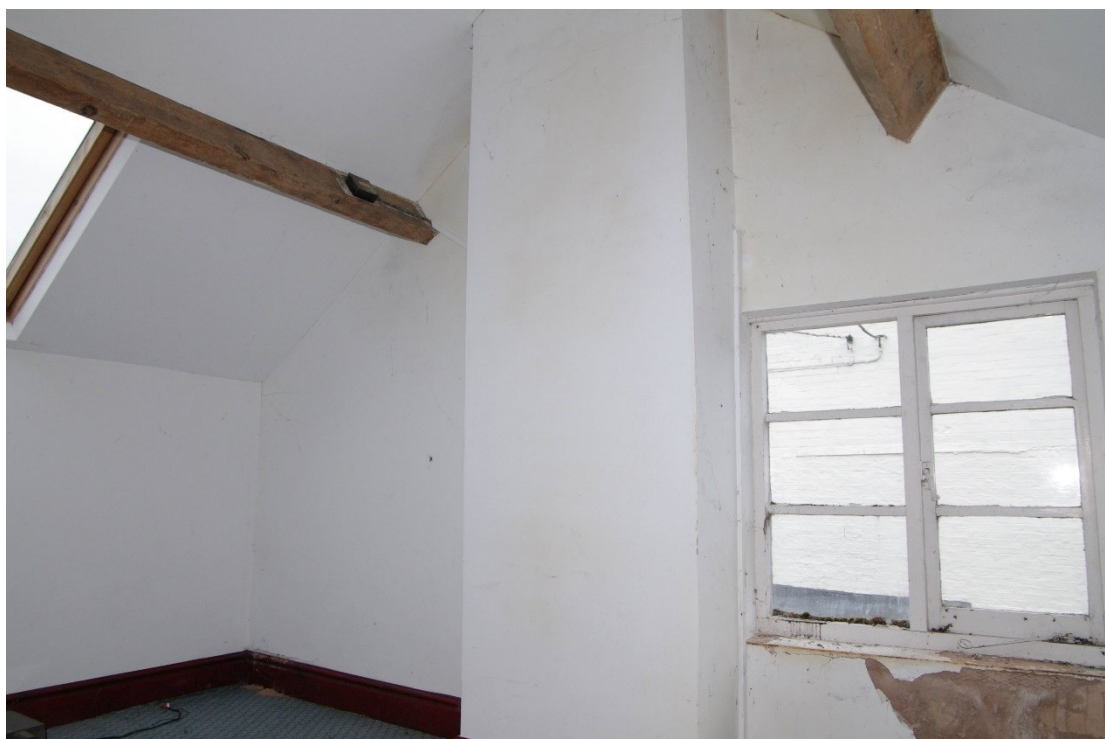
Figure 29 North range building, first floor, west room Looking south-west
