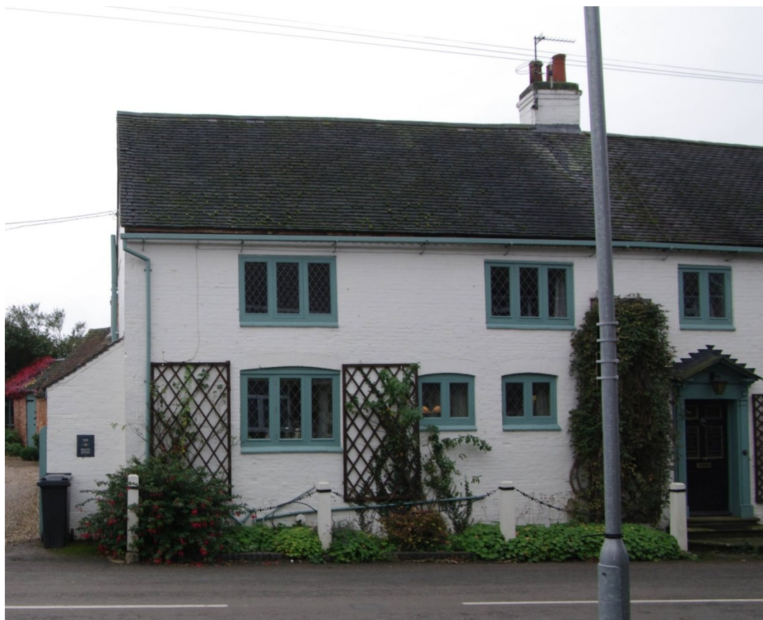
Figure 36 Eastern end of The White House north facing elevation Looking south
