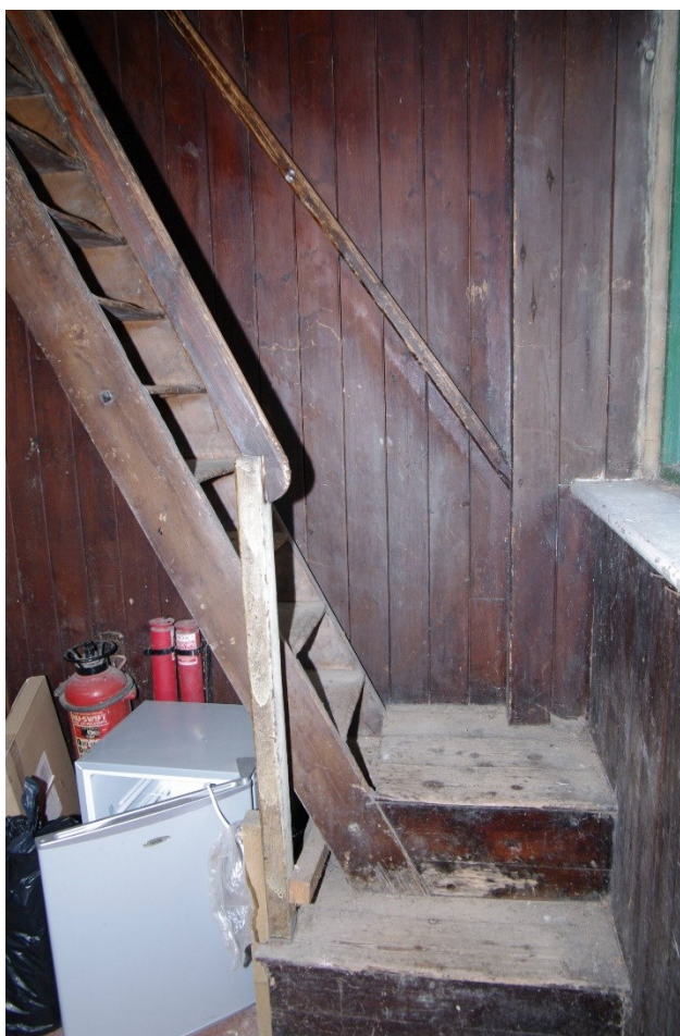
Figure 26 North range ground floor, west end room stairs Looking east
