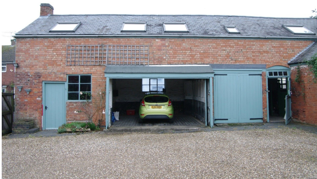
Figure 24 North range, south facing elevation Looking north. 1m scale
