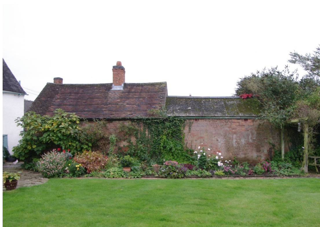
Figure 14 Outbuildings, west facing elevation Looking east
