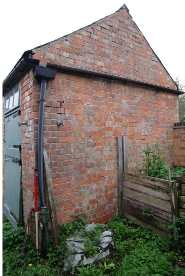
Figure 33 East range, south facing gable end Looking north-east. 1m scale
