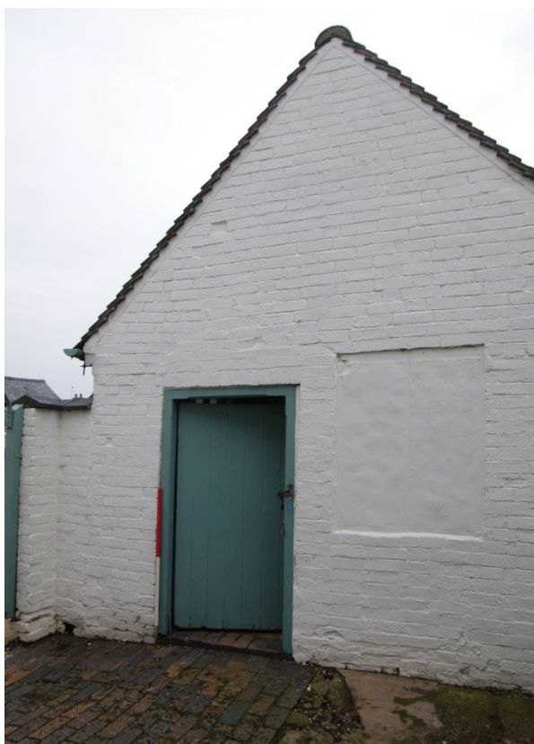
Figure 15 Outbuildings, north facing elevation Looking south. 1m scale
