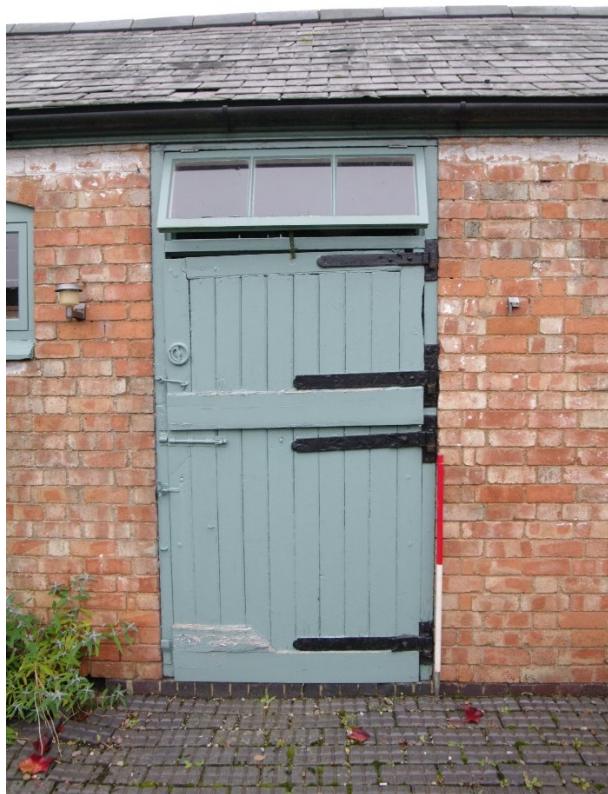
Figure 32 East range, west facing elevation door detail Looking east. 1m scale
