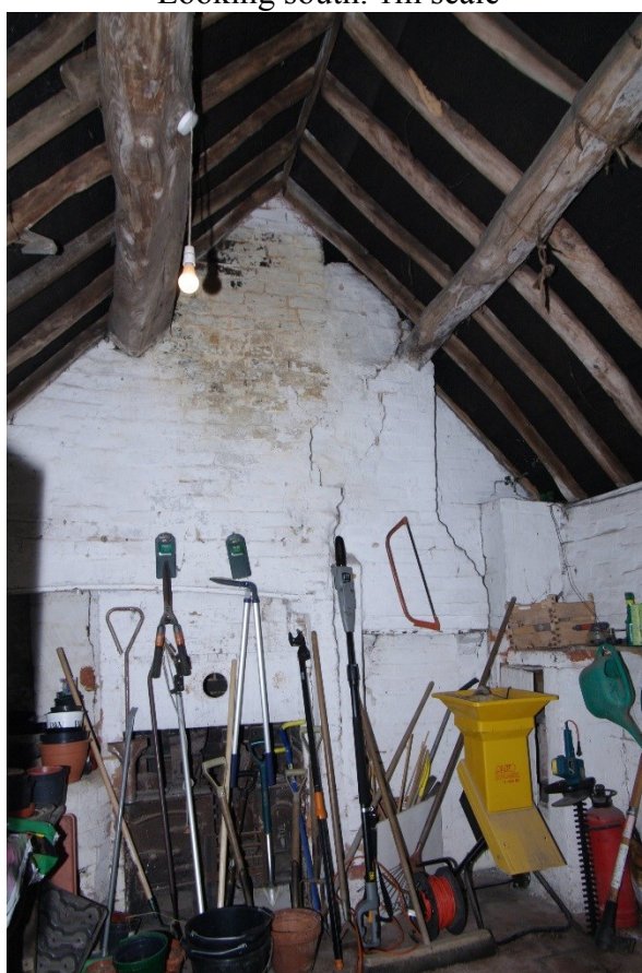
Figure 16 Inside northern end of northern outbuilding Looking south
