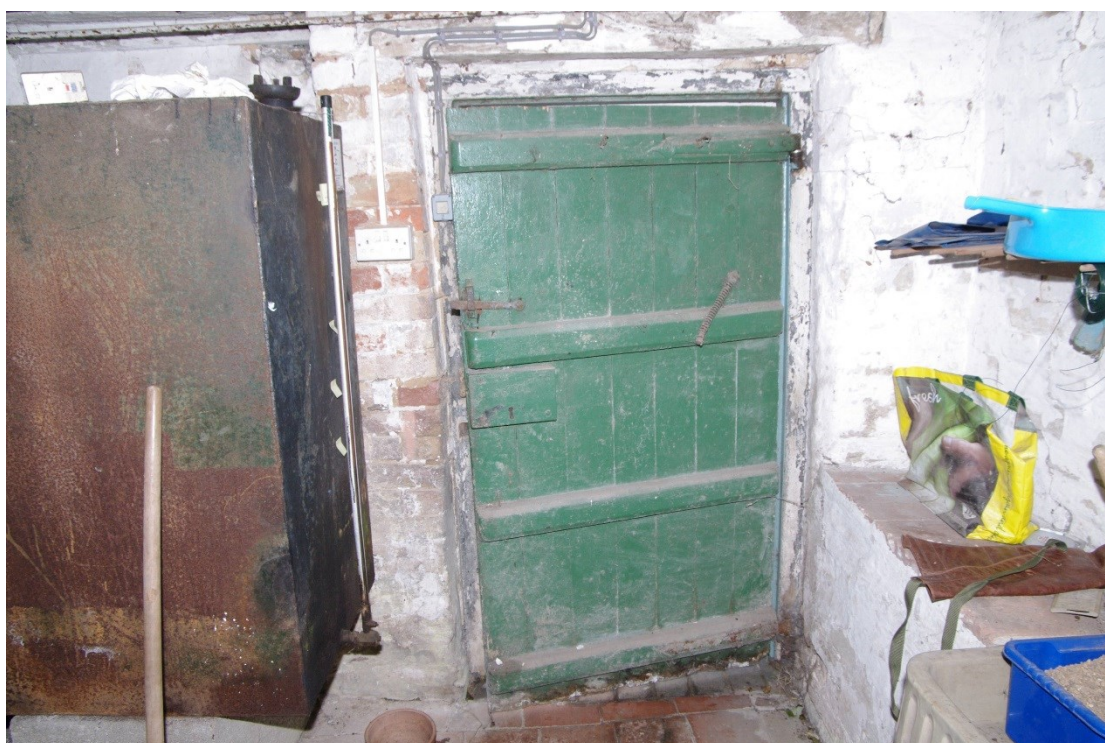
Figure 18 Outbuildings northern room, door detail Looking north
