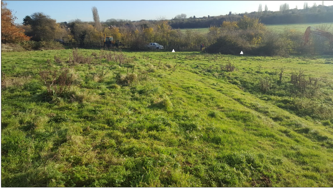
Figure 4: The site area prior to groundworks, looking east towards Melton Mowbray. Earthworks are visible beyond in the foreground. The plot (staked out, triangle markers) is in front of the contractors.
