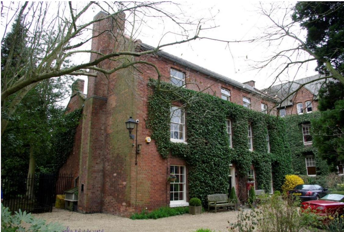
Figure 4. School House west and south facing elevation elevations. Looking north-east
