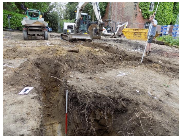
d. Site under excavation showing bioturbation
