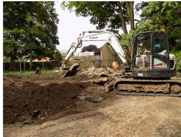
b. Removal of tree roots
