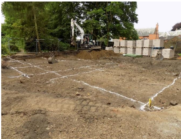
c. Foundations to be excavated for new building (facing South)
