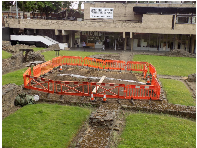
c. Preservation works in progress
