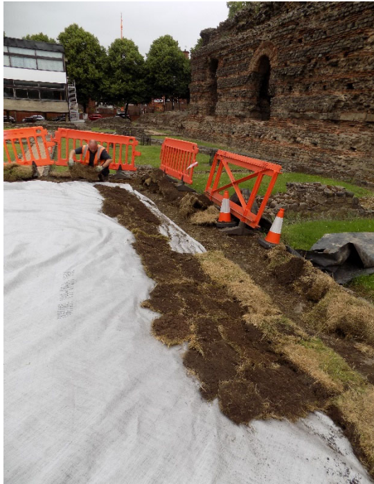
a. Preservation in situ of floor: covering with terram for protection
