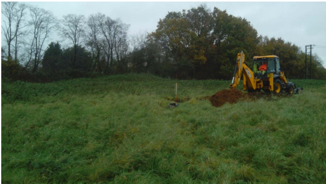
Figure 6: Trench excavation in progress
