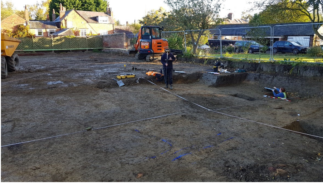
Figure 4: General view northeast across excavation area
